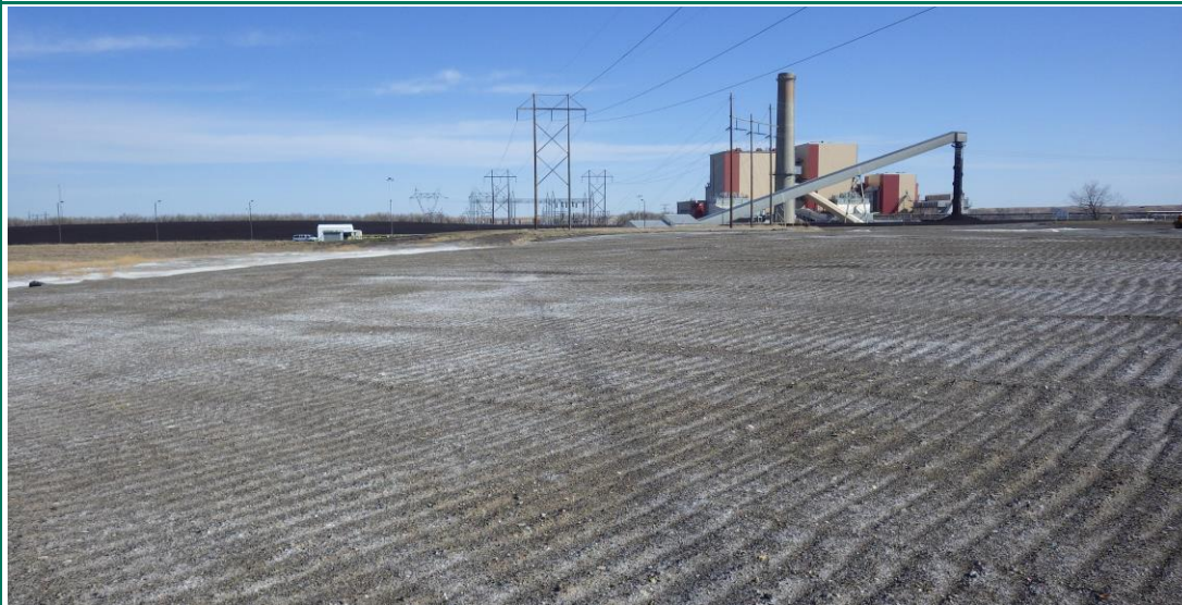
Photograph 11 Recently placed and graded bottom ash (IMGP2237.JPG)
