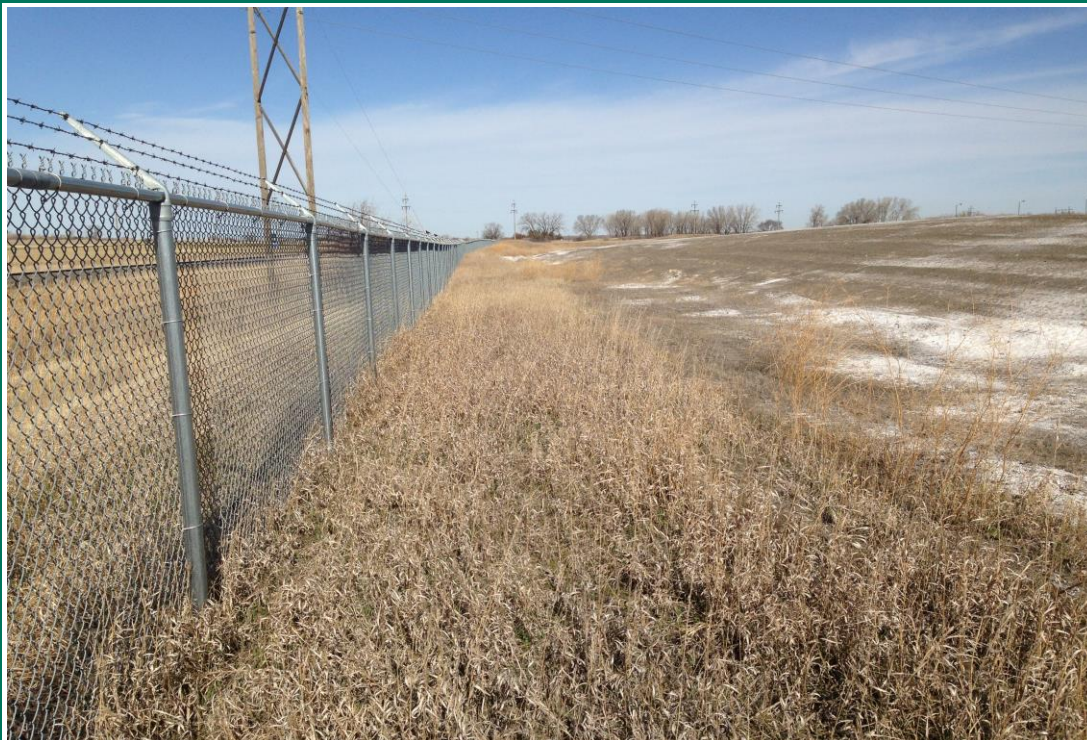
Photograph 4 South crest (contact water channel not well defined) (IMG_3719.JPG)
