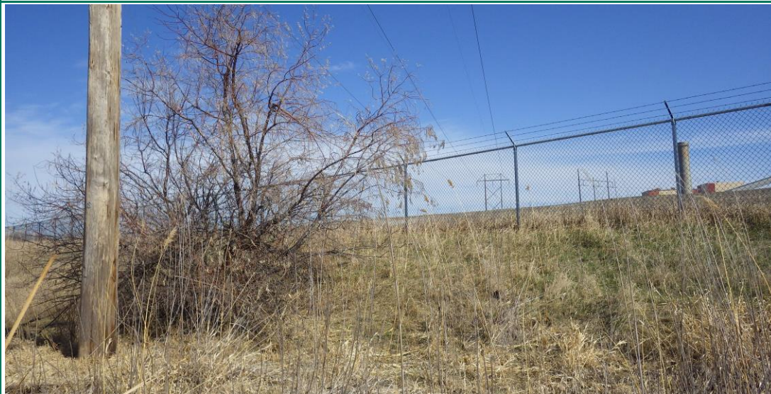
Photograph 17 Tree at toe of south exterior slope (IMGP2252.JPG)
