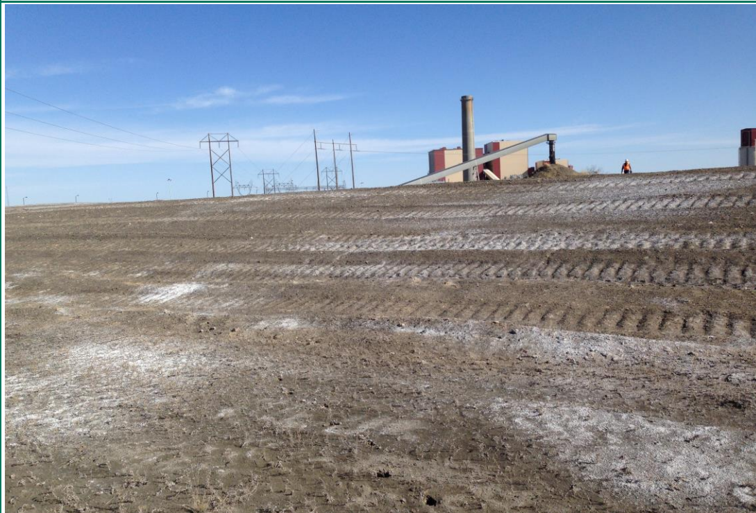
Photograph 5 CCR slope on south side (15 and 25% slope, approximately 10' tall) (IMG_3721.JPG)
