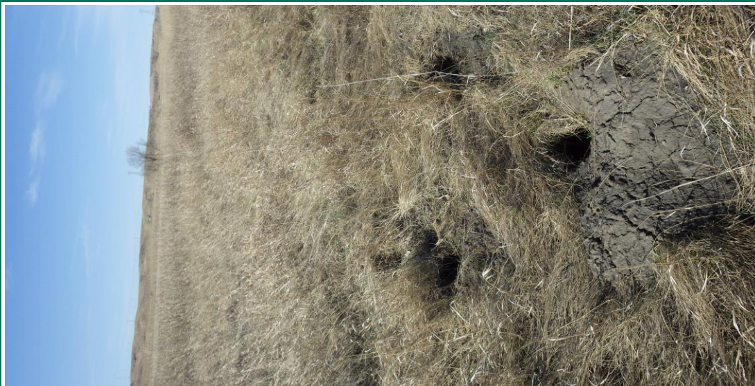
Photograph 14 Animal burrows on northwest exterior slope (IMGP2247.JPG)
