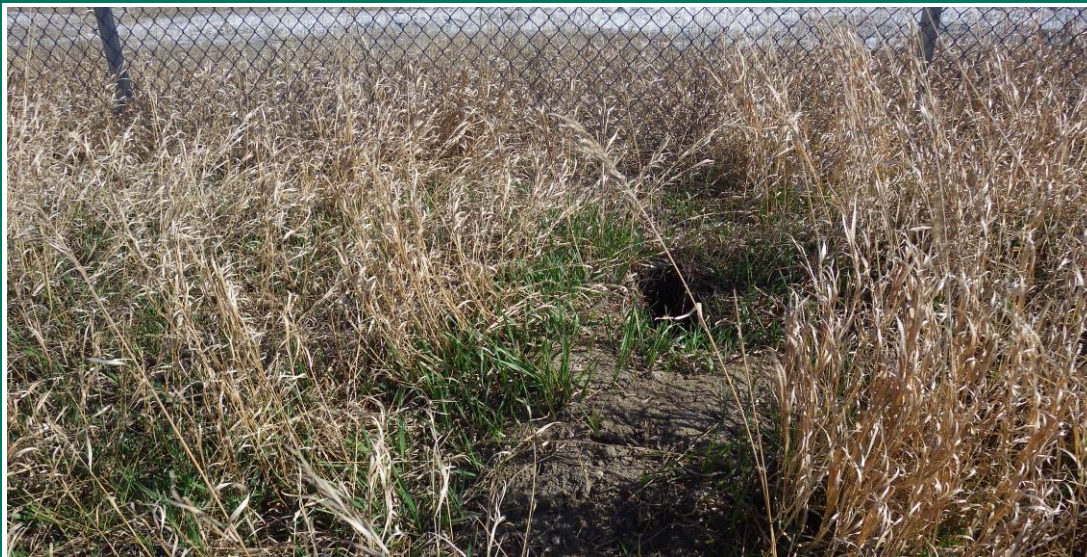
Photograph 18 Grassy vegetation and animal burrows on south exterior slope (IMGP2253.JPG)
