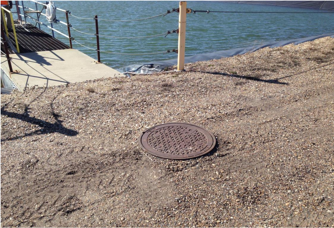
Photograph 21 - Center Cell Manhole for center cell outflow (IMG_3669.JPG)
