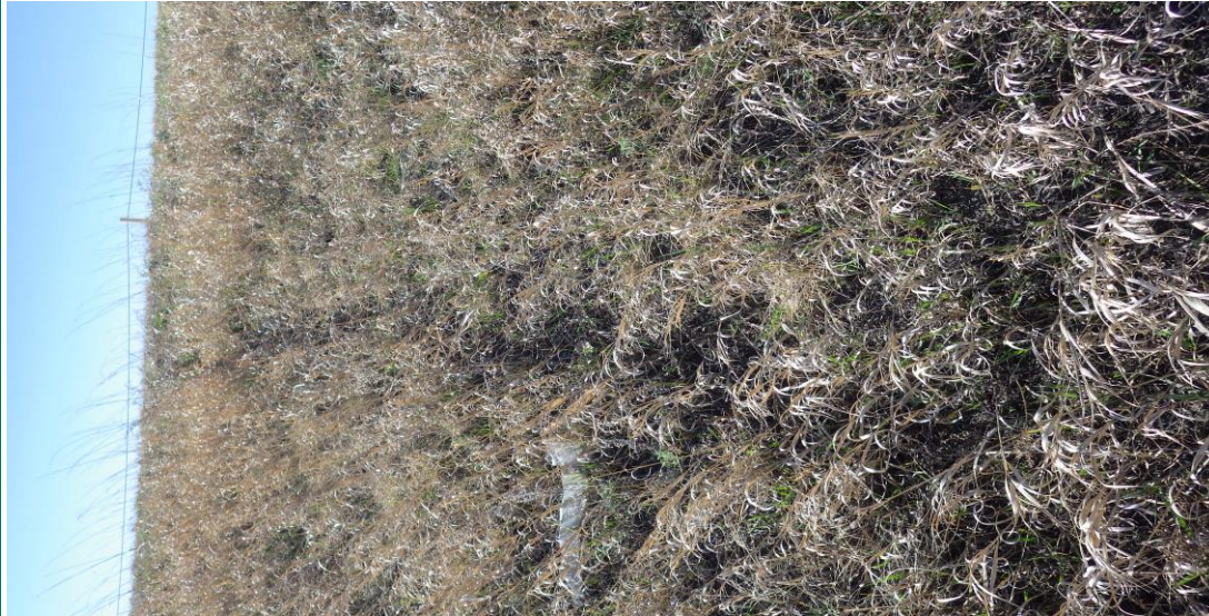
Photograph 26 - South Cell Erosion rills on the east downstream slope (IMG2183.JPG)
