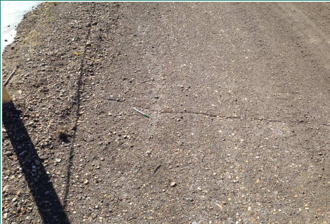
Photograph 8 - North Cell Small crack along crest (west end of north side) (IMG_3637.JPG)
