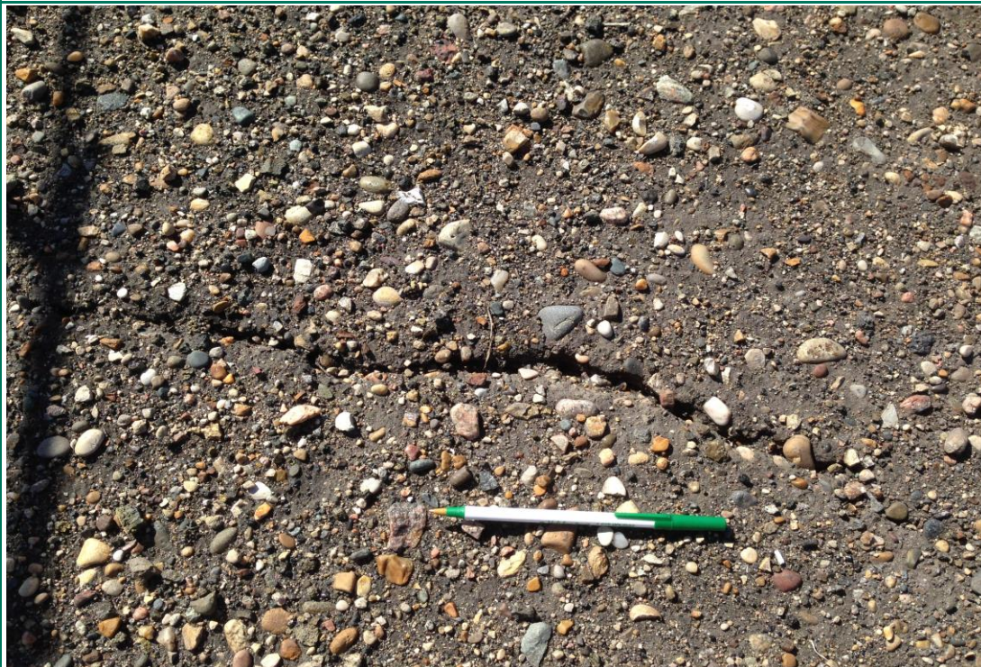
Photograph 7 - North Cell Small crack along crest (center of north side) (IMG_3635.JPG)
