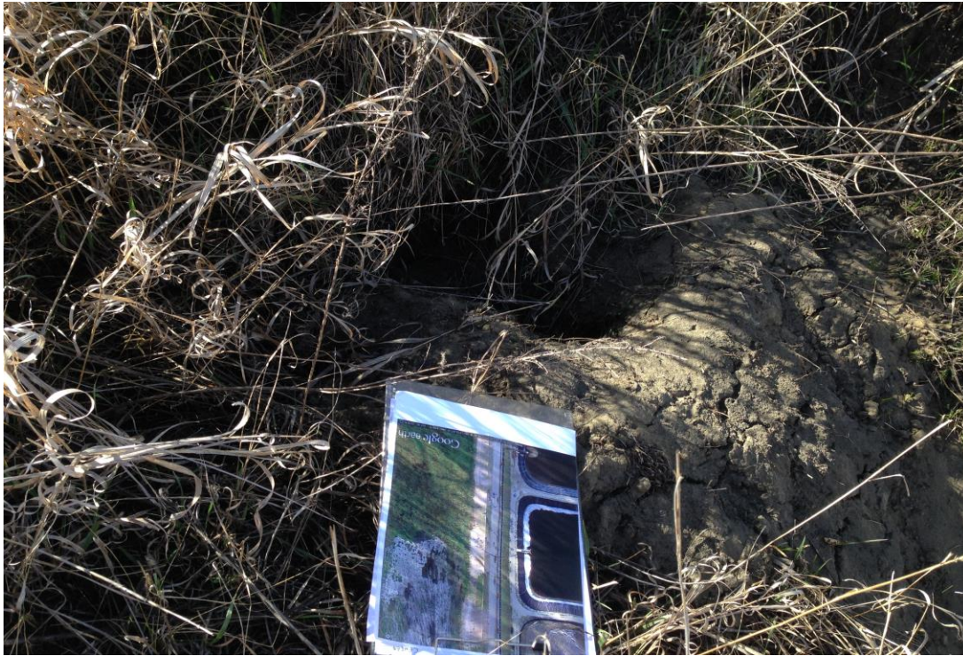
Photograph 23 - Center Cell Small animal burrow at the toe of the east downstream slope (IMG_3675.JPG)
