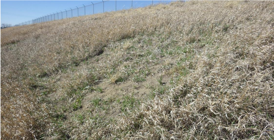
Photograph 28 - South Cell Bare spot on south downstream slope (IMGP2191.JPG)
