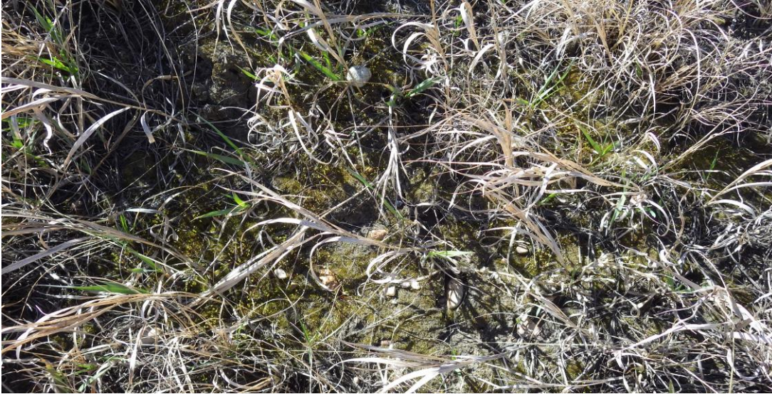
Photograph 27 - South Cell Mossy vegetation on the east downstream slope (no seepage observed) (IMGP2184.JPG)
