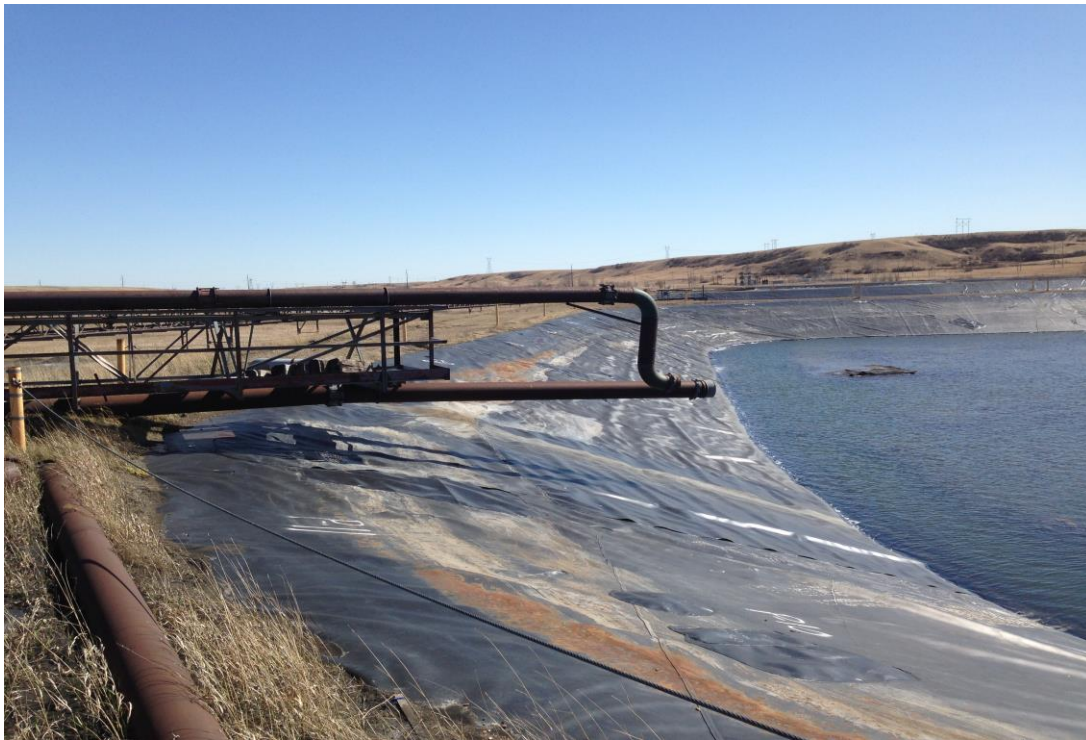
Photograph 6 - North Cell Bottom ash inlet piping and trestle (IMG_3633.JPG)
