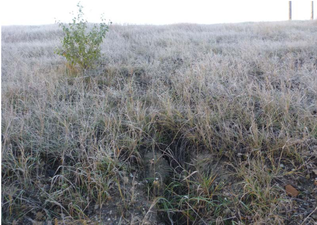
Photograph 6 Erosion rills and woody vegetation on north exterior embankment (P1030345.JPG)
