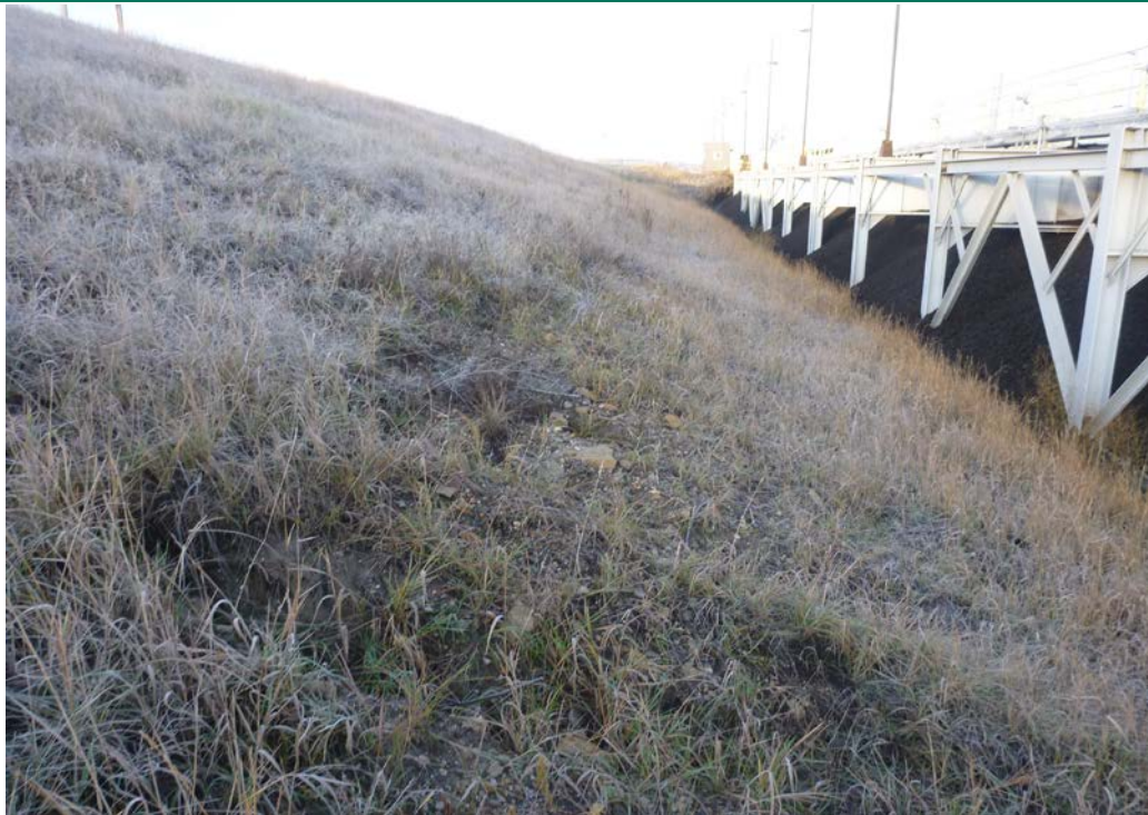
Photograph 7 Erosion rills on north exterior embankment near coal unloading area (looking west) (P1030346.JPG)
