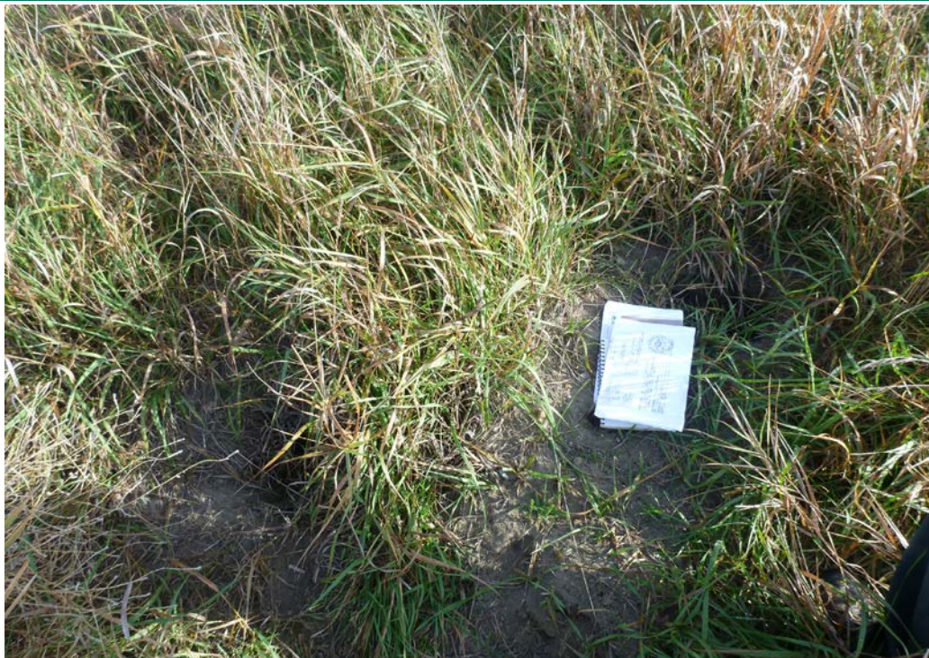
Photograph 20 Animal burrows on south exterior embankment (P1030391.JPG)
