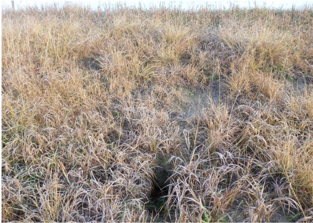
Photograph 9 Animal burrow on north exterior embankment (P1030358.JPG)
