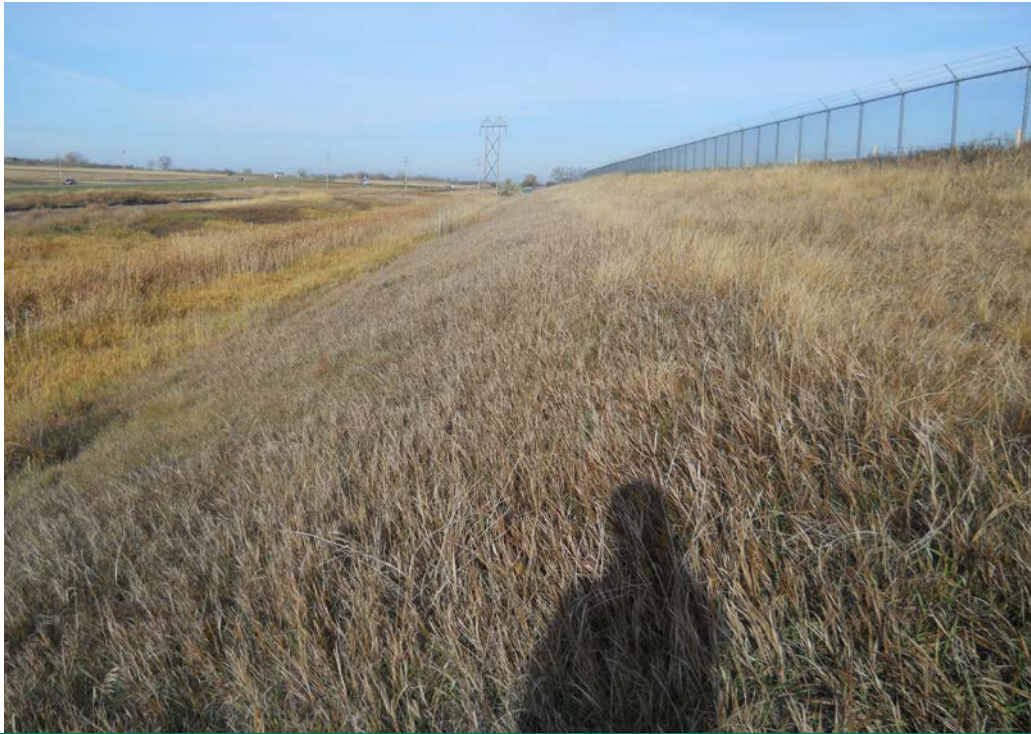
Photograph 9 (South Cell) Vegetation on downstream slope (DSCN0802.JPG)
