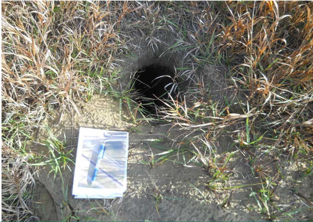
Photograph 11 (South Cell) Large animal burrow on south downstream slope (DSCN0806.JPG)
