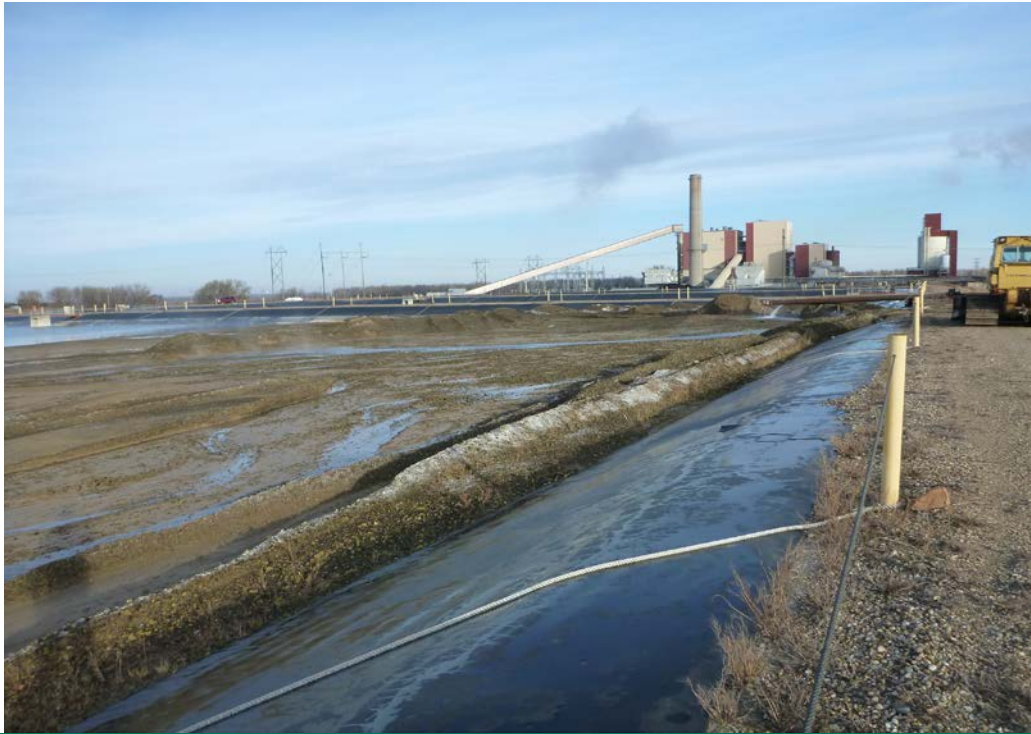
Photograph 23 (South Cell) Bottom ash deposition on the east side of of the South Cell (P1030383.JPG)
