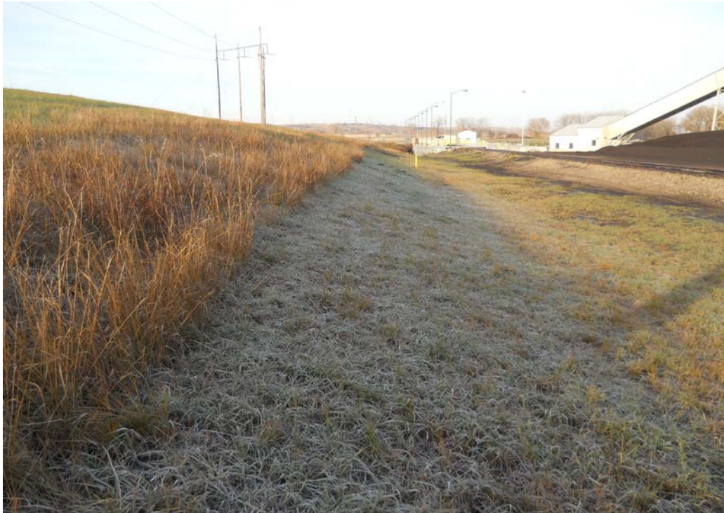
Photograph 2 (North Cell) Grass vegetation on north downstream slope (DSCN0789.JPG)
