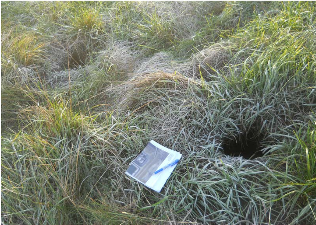
Photograph 1 (North Cell) Animal burrows on north downstream slope (DSCN0790.JPG)
