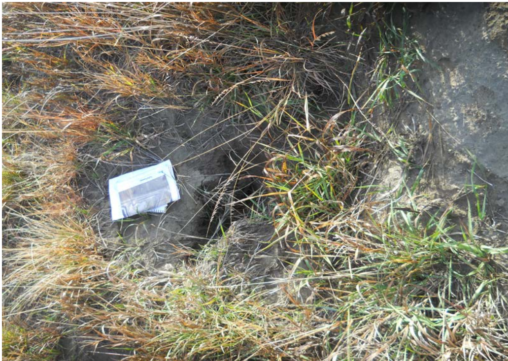
Photograph 10 (South Cell) Large animal burrow on south downstream slope (DSCN0803.JPG)
