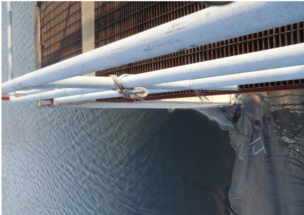
Photograph 12 (North Cell) North outlet hydraulic structure and geomembrane attachment to concrete (DSCN0792.JPG)
