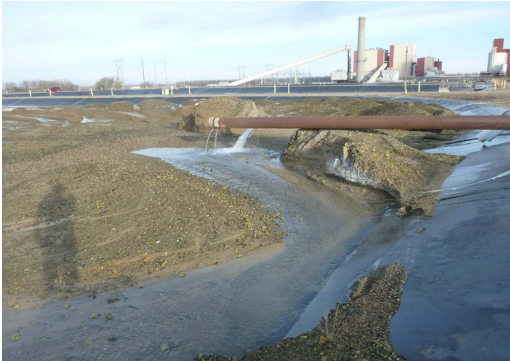
Photograph 24 (South Cell) Bottom ash conveyance water and geomembrane rub sheet on the east side of the South Cell (P1030384.JPG)
