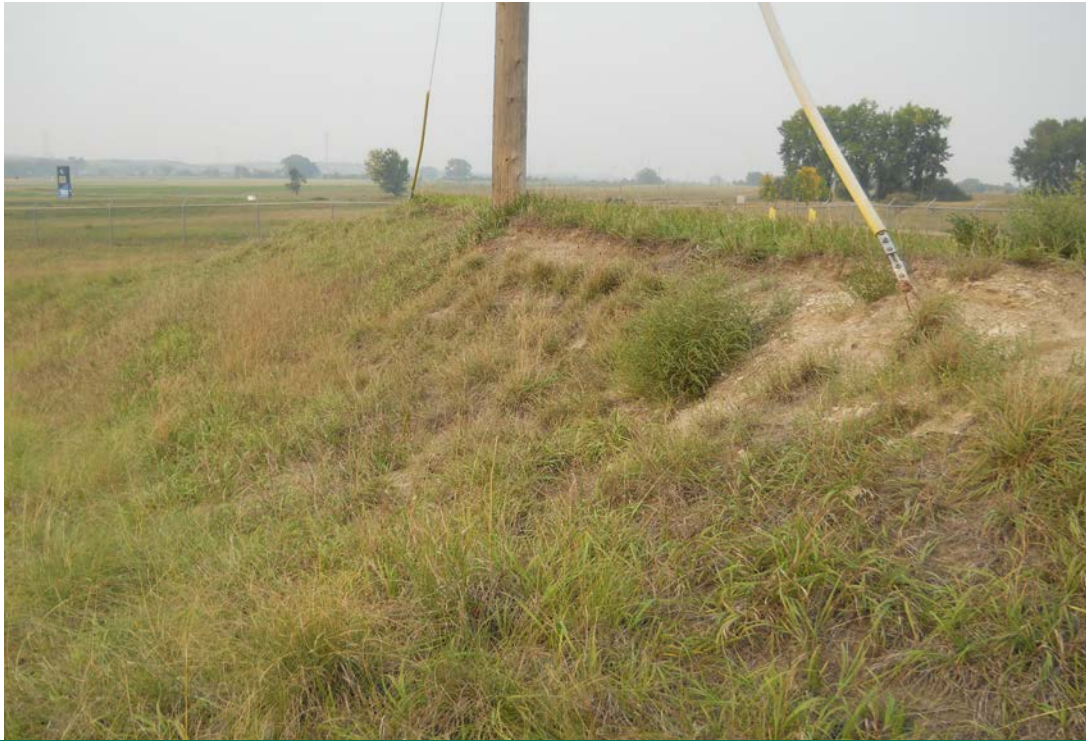
Photograph 9 (North berm upstream slope) Steep slope/erosion on south side of power pole (DSCN1586.JPG)
