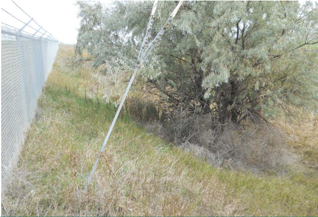
Photograph 17 (South toe) Tree along south downstream berm slope toe (DSCN1594.JPG)
