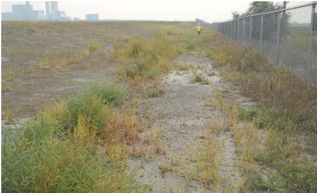
Photograph 18 (South berm crest) South perimeter berm crest with lack of well-defined contact water channel/berm (looking east) (DSCN1588.JPG)
