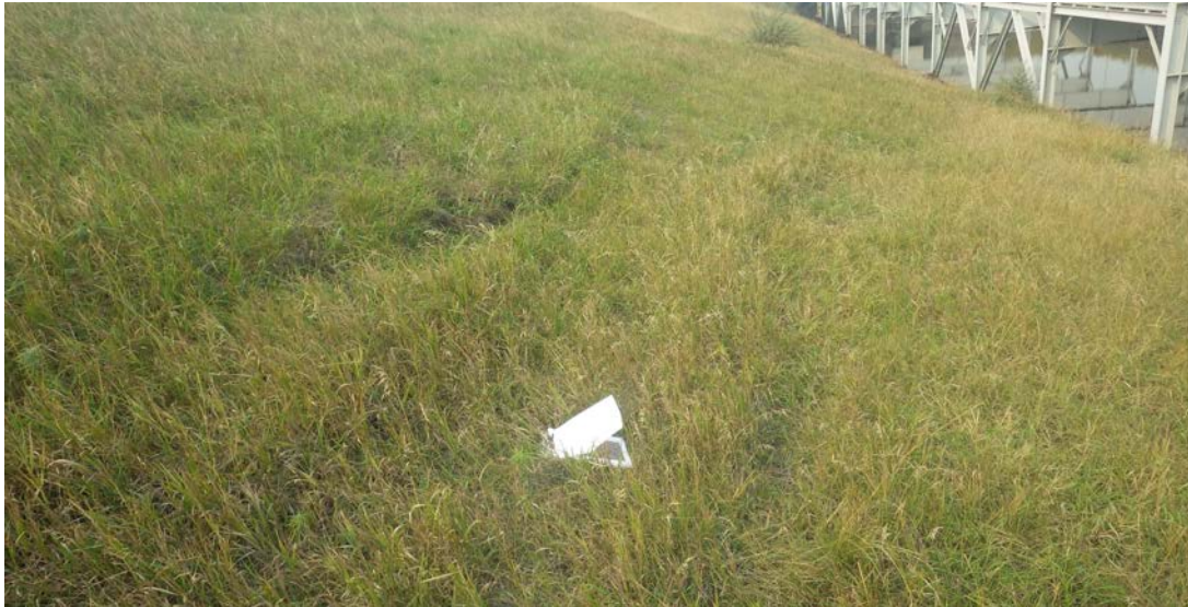
Photograph 4 (North berm downstream slope) Rutting along the north berm downstream slope (IMGP5404.JPG)
