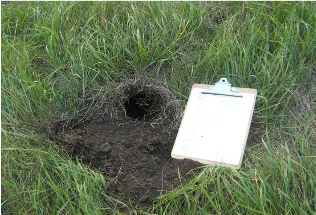
Photograph 5 (North berm downstream slope) Animal burrow on north berm downstream slope of the north cell. (DSCN1537.JPG)
