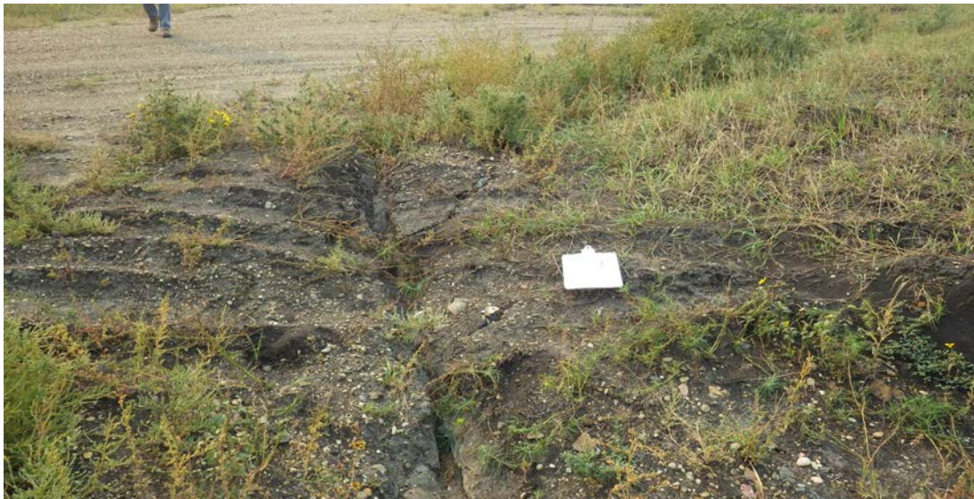
Photograph 6 (North berm downstream slope) Erosion rill on the north side of the north berm crest gravel road. (IMGP5390.JPG)
