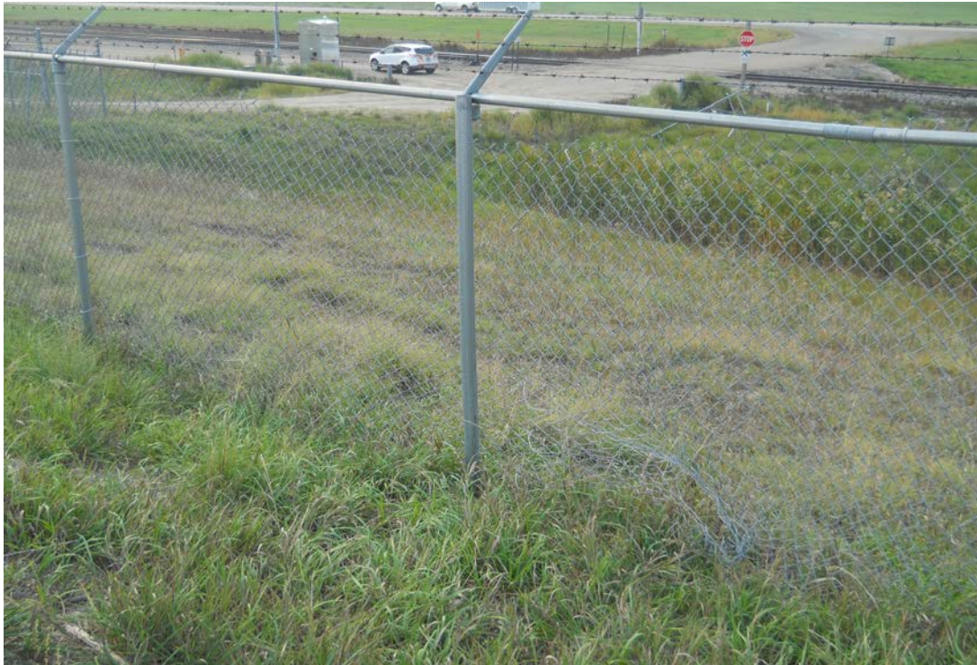
Photograph 16 (South berm downstream slope) Fence damage on the south berm downstream slope of the south cell. (DSCN1553.JPG)
