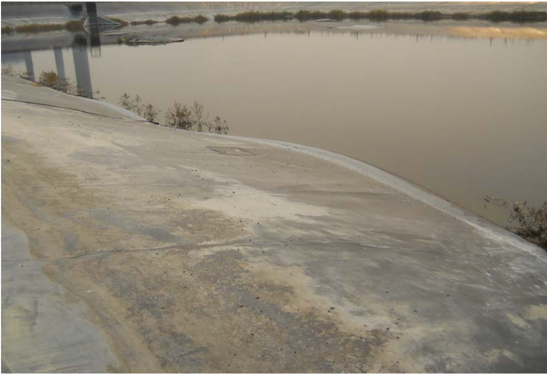
Photograph 20 (Center cell berm upstream slope) Water trapped under geomembrane liner along north berm upstream toe of the center cell. (DSCN1568.JPG)
