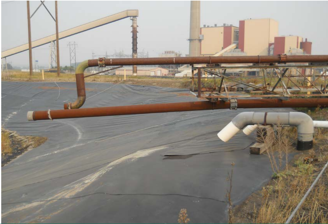
Photograph 7 (North cell berm upstream slope) Bottom ash inlet piping and trestle entering north cell. (DSCN1540.JPG)
