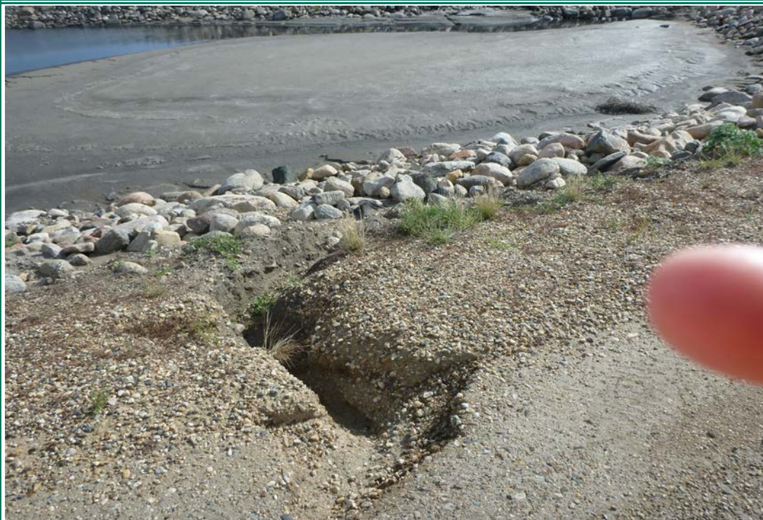
Photograph 17 (Center cell berm upstream slope) Erosion of intercell gravel road between west cell and center cell (P1040235.JPG)
