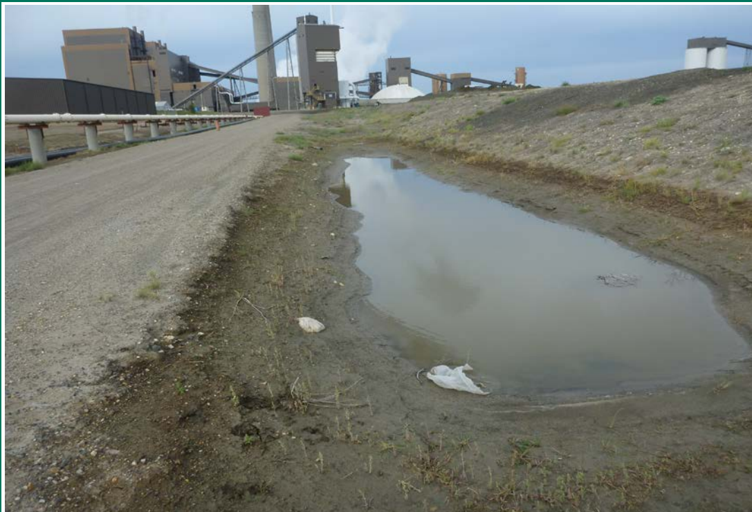
Photograph 2 (South berm downstream slope) Water ponded at low point along the south berm downstream slope (P1040193.JPG)
