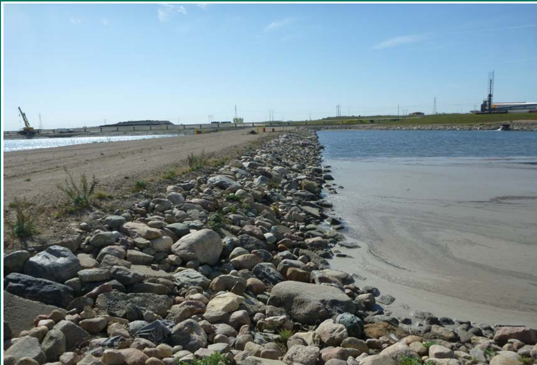
Photograph 30 (Center cell berm upstream slope) East side of center cell berm upstream slope riprap (P1040260.JPG)
