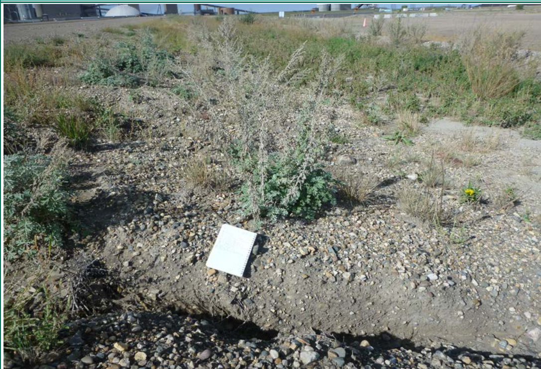
Photograph 25 (North berm downstream slope) East cell north berm downstream slope erosion rills (6-12 inches deep) (P1040253.JPG)
