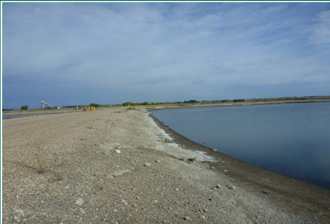
Photograph 18 (East cell berm upstream slope) East cell berm upstream slope fly ash protective cover (P1040238.JPG)
