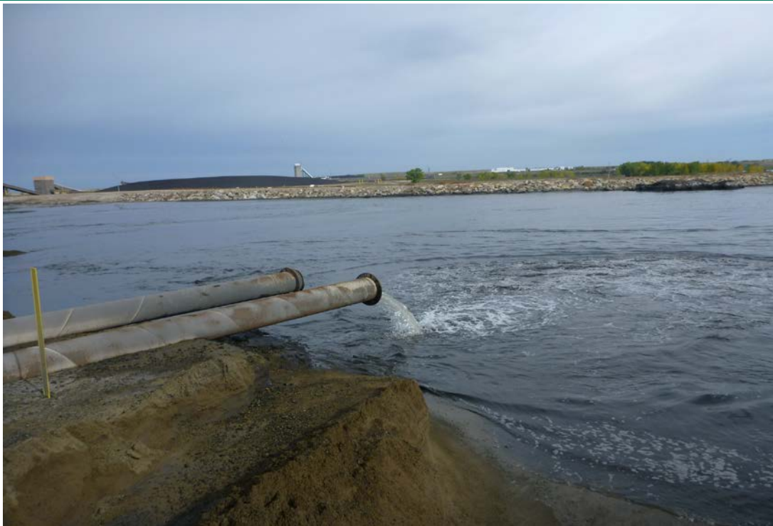
Photograph 6 (West cell berm upstream slope) CCR discharge pipes (P1040209.JPG)
