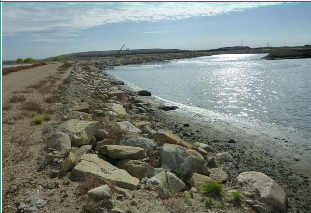
Photograph 13 (West cell berm upstream slope) Berm upstream slope with riprap (P1040230.JPG)
