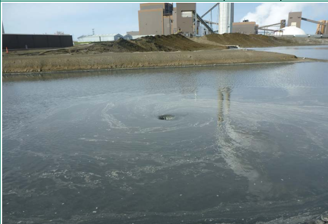
Photograph 16 (West cell) Decant pipe inlet from west cell to center cell (P1040233.JPG)
