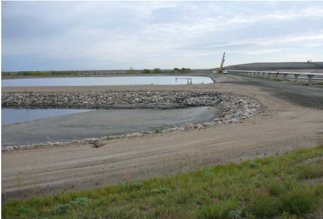
Photograph 3 (Center cell berm upstream slope) Center cell riprap and sediment accumulation from plant drains (P1040195.JPG)
