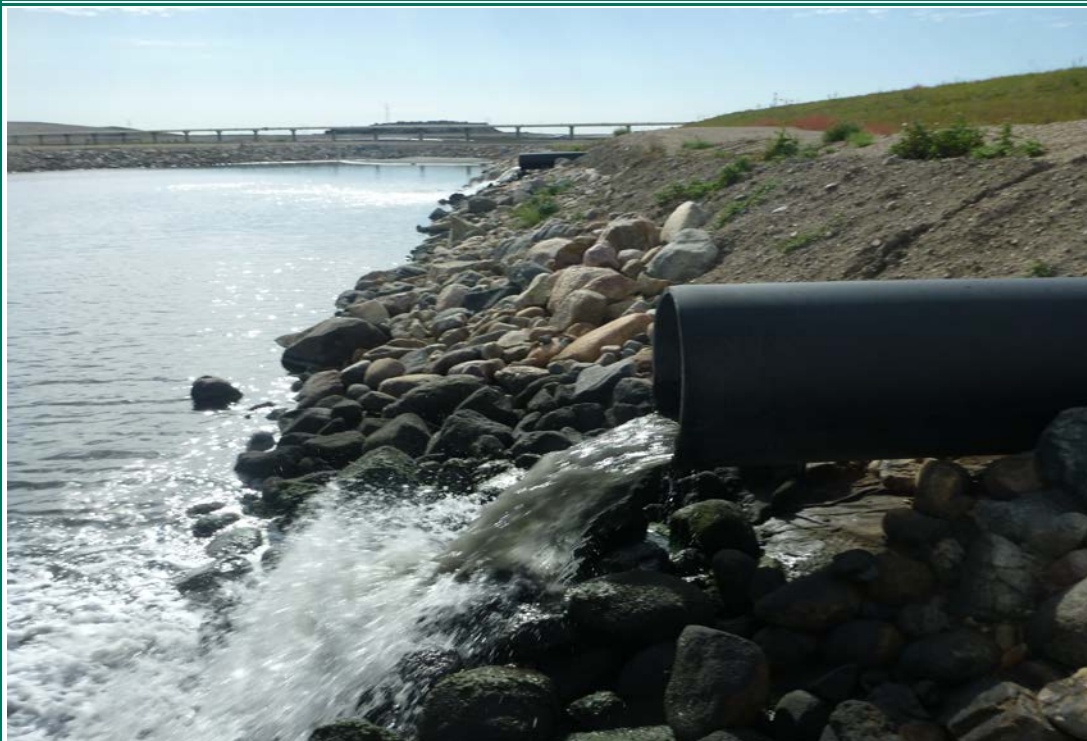
Photograph 15 (Center cell berm upstream slope) North decant outlet between the west cell and center cell (P1040232.JPG)
