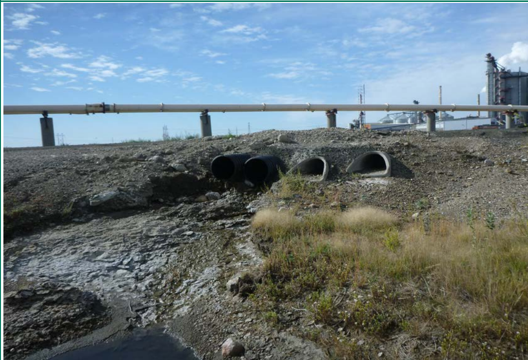
Photograph 19 (East cell berm upstream slope) Culvert outlet from ash pipelines ditch to the east cell (P1040239.JPG)
