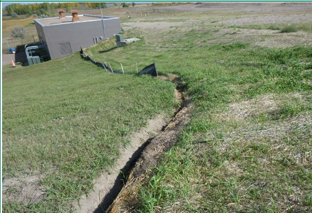
Photograph 27 (North berm downstream slope) Silt fence trench to be filled in (P1040255.JPG)
