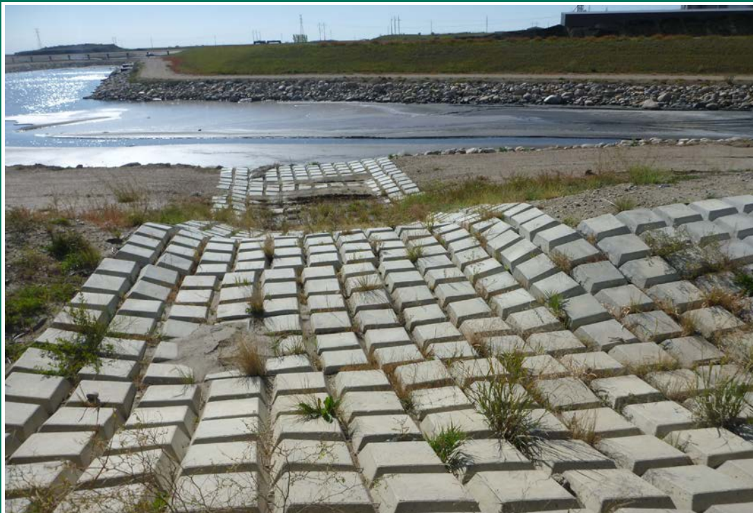
Photograph 28 (North surface water channel inlet to Center Cell) Articulated Concrete Block (ACB) armoring (P1040257.JPG)
