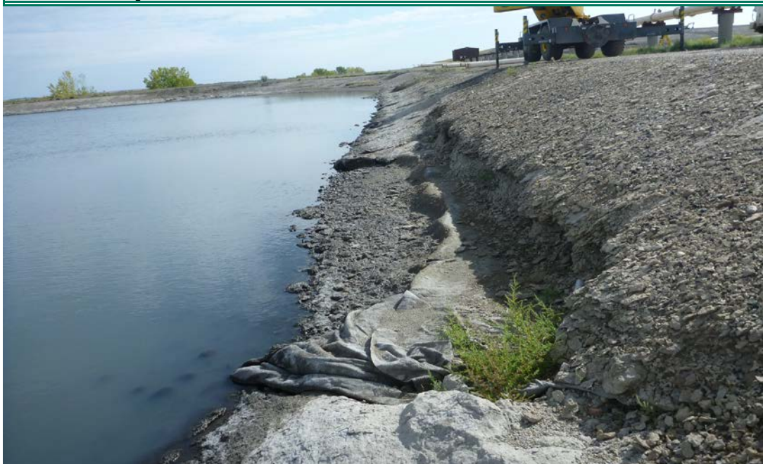
Photograph 21 (East cell berm upstream slope) Oversteepened fly ash protective cover on the south upstream slope of the east cell and exposed geotextile (P1040243.JPG)
