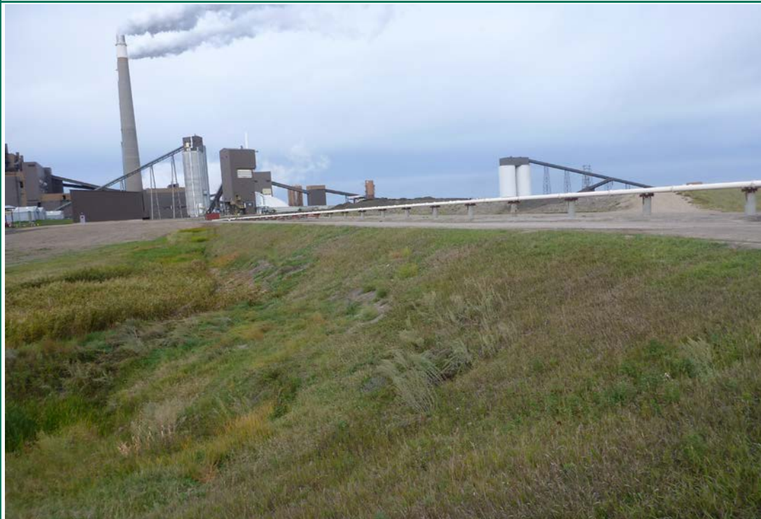
Photograph 1 (South toe) South toe, no seeps or burrows noted (P1040189.JPG)
