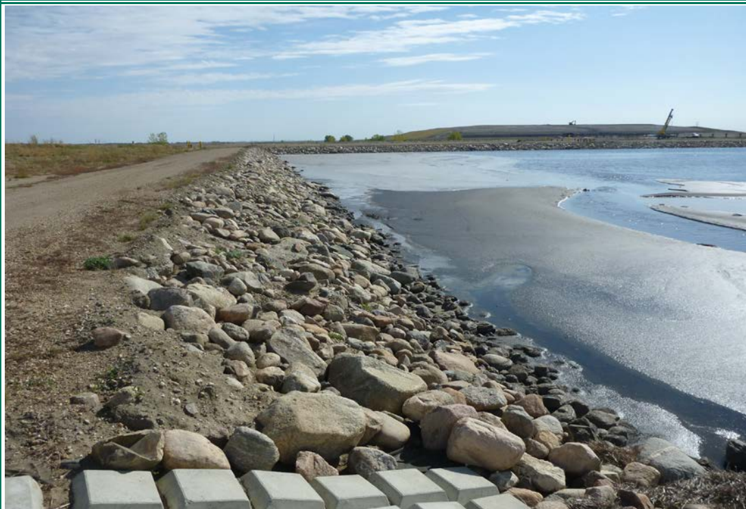
Photograph 29 (Center cell berm upstream slope) Center cell berm upstream slope riprap (P1040258.JPG)
