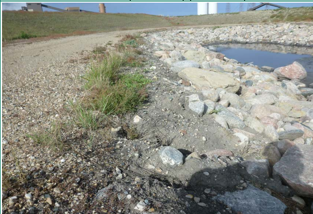
Photograph 12 (Center cell berm upstream slope) Center cell gravel road, some minor erosion into the riprap (P1040229.JPG)
