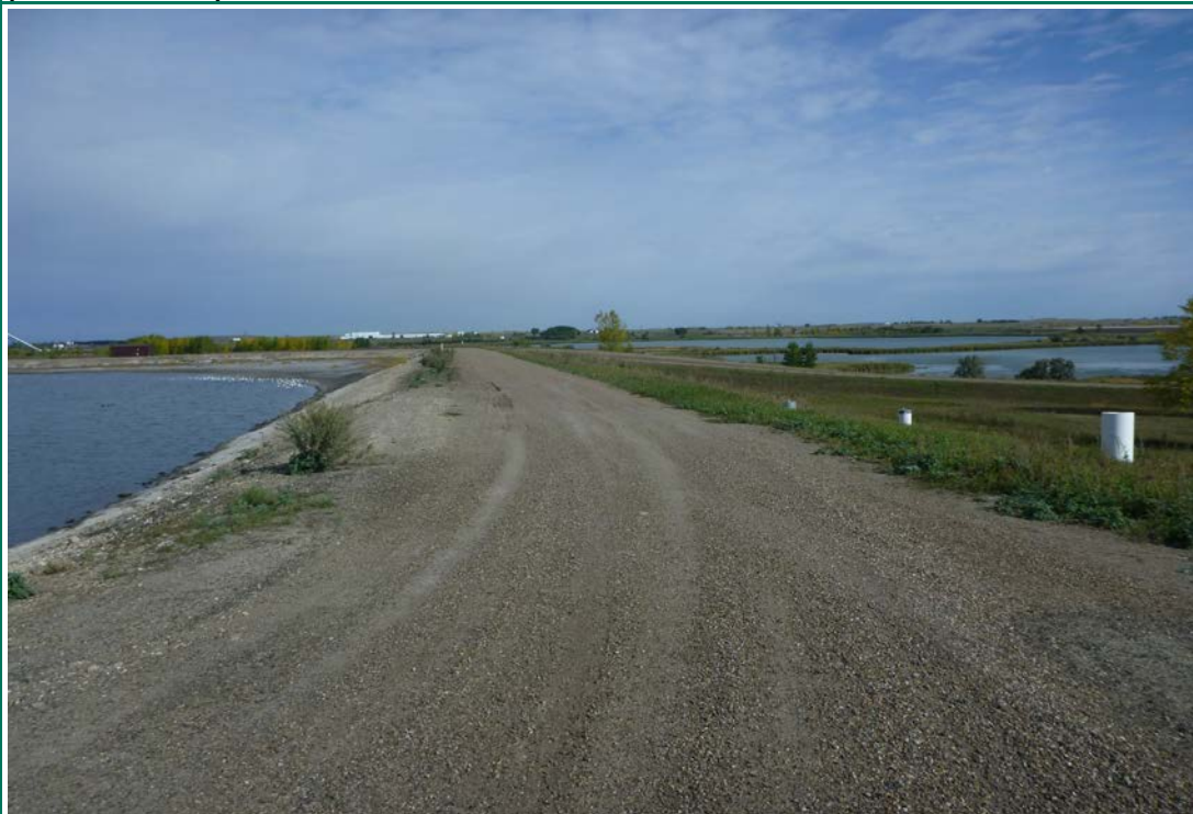
Photograph 22 (East cell berm crest) East perimeter berm crest gravel road, minor vegetation growing on berm upstream slope (P1040245.JPG)
