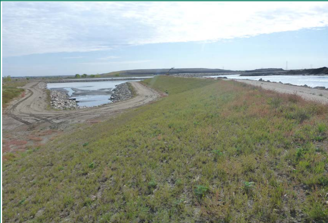
Photograph 11 (West cell/center cell intercell berm) West cell/center cell intercell berm (minor erosion) (P1040223.JPG)
