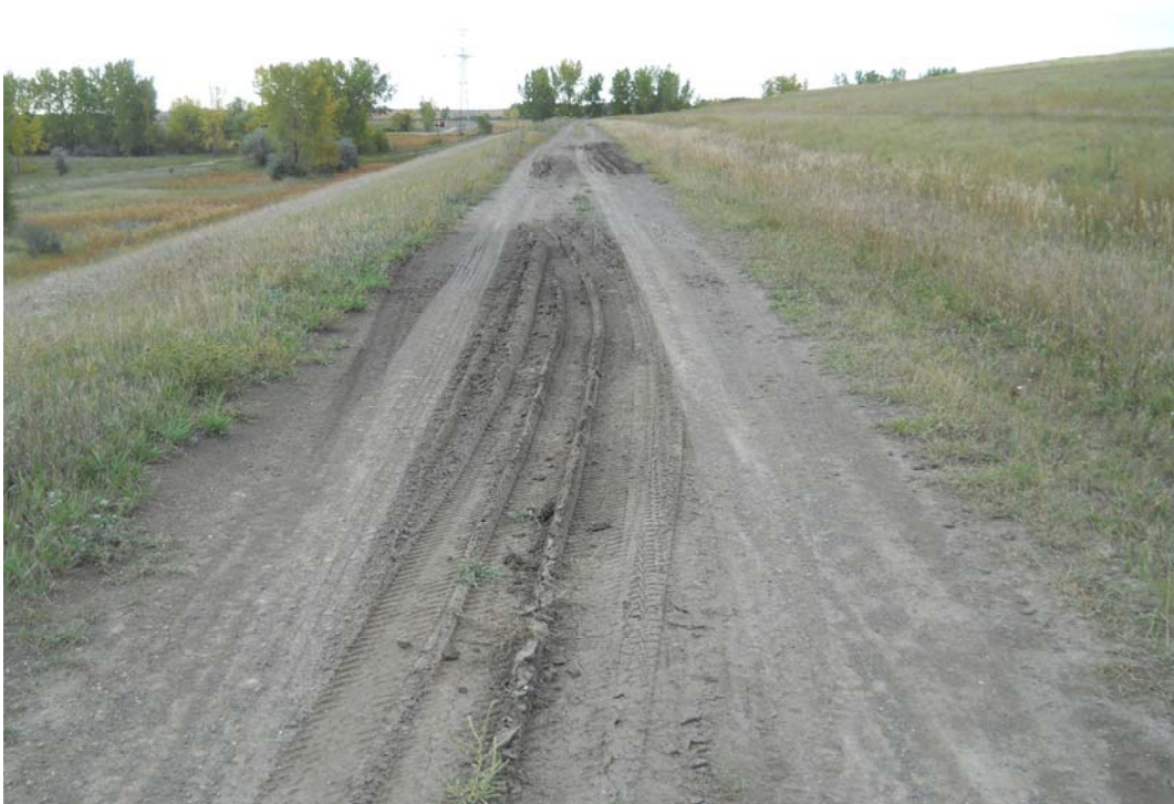
Photograph 4 (East berm crest) Rutting of berm crest perimeter access road (DSCN1678.JPG)
