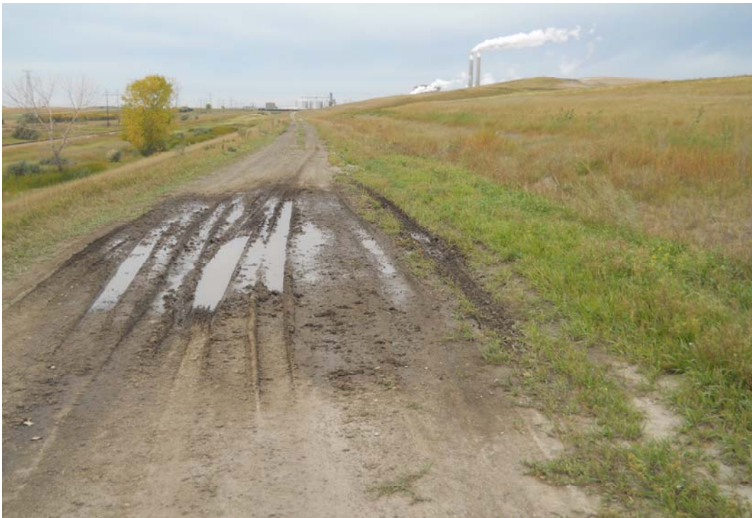
Photograph 8 (South berm crest) Rutting of berm crest perimeter access road (DSCN1693.JPG)
