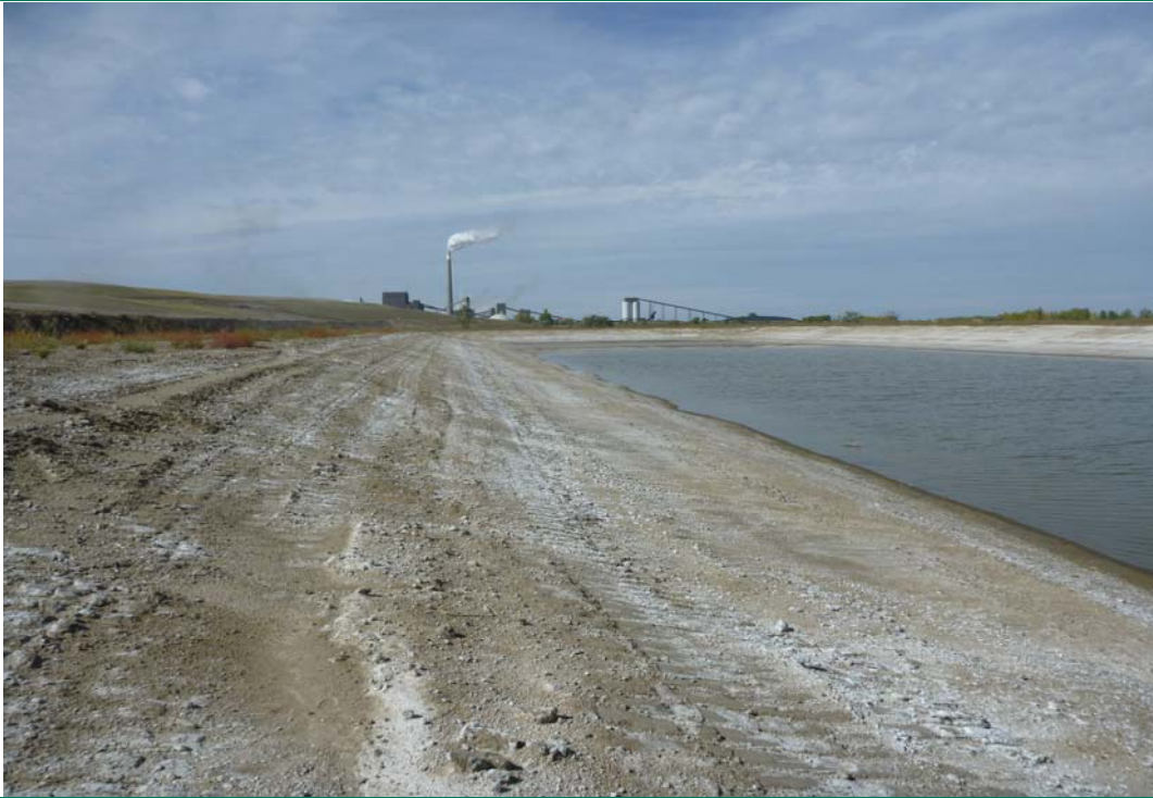
Photograph 25 (Contact water collection area) Fly ash protective cover in contact water collection area (P1040264.JPG)
