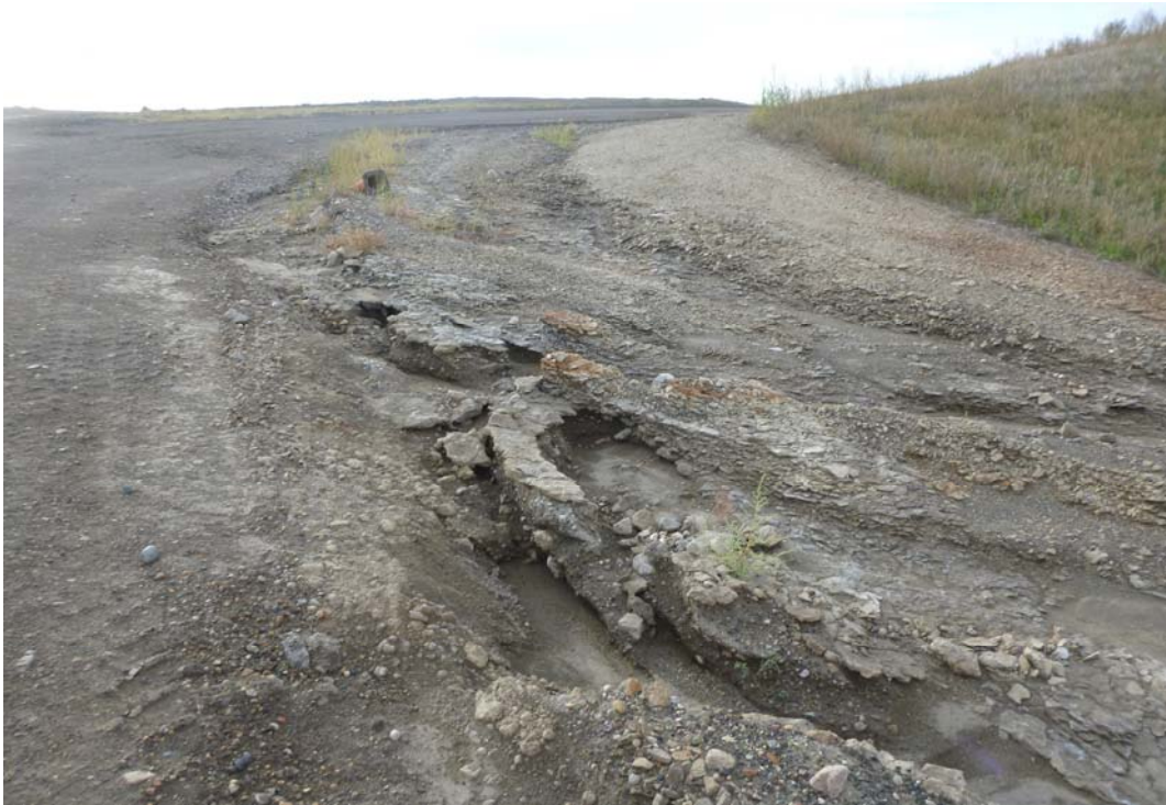
Photograph 14 (Northwest CCR slope) Minor erosion of fly ash at interface between Upstream Raise 92 and Southeast 16 (P1040166.JPG)
