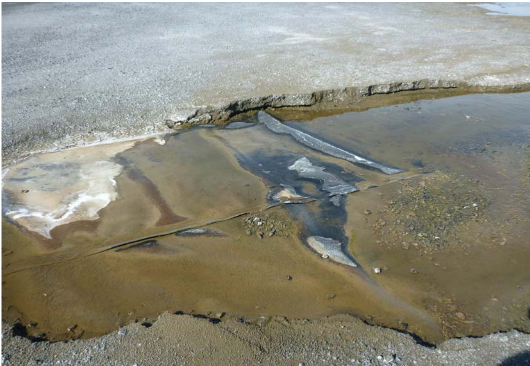
Photograph 24 (Contact water collection area) Top of geomembrane liner in contact water collection area (P1040263.JPG)
