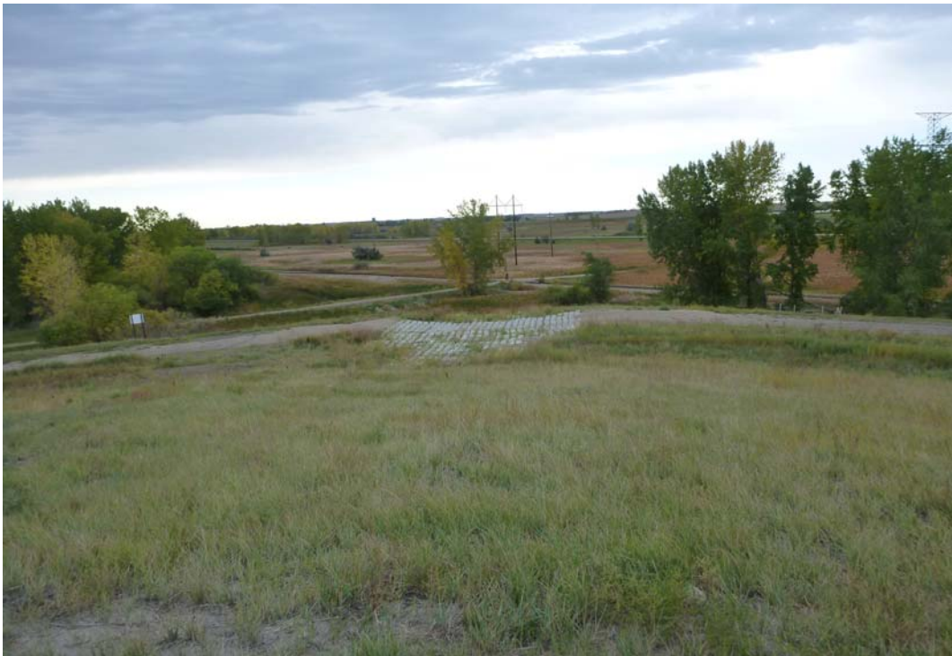
Photograph 22 (Southeast CCR downstream slope) Articulated Concrete Block (ACB) downchute (P1040184.JPG)
