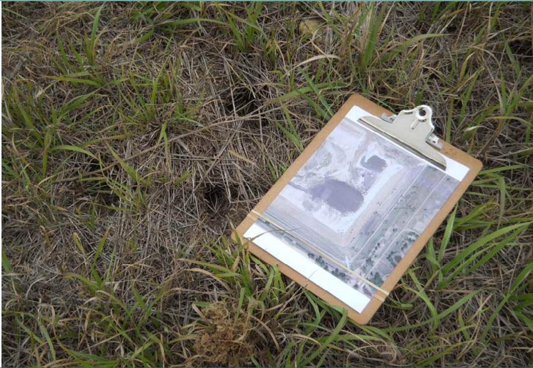
Photograph 5 (East berm downstream slope) Small animal burrows (DSCN1683.JPG)
