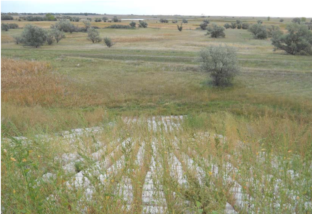
Photograph 6 (Northeast berm downstream slope) Downchute channel below berm crest perimeter access road (DSCN1688.JPG)
