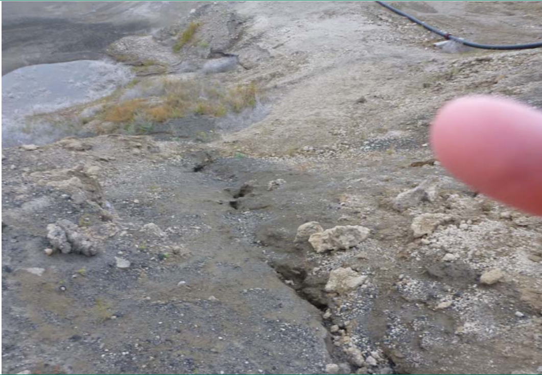
Photograph 9 (North CCR slope) Erosion of placed CCR materials (P1040150.JPG)
