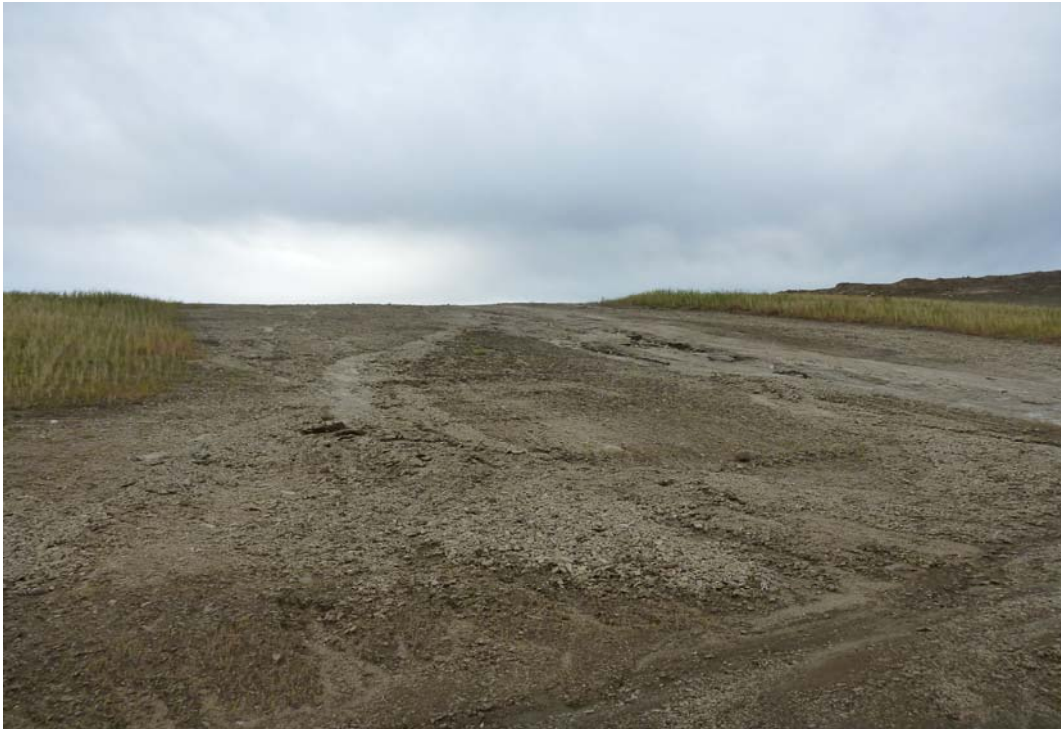
Photograph 12 (North CCR slope) Minor erosion of fly ash slope due to channelized water flow (P1040162.JPG)
