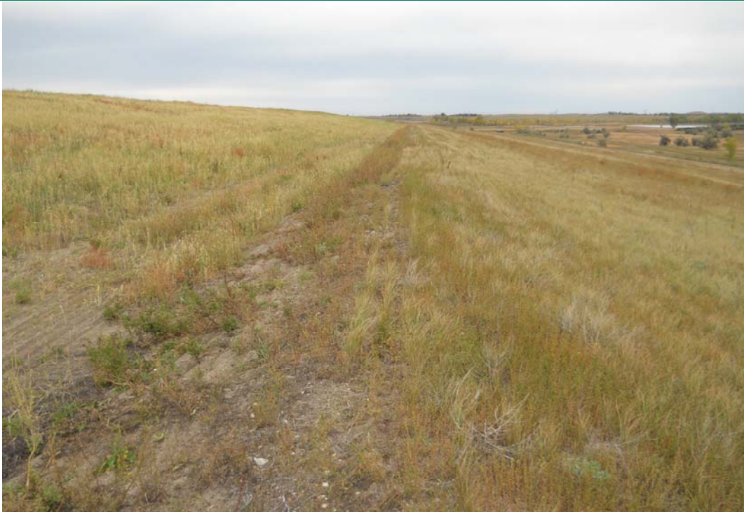
Photograph 1 (East CCR downstream slope) Boundary between CCR downstream slope with temporary cover (upslope) and CCR downstream slope with final cover (downslope) (DSCN1660.JPG)
