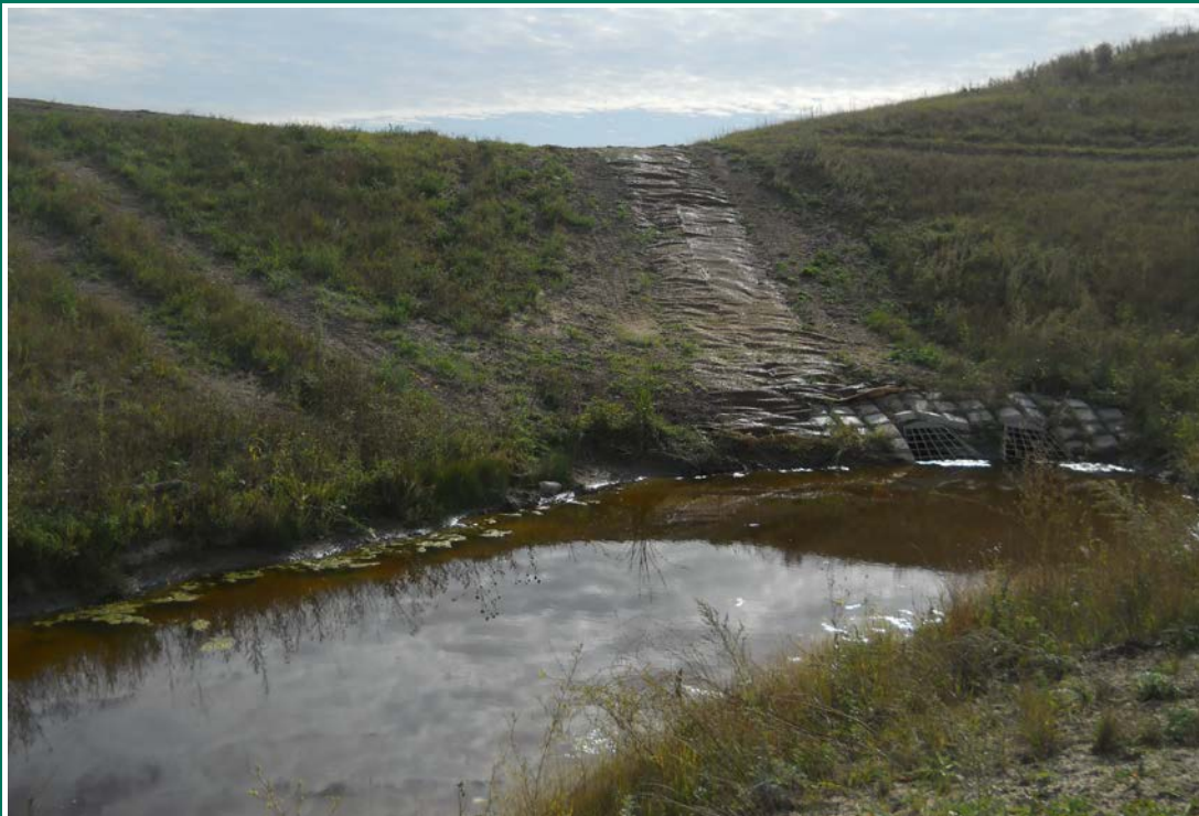
Photograph 10 (Southwest berm downstream slope) Southwest surface water ditch and southwest culvert inlets, 1 foot of water in ditch (DSCN1715.JPG)
