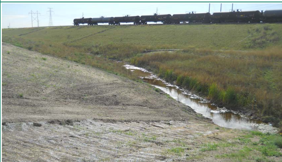
Photograph 12 (South berm downstream slope) Outlet of southwest culverts and erosion control blankets installed on south berm downstream slope (DSCN1719.JPG)
