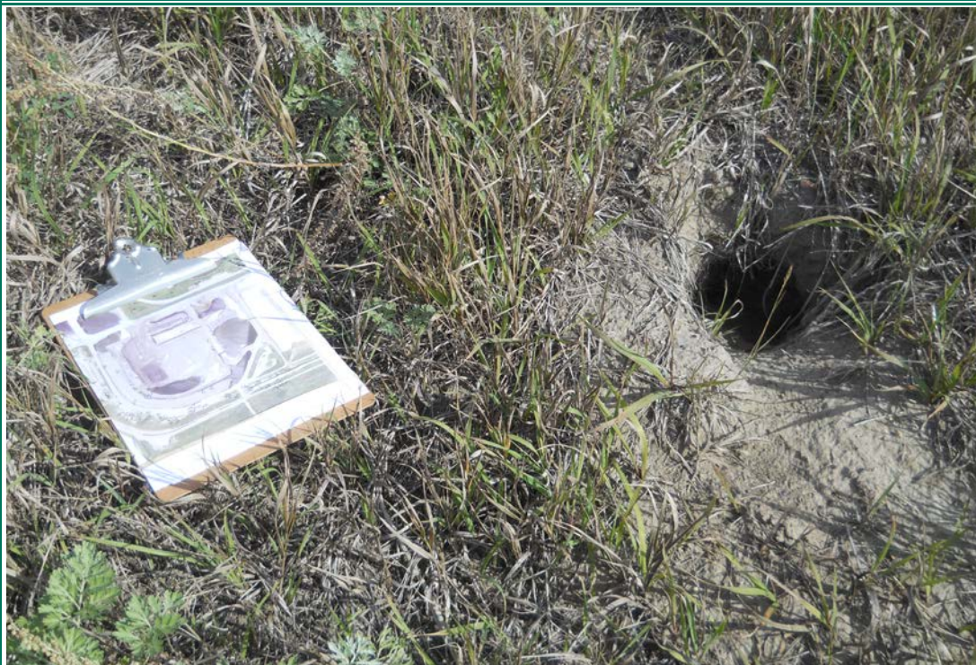
Photograph 19 (South berm downstream slope) Animal burrow (DSCN1738.JPG)
