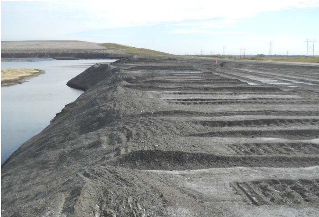
Photograph 15 (South CCR upstream slope) CCR placement in Upstream Raise 91 (DSCN1727.JPG)
