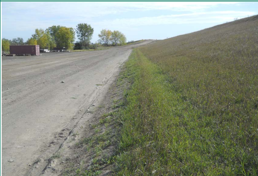
Photograph 25 (North toe) North toe in good condition (DSCN1752.JPG)
