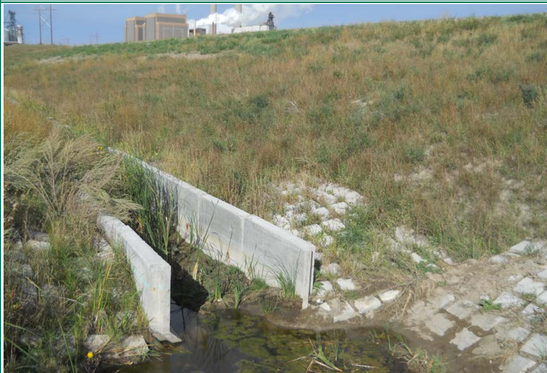
Photograph 17 (South berm downstream slope) South berm downstream slope and concrete surface water channel (DSCN1731.JPG)
