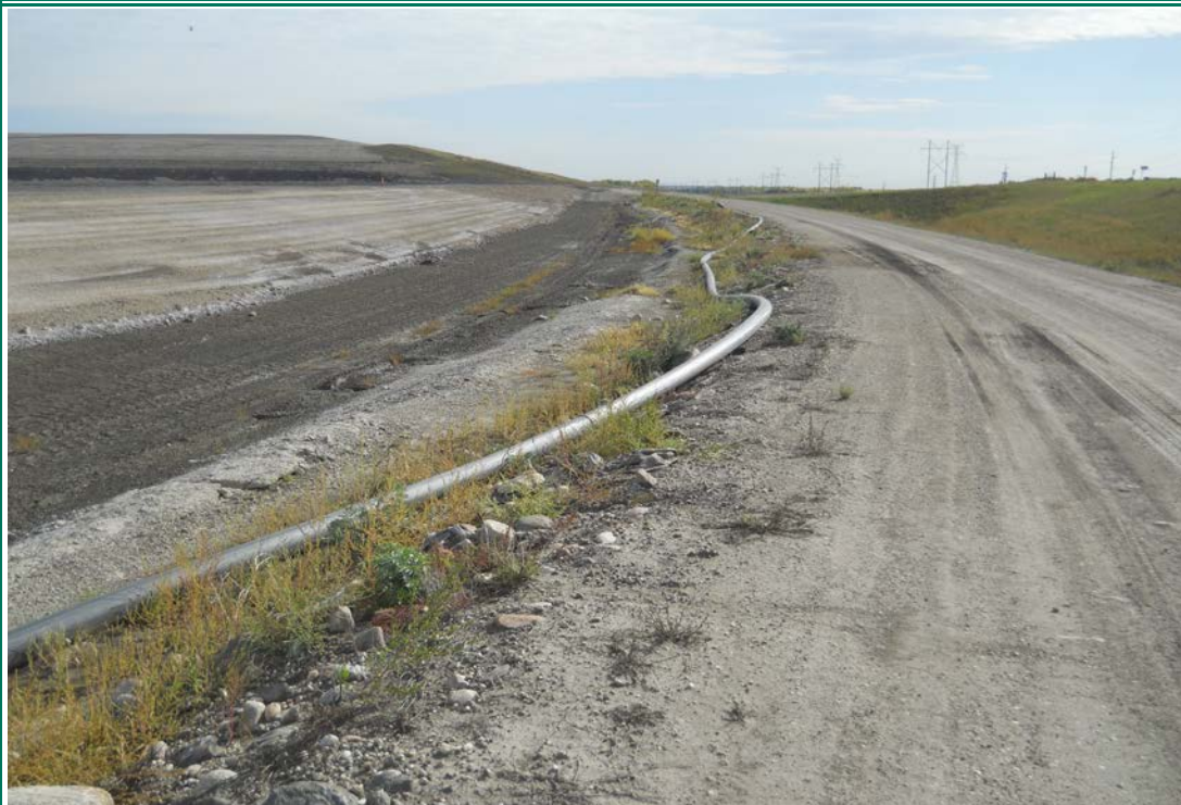
Photograph 13 (South berm upstream slope) Berm upstream slope of Upstream Raise 91 and contact water control channel (DSCN1723.JPG)
