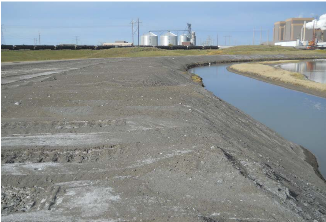
Photograph 16 (South CCR upstream slope) CCR placement in Upstream Raise 91 (DSCN1728.JPG)
