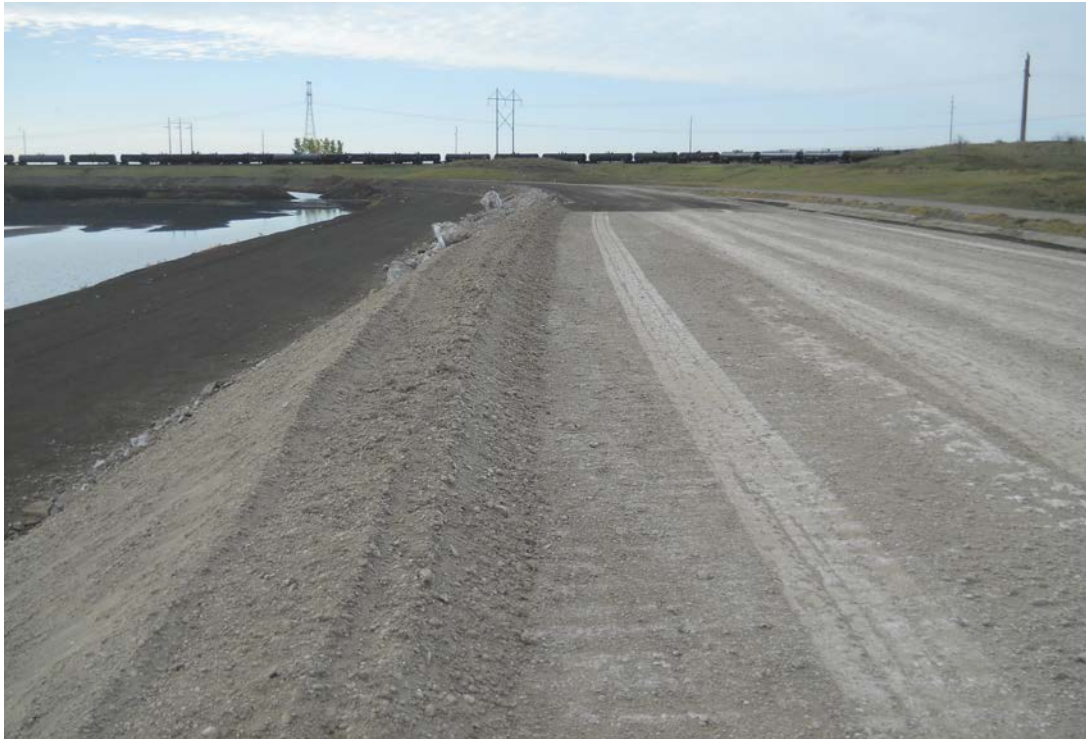
Photograph 3 (West CCR crest) CCR material placement (DSCN1699.JPG)
