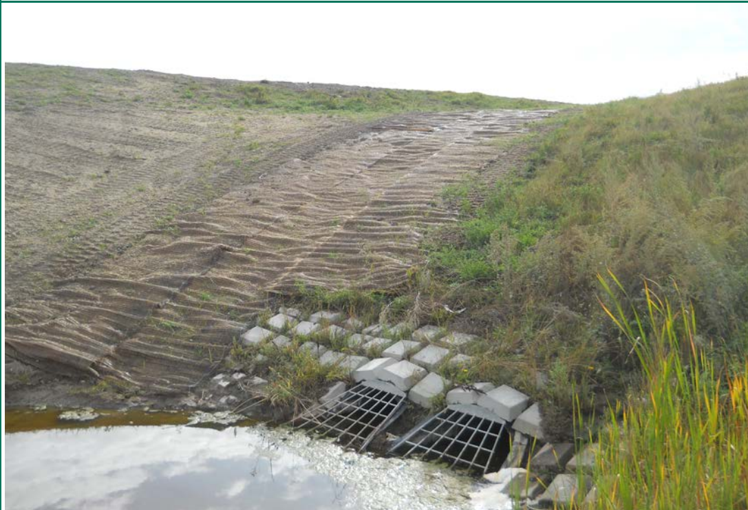
Photograph 5 (West berm downstream slope) Erosion control blanket on west berm downstream slope of Upstream Raise 91 (DSCN1705.JPG)
