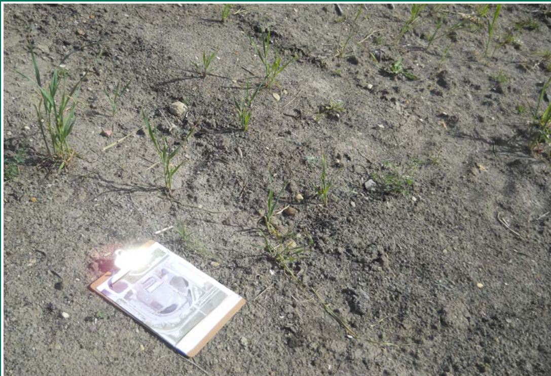
Photograph 18 (South berm downstream slope) Scarce vegetation on south berm downstream slope (recently repaired) (DSCN1734.JPG)
