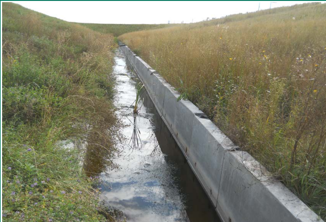
Photograph 14 (South toe) Approximately 1 foot of water in concrete surface water channel (DSCN1726.JPG)
