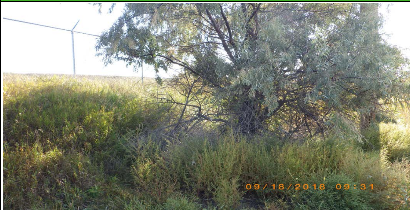
Photograph 13 (South berm) Tree along south downstream berm slope toe (34ccs.JPG)
