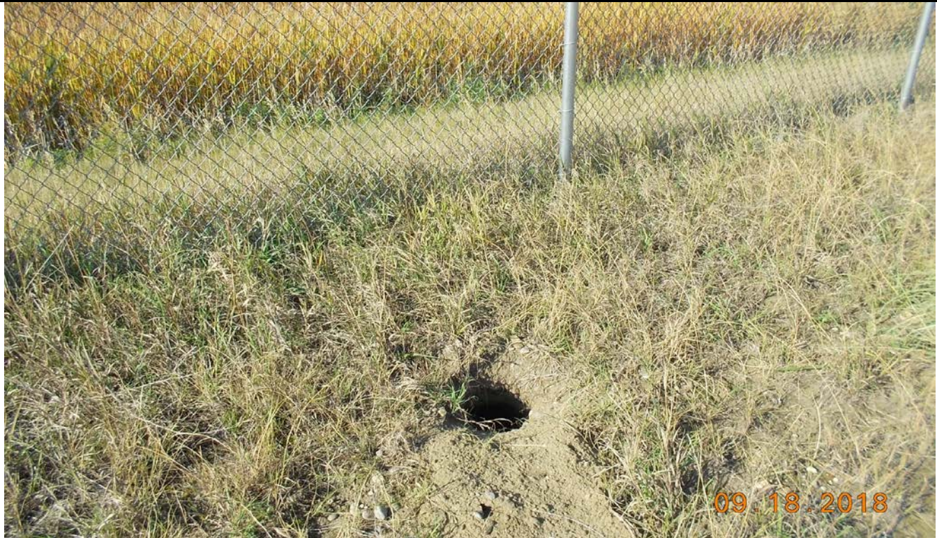
Photograph 19 (South berm) Animal burrows on south berm crest (SS PDS (2).JPG)
