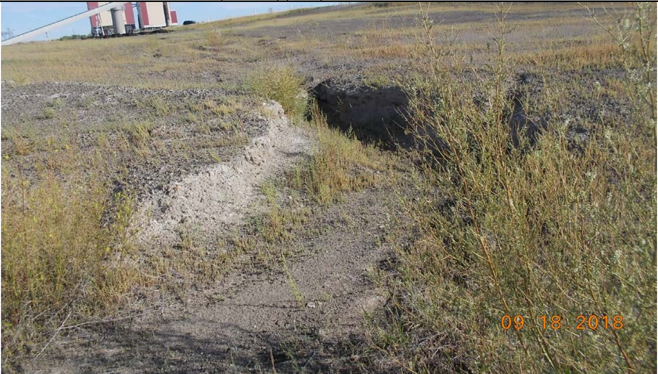
Photograph 20 (South berm) Erosion of placed CCR material on the south side (SS PDS (37).JPG)
