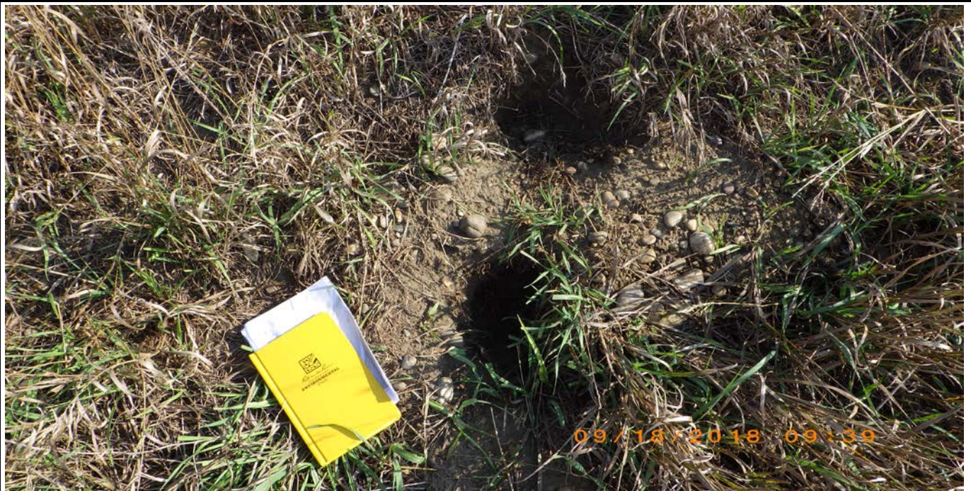
Photograph 16 (South berm) Animal burrows on south downstream slope (37ccs.JPG)
