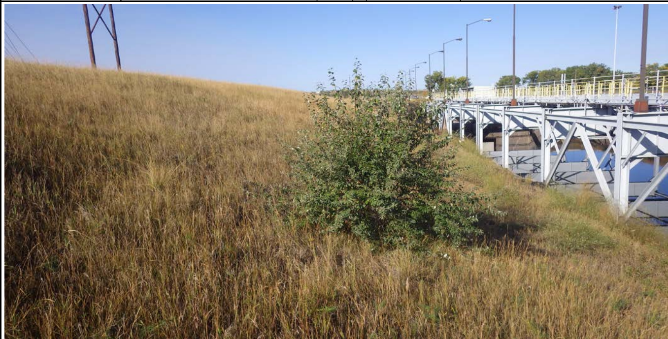
Photograph 4 (North downstream slope) Woody vegetation on downstream slope (IMGP6260.JPG)
