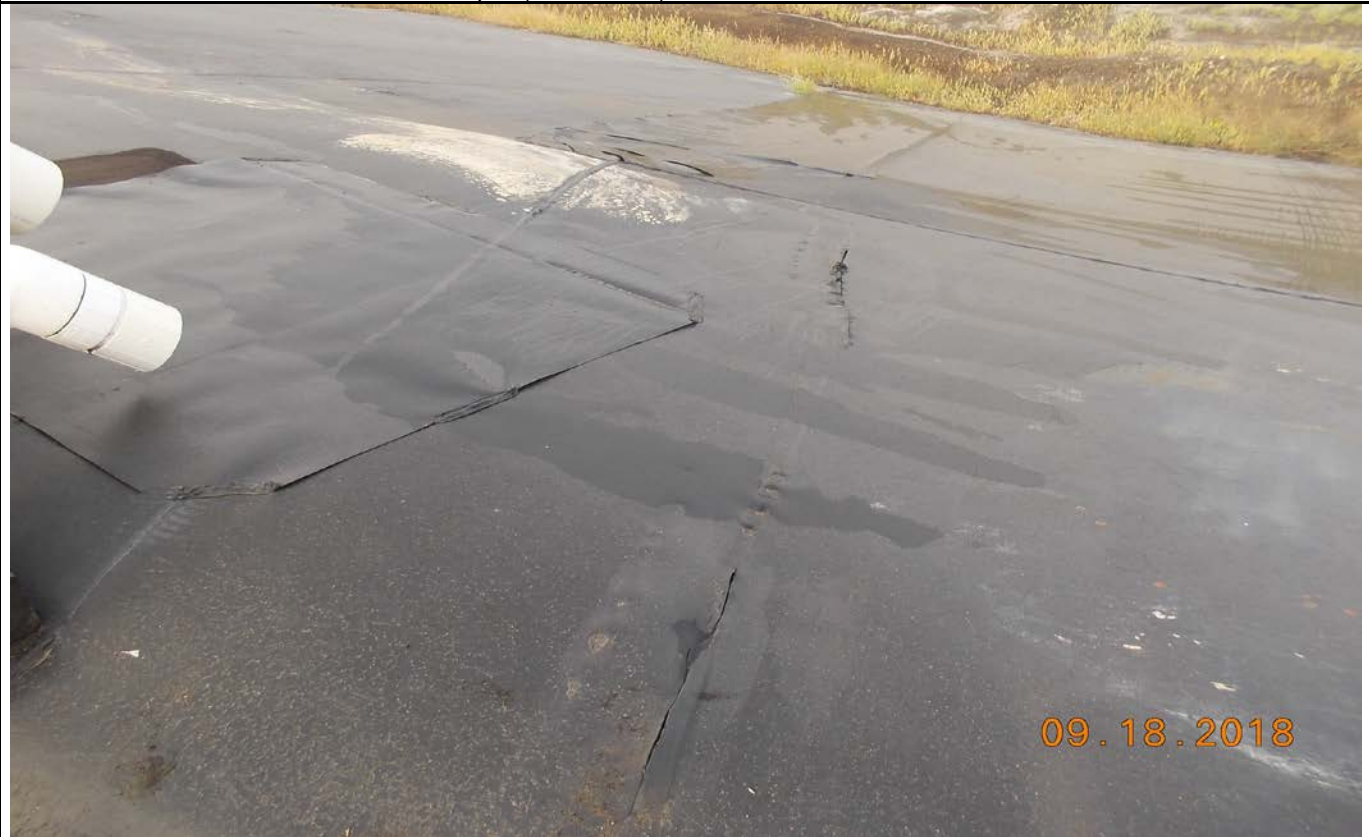
Photograph 18 (North Cell east upstream slope) Minor geomembrane damage on upstream slope and retention pond/coal pit sump inlet piping (SS PDS (6).JPG)
