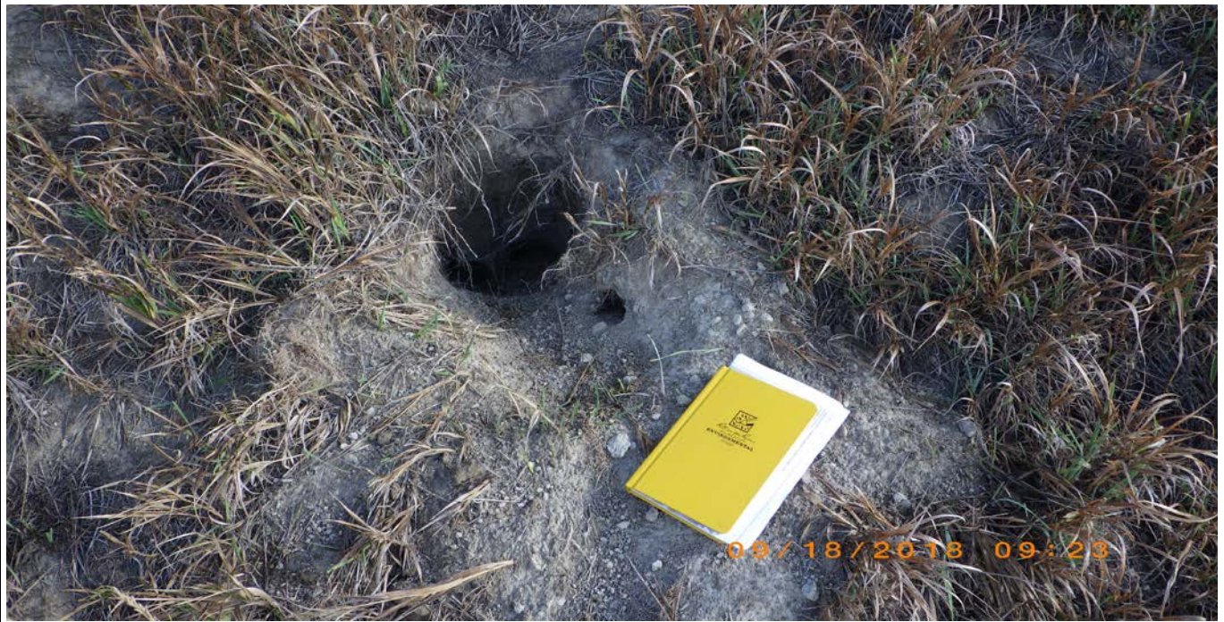
Photograph 17 (South downstream slope) Animal burrow on south downstream slope (29ccs.JPG)
