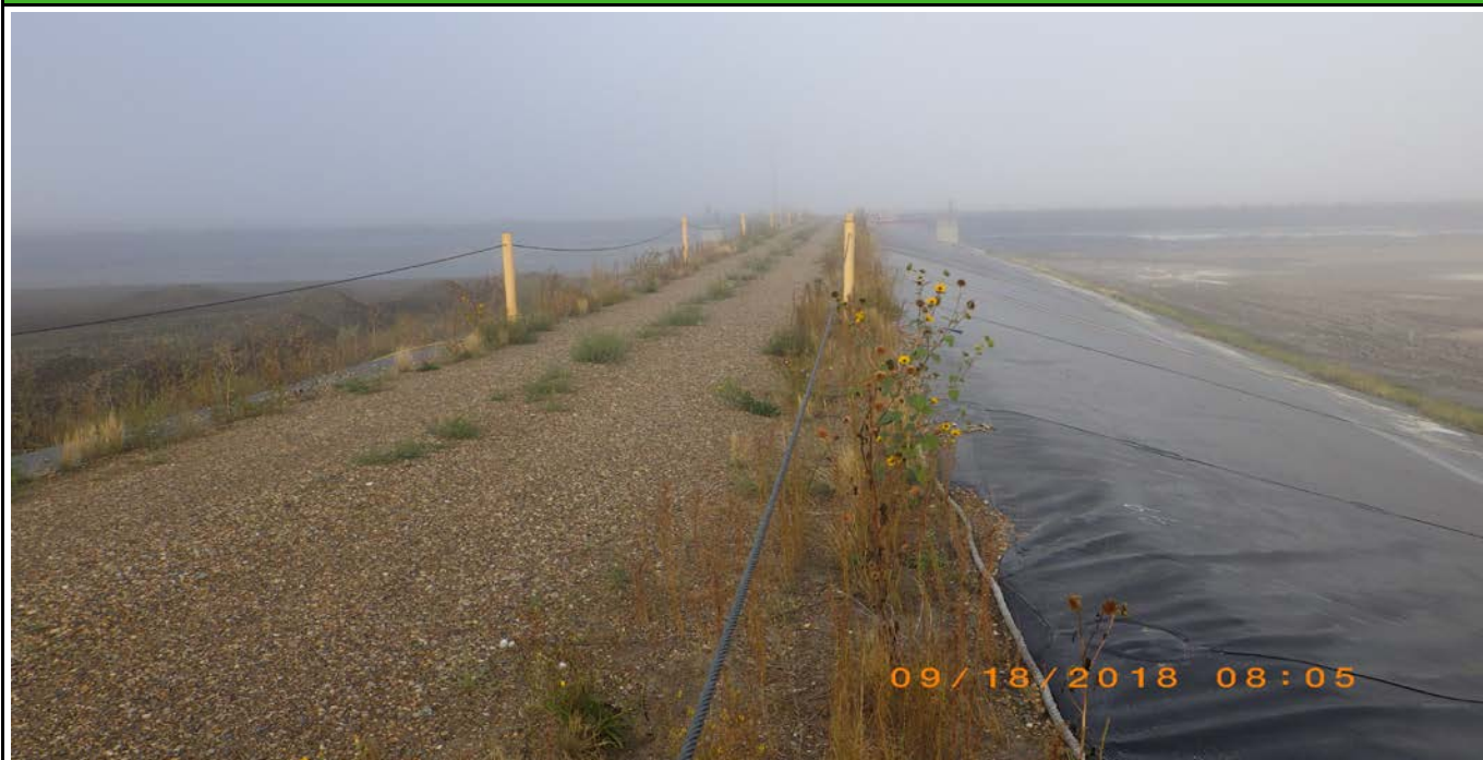
Photograph 13 (Center/South Cell berm crest) Center/South Cell crest with gravel road surface (15ccs.JPG)
