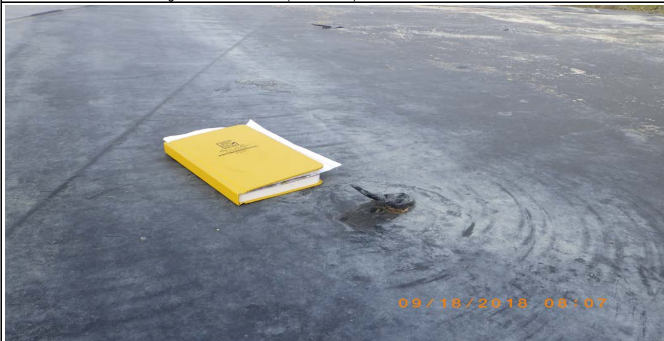
Photograph 14 (Center Cell east upstream slope) Failed geomembrane extrusion bead repair (16ccs.JPG)
