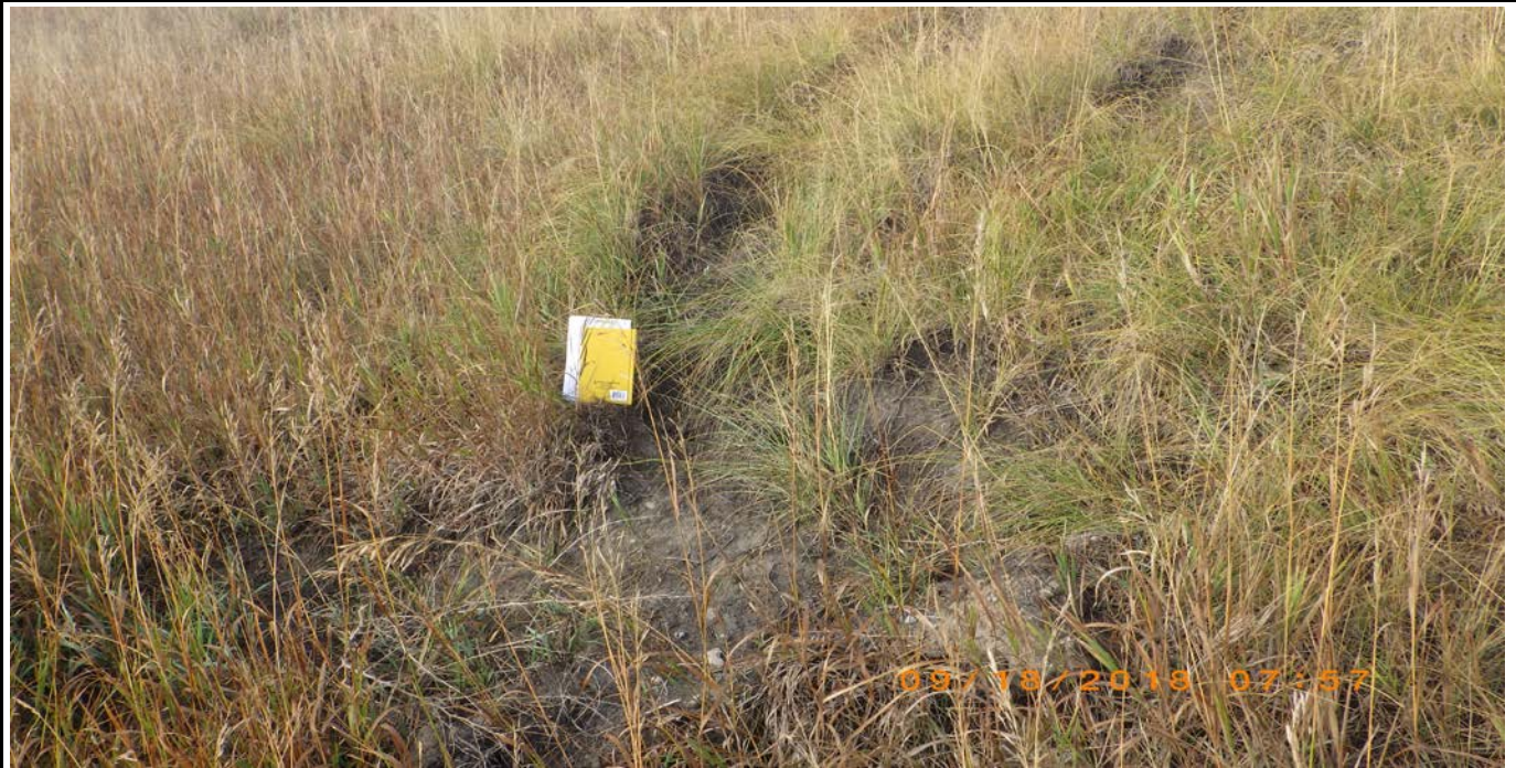
Photograph 10 (East downstream slope) Erosion and rutting on downstream slope near the toe (9ccs.JPG)
