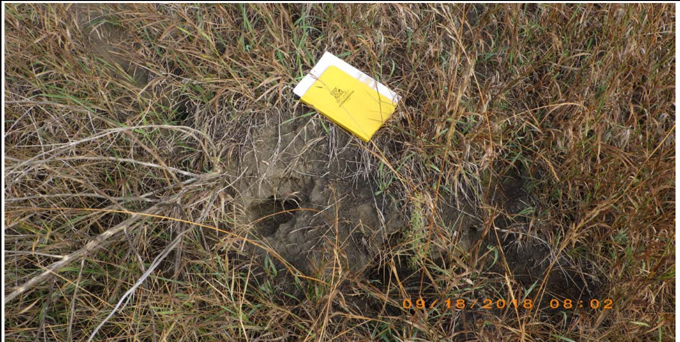
Photograph 12 (East toe) Animal burrows at the toe of the slope (12ccs.JPG)
