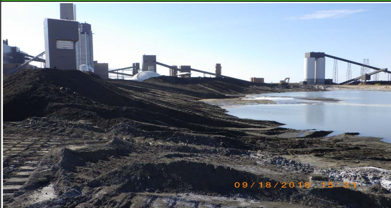
Photograph 11 (South berm upstream slope) Bottom ash discharge pipes and bottom ash dewatering stockpiles (8ccs.JPG)
