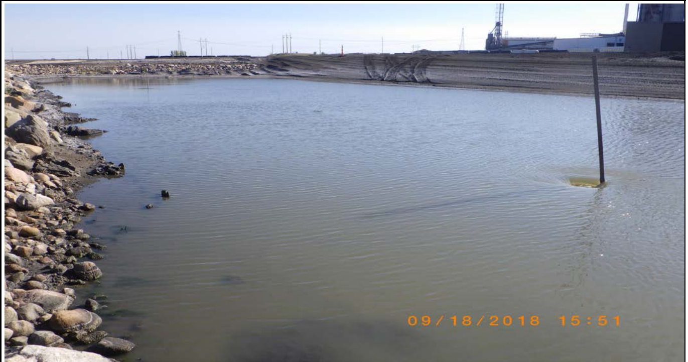
Photograph 19 (West Cell interior) Decant pipe inlet from west cell to center cell (24ccs.JPG)
