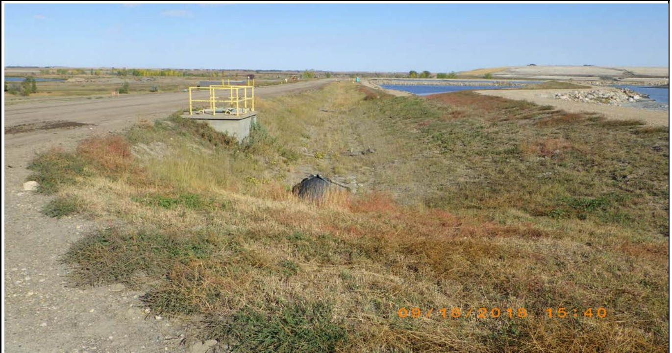
Photograph 13 (North drainage ditch) Culvert and channel with recently established vegetation (15ccs.JPG)
