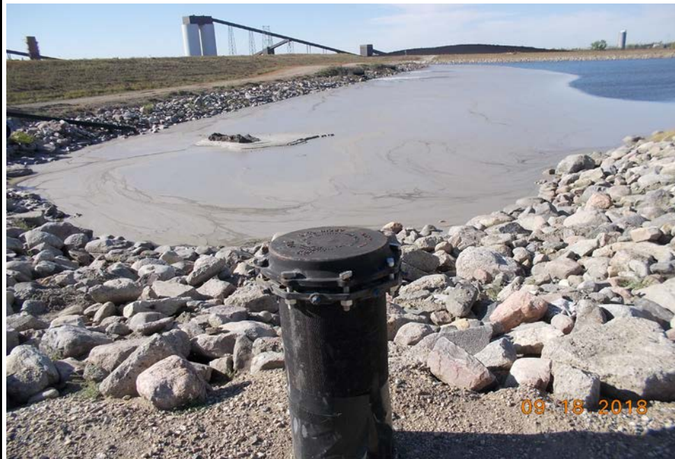
Photograph 20 (Center Cell upstream slope) Cross-over pipe riser and upstream slope riprap (1PDS.JPG)
