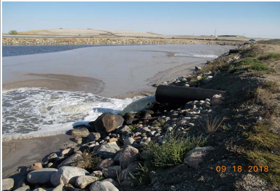
Photograph 25 (Center Cell upstream slope) Center cell upstream slope riprap and west cell decant piping outlet to the center cell (17PDS.JPG)
