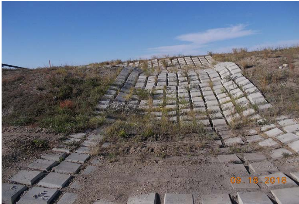
Photograph 23 (North upstream slope) Articulated Concrete Block (ACB) armored downchute channel (11PDS.JPG)
