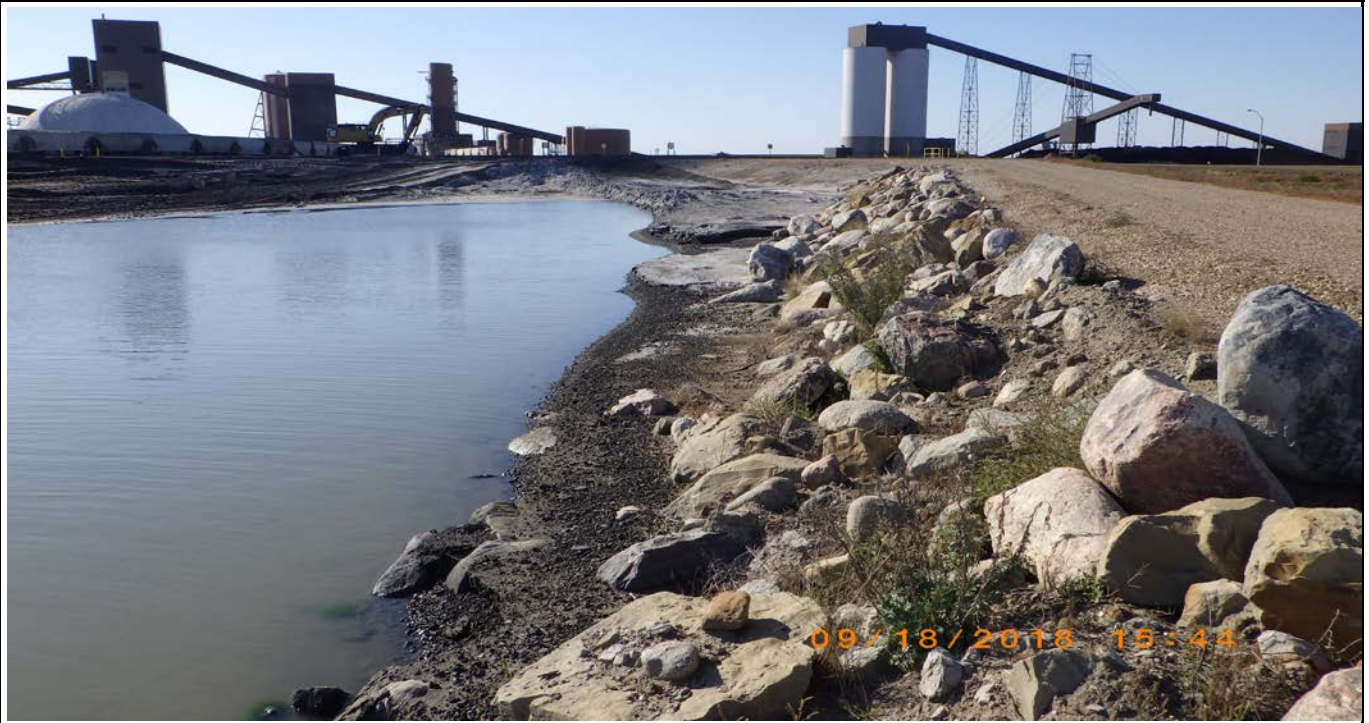
Photograph 15 (North berm upstream slope) West cell riprap on upstream slope (18ccs.JPG)
