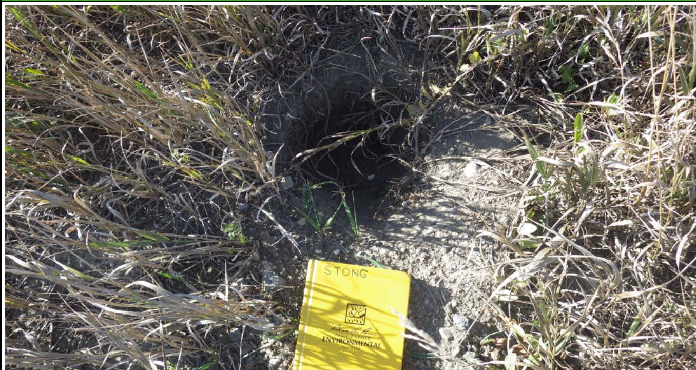
Photograph 5 (East berm downstream toe) Animal burrow at the downstream toe (IMGP6335.JPG)
