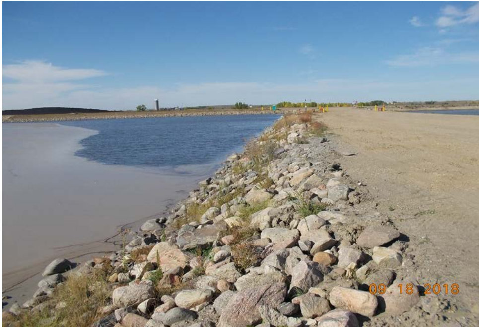
Photograph 21 (Center Cell upstream slope) Center cell upstream slope riprap (2PDS.JPG)
