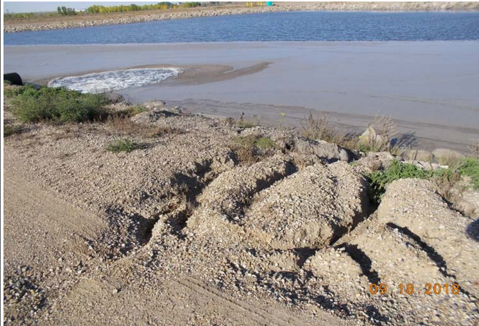
Photograph 26 (West/Center Cell crest road) Erosion of gravel surface on intercell-crest road between the west cell and the center cell (18PDS.JPG)
