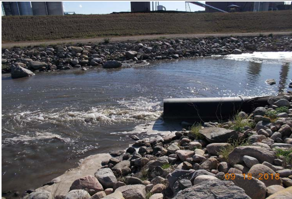
Photograph 24 (Center Cell upstream slope) Center cell upstream slope riprap and plant drains inflow pipe (14PDS.JPG)
