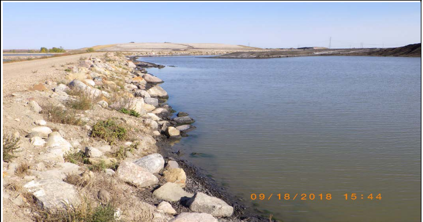
Photograph 17 (North berm upstream slope) West cell riprap on upstream slope (20ccs.JPG)
