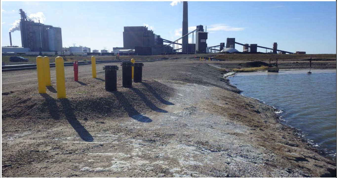
Photograph 1 (South berm crest) Cleanout and valve control for Upstream Raise 91 and east cell cross-over pipes (IMGP6327.JPG)
