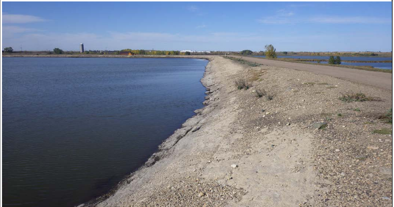
Photograph 2 (East berm upstream slope) Upstream slope fly ash protective cover (IMGP6328.JPG)
