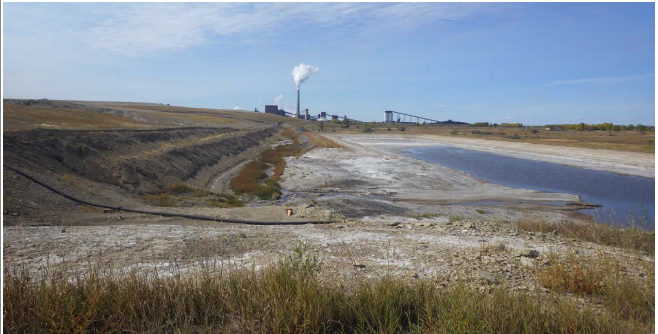
Photograph 1 (SE corner of contact water area (CWA)) Contact water collection area and seepage channel (IMGP6292.JPG)
