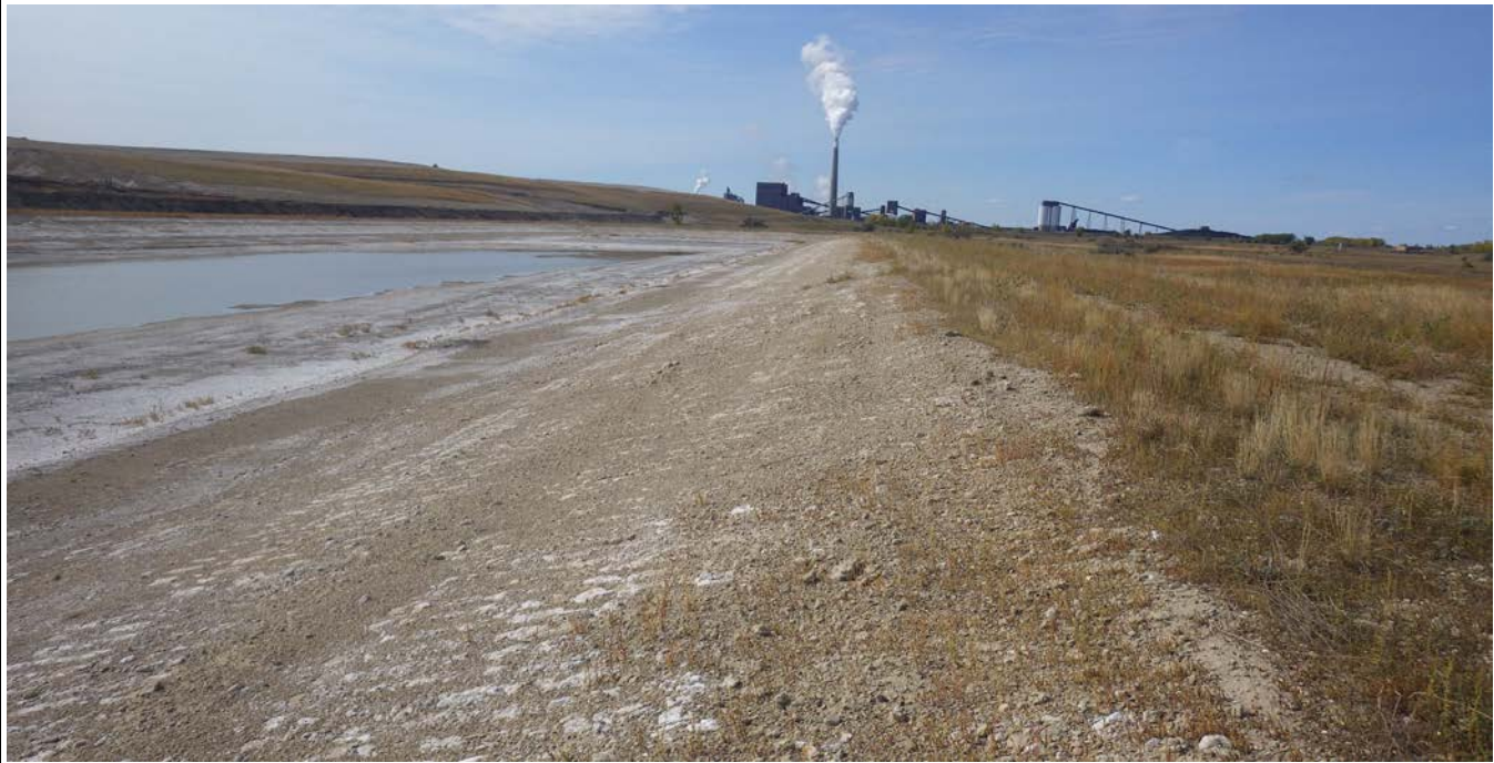
Photograph 3 (CWA north upstream slope) Fly ash protective cover on contact water collection area upstream slope (IMGP6295.JPG)
