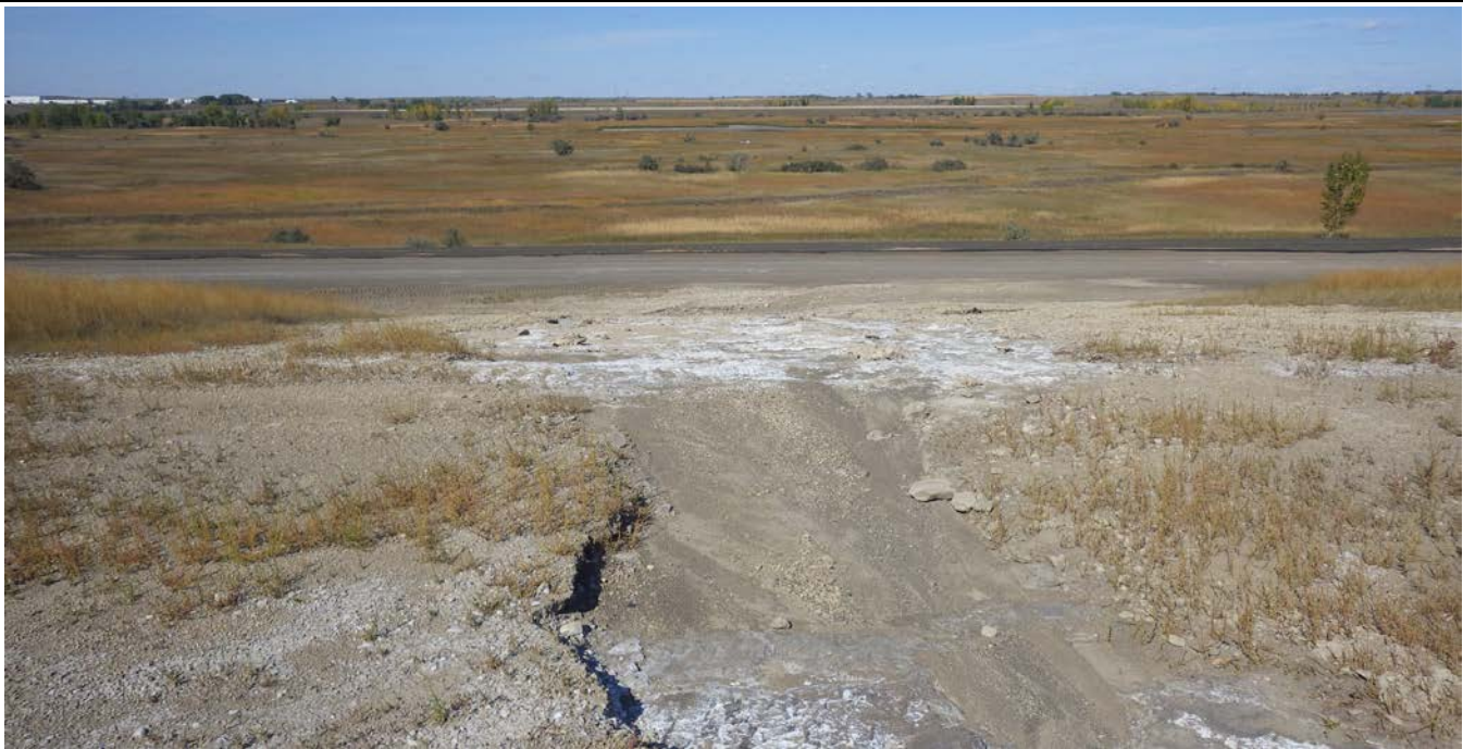
Photograph 8 (North CCR slope) Eroded fly ash slope due to channelized water flow (IMGP6318.JPG)
