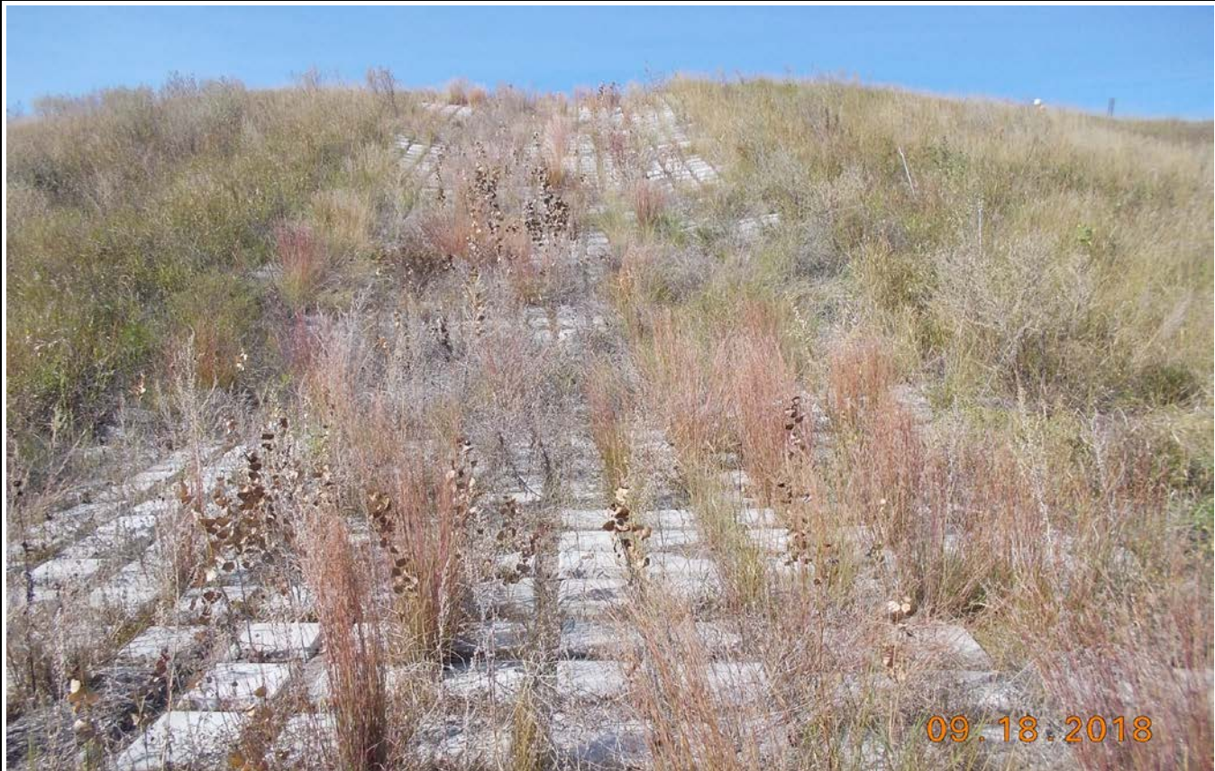
Photograph 25 (Southeast toe) Articulated Concrete Block (ACB) on southeast downstream slope (PDS 13 CCS SE16.JPG)
