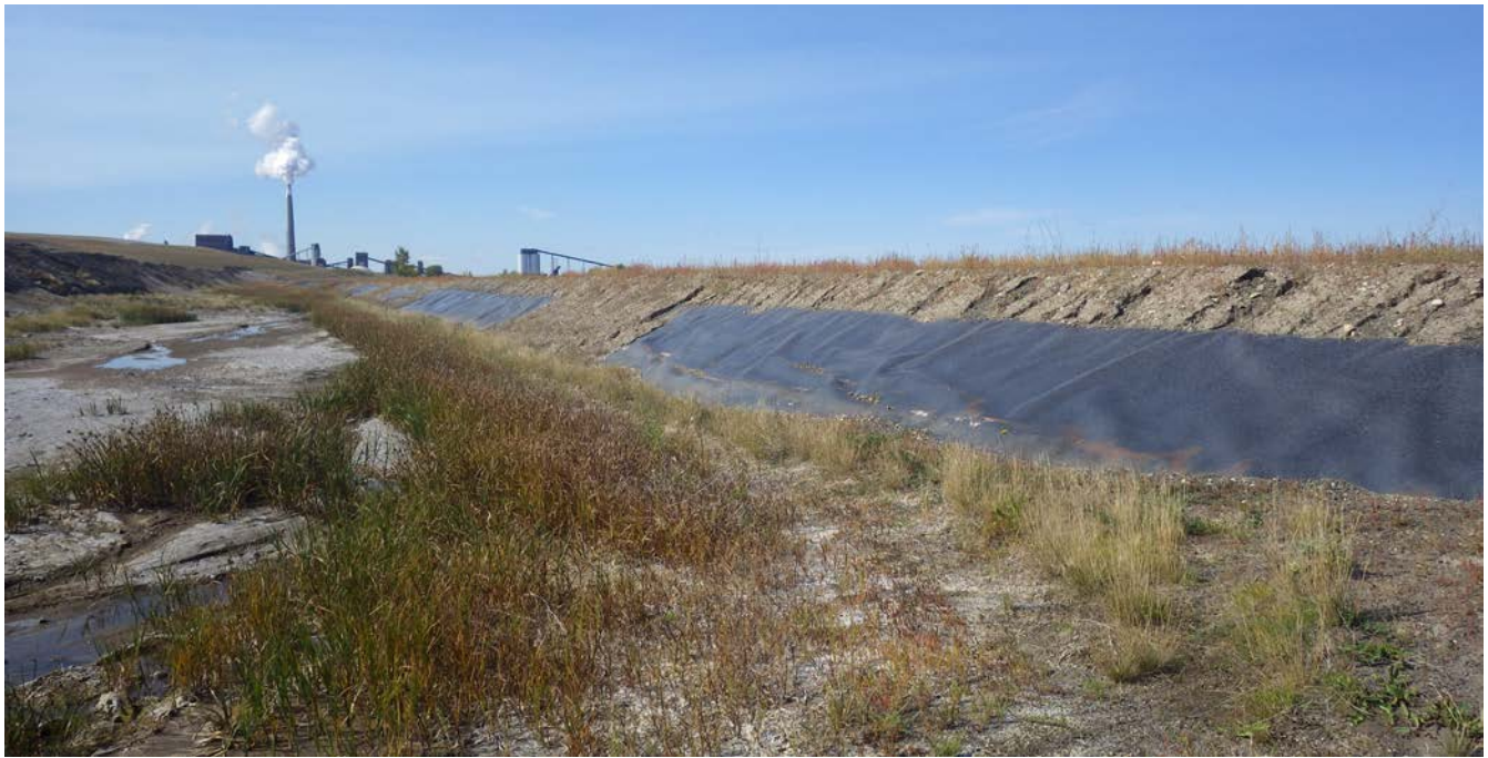
Photograph 5 (CWA ditch) Exposed geomembrane on upstream slope (IMGP6303.JPG)
