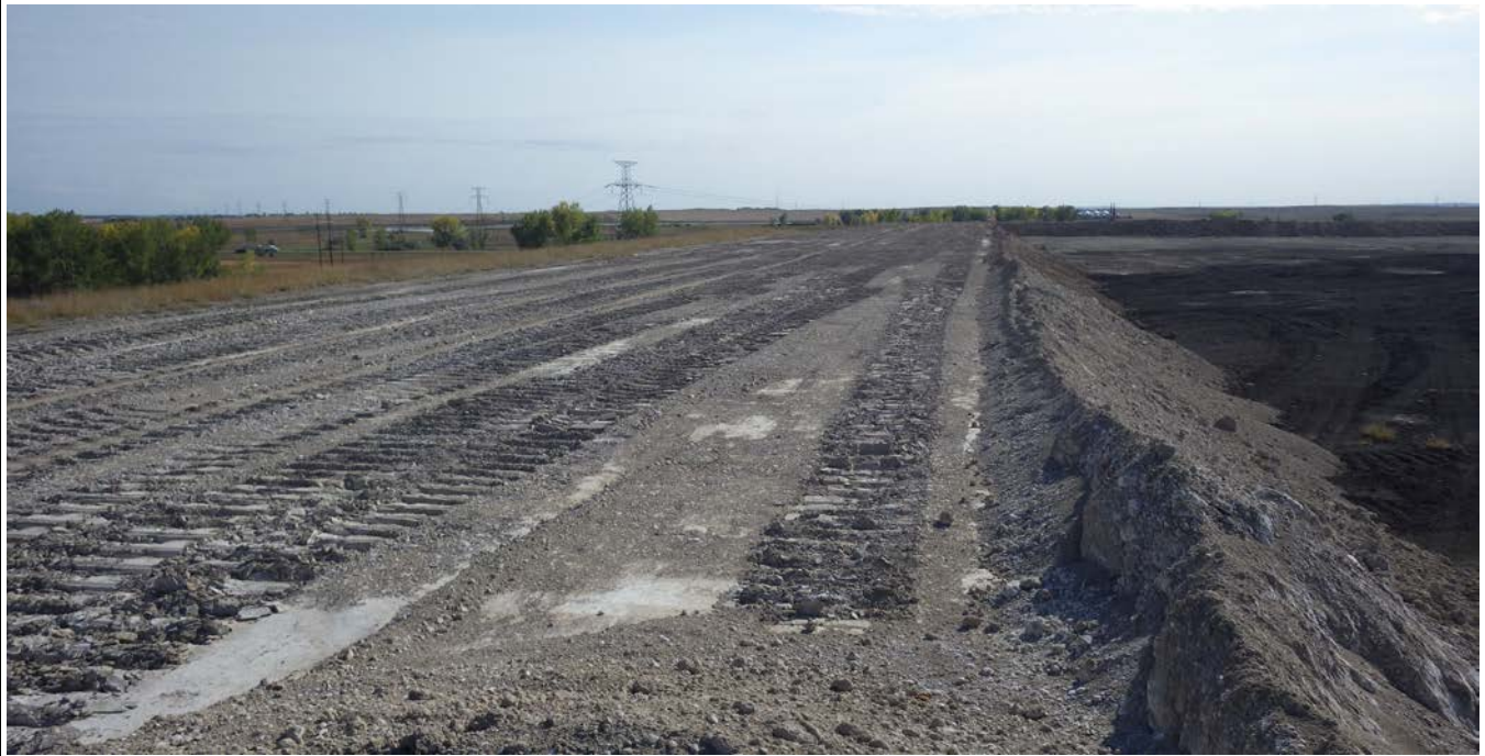
Photograph 11 (CCR placement) Fly ash berm around rejects placement (approximately 35-40 feet wide) (IMGP6325.JPG)
