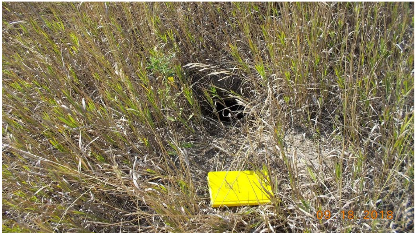
Photograph 24 (East downstream toe) Animal burrow near downstream toe (PDS 10 CCS SE16.JPG)
