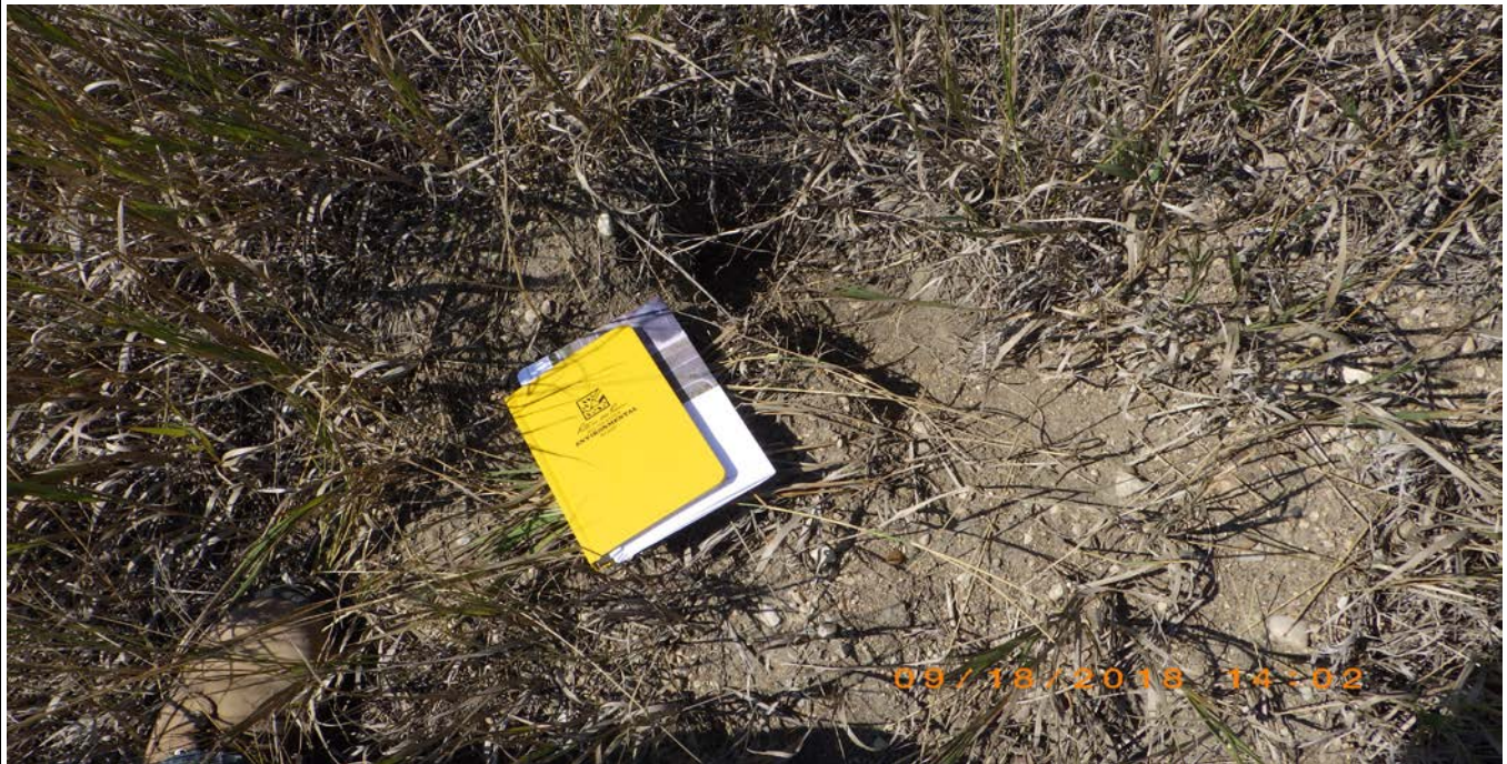
Photograph 19 (South downstream slope) Animal burrow on downstream slope (29ccs.JPG)
