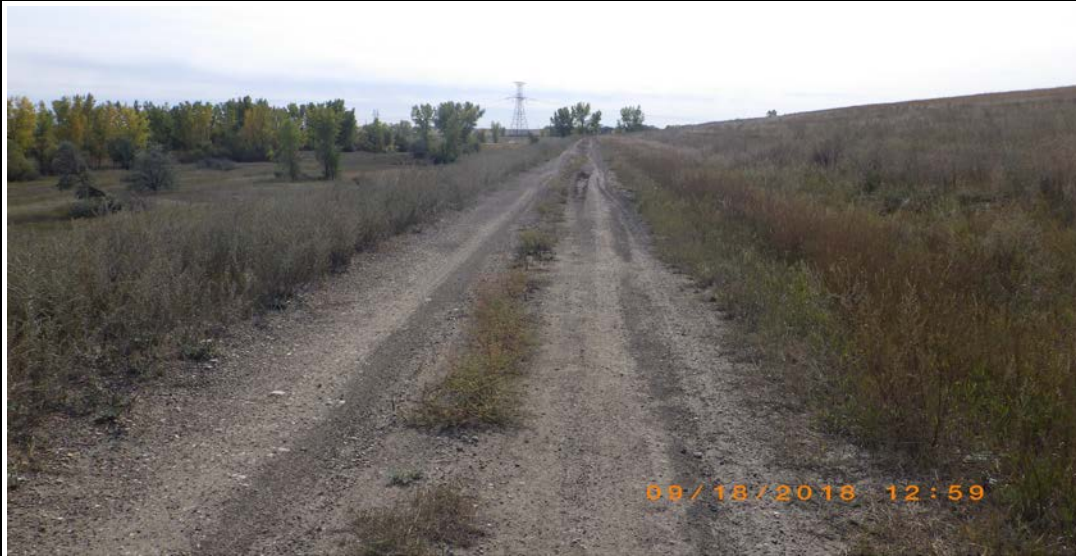
Photograph 13 (East downstream slope access road) Minor rutting of berm crest perimeter access road (4ccs.JPG)
