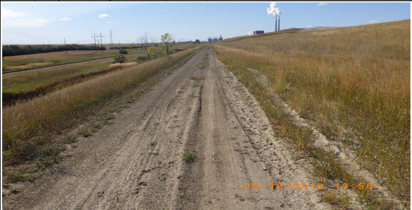
Photograph 18 (South downstream access road) Minor rutting of berm crest perimeter access road (25ccs.JPG)
