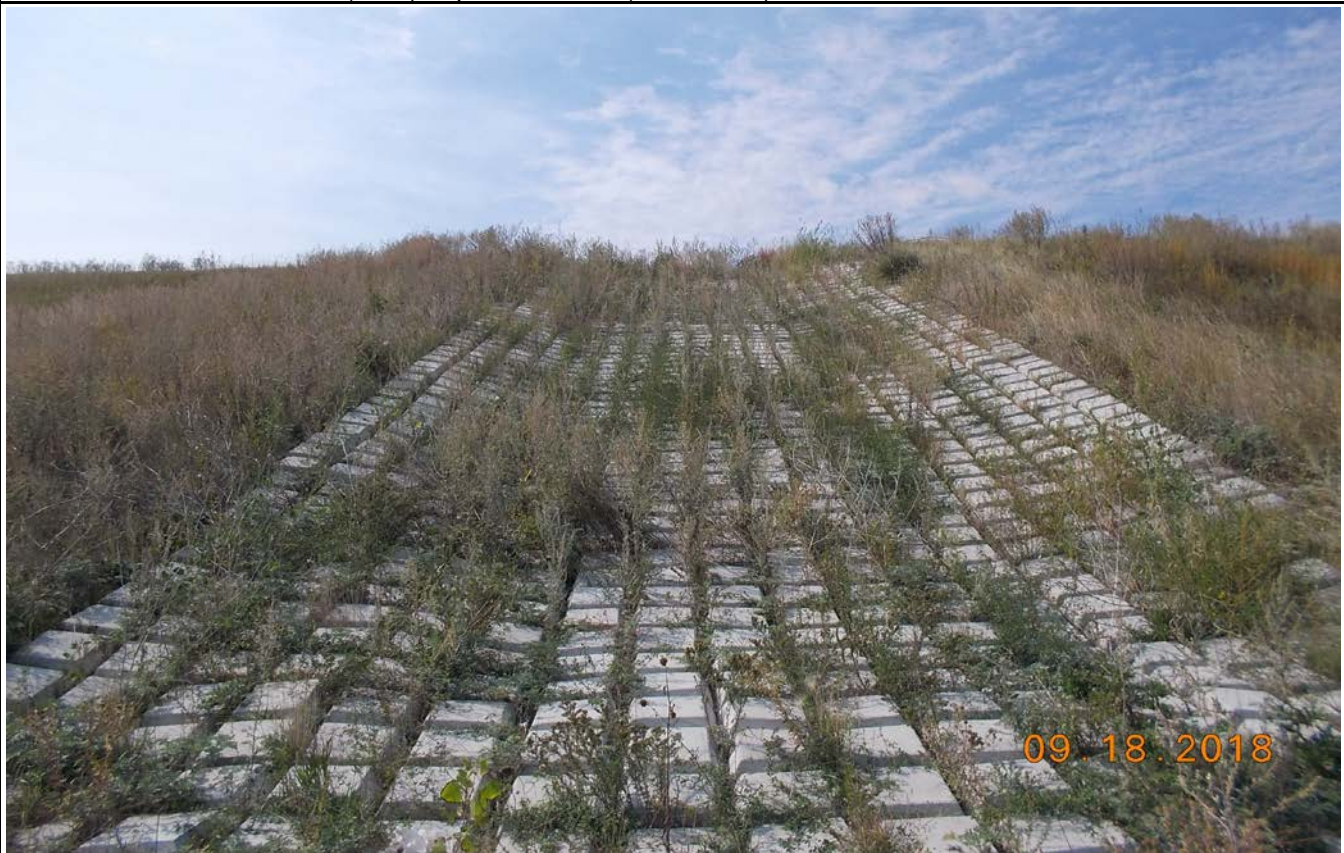
Photograph 22 (Northeast corner) Articulated Concrete Block (ACB) on northeast downstream slope (PDS 1 CCS SE16.JPG)
