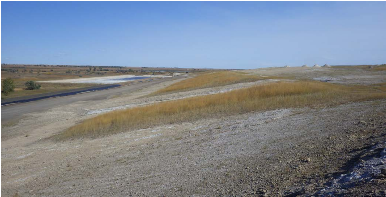
Photograph 7 (North CCR slope) Temporary cover on north fly ash slope (IMGP6317.JPG)
