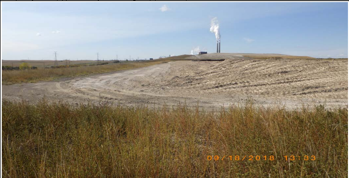
Photograph 16 (Southeast CCR crest) Southwest Section 16 fly ash slope and contact water ditch at top of temporary cover (16ccs.JPG)
