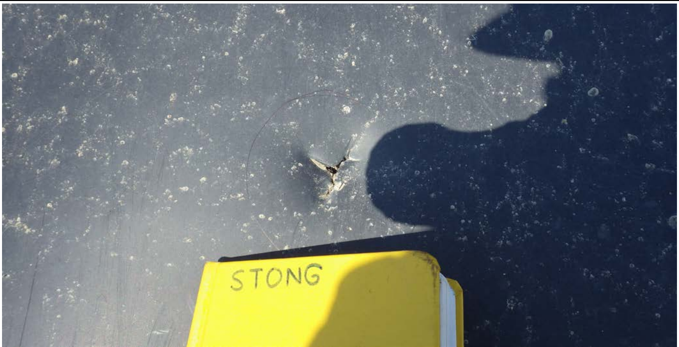
Photograph 6 (CWA ditch) Damage to exposed geomembrane on upstream slope (not in-contact with water) (IMGP6305.JPG)
