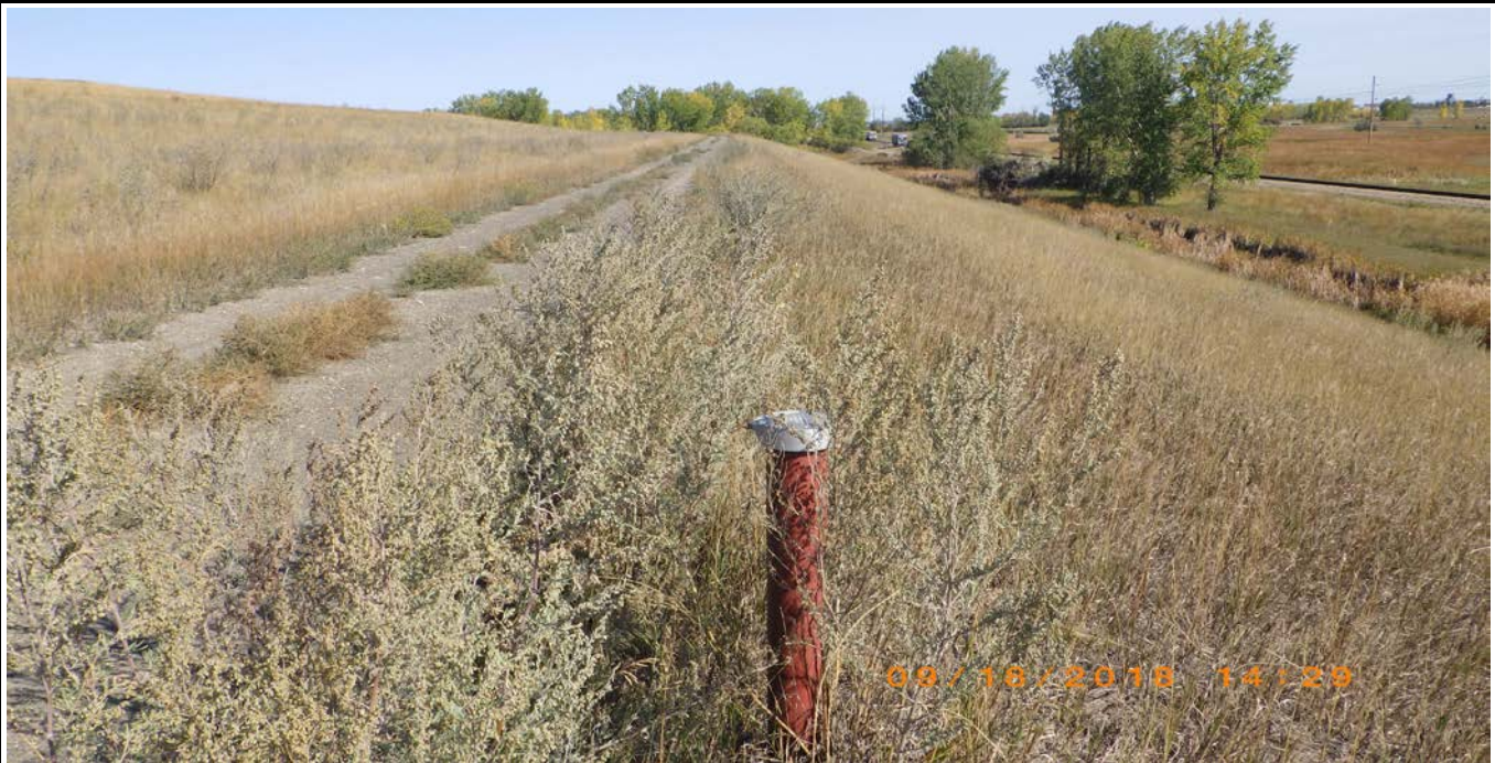
Photograph 20 (South downstream slope) Piezometer near berm crest perimeter access road and downstream slope vegetation (31ccs.JPG)
