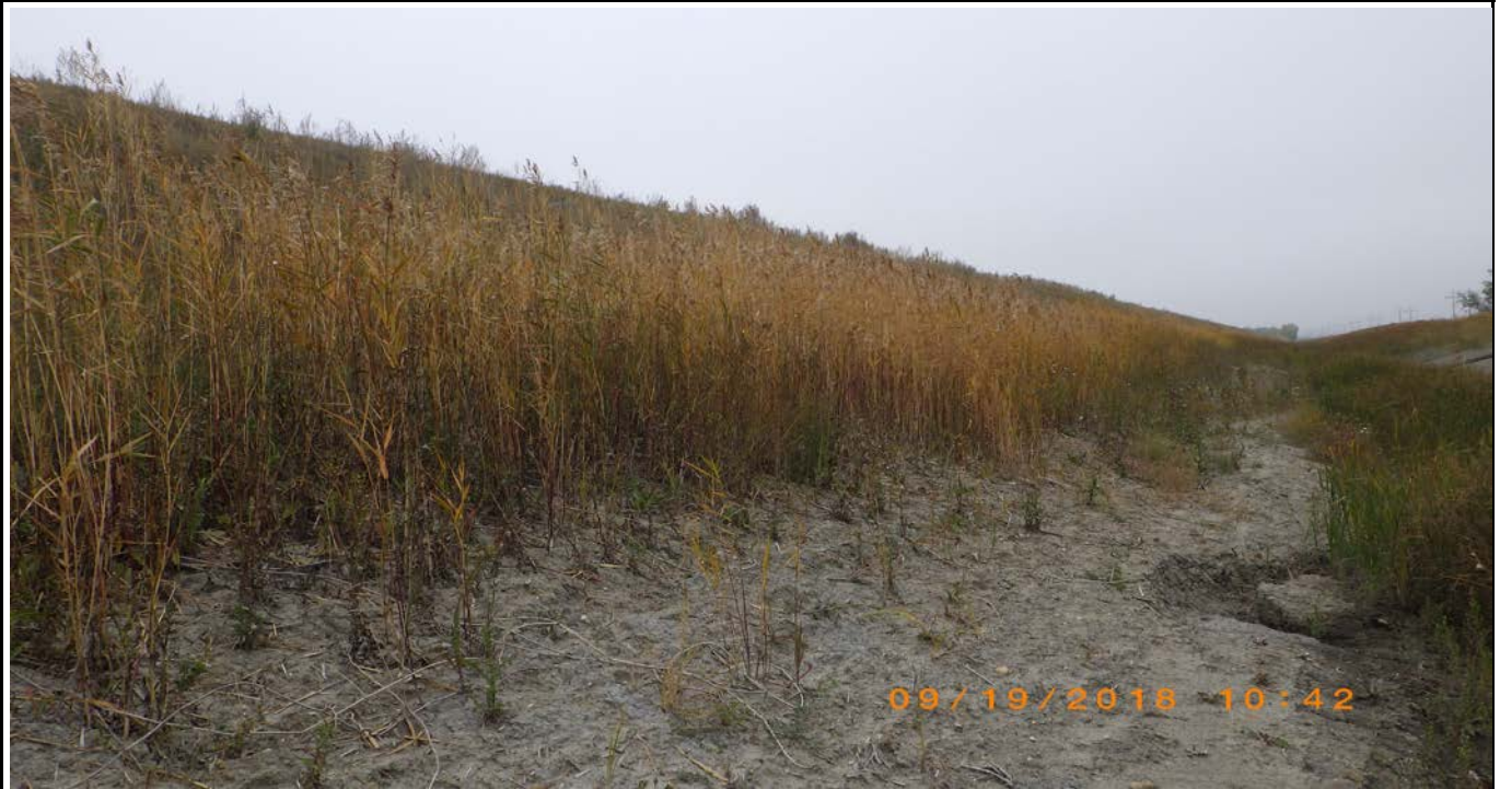
Photograph 16 (South toe) Sparse vegetation on south downstream slope near the toe (21ccs.JPG)
