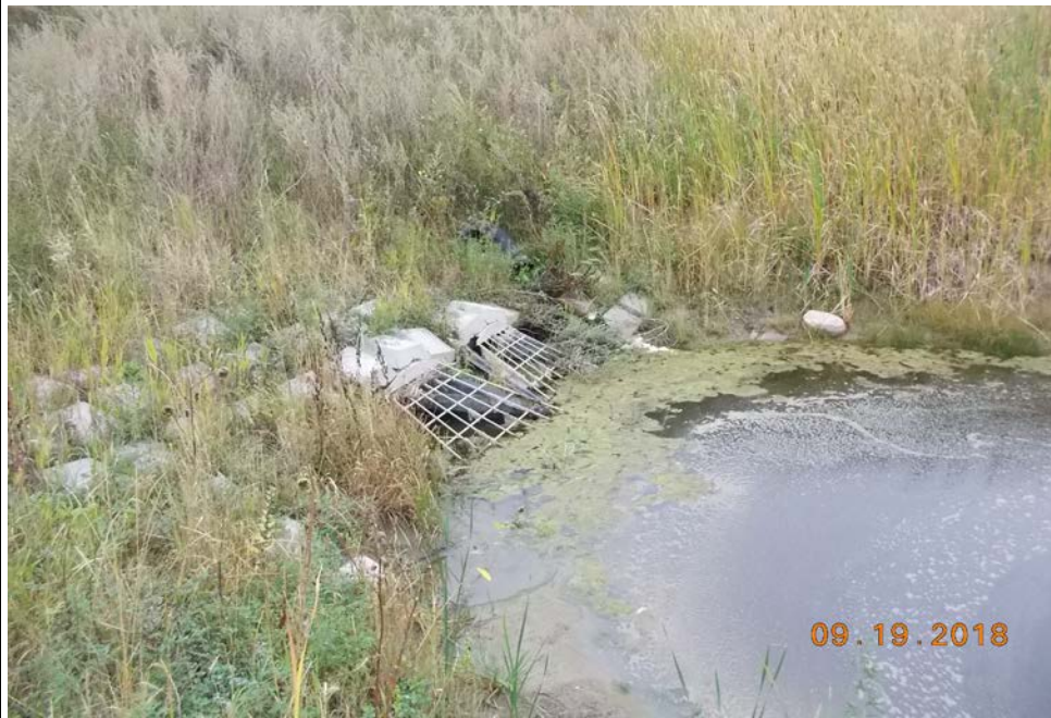
Photograph 19 (West toe and ditch) Inlet side of surface water drainage culvert on west side of Upstream Raise 91 (2PDS.JPG)
