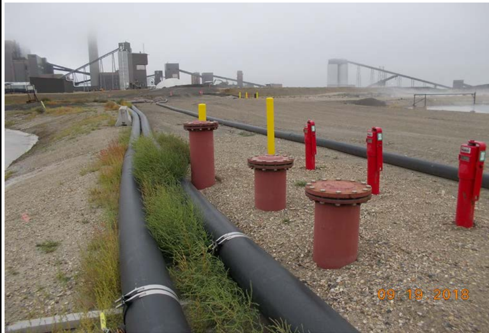
Photograph 23 (North berm upstream slope) Cleanouts and valve controls for Upstream Raise 91 to Drains Pond System cross-over pipes (14PDS.JPG)
