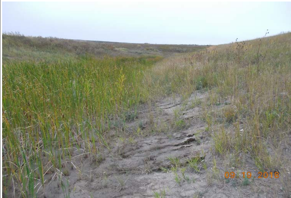
Photograph 21 (West downstream slope) Minor erosion and sparse vegetation on west downstream slope (10PDS.JPG)
