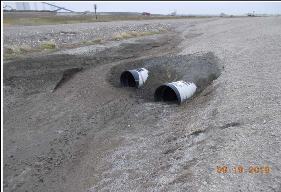
Photograph 24 (West upstream slope) Perimeter channel contact water culverts (20PDS.JPG)
