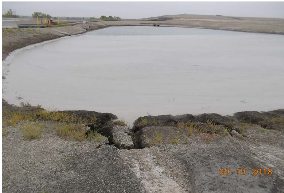
Photograph 22 (NW crest and pond) Minor erosion of fly ash shell near northwest corner of Upstream Raise 91 (12PDS.JPG)
