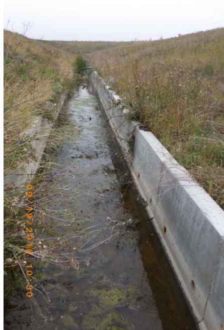
Photograph 14 (South toe) Approximately 1 foot of water in concrete surface water drainage (15ccs.JPG)
