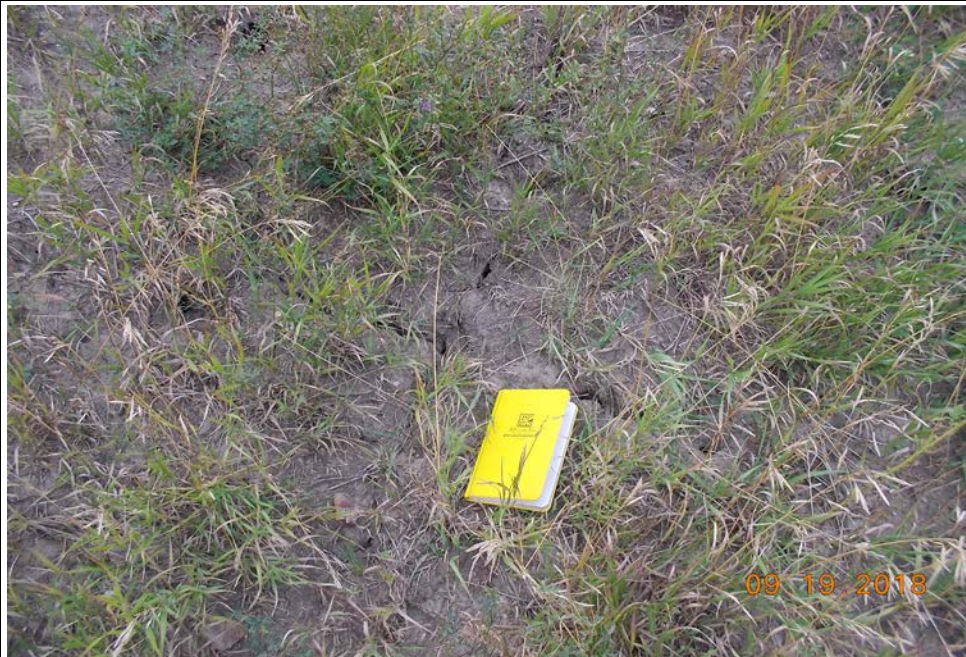
Photograph 20 (West downstream slope) Minor erosion and sparse vegetation on west downstream slope (5PDS.JPG)
