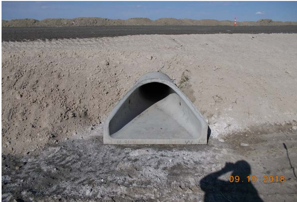
Photograph 24 (North contact water ditch and haul road) Recently installed concrete culvert under north haul road (25PDS.JPG)
