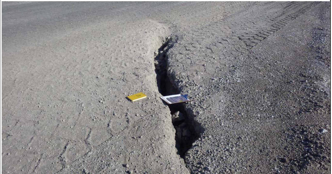
Photograph 10 (North CCR downstream slope) Crack in fly ash CCR crest (approximately 10 inches wide) (IMG6427.JPG)
