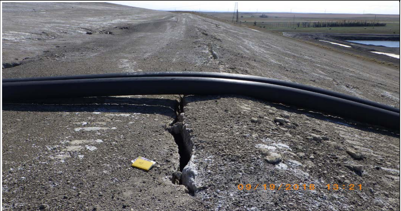
Photograph 12 (West CCR downstream slope) Crack on CCR downstream slope bench at elevation 1974 feet (approximately 6 inches wide, 6 feet deep, 6 inches offset vertically) (6ccs.JPG)
