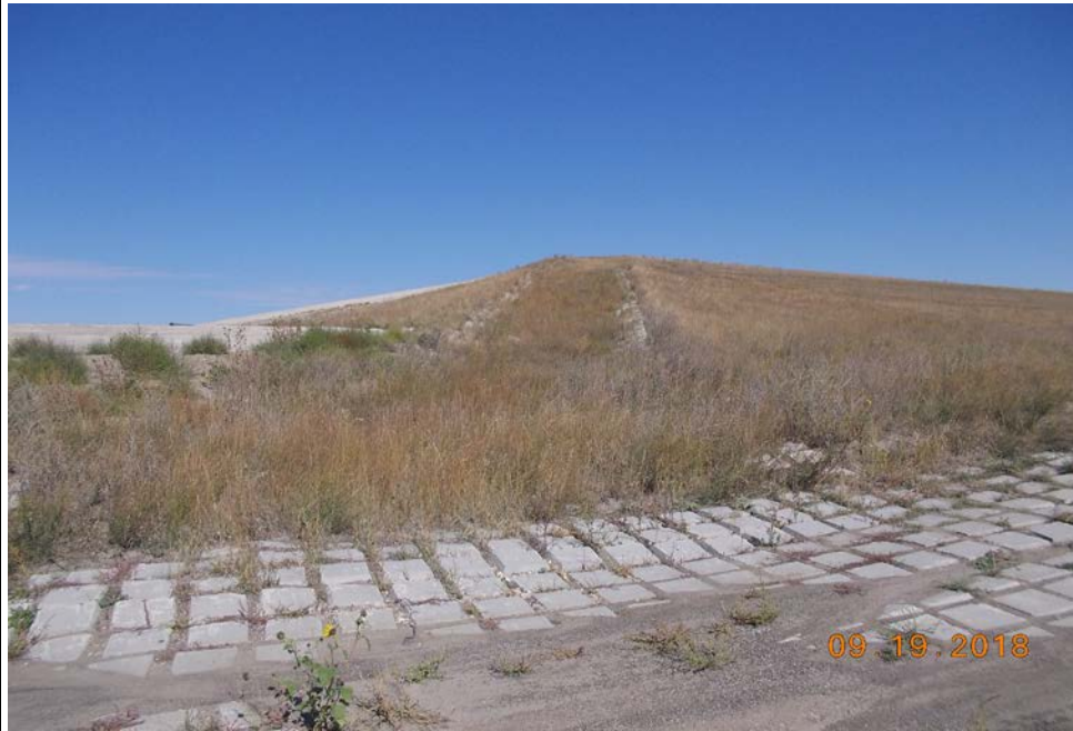
Photograph 21 (SW CCR covered downstream slope) Articulated Concrete Block (ACB) downchute, thick vegetation between blocks along the slope (1PDS.JPG)
