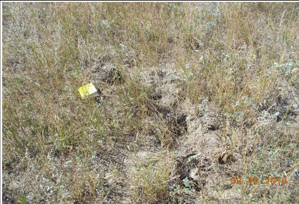
Photograph 22 (South CCR downstream slope) Animal burrows near the perimeter road on the CCR downstream slope (9PDS.JPG)
