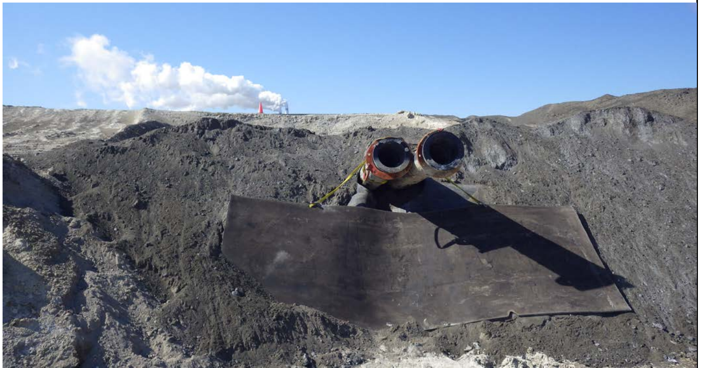
Photograph 2 (West CCR upstream slope) Gravity drain outlet pipes (IMGP6390.JPG)
