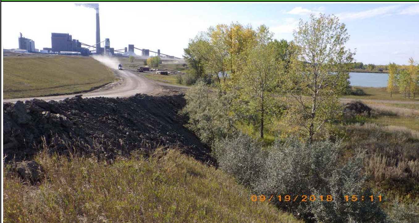
Photograph 19 (North berm downstream slope and haul road) Steep downstream slope below recently re-constructed haul road ramp (66ccs.JPG)
