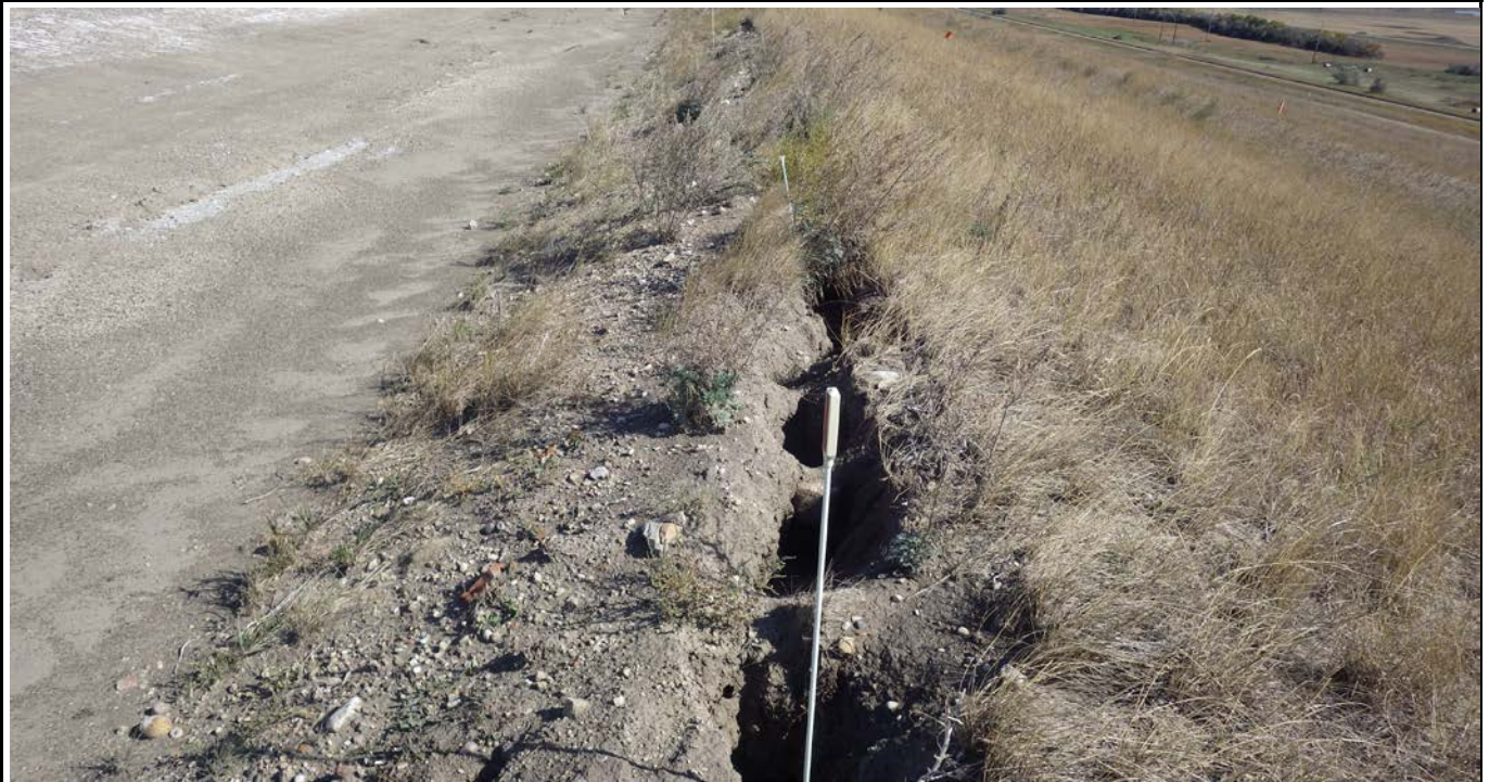
Photograph 5 (South CCR covered downstream slope) Cracking of the final cover slope near the bench at elevation 1974 feet (IMGP6397.JPG)
