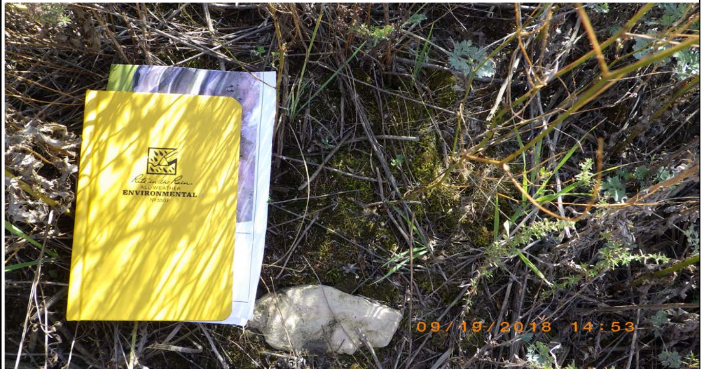
Photograph 18 (North downstream slope) Mossy vegetation in grass (no seepage) (56ccs.JPG)
