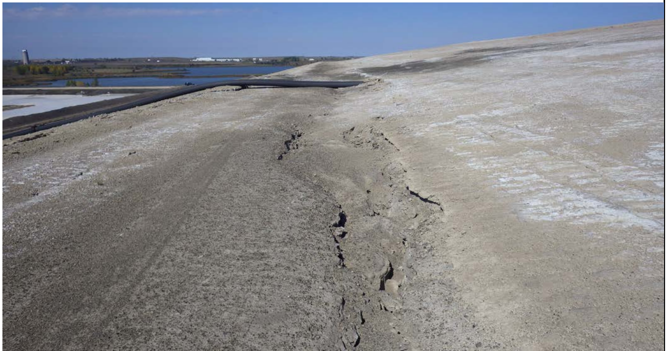
Photograph 3 (West CCR downstream slope) Crack and erosion in fly ash CCR downstream slope (IMGP6392.JPG)
