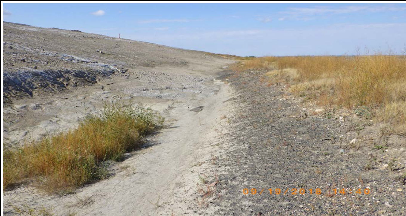
Photograph 16 (East CCR downstream slope) Contact water ditch at elevation 1950 feet on east CCR downstream slope (48ccs.JPG)
