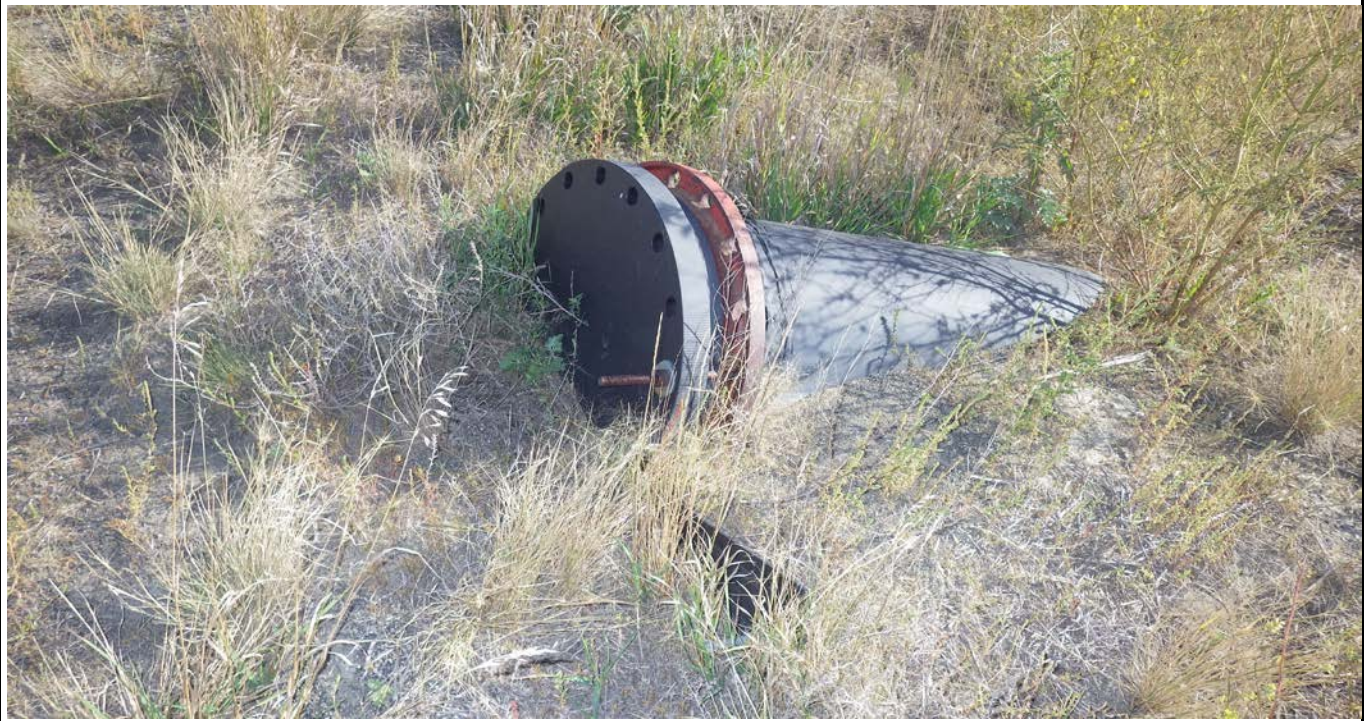
Photograph 11 (North CCR downstream slope) Sump riser on east half of Upstream Raise 92 (IMGP6429.JPG)
