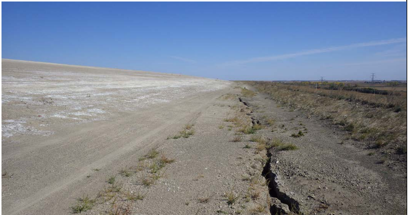
Photograph 4 (South CCR downstream slope) Crack in fly ash bench (within the contact water separation channel) (IMGP6395.JPG)
