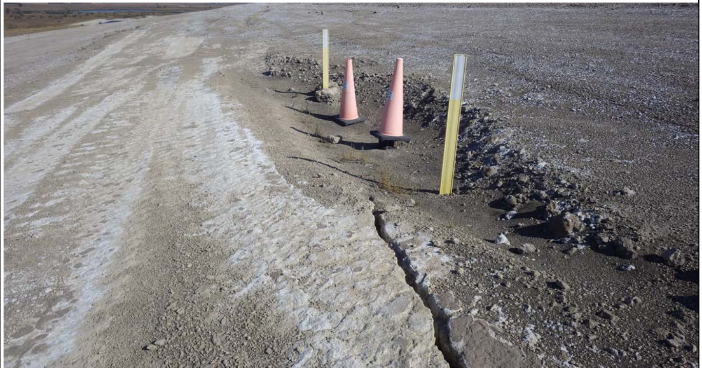
Photograph 9 (North CCR downstream slope) Crack in fly ash near piezometers (IMG6425.JPG)
