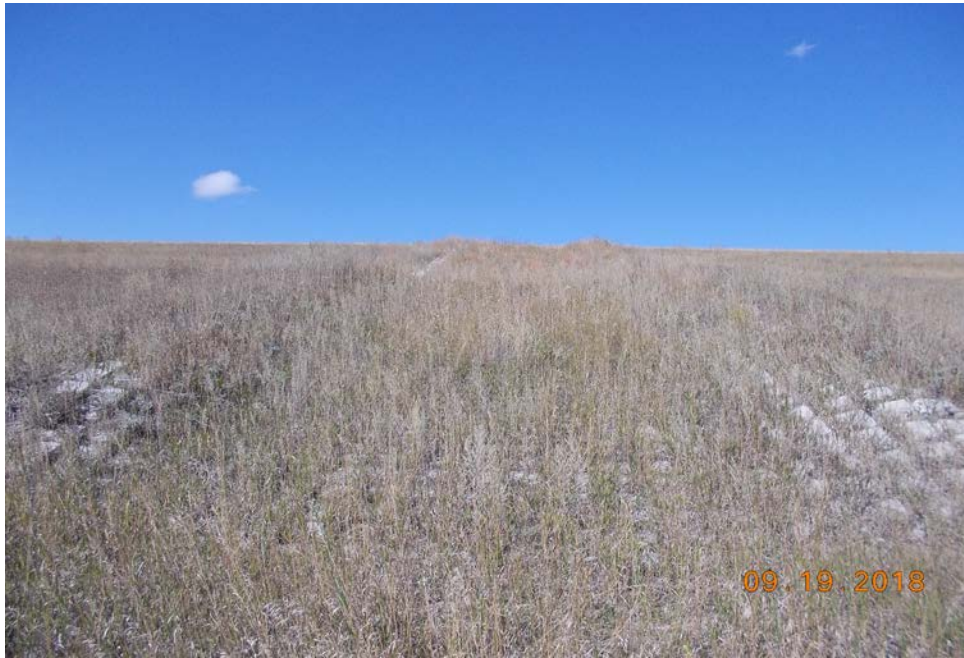
Photograph 23 (South CCR covered downstream slope) Articulated Concrete Block (ACB) downchute on covered CCR downstream slope (19PDS.JPG)
