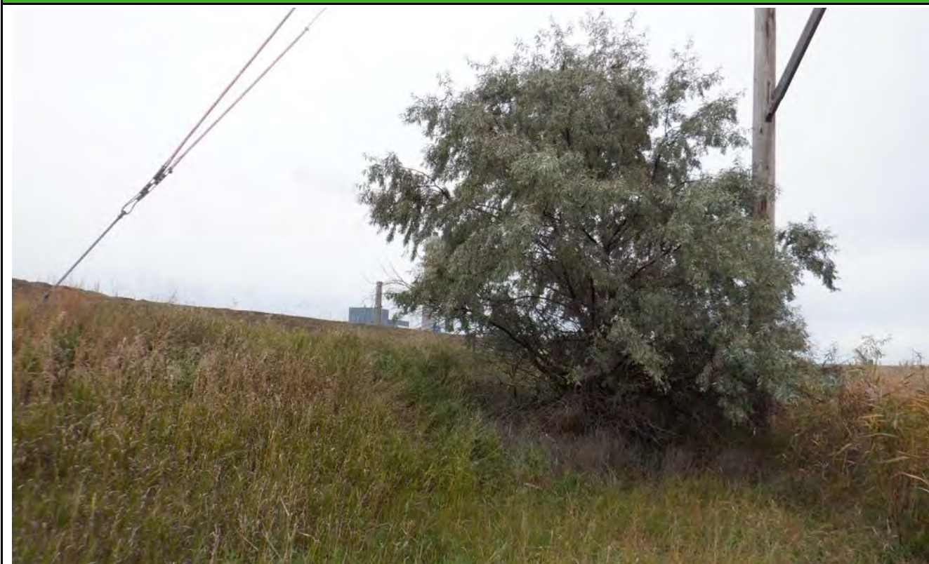
Photograph 7 (South downstream slope) Tree to be removed with site restoration activities (DSCF0628.JPG)
