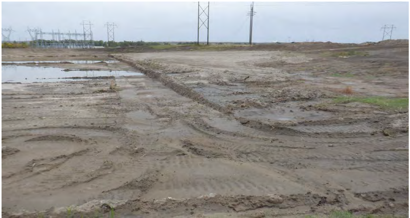
Photograph 6 (South berm crest) Approximate west end of consolidated Bottom Ash Landfill footprint to be closed with permitted material remaining in place (containment berm to be constructed as part of site restoration) (DSCF0626.JPG)
