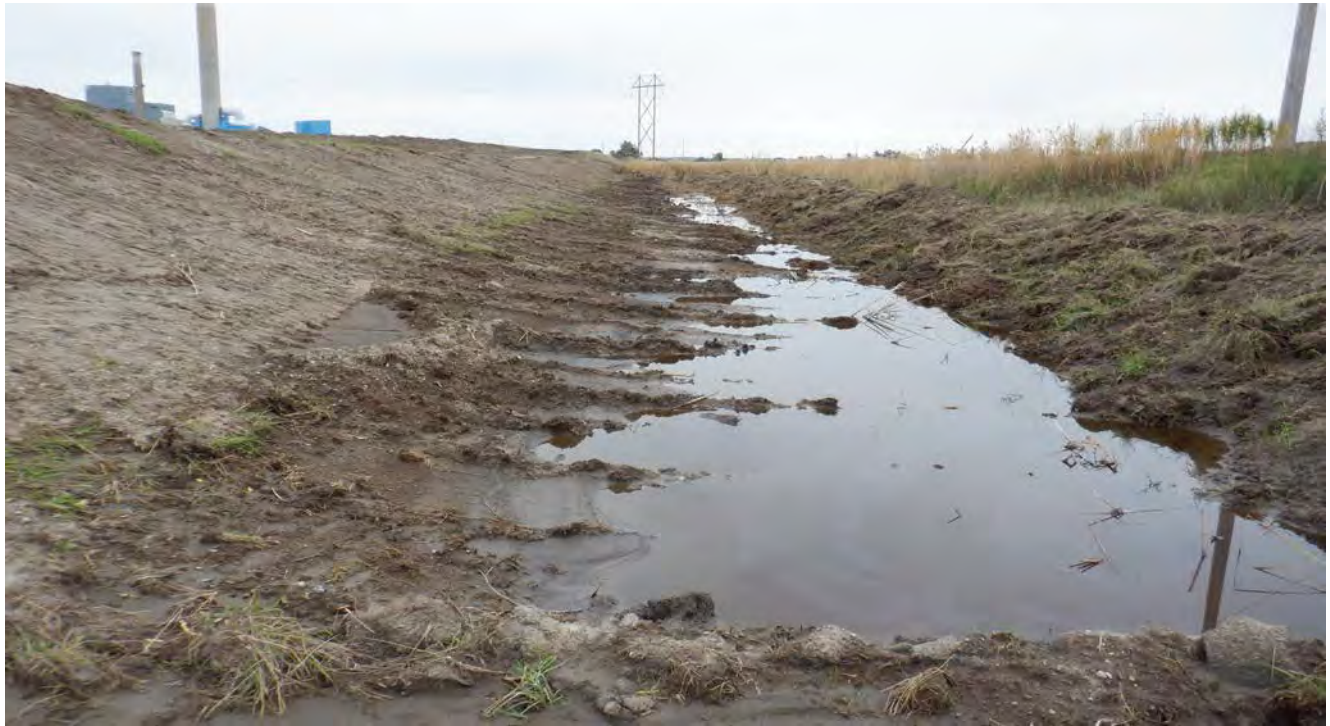
Photograph 5 (South downstream slope) South downstream slope and surface water ditch (previously cleared and grubbed as part of restoration) (DSCF0625.JPG)
