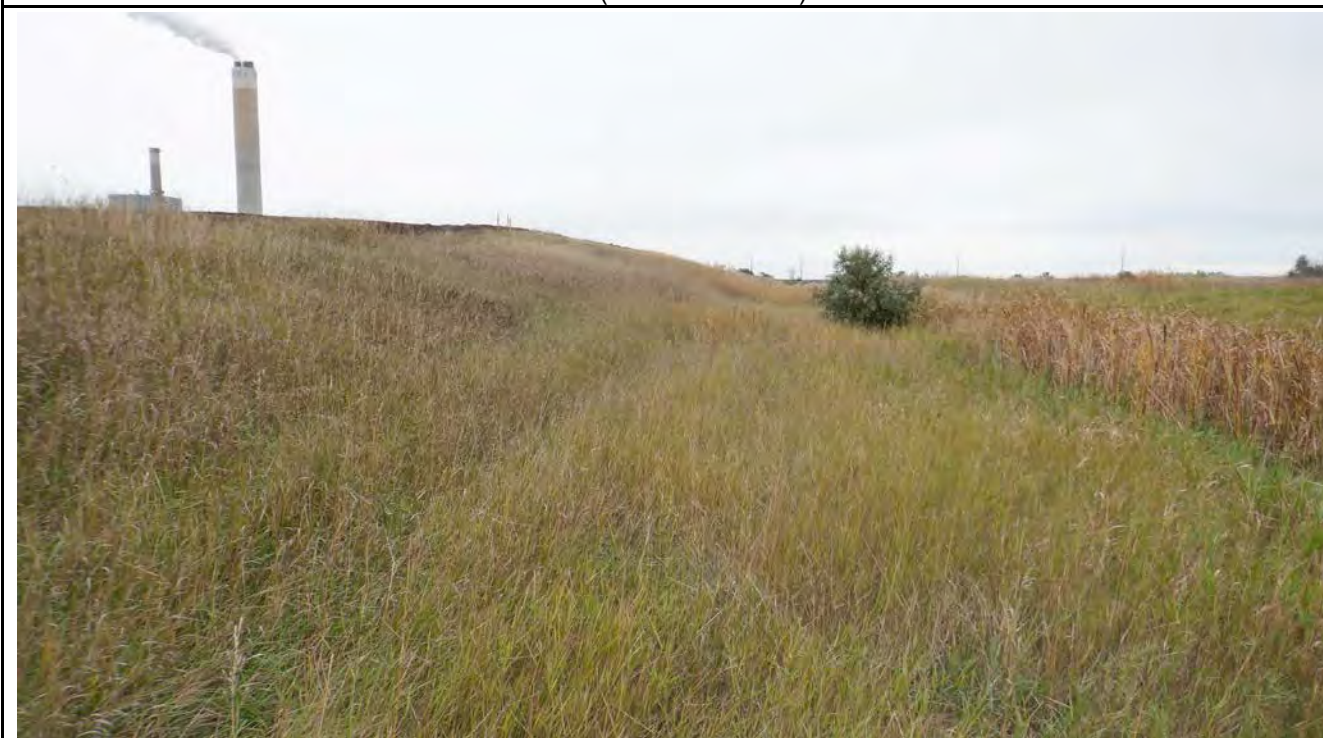
Photograph 8 (South downstream slope) Grass vegetation on the south downstream slope and woody vegetation to be removed as part of site restoration (DSCF0630.JPG)
