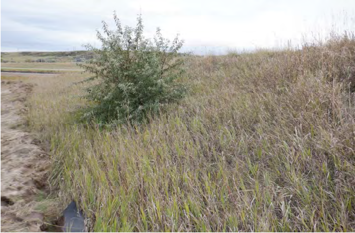
Photograph 9 (East downstream slope) Woody vegetation on east downstream slope of south cell (DSCF0656.JPG)
