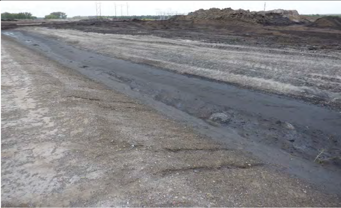
Photograph 11 (South berm crest) Interior of south cell (contact water control ditch and grading to achieve top of waste grades in preparation for closure) (DSCF0660.JPG)
