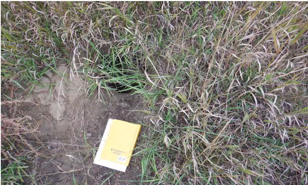
Photograph 12 (South downstream slope) Large animal burrow on south downstream slope (DSCF0662.JPG)
