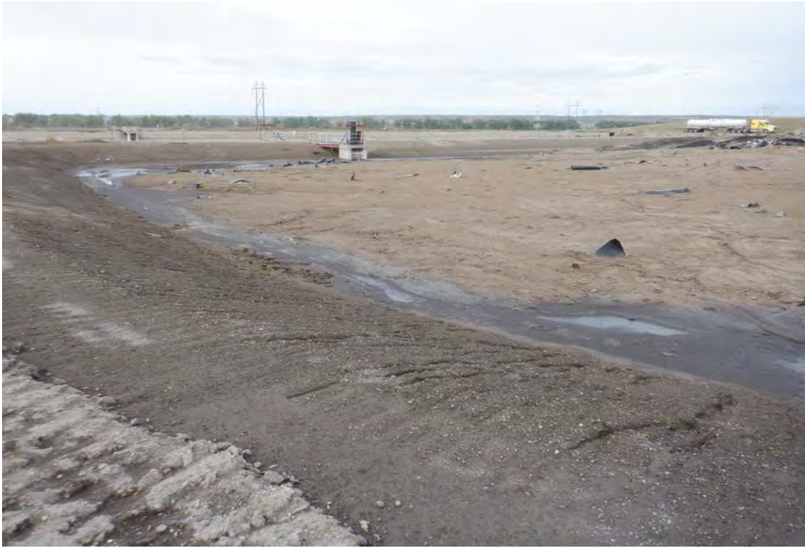
Photograph 13 (SW south cell berm crest) Interior of south cell (CCR, CCR mixed soils, and geomembrane liner being placed to achieve closure grades during restoration activities) and south cell dewatering sump shown in the background at the existing concrete outfall structure (DSCF0663.JPG)
