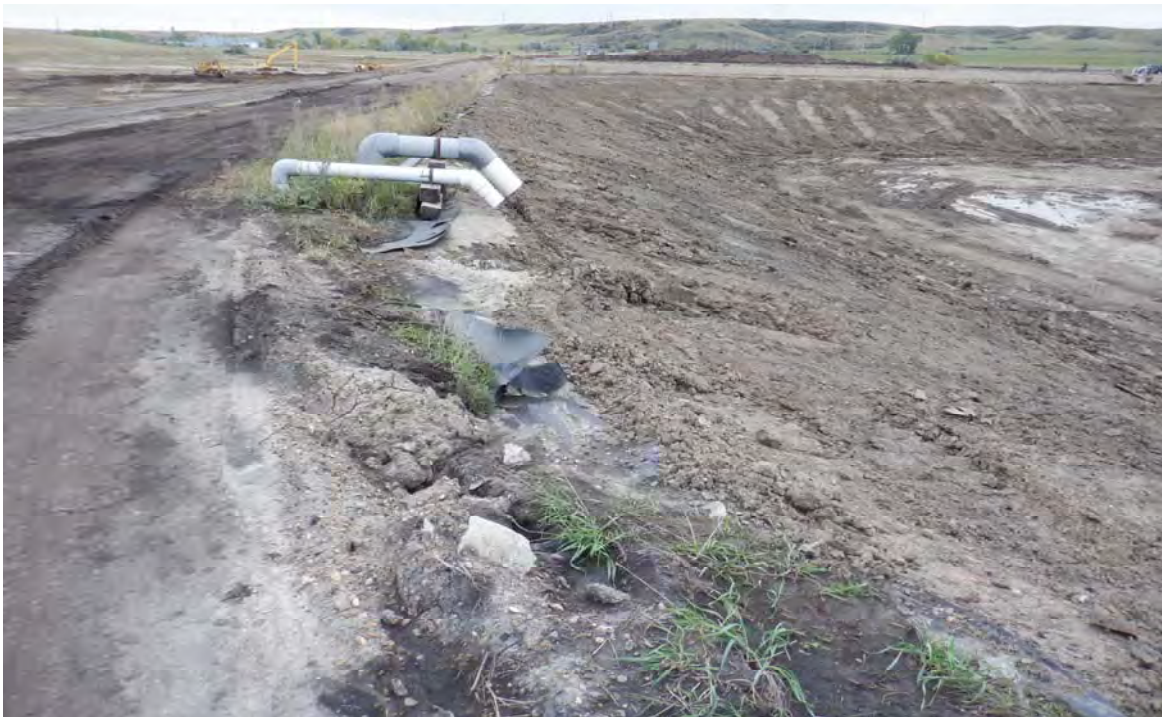
Photograph 4 (NE berm crest) Historic inflow to the north cell (to be removed during restoration activities) (DSCF0645.JPG)
