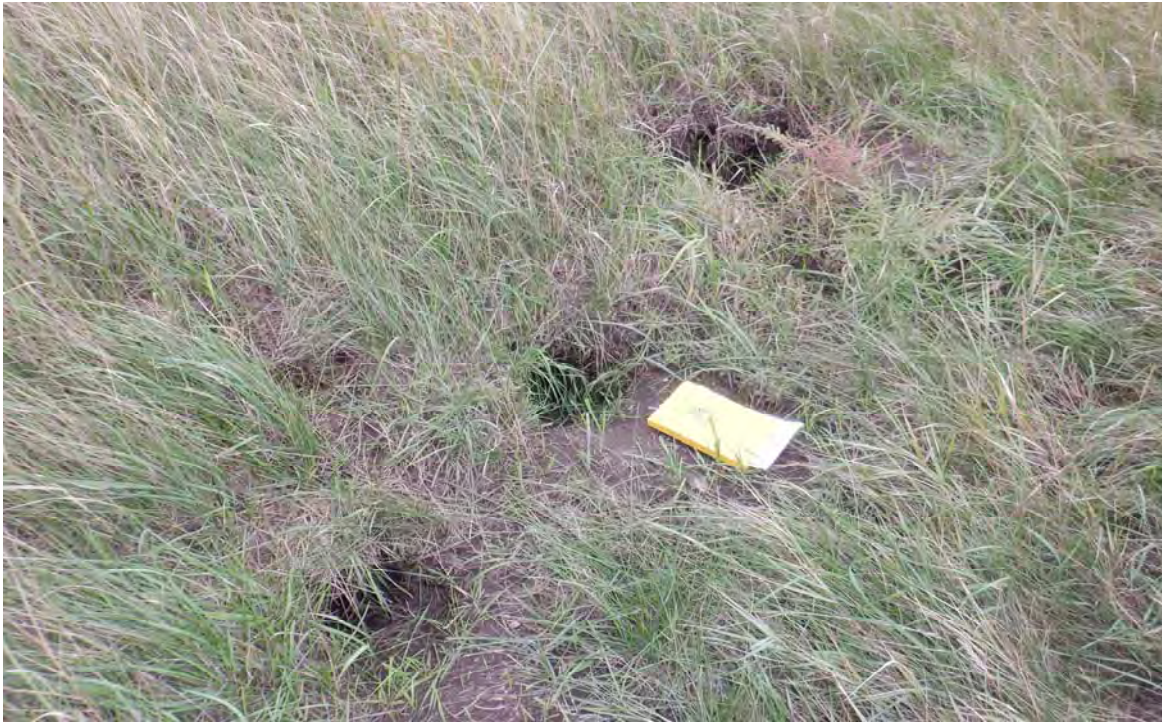
Photograph 3 (North upstream slope) Animal burrows on north downstream slope (DSCF0643.JPG)
