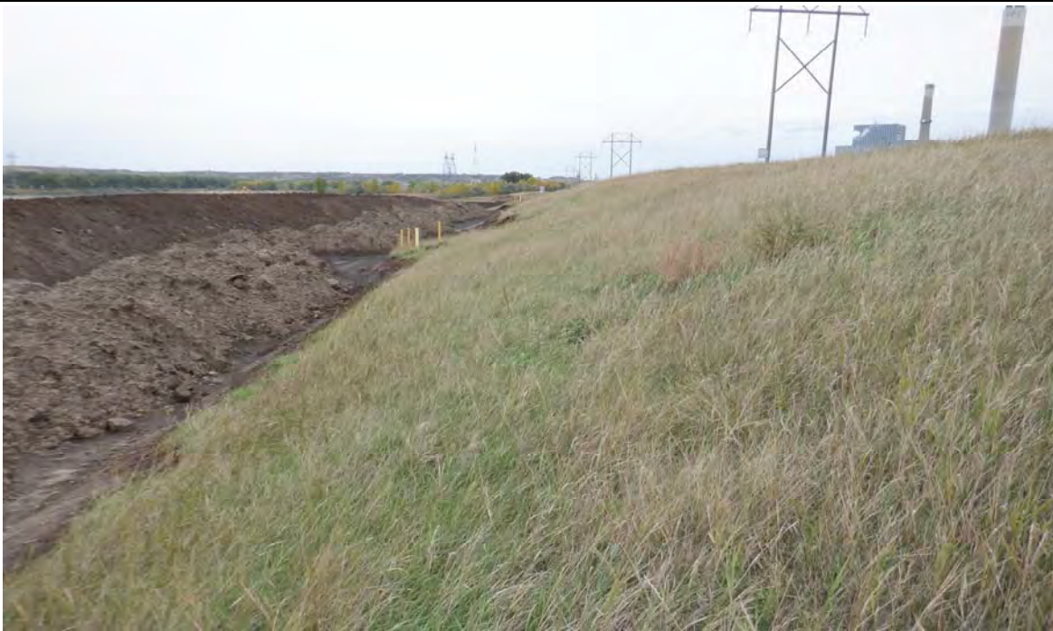
Photograph 2 (North downstream slope) Grass vegetation on north downstream slope and temporary stockpile at toe of slope related to site restoration activities (DSCF0641.JPG)
