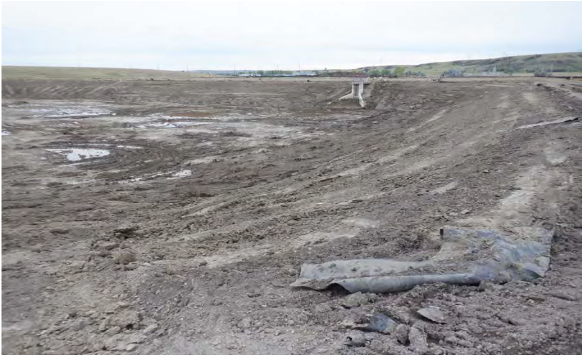
Photograph 1 (NW berm crest) Interior of north cell (bottom ash and liner system removed during restoration activities) (DSCF0639.JPG)
