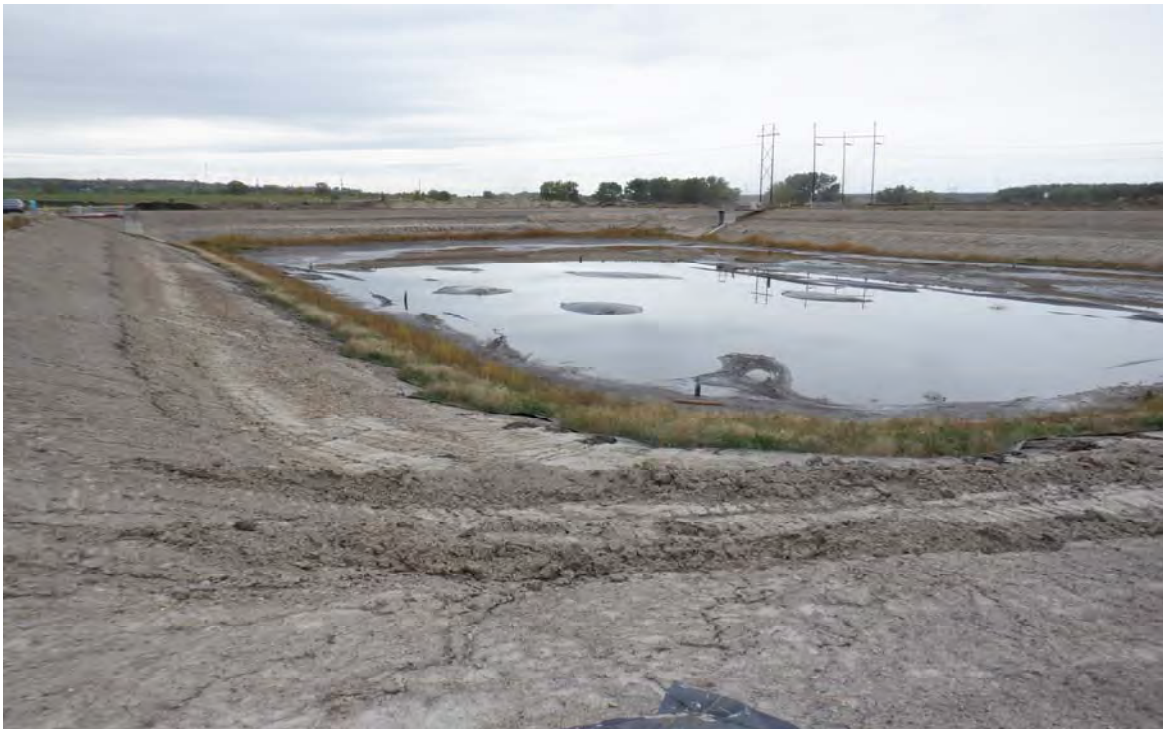
Photograph 6 (SE center cell berm crest) Interior of center cell (actively being dewatered during the inspection and geomembrane liner on side slopes removed as a part of restoration) (DSCF0650.JPG)
