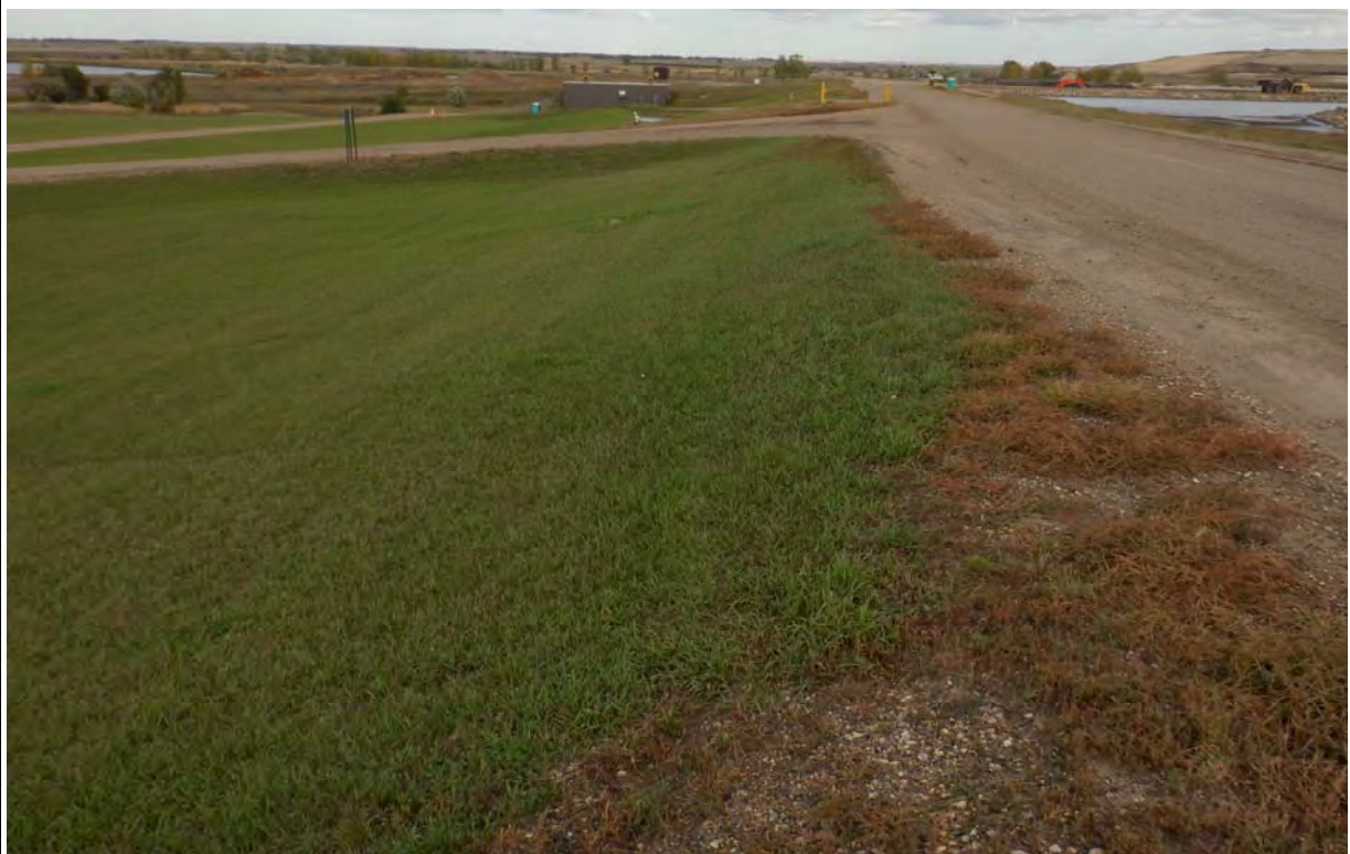
Photograph 12 (West cell north downstream slope and berm crest) Haul road and downstream slope of berm in good condition (typical) (DSCF0523.JPG)
