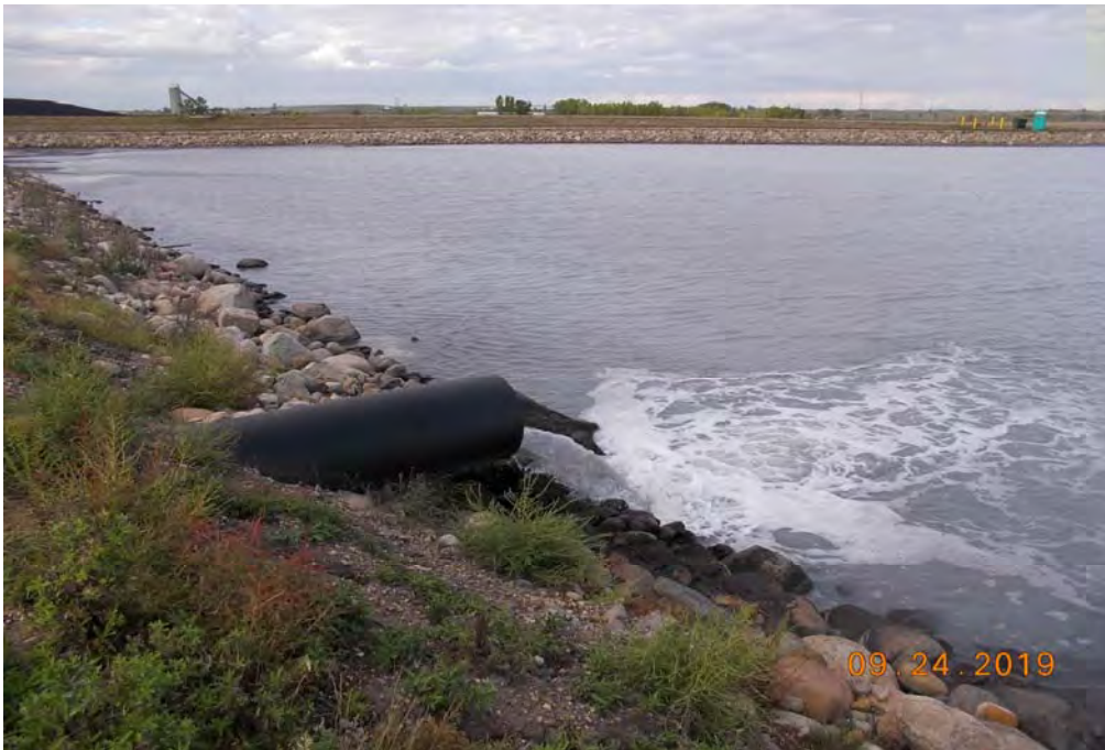
Photograph 17 (Center cell west upstream slope) Inlet from west cell into center cell (PDS DPS (4).JPG)
