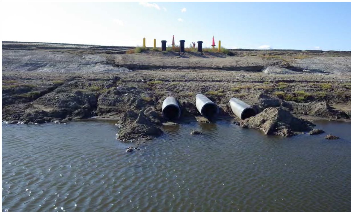
Photograph 4 (East cell south upstream slope) Cross-over pipes from Upstream Raise 91 (IMGP7008.JPG)
