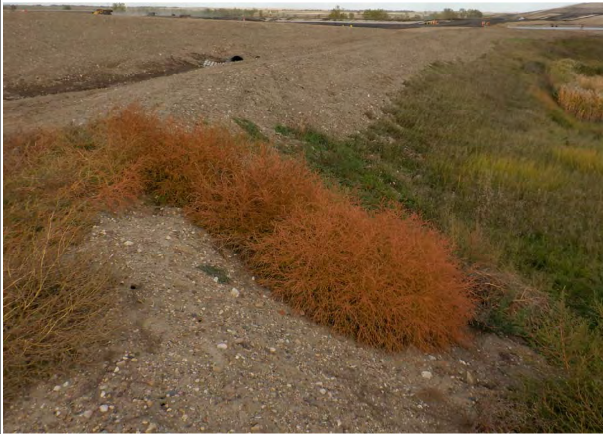
Photograph 7 (Center cell south downstream slope) Contact water control berm and downstream slope (to be seeded) (DSCF0513.JPG)
