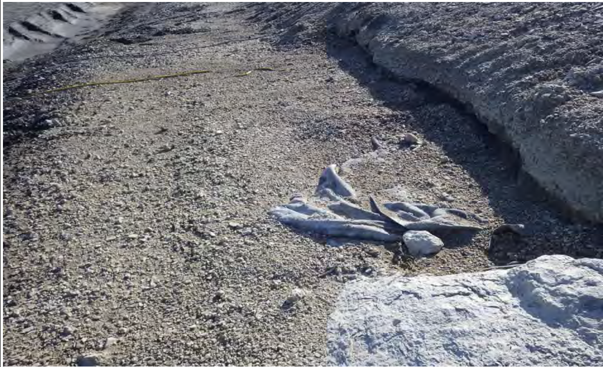
Photograph 5 (East cell south upstream slope) Exposed geotextile, upstream fly ash protective cover slope (IMGP7009.JPG)
