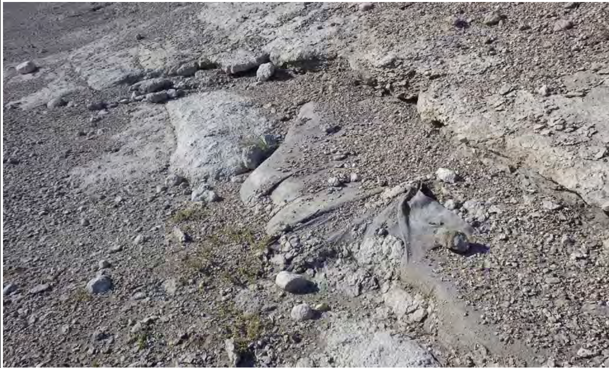
Photograph 3 (East cell west upstream slope) Exposed geotextile, upstream fly ash protective cover slope (IMGP7006.JPG)
