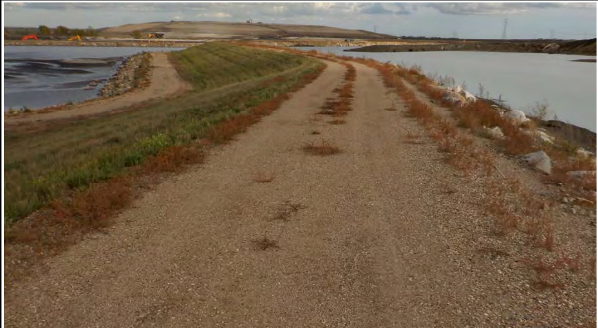
Photograph 14 (West cell east berm crest) Crest road between center cell and west cell (gravel, good condition) (DSCF0526.JPG)
