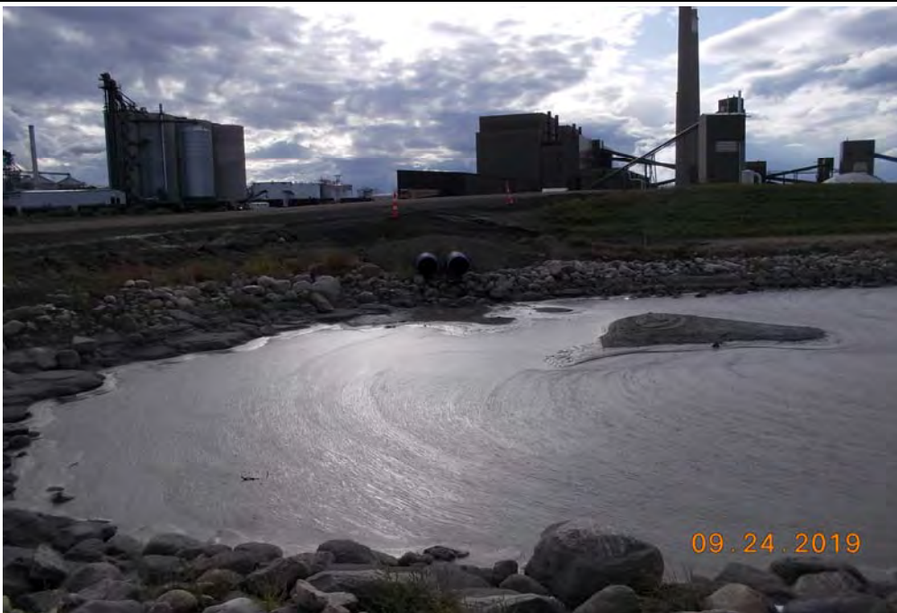
Photograph 20 (Center cell southeast berm crest) Culvert pipe inlets to the south side of the center cell, no flow (PDS DPS (20).JPG)
