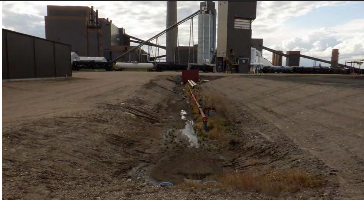
Photograph 8 (Center cell south downstream slope) Bottom ash and flue-gas desulfurization pipelines and contact water drainage directed toward the center cell via culverts (DSCF0514.JPG)
