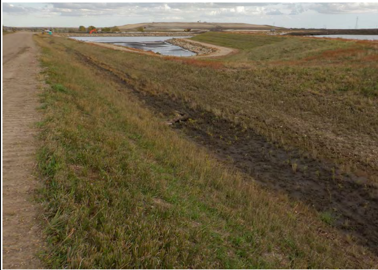
Photograph 13 (West cell and Center cell north ditch) North side contact water drainage ditch and center cell berm, good condition (DSCF0525.JPG)
