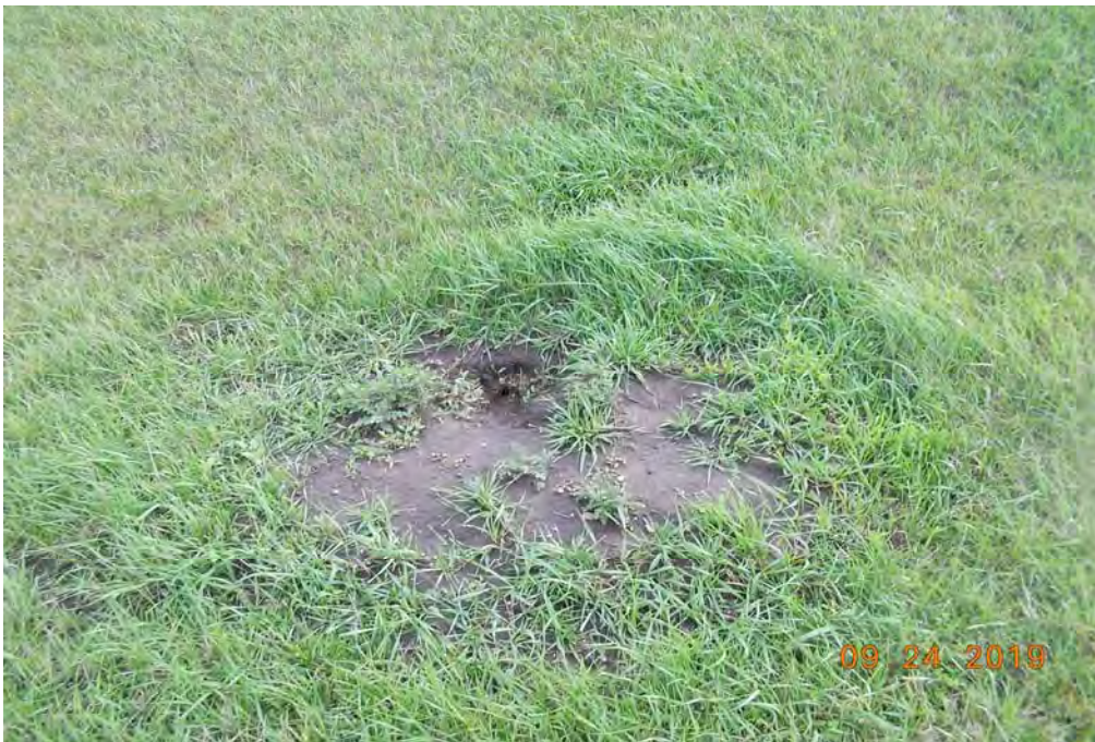
Photograph 18 (Center cell north downstream slope) Large animal burrow (PDS DPS (11).JPG)
