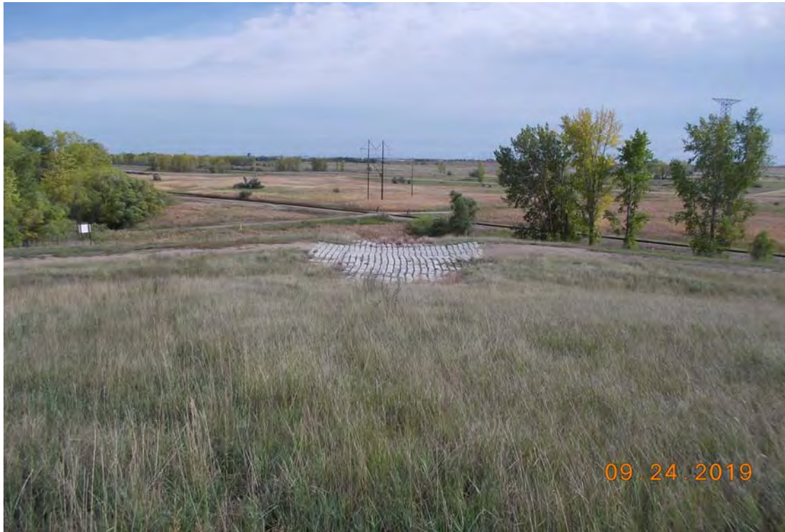
Photograph 4 (Southeast CCR downstream slope) Articulated Concrete Block (ACB) downchute on southeast corner, well-vegetated (PDS SE16 (10).JPG)
