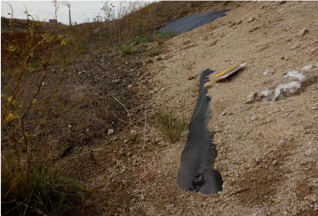
Photograph 9 (North CWCA channel) Wrinkle in exposed geomembrane liner on upstream slope (DSCF0479.JPG)
