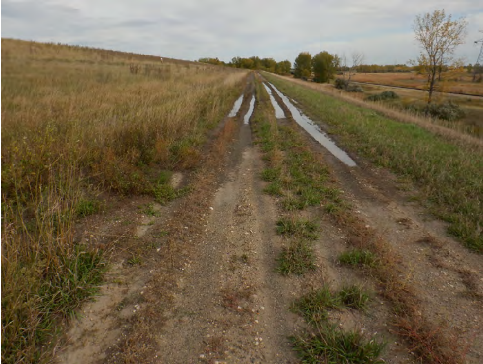
Photograph 3 (South berm crest access road) Standing water in access road on the south berm crest (DSCF0506.JPG)
