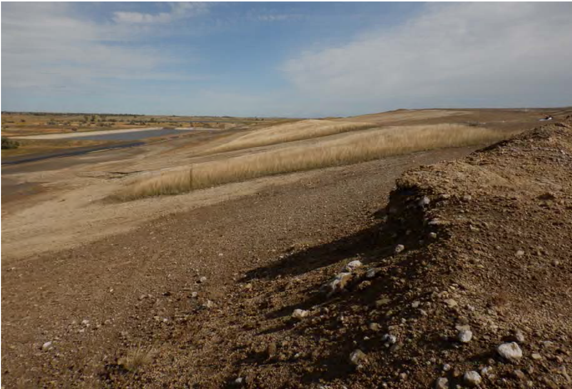
Photograph 12 (North CCR downstream slope) Temporary cover on north fly ash slope (DSCF0488.JPG)
