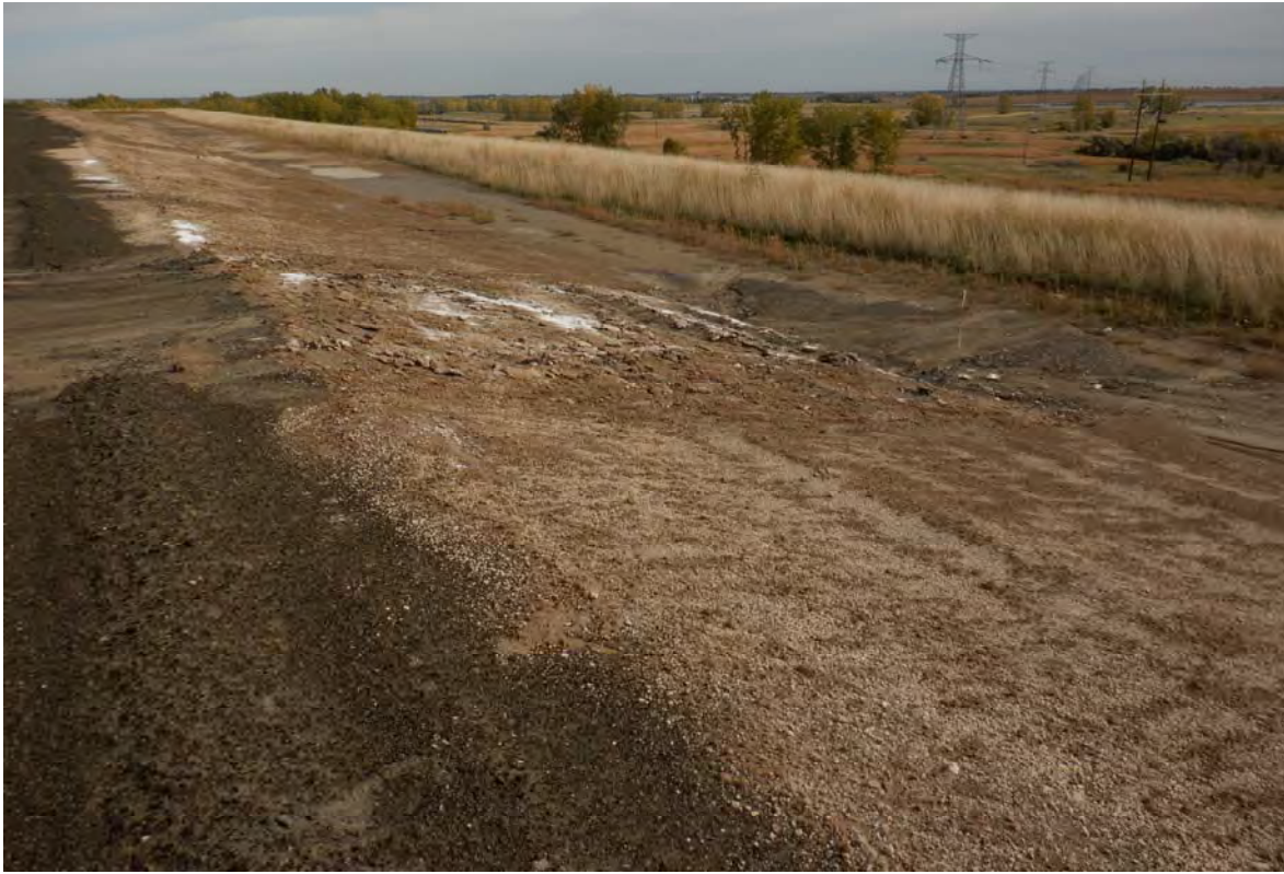
Photograph 17 (South CCR downstream slope (no cover)) Erosion of fly ash on the south CCR downstream slope (DSCF0504.JPG)
