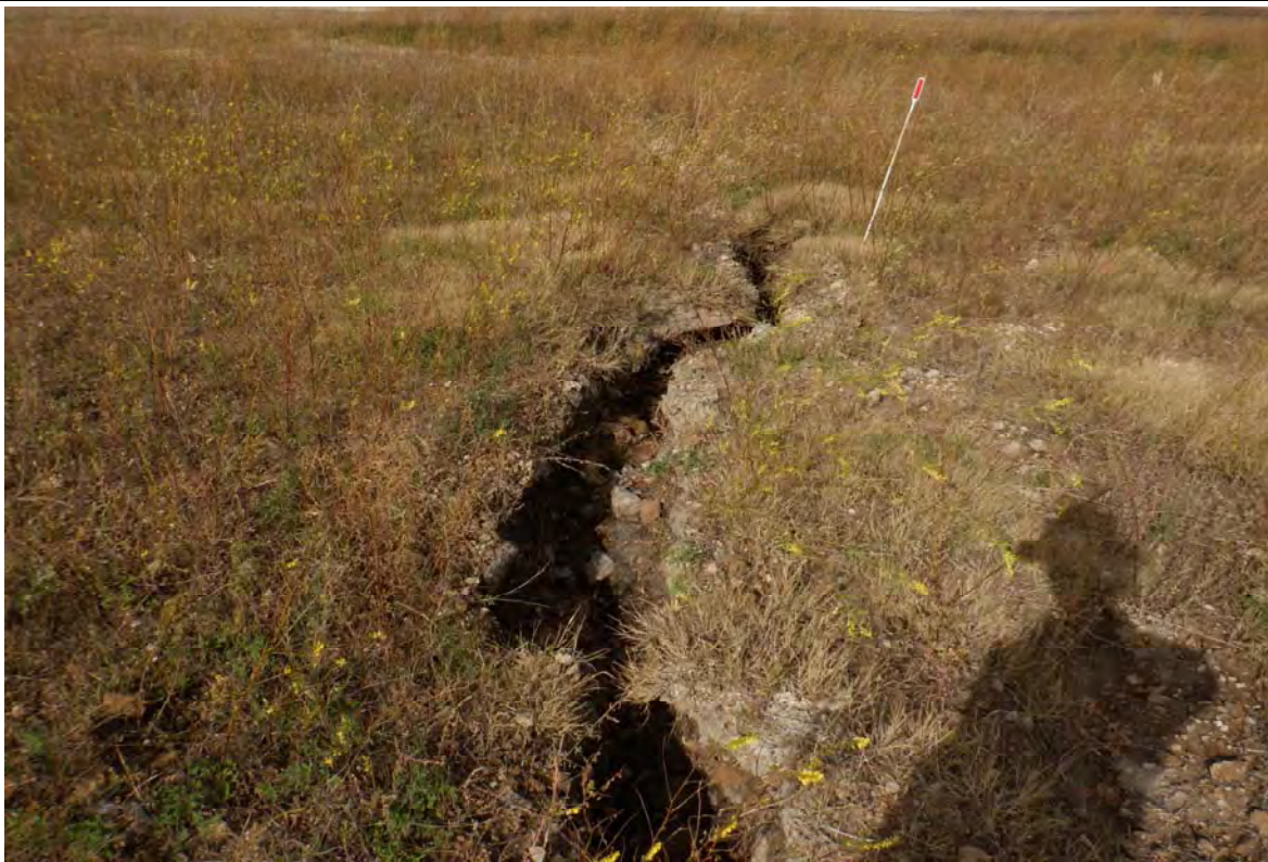
Photograph 14 (Northeast CCR downstream slope) Erosion rill in temporary cover on northeast CCR downstream slope (DSCF0499.JPG)
