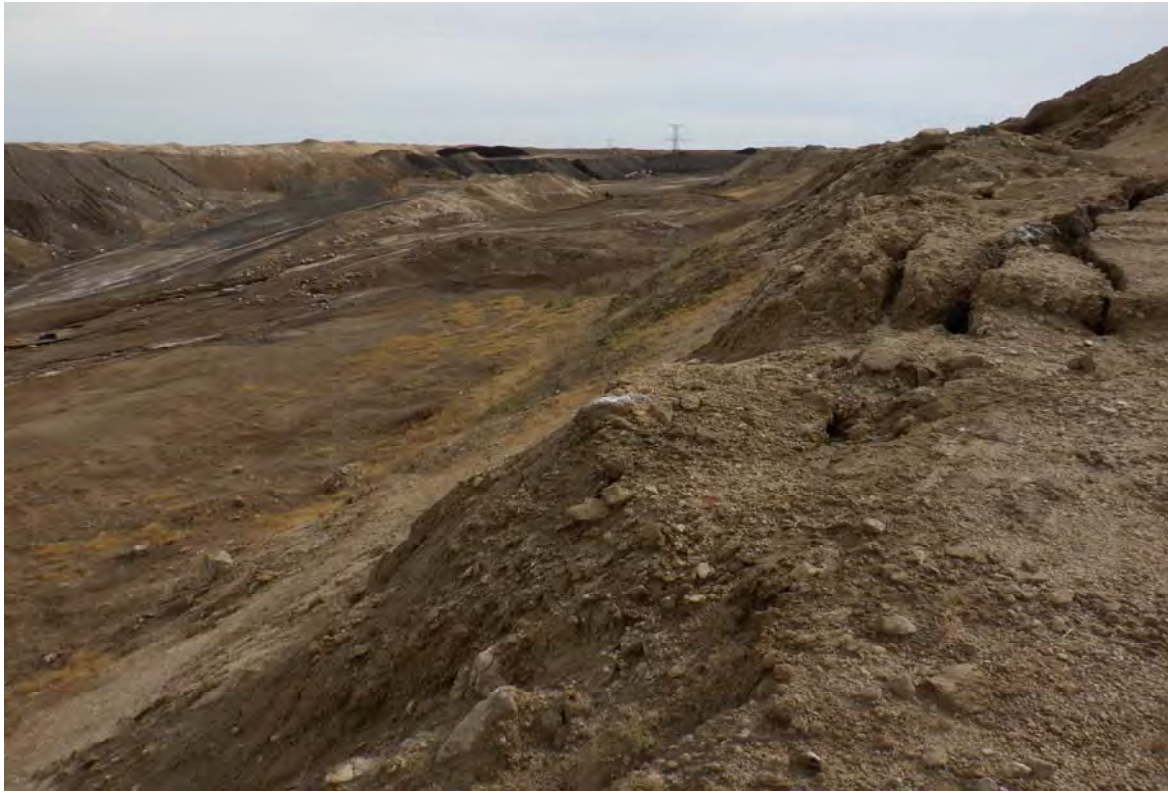
Photograph 13 (C&D area) Minor erosion on interior slopes to historic C&D access area of Southeast 16 (DSCF0495.JPG)
