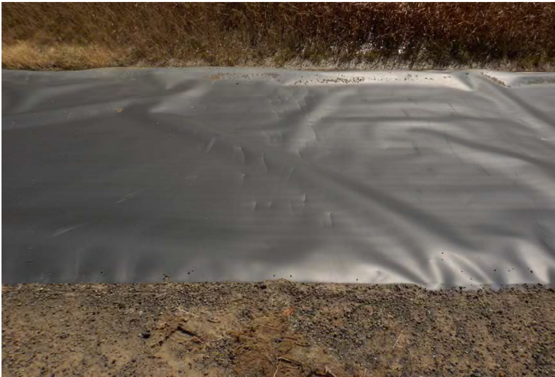
Photograph 10 (North CWCA channel) Exposed geomembrane on upstream slope of CWCA channel and damage from animals (DSCF0482.JPG)
