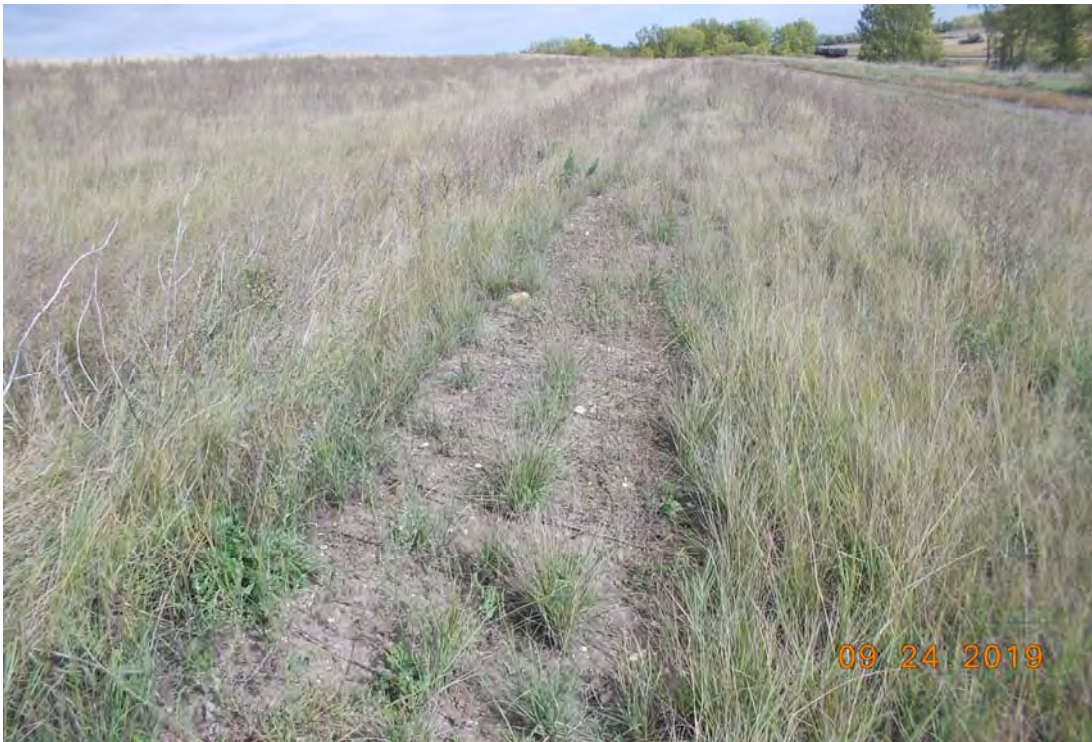
Photograph 5 (South CCR downstream slope (covered)) Sparse vegetation on final cover of downstream slope side of terrace berm (PDS SE16 (13).JPG)
