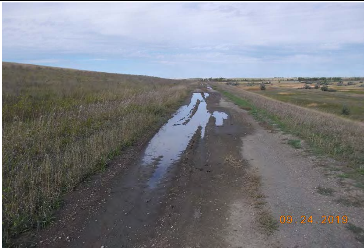
Photograph 2 (East berm crest access road) Standing water in access road on the east berm crest (PDS SE16 (6).JPG)
