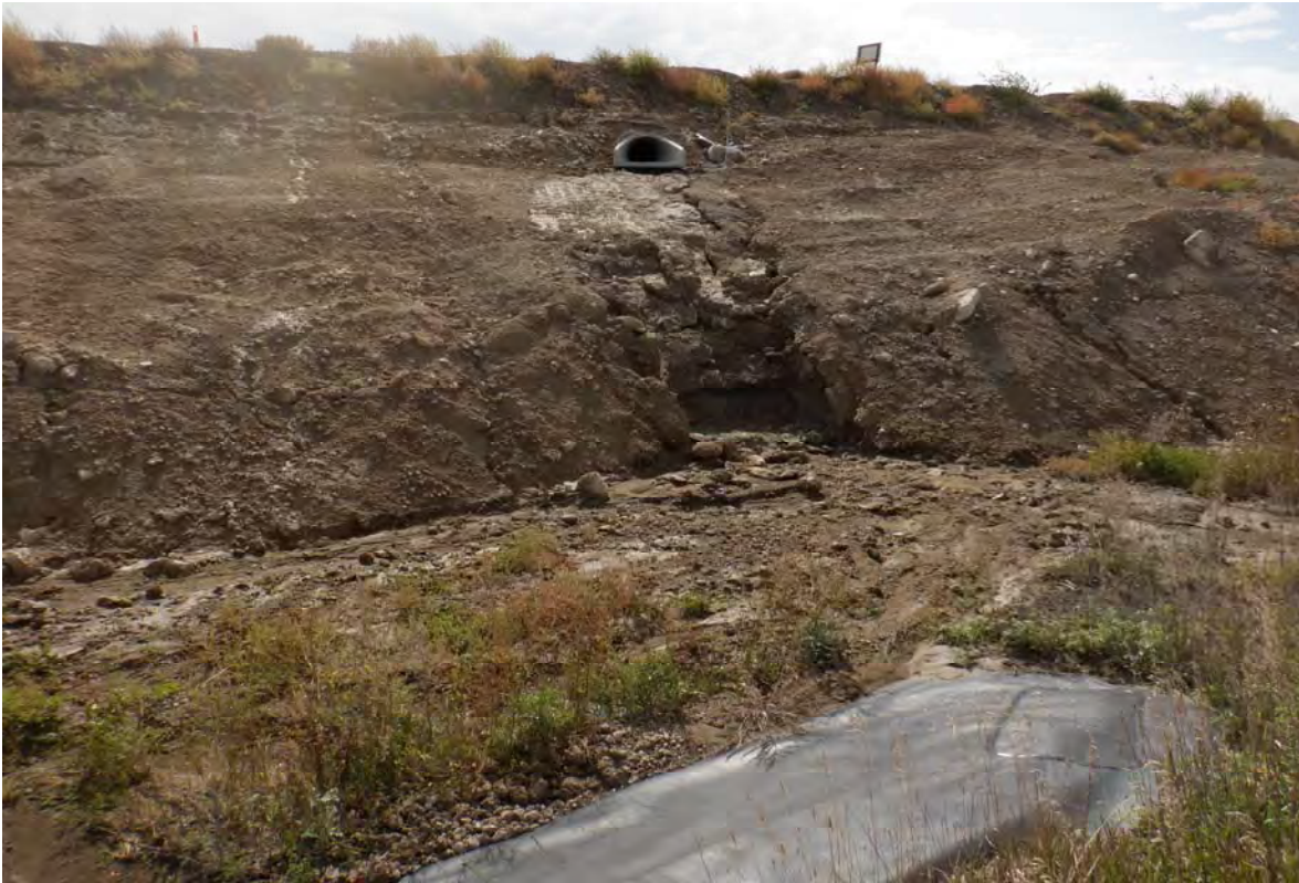
Photograph 11 (North CWCA channel) Erosion of fly ash below culvert, Upstream Raise 92 area to CWCA channel (DSCF0485.JPG)
