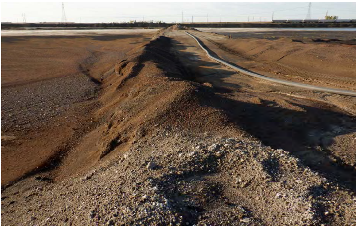
Photograph 19 (Upstream Raise interior) Upstream Raise 91 interior and FGD inflow pipe (DSCF0544.JPG)
