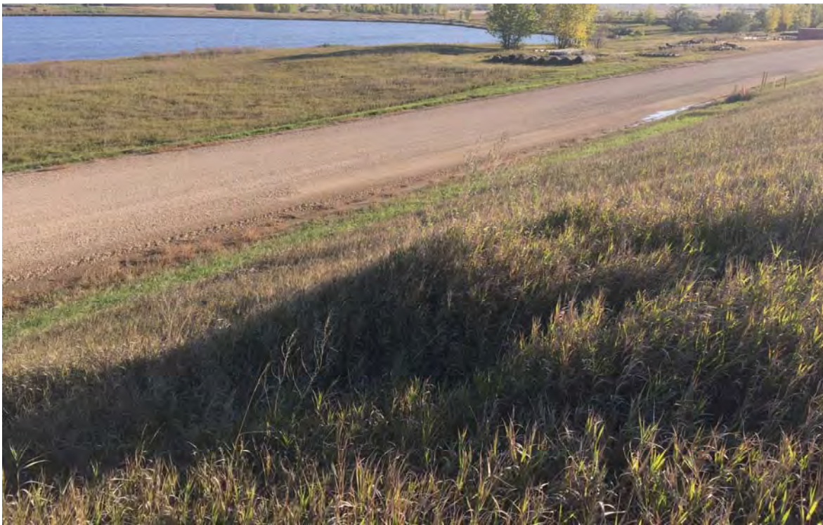
Photograph 14 (North downstream slope and toe) Irregular slope geometry on the north downstream slope, well-vegetated (11.JPG)
