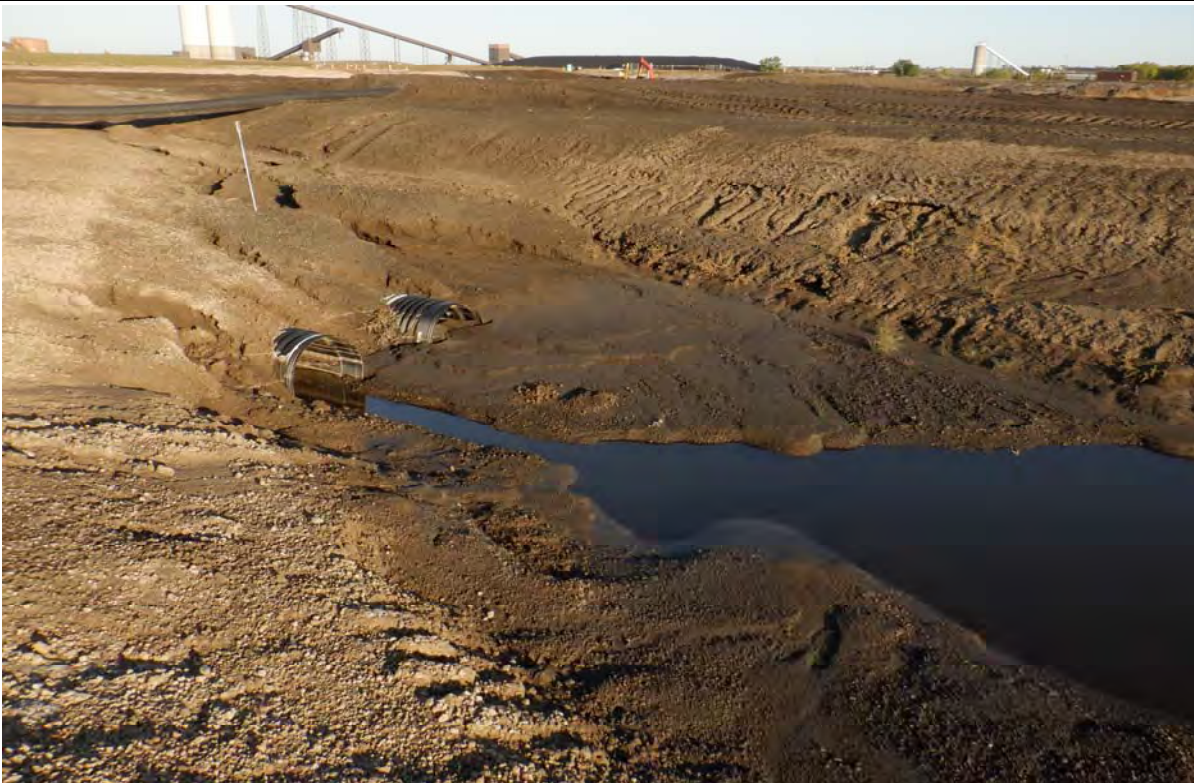
Photograph 18 (North perimeter ditch) Inlet perimeter ditch culverts to northwest contact water pool (DSCF0542.JPG)
