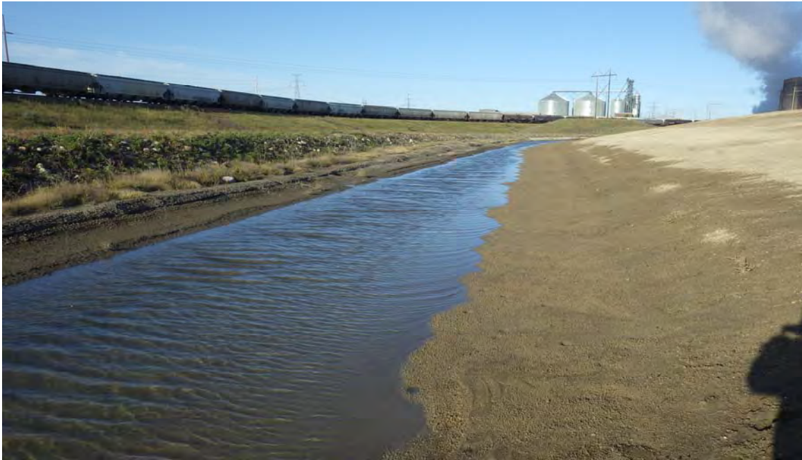
Photograph 9 (South CCR downstream slope) Perimeter channel and downstream CCR slope saturated to approximately elevation 1919 feet (IMGP6988.JPG)
