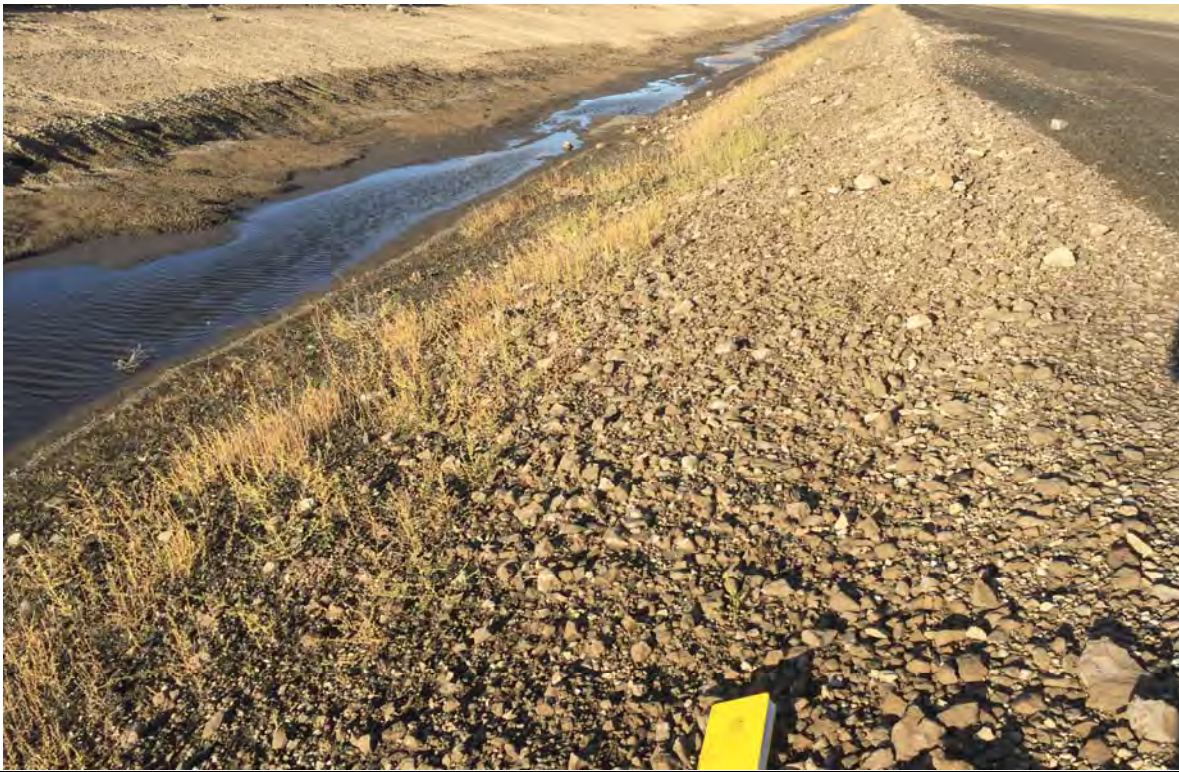
Photograph 13 (North perimeter ditch) North berm upstream slope fly ash protective cover and perimeter channel (7.JPG)
