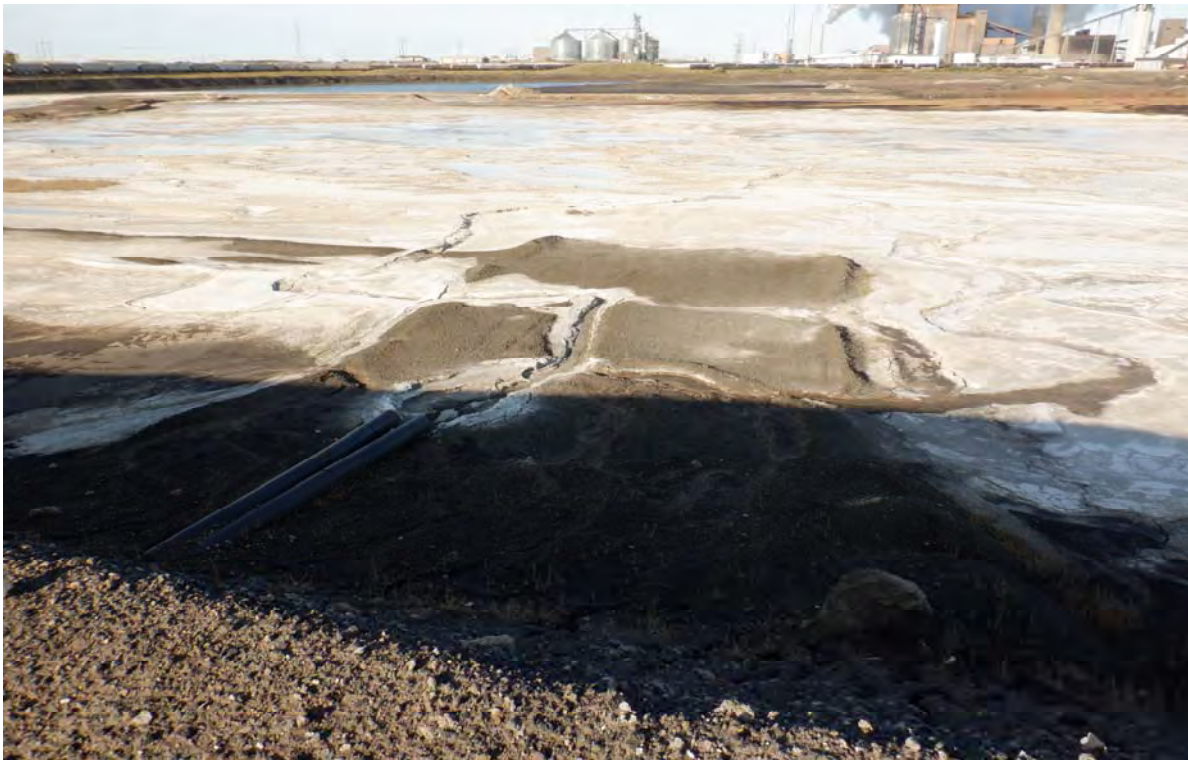
Photograph 22 (East CCR berm crest and upstream slope) Inflow piping from Upstream Raise 92 (DSCF0549.JPG)
