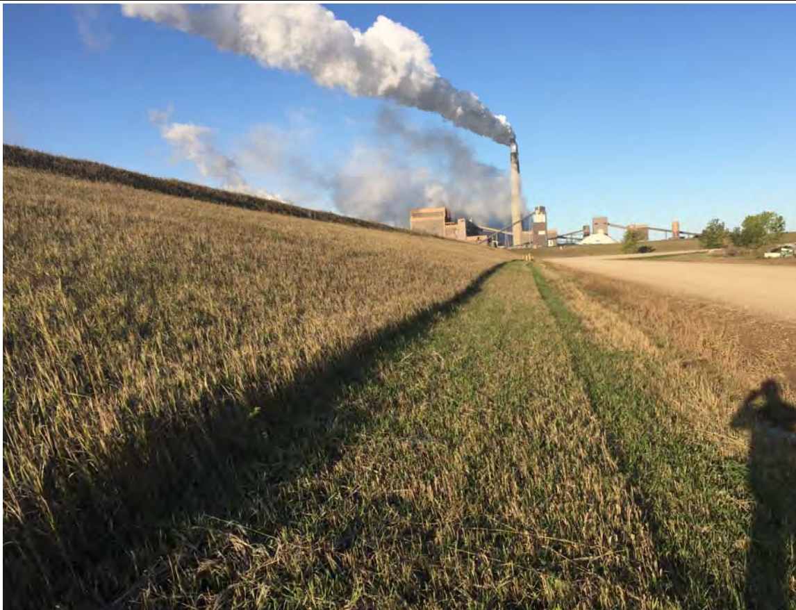
Photograph 12 (North downstream slope and toe) Well-vegetated downstream slope and toe (2.JPG)
