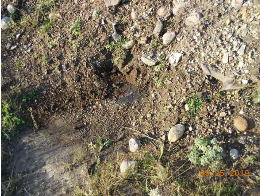
Photograph 7 (Southwest berm upstream slope) Erosion of fly ash protective cover and exposed geomembrane (PDS UR91 (2).jpg)
