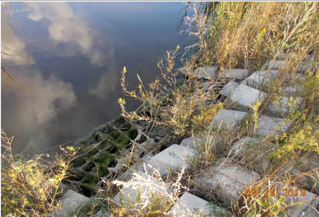
Photograph 2 (Southwest toe and ditch) Inlet side of surface water drainage culvert, algae on trash guard limiting full flow (PDS UR91 (15).JPG)
