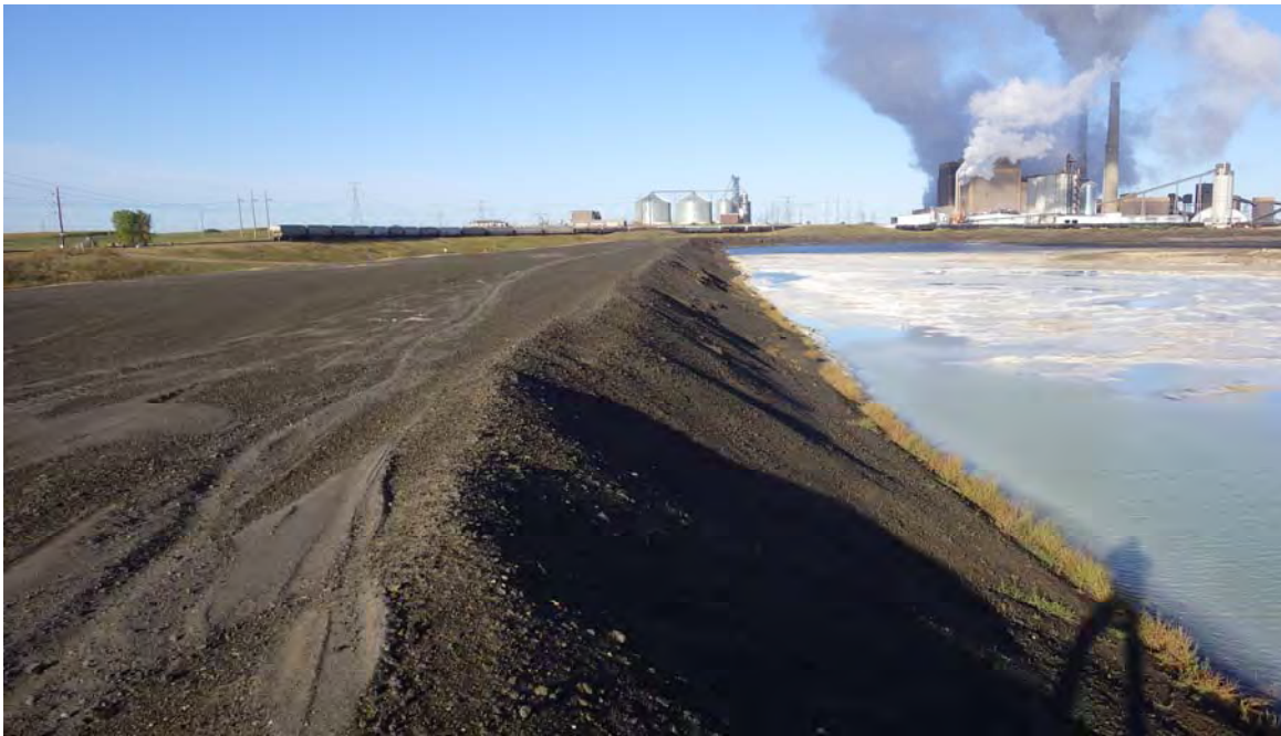
Photograph 10 (South CCR upstream slope and berm crest) CCR berm crest, CCR upstream slope and Flue Gas Desulfurization (FGD) pool (IMGP6992.JPG)
