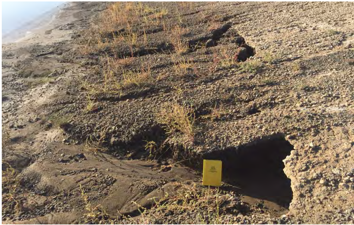
Photograph 15 (Northwest berm crest) Erosion of berm upstream fly ash slope near the northwest contact water pool of Upstream Raise 91 (18.JPG)
