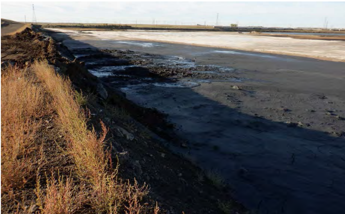
Photograph 21 (East CCR berm crest and upstream slope) CCR material deposition on east side of Upstream Raise 91 (DSCF0548.JPG)
