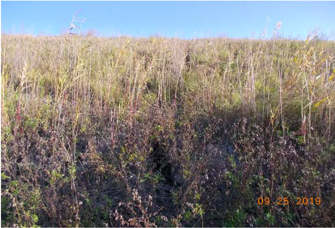
Photograph 1 (South berm downstream slope) Large erosion rill on vegetated slope (PDS UR91 (5).JPG)
