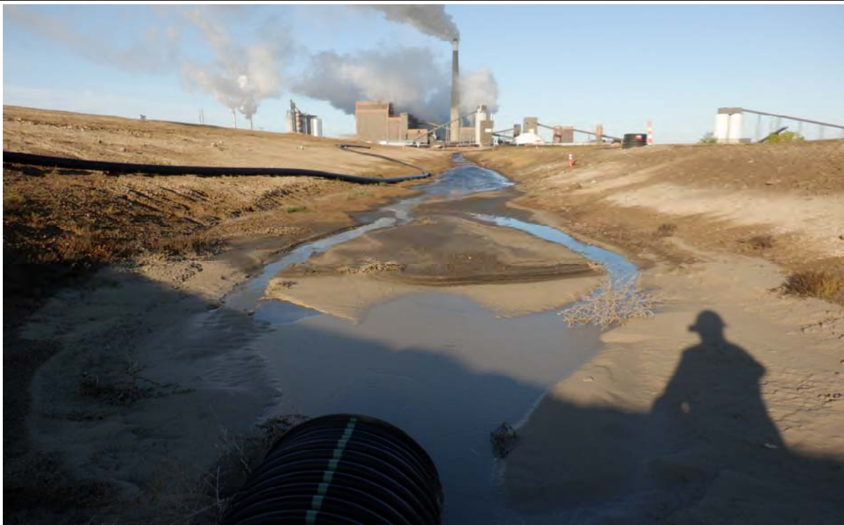
Photograph 20 (North perimeter ditch) Culvert and drainage from Upstream Raise 92 in perimeter ditch (DSCF0546.JPG)
