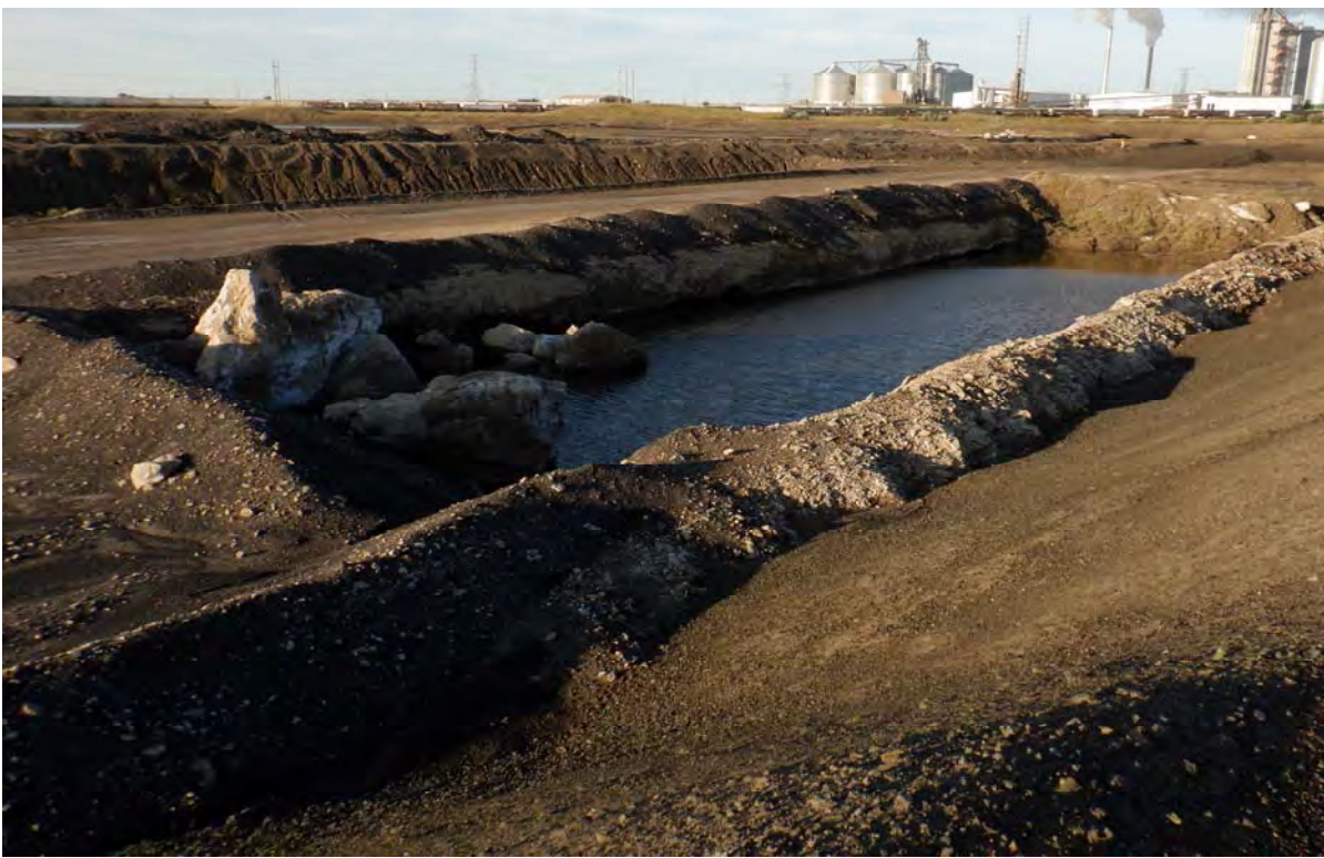
Photograph 17 (North CCR upstream slope) Upstream Raise 91 interior and CCR placement (DSCF0540.JPG)
