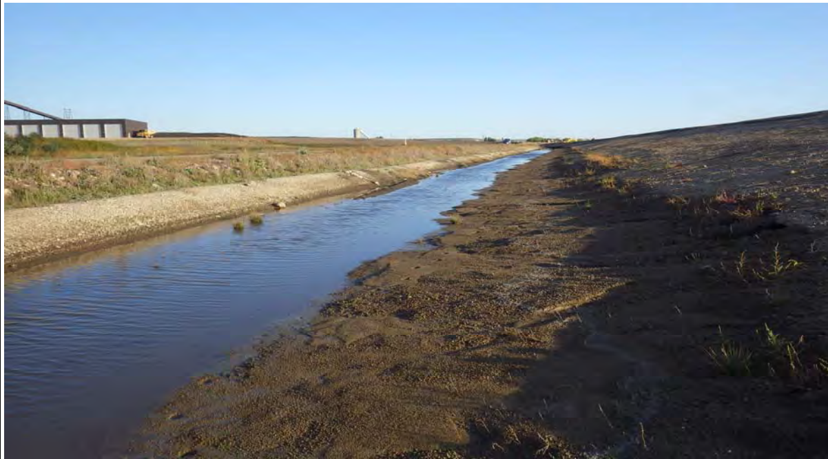
Photograph 5 (West CCR downstream slope) Perimeter channel and CCR downstream slope saturated to approximately elevation 1919 feet (IMGP6978.JPG)
