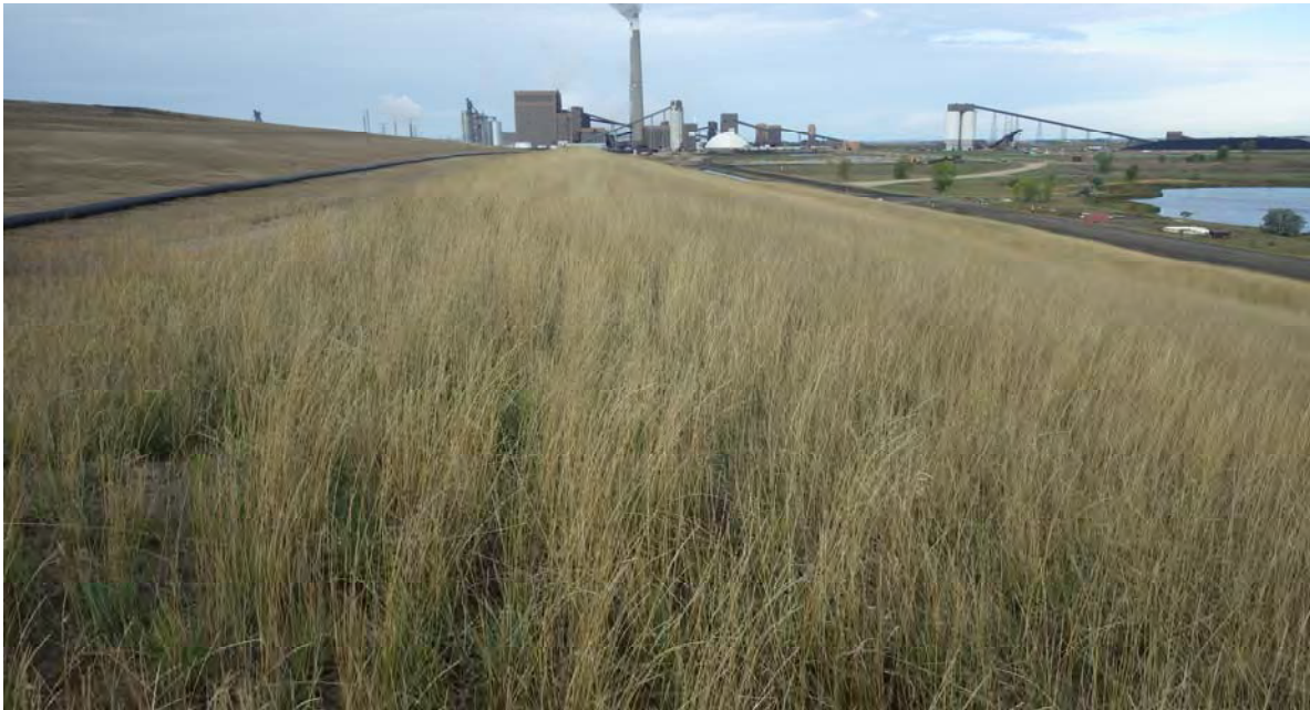
Photograph 2 (North CCR downstream slope) Temporary cover on north CCR slope (IMGP6859.JPG)
