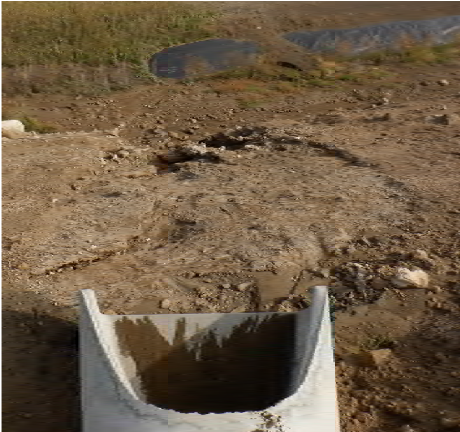
Photograph 23 (North berm downstream slope) Culvert outlet conveying contact water from Upstream Raise 92 to Southeast 16 contact water channel (DSCF0461.JPG)
