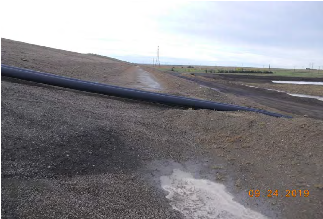
Photograph 12 (West CCR downstream slope (no cover)) Gravity drains between Upstream Raise 92 and Upstream Raise 91 (PDS UR92 (8).JPG)
