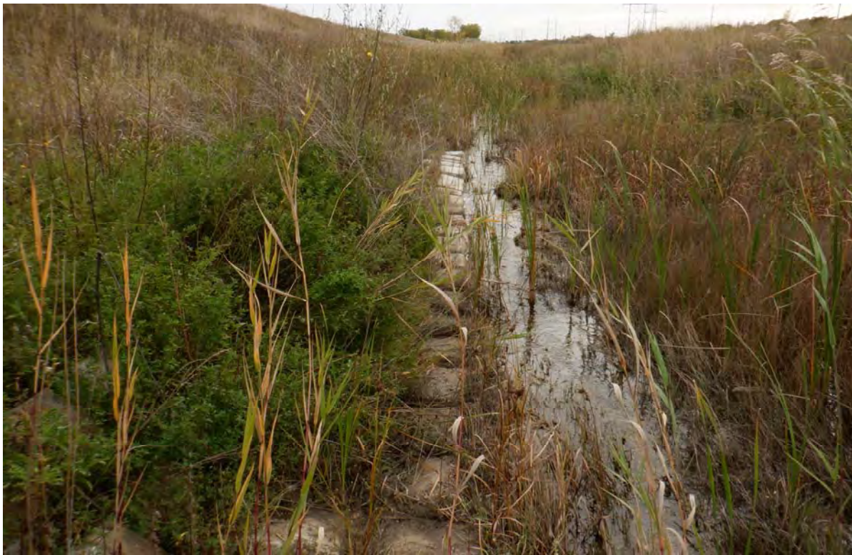
Photograph 21 (South berm downstream slope and toe) ACB completed to the toe of the berm downstream slope instead of across the south drainage channel, minor woody vegetation (DSCF0452.JPG)
