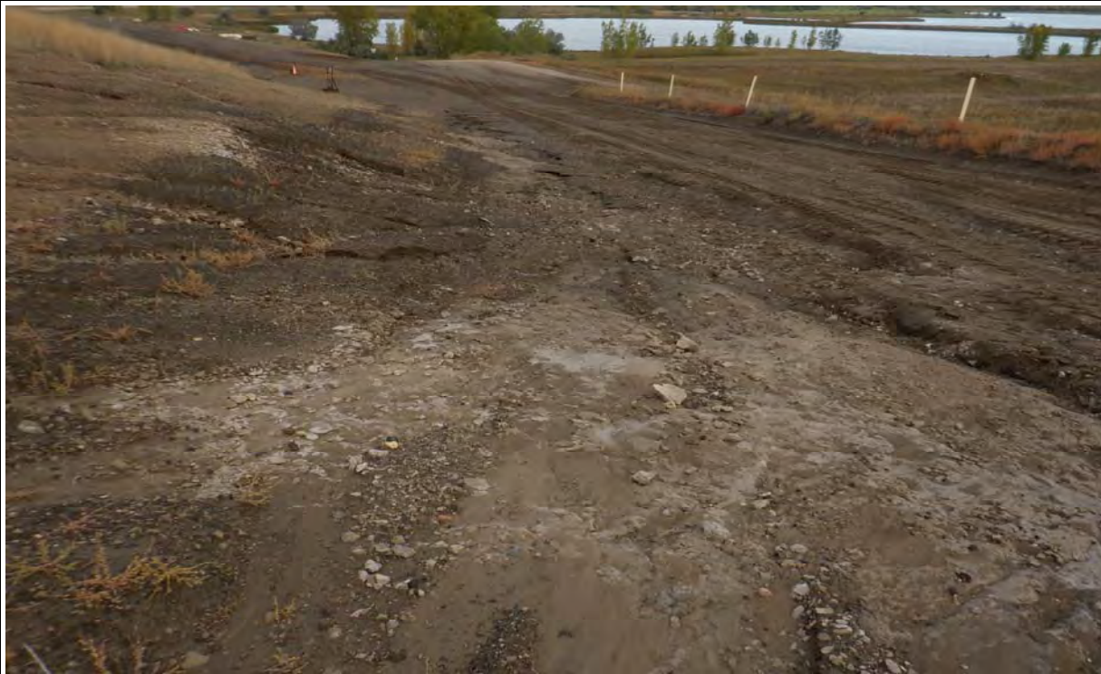
Photograph 14 (North haul ramp) Minor erosion of fly ash along inside of ramp (north side) (DSCF0414.JPG)
