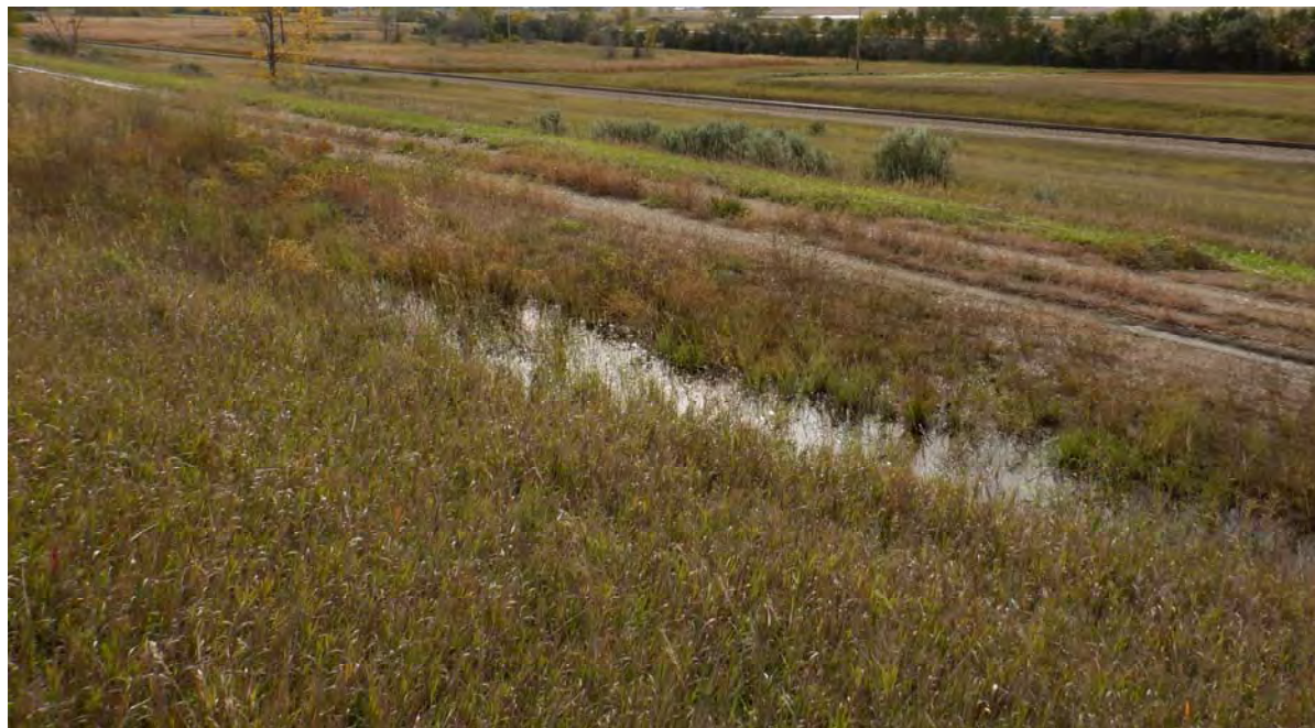
Photograph 22 (Southeast CCR downstream slope (covered)) Standing water at southeast toe of CCR downstream slope (covered) above perimeter road (DSCF0457.JPG)
