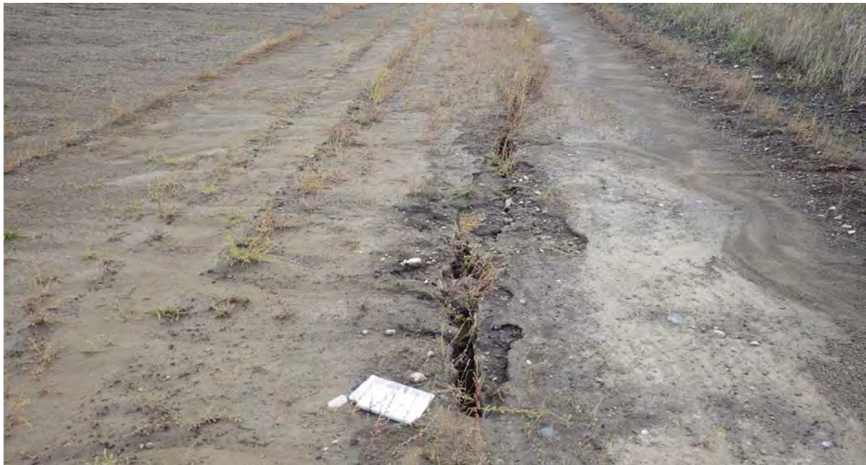
Photograph 5 (South CCR downstream slope (no cover)) Cracking along south side within the contact water control ditch (IMGP6874.JPG)
