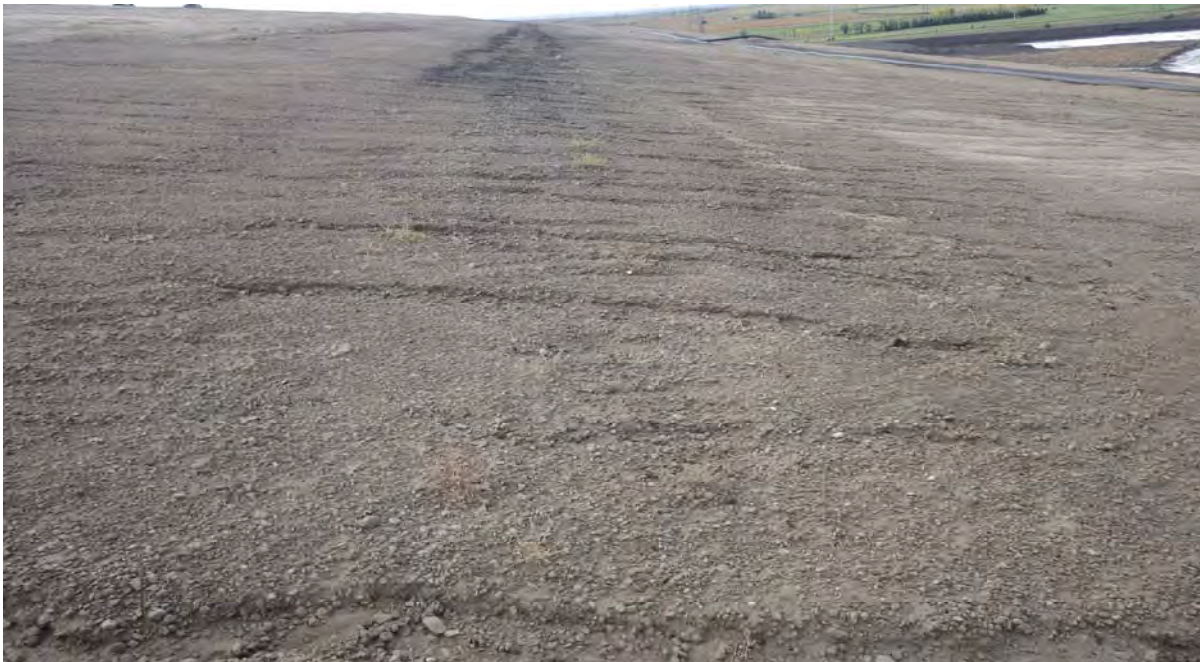
Photograph 4 (West CCR downstream slope (no cover)) Minor fly ash erosion on west downstream slope (IMGP6865.JPG)
