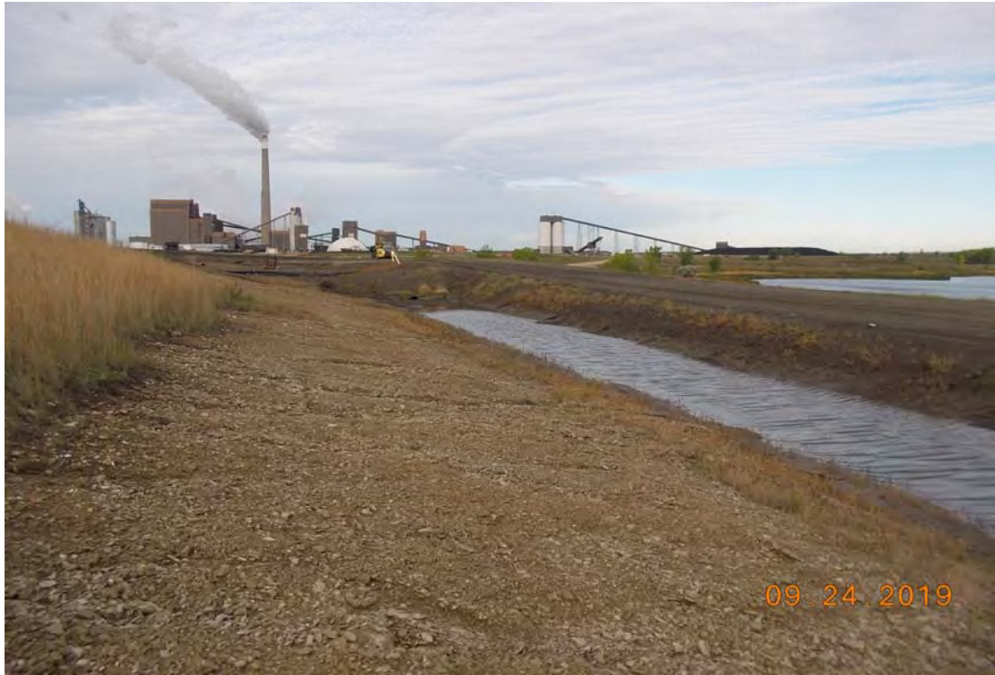
Photograph 11 (North CCR downstream slope) Perimeter contact water control ditch and partially plugged HDPE culvert directing contact water to Upstream Raise 91 (PDS UR92 (5).JPG)
