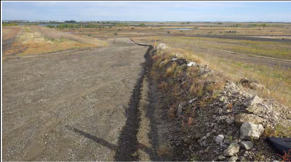
Photograph 9 (East haul ramp) Safety berm along portion of east ramp (IMGP6894.JPG)
