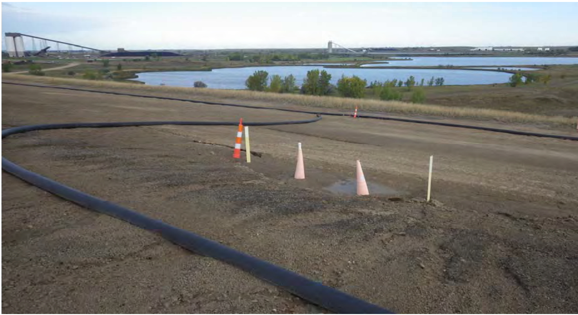
Photograph 1 (North CCR downstream slope (no cover)) Crack in fly ash near piezometers (IMGP6856.JPG)
