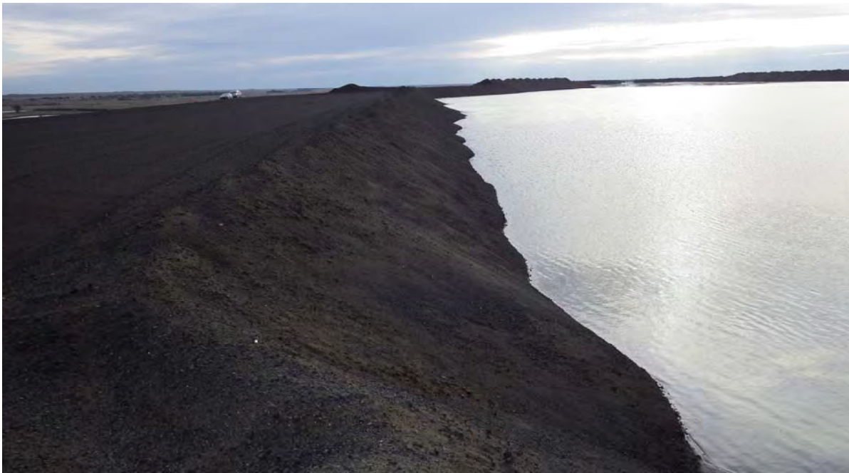
Photograph 3 (Northwest CCR crest and upstream slope) Bottom ash berm crest and upstream slope on northwest Flue Gas Desulfurization (FGD) Pool corner (IMGP6862.JPG)
