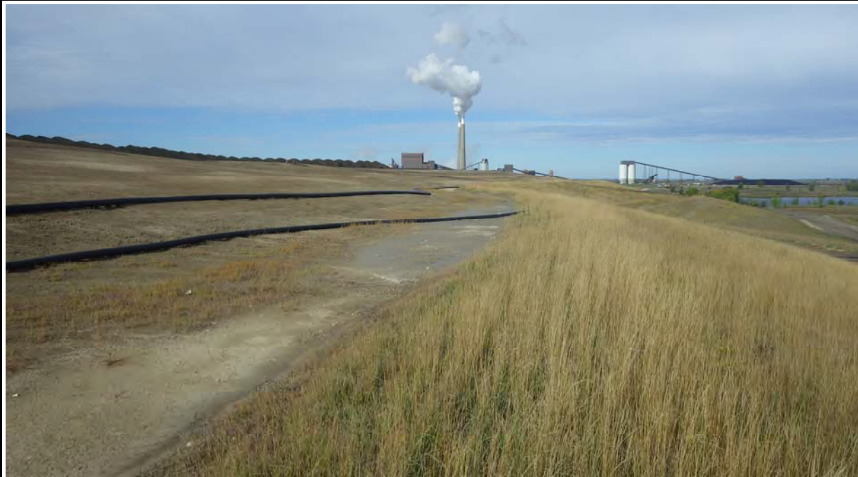
Photograph 10 (North CCR downstream slope) Contact water control ditch and temporary cover below elevation 1950 feet (IMGP6896.JPG)
