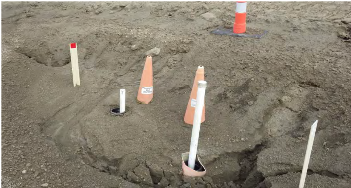
Photograph 6 (South CCR downstream slope (no cover)) Cracking and erosion of fly ash around piezometers (IMGP6876.JPG)
