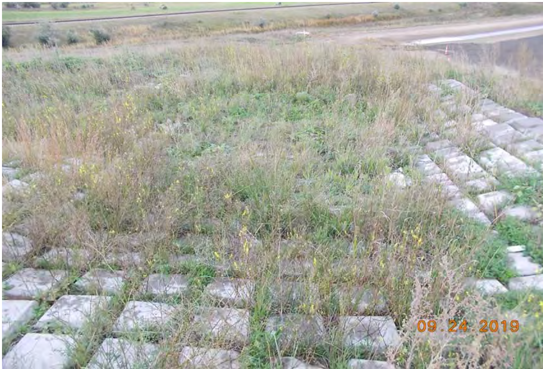
Photograph 13 (Southwest downstream downchute channel) Articulated Concrete Block (ACB) downchute channel with established vegetation (PDS UR92 (10).JPG)
