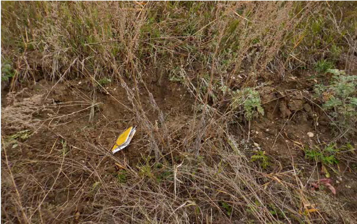
Photograph 17 (South berm downstream slope and toe) Oversteepened toe of slope area (DSCF0439.JPG)
