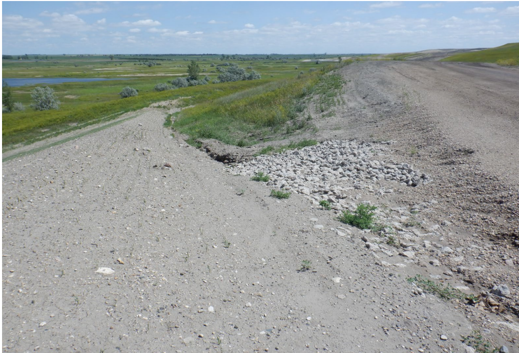
Photograph 7 (July 2020) Drainage channel that directs water toward the composite-lined Southeast 16 landfill contact water containment area. (DSCF1170.JPG)
