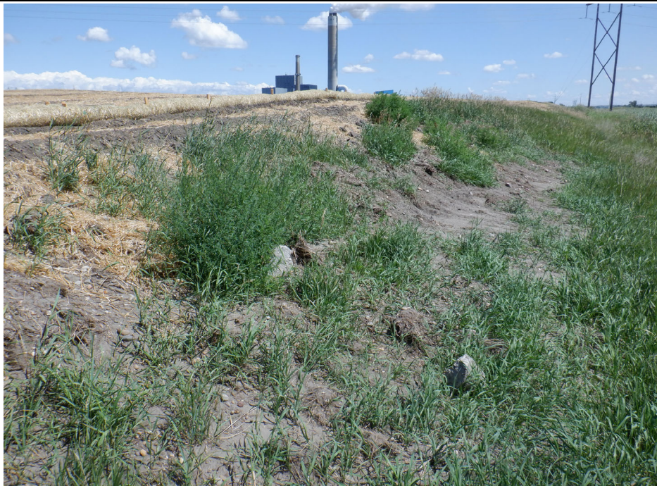
Photograph 4 (South Perimeter Berm Downstream Slope) Minor erosion and bare vegetation on the southern downstream slope. (IMG_DSCF1014.JPG)
