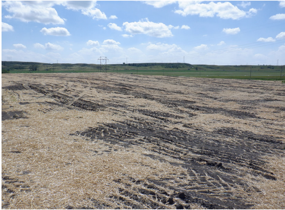
Photograph 7 (Final Cover) Recently seeded and mulched final cover. (IMG_DSCF1048.JPG)
