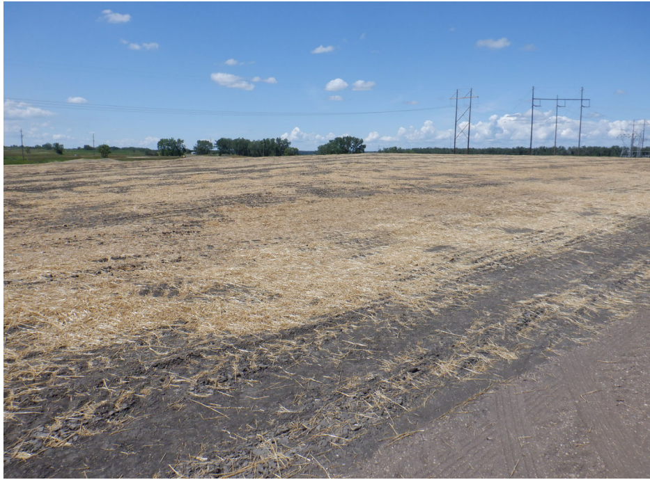
Photograph 1 (East Final Cover Slope) Bottom ash landfill closed and covered. (IMG_DSCF1005.JPG)
