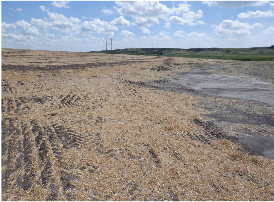
Photograph 5 (West Perimeter Berm Downstream Slope and Toe) Recently seeded and mulched downstream slope/toe and final cover (background). (IMG_DSCF1039.JPG)
