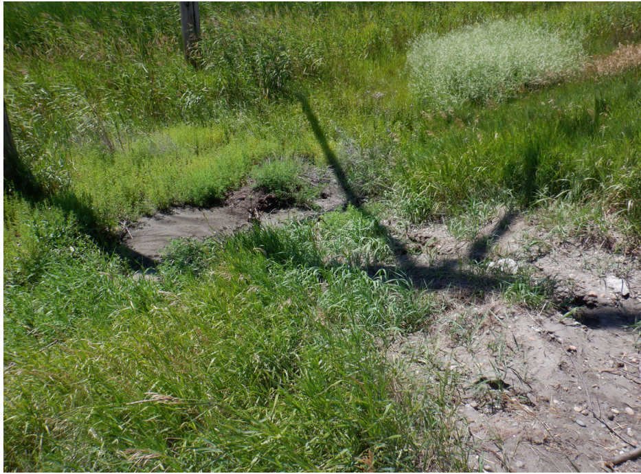
Photograph 3 (South Perimeter Berm Downstream Slope) Small rodent burrows on the slope and near the toe of the facility. (IMG_DSCF1011.JPG)
