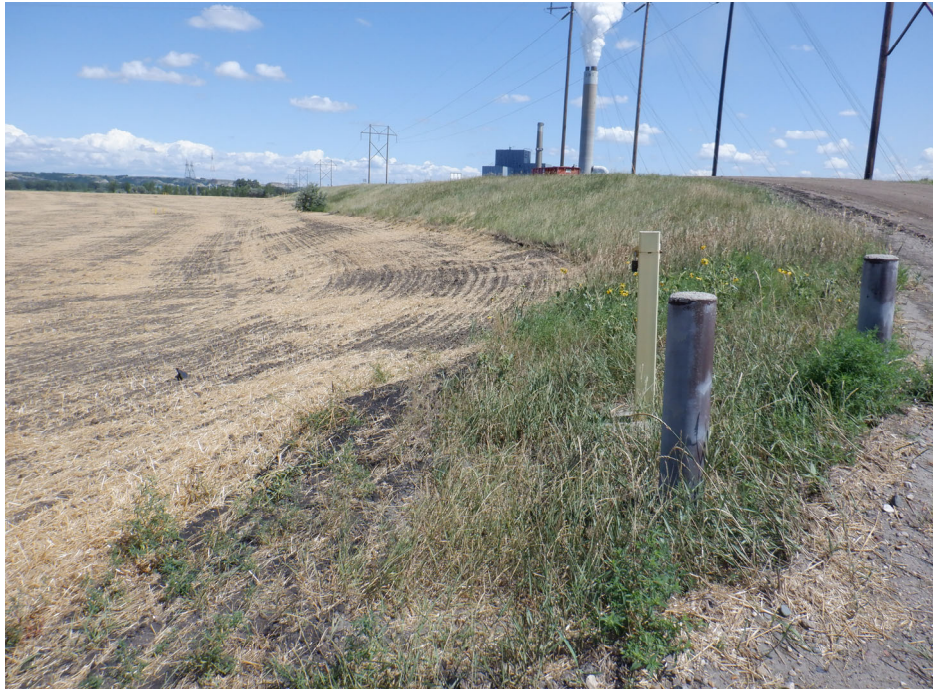
Photograph 6 (North Perimeter Berm Downstream Slope and Toe) Well vegetated perimeter berm downstream slope and recently seeded and mulched toe. (IMG_DSCF1041.JPG)
