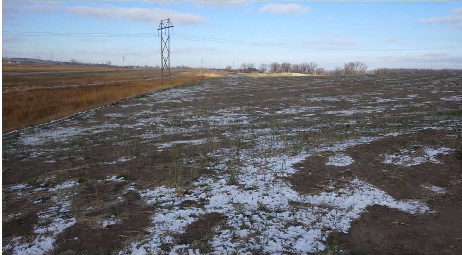
Photograph 10 (South Final Cover Slope) Recently seeded and mulched area (vegetation beginning to grow, October 2020). (IMG_7391.JPG)
