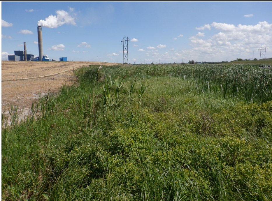
Photograph 2 (South Perimeter Berm Toe) Vegetation in surface water drainage ditch. (IMG_DSCF1024.JPG)
