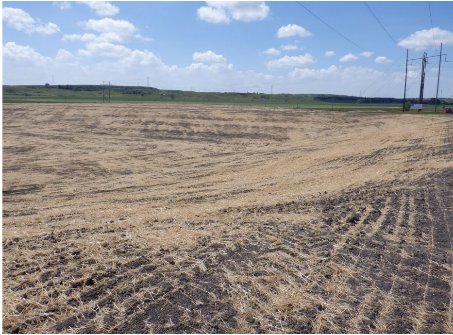
Photograph 1 (NE berm crest of historic north cell) Interior of north cell and center cell (bottom ash, liner system, and a portion of the underlying clay removed during restoration activities). (IMG_DSCF0954.JPG)
