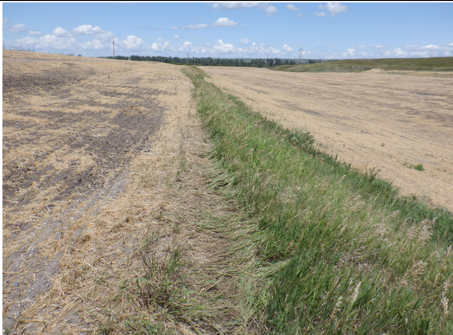
Photograph 4 (South cell east berm downstream slope) Lower east berm downstream slope with historic well-established grass vegetation mid-slope and recently seeded and mulched areas on the upper slope and near the toe of the slope. (IMG_DSCF0972.JPG)
