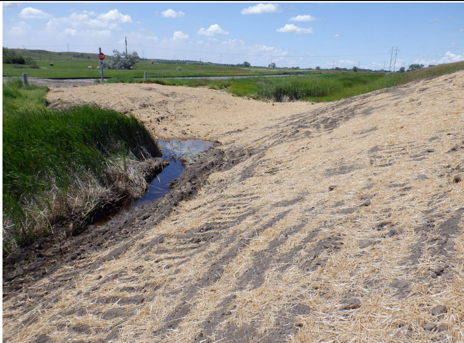
Photograph 6 (Southeast corner of south cell) Drainage ditch at the toe of the south slope of the south cell and recently seeded and mulched lower berm downstream slopes. (IMG_DSCF0974.JPG)
