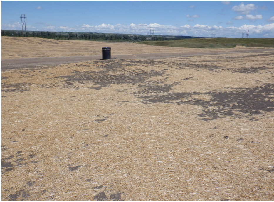
Photograph 11 (Top of south cell) Top of final cover recently seeded and mulched and south cell sump riser pipe. (IMG_DSCF0995.JPG)
