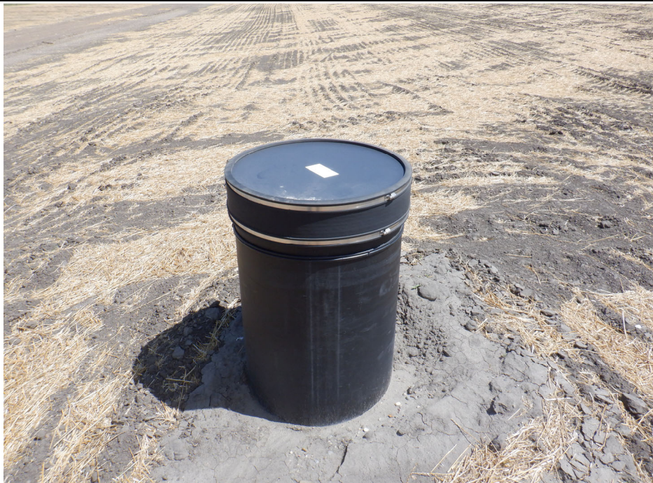
Photograph 12 (Top of south cell) South cell sump riser pipe with removable sump cap in place. (IMG_DSCF0997.JPG)
