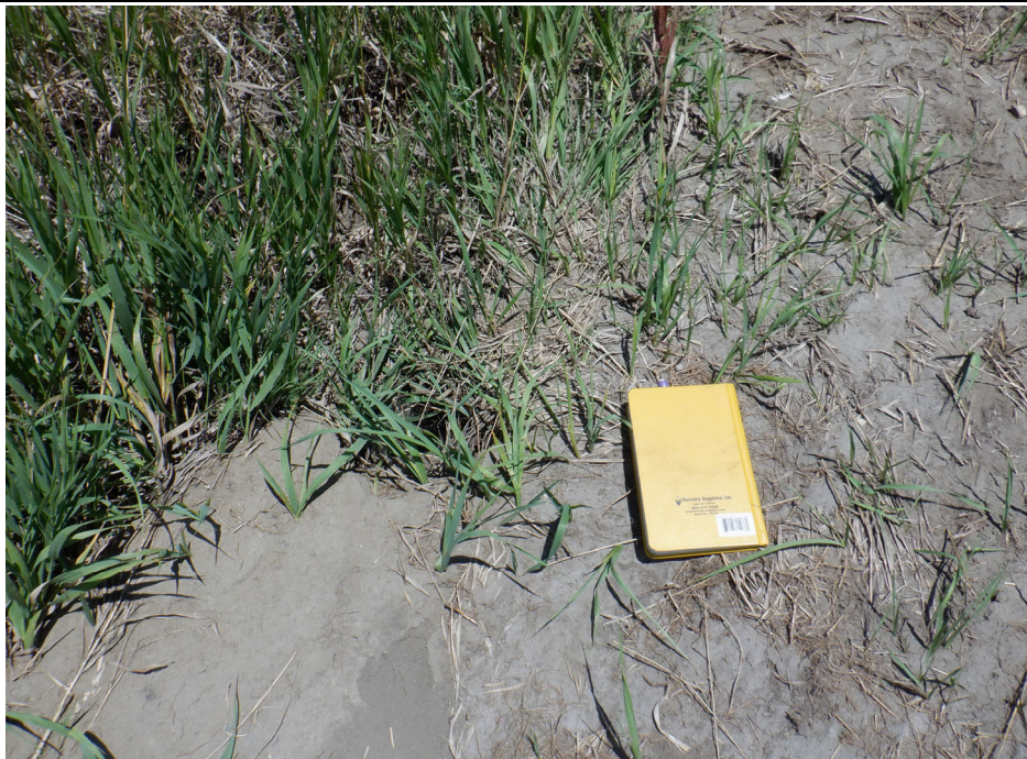
Photograph 8 (South berm downstream slope) Small animal burrow on south downstream slope. (IMG_DSCF0978.JPG)
