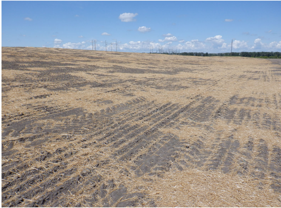
Photograph 3 (East side of south cell) South cell final cover recently seeded and mulched. (IMG_DSCF0967.JPG)
