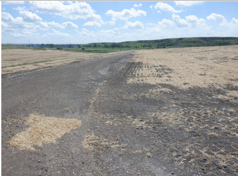
Photograph 2 (NE berm crest of south cell) East berm access road with no signs of damage and recently seeded and mulched east final cover crown area. (IMG_DSCF0966.JPG)
