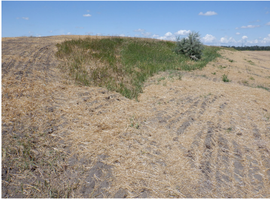
Photograph 5 (South cell east berm downstream slope) Woody vegetation on east downstream slope of south cell. (IMG_DSCF0973.JPG)
