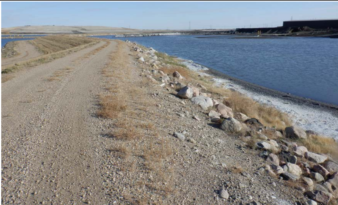
Photograph 21 (West cell east berm) Berm crest between west and center cells, and west cell upstream slope riprap in good condition. (IMG_DSCF1792.JPG)
