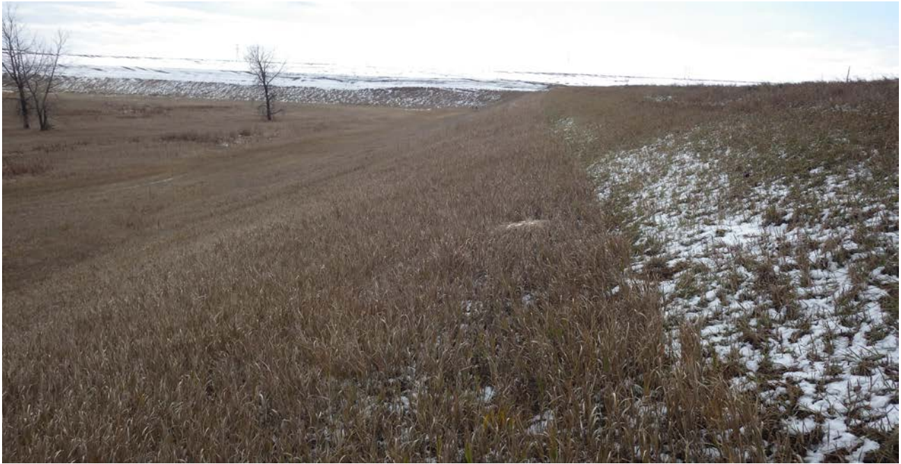
Photograph 15 (East cell east berm) Downstream slope and toe, good vegetation. (IMG_7441.JPG)
