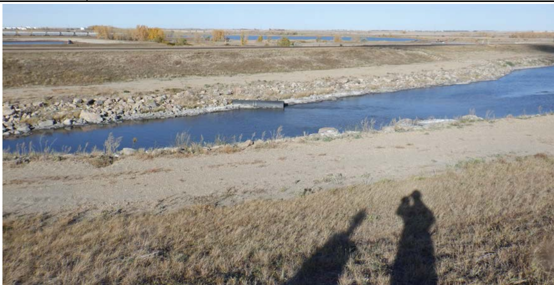
Photograph 22 (Center cell north berm) Center cell upstream slope and plant drains inlet in good condition. (IMG_DSCF1794.JPG)
