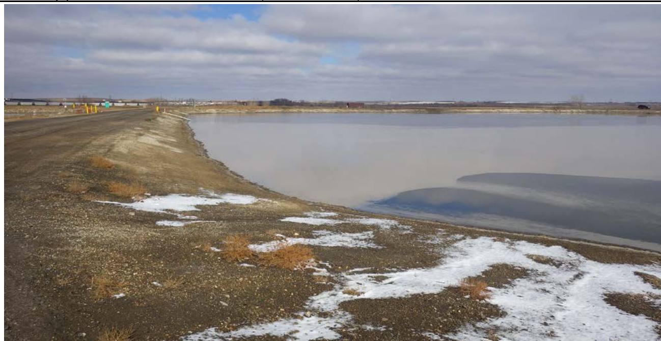
Photograph 20 (East cell west berm) Upstream slope and crest road, fly ash protective cover and gravel, good condition. (IMG_7448.JPG)
