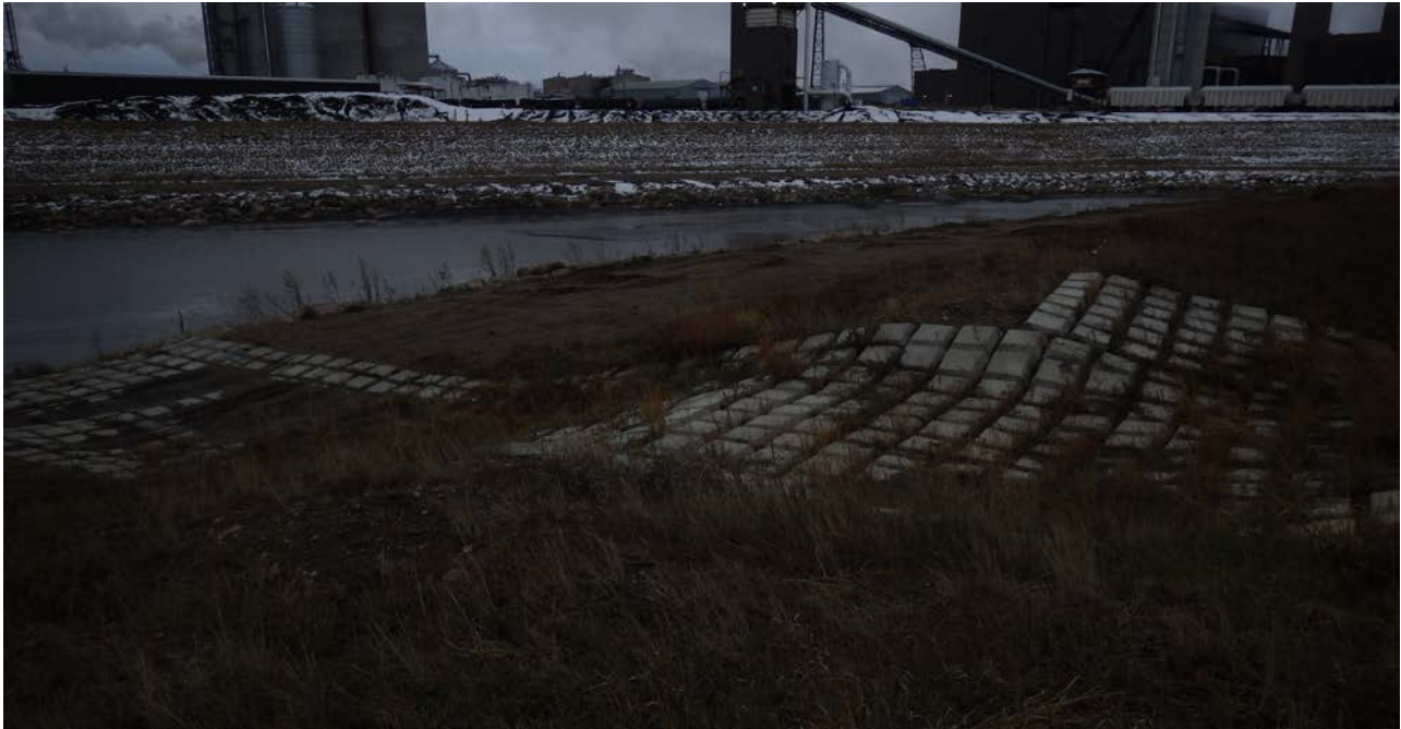
Photograph 11 (Center cell north berm) Stormwater downchute channel (concrete block armoring), good condition. (IMG_7377.JPG)
