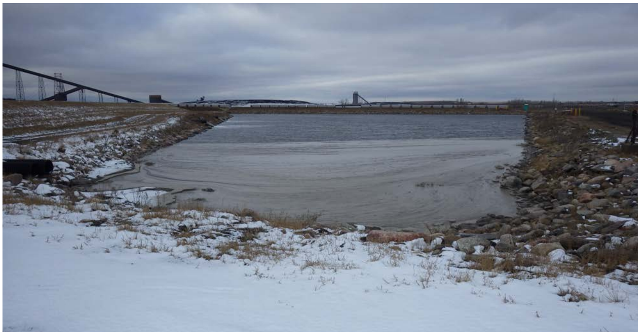
Photograph 13 (Center cell) View from south end, upstream slope riprap in good condition. (IMG_7381.JPG)
