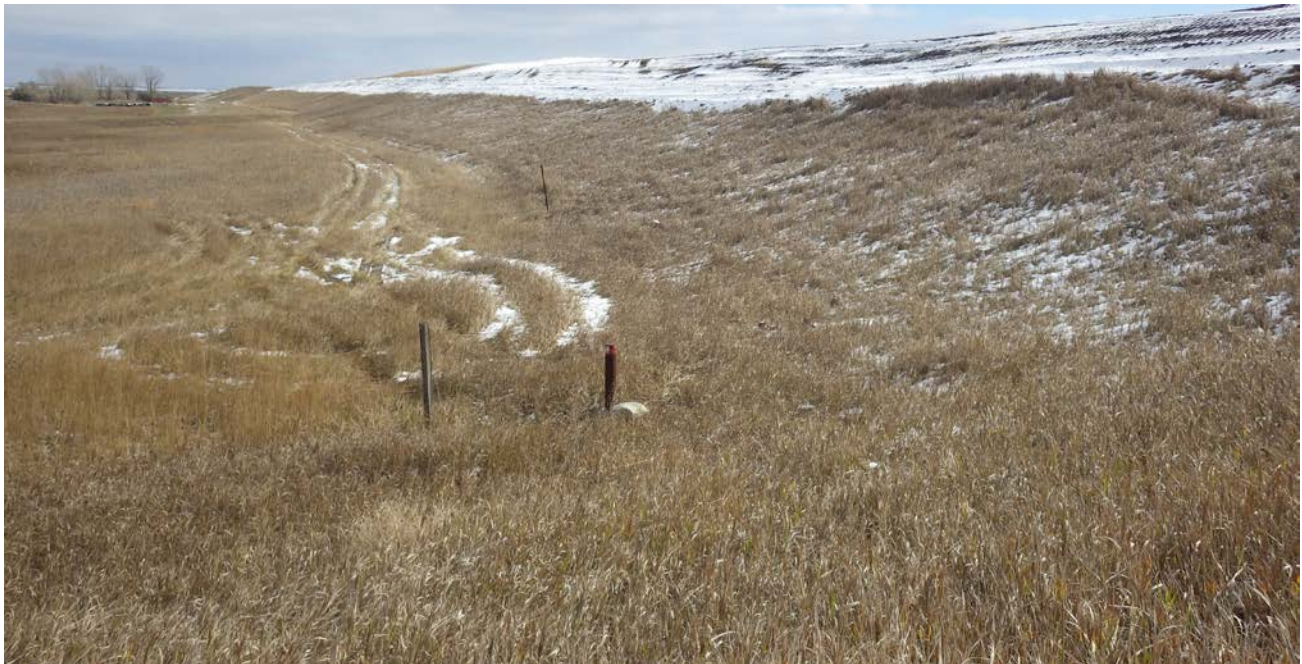
Photograph 18 (East cell east berm) Downstream slope and toe, good vegetation. (IMG_7445.JPG)
