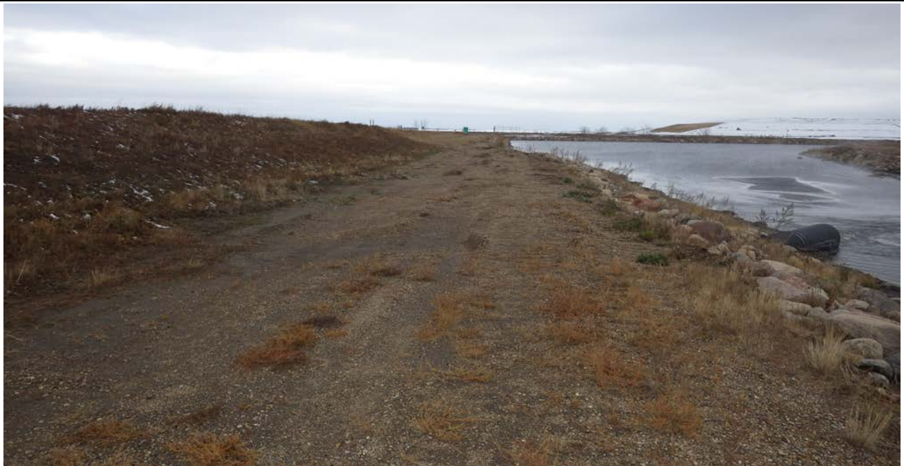
Photograph 10 (Center cell north berm) Crest road and upstream slope with gravel and riprap, good condition. (IMG_7375.JPG)
