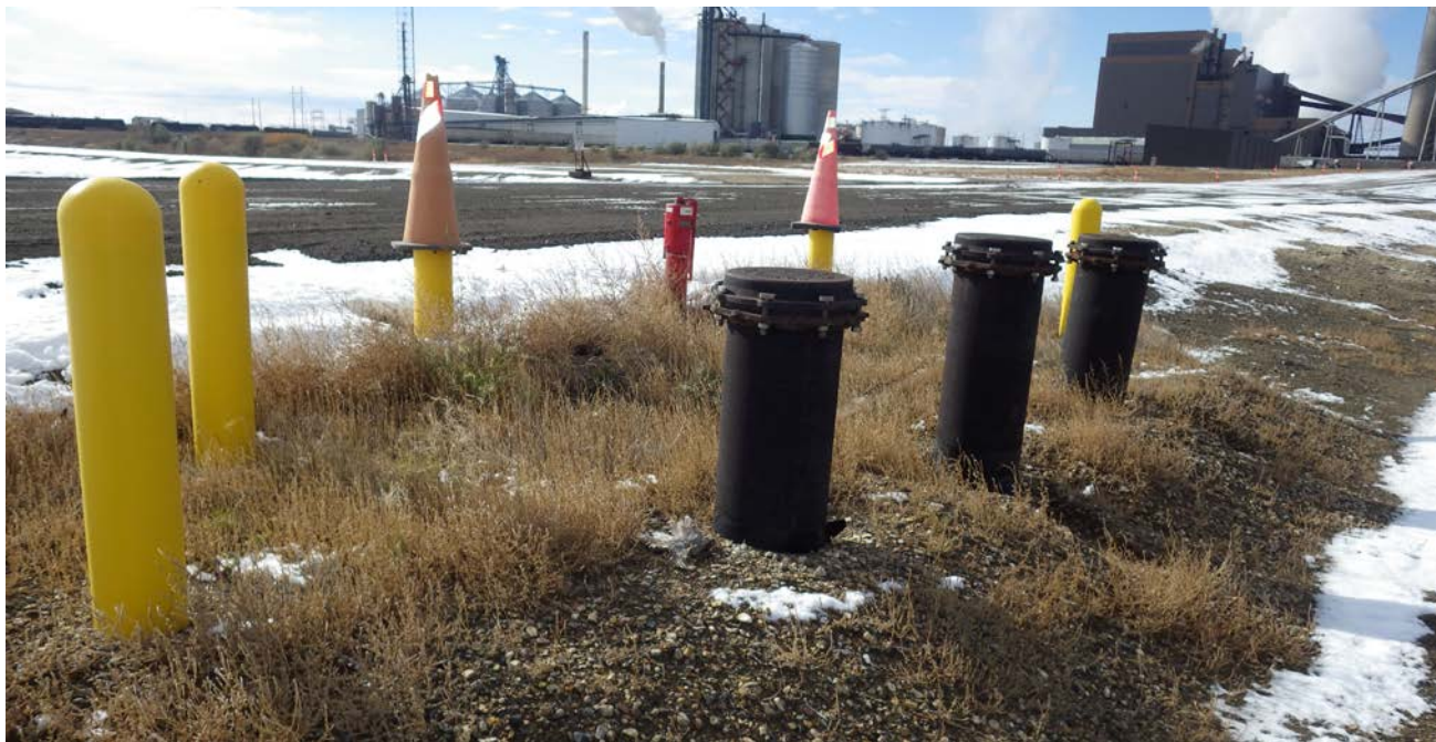
Photograph 19 (East cell south berm) Cross-over pipe cleanouts and valve control. (IMG_7446.JPG)
