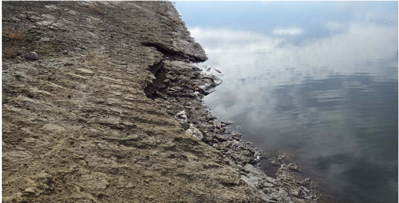
Photograph 17 (East cell east berm) Upstream slope fly ash protective cover, minor erosion at water line. (IMG_7443.JPG)
