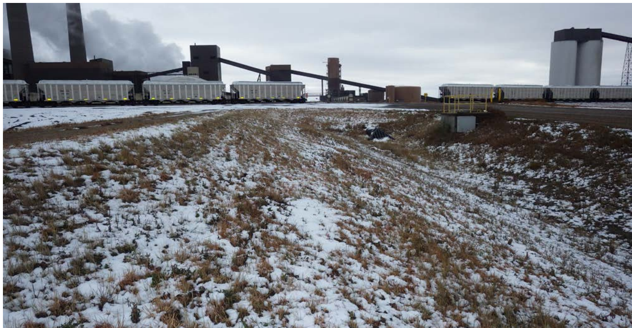
Photograph 3 (West cell north berm) Stormwater drainage on north side of west cell, good condition. (IMG_7359.JPG)
