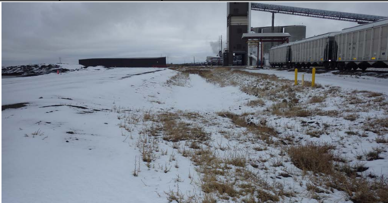
Photograph 4 (West cell west berm) Downstream slope and stormwater drainage, poor vegetation on slope. (IMG_7360.JPG)
