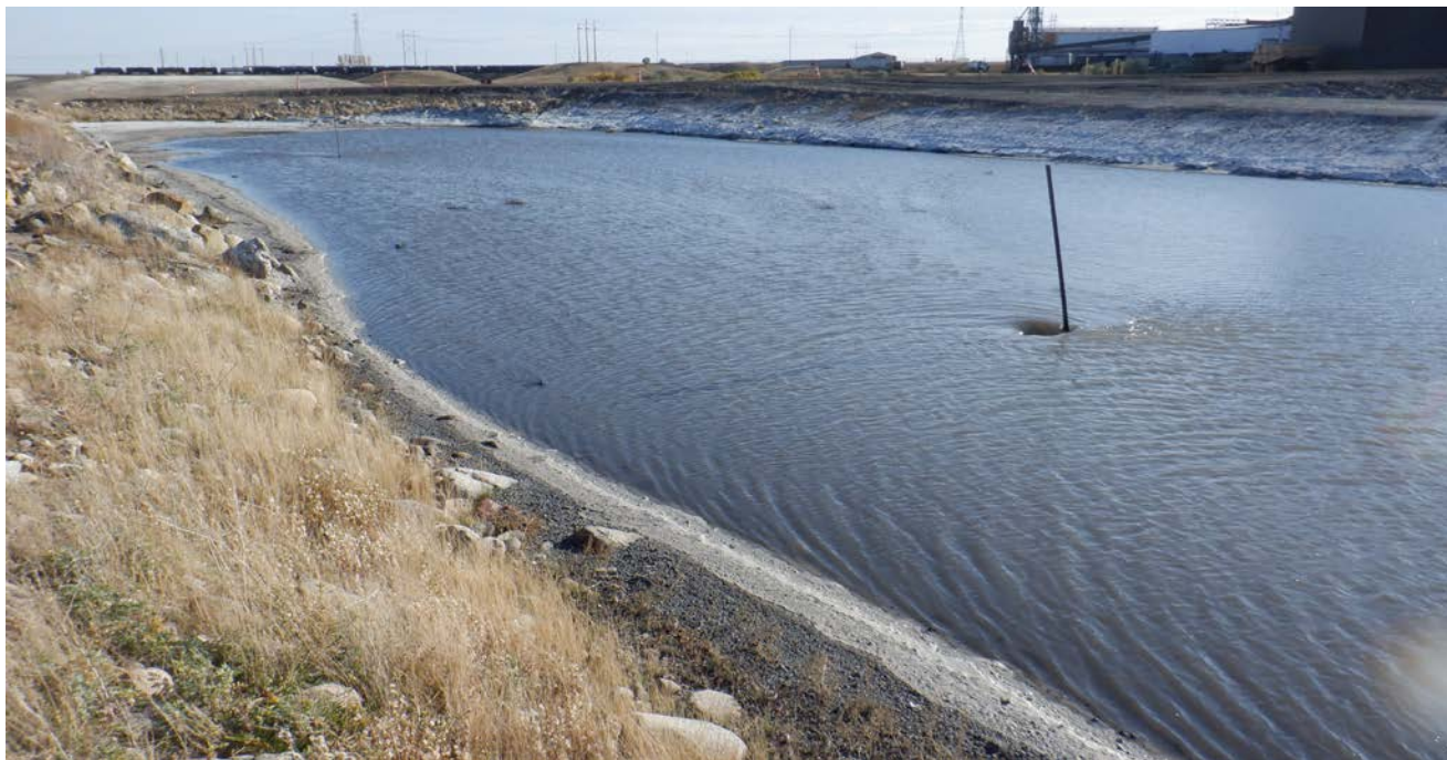
Photograph 23 (West cell east berm, center cell west berm) West cell upstream slope and decanting of water to center cell. (IMG_DSCF1795.JPG)
