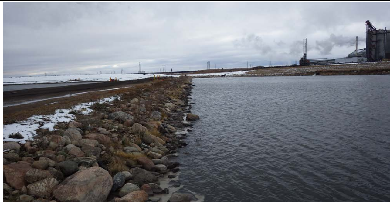
Photograph 12 (Center cell east berm) Upstream slope with riprap, good condition. (IMG_7378.JPG)
