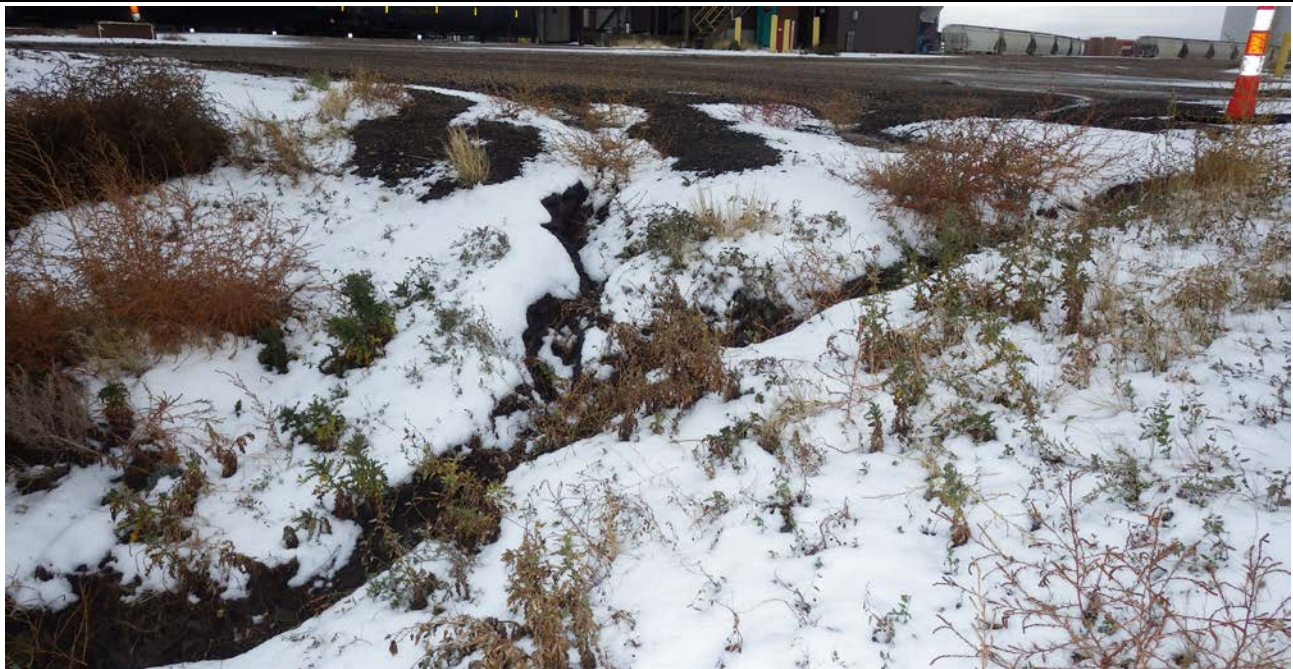
Photograph 6 (West cell south berm) Downstream slope, erosion rill. (IMG_7367.JPG)
