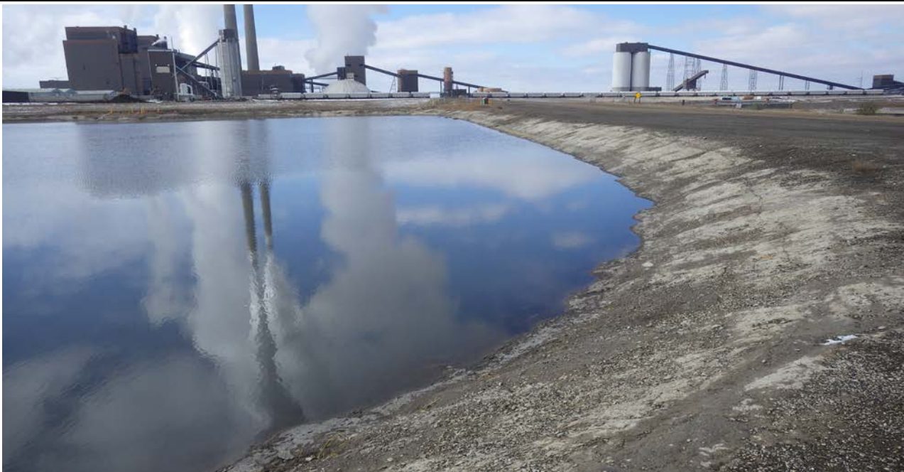
Photograph 14 (East cell north berm) Upstream slope fly ash protective cover, good condition. (IMG_7440.JPG)
