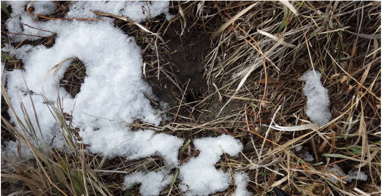
Photograph 16 (East cell east berm) Downstream slope, small animal burrow. (IMG_7442.JPG)
