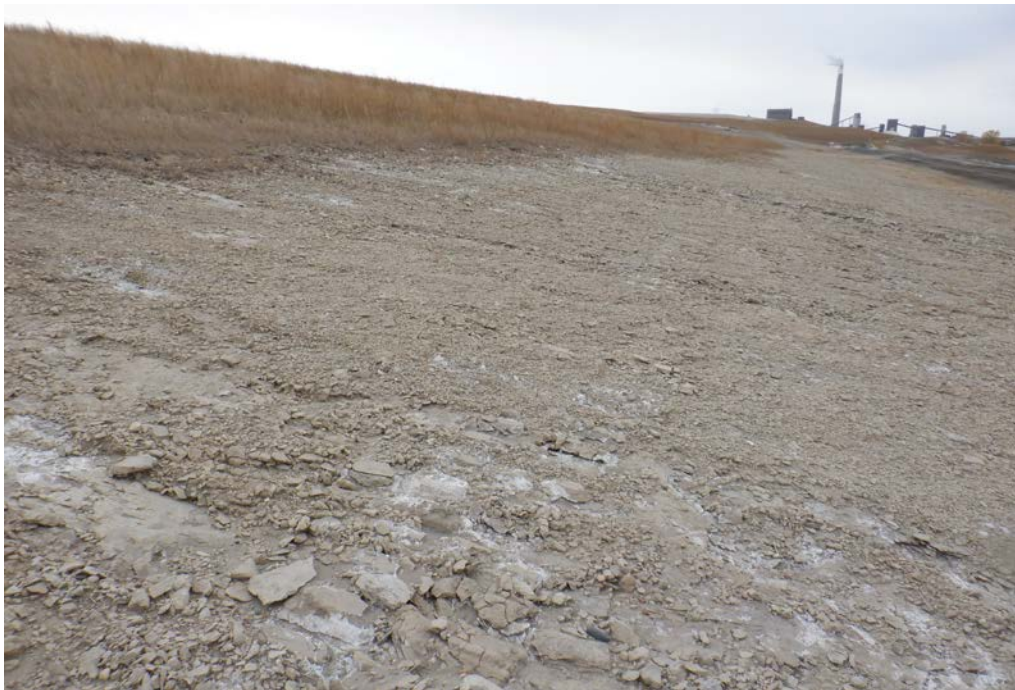
Photograph 6 (North CCR downstream slope) Minor erosion of fly ash slope. Upper temporary cover in good condition.
