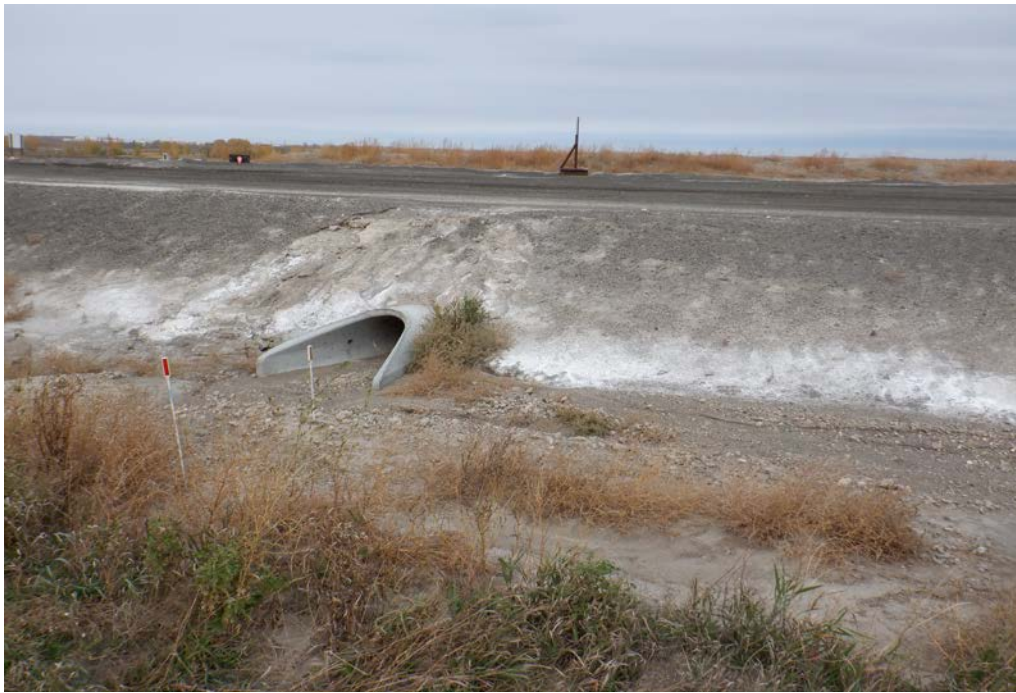
Photograph 9 (Northwest entrance) Concrete culvert and surface water drainage ditch. (IMG_DSCF1691.JPG)
