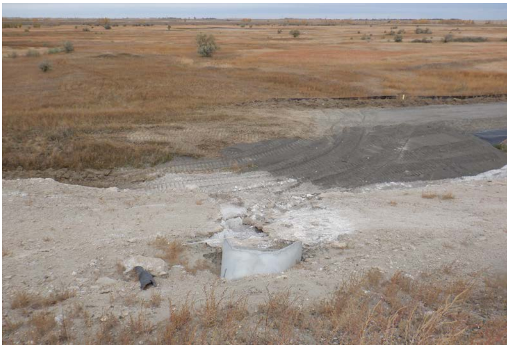
Photograph 8 (Northwest entrance) Erosion around culvert outlet to Contact Water Collection Channel. (IMG_DSCF1689.JPG)
