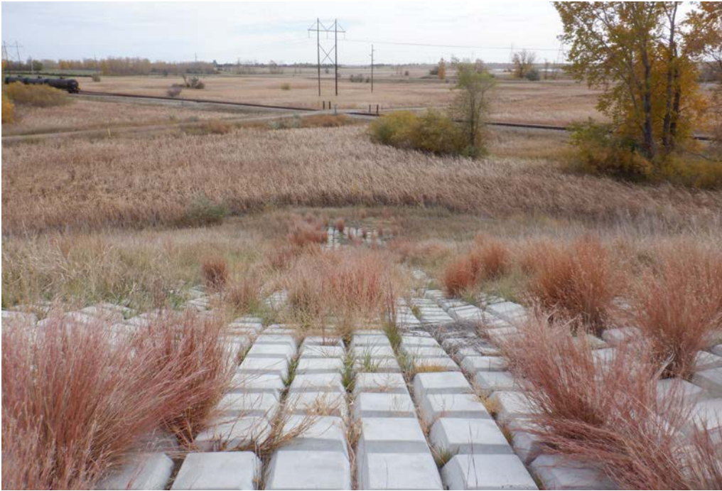
Photograph 17 (Southeast perimeter berm downstream slope) Southeast downchute channel. (DSCF1657.JPG)
