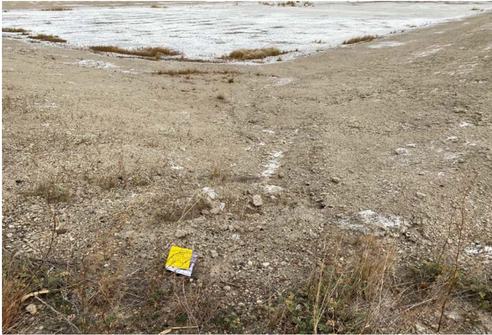
Photograph 11 (Contact water collection area perimeter berm upstream slope) Minor erosion of fly ash slope. (IMG_AD7P.JPG)
