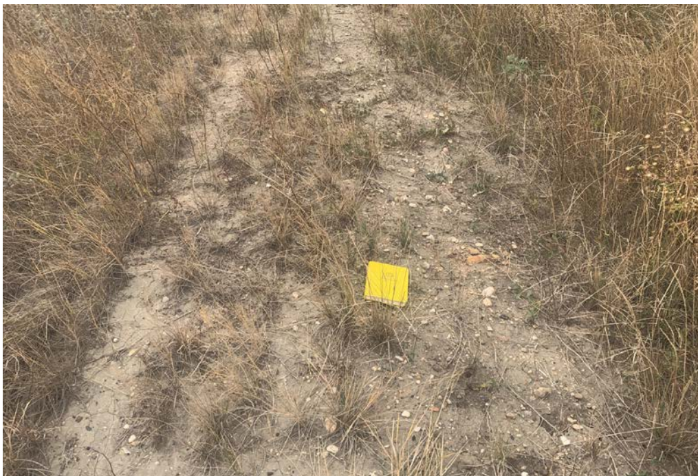
Photograph 14 (South final cover slope) Sparse vegetation on the crest of the southern terrace channel. (IMG_4581.JPG)
