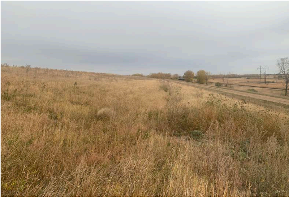
Photograph 15 (South final cover slope) Well vegetated final cover (typical final covered slopes) (IMG_4582.JPG)
