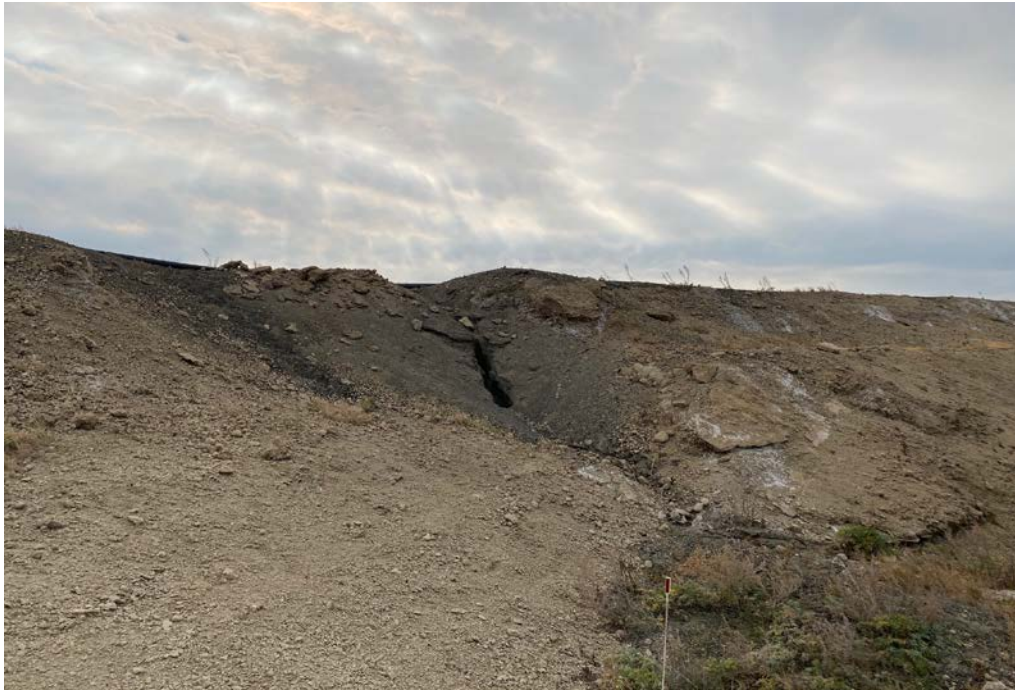
Photograph 13 (North CCR downstream slope (no cover)) Erosion of fly ash on SE16 north CCR downstream slope. (IMG_AD15P.JPG)
