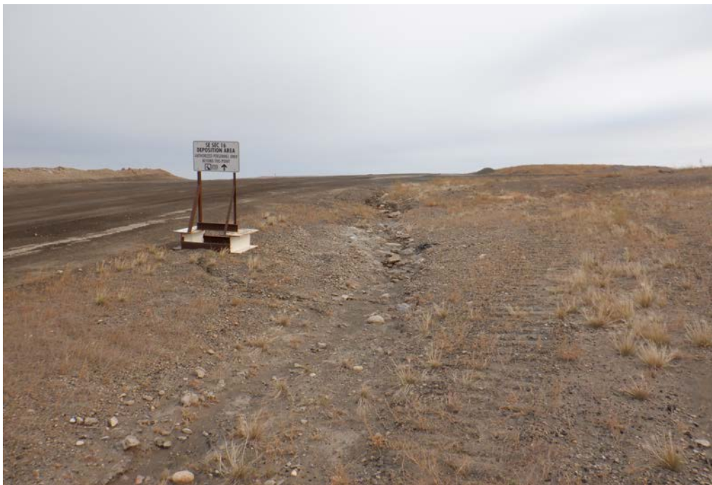
Photograph 10 (Northwest access ramp) Minor erosion along road to SE16 deposition area. (IMG_DSCF1693.JPG)
