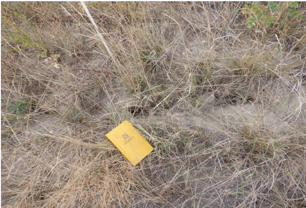
Photograph 2 (East CCR downstream slope (Temporary cover)) Animal burrows on temporary cover. (IMG_DSCF1664.JPG)
