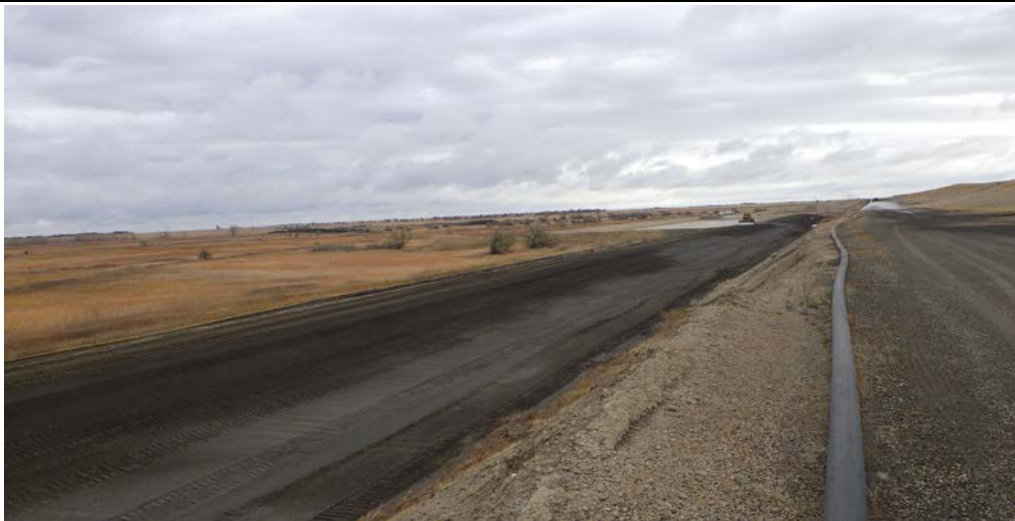
Photograph 12 (Haul Road) Protective cover (bottom ash) placed over exposed liner within the contact water collection channel. (IMG_RIMG0551.JPG)
