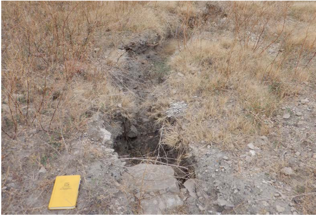
Photograph 5 (North CCR downstream slope (Temporary cover)) Erosion rill from contact water ditch. (IMG_DSCF1675.JPG)
