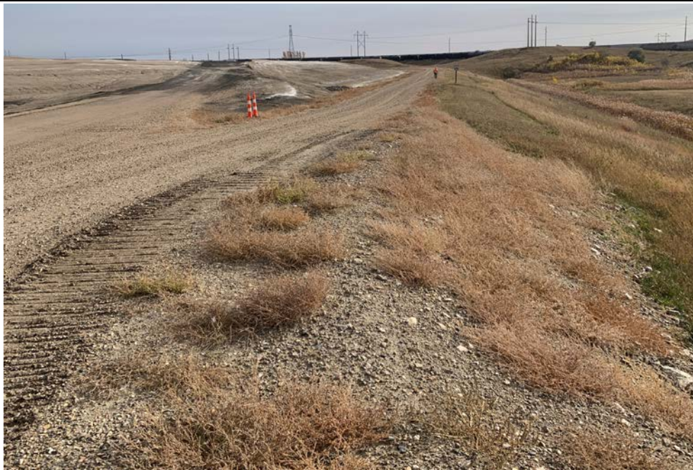
Photograph 11 (West perimeter berm crest and downstream slope) Well-vegetated perimeter downstream slope. Perimeter berm crest in good condition.
