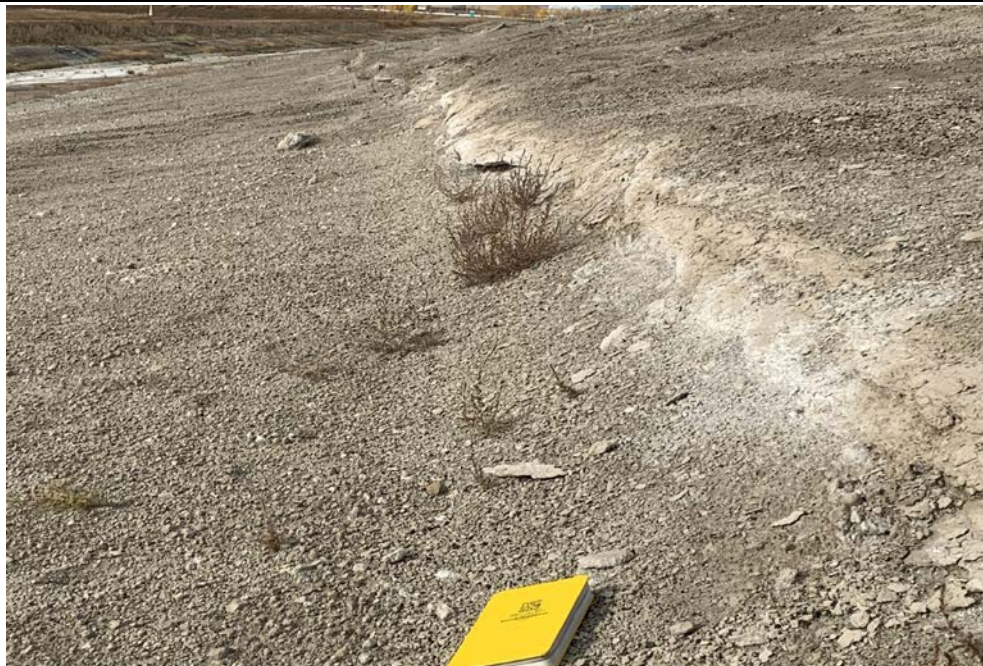
Photograph 13 (Northwest CCR downstream slope) Minor erosion of fly ash. (IMG_4599.JPG)
