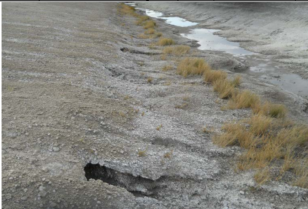
Photograph 10 (North CCR downstream slope) Minor erosion in fly ash to the perimeter contact water channel. (IMG_AD14.JPG)
