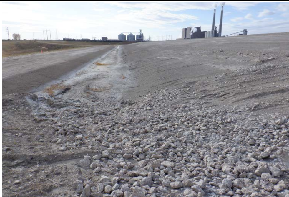
Photograph 5 (South perimeter channel) Concrete rubble erosion protection at southeast end of contact water channel.
