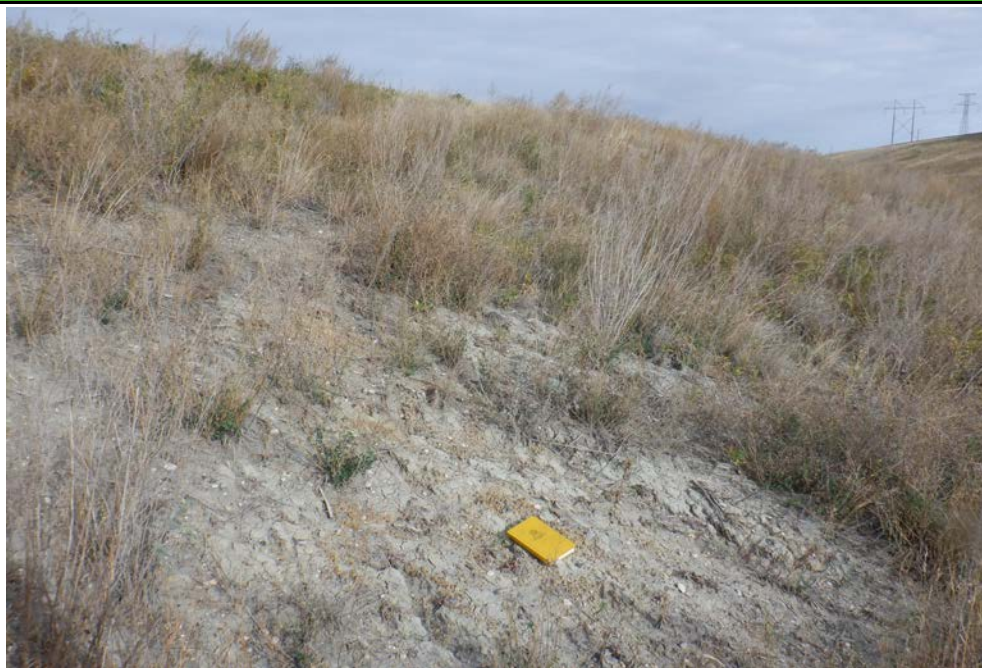
Photograph 1 (South berm downstream slope) Isolated area of sparse vegetation on downstream slope. (IMG_DSCF1699.JPG)
