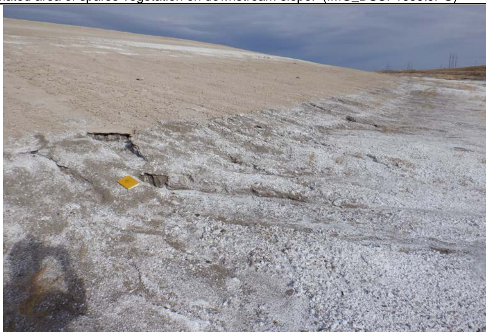
Photograph 2 (South CCR downstream slope (no cover)) Minor erosion of fly ash. (IMG_DSCF1700.JPG)
