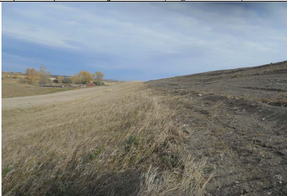
Photograph 8 (North perimeter berm downstream slope) Well-vegetated downstream slope and seed/mulch from recent haul road safety berm construction. (IMG_AD3.JPG)
