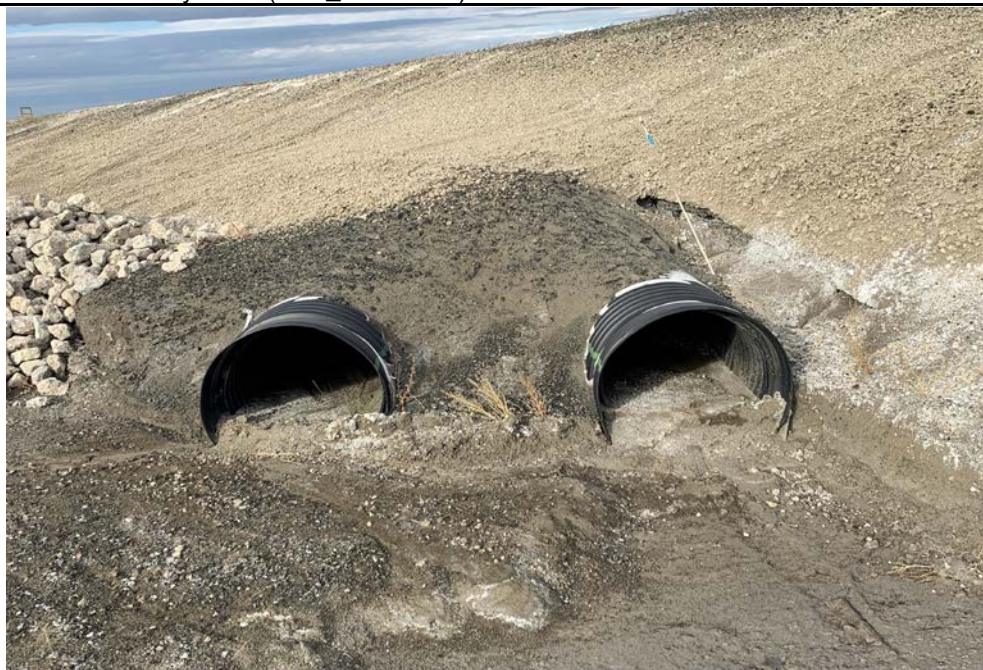
Photograph 14 (Northwest CCR downstream slope) Contact water culvert partially filled with sediment. (IMG_4601.JPG)
