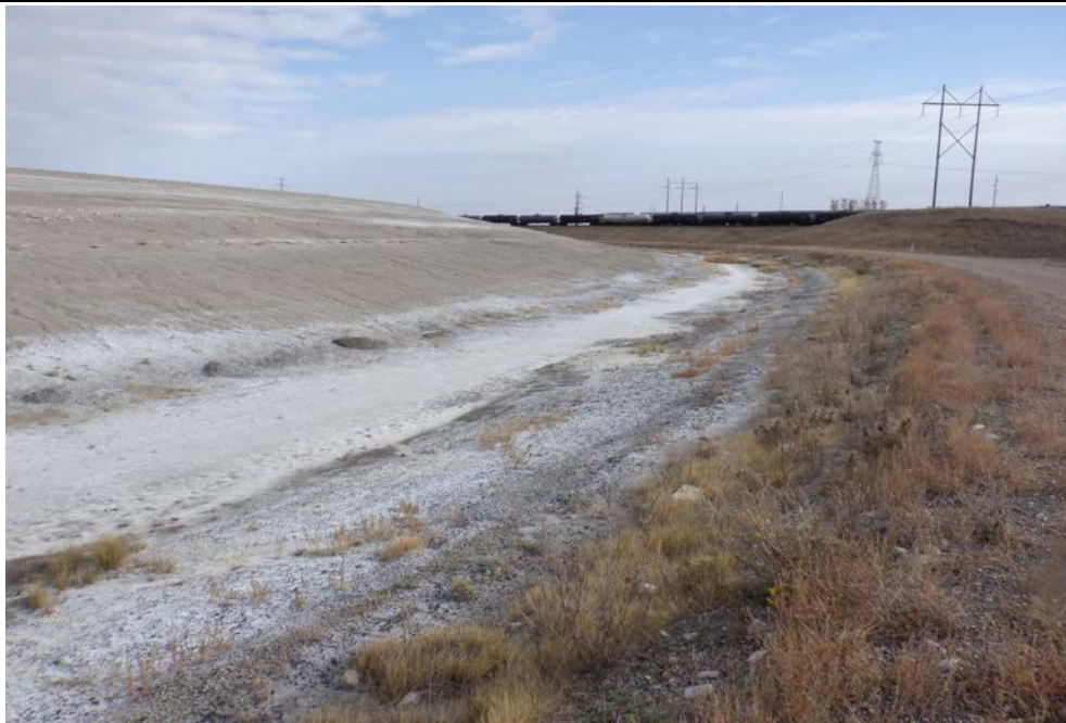
Photograph 9 (Southwest CCR downstream slope) Downstream CCR slope, perimeter contact water channel (dry), and perimeter berm upstream slope with a minor amount of vegetation present. (IMG_DSCF1696.JPG)
