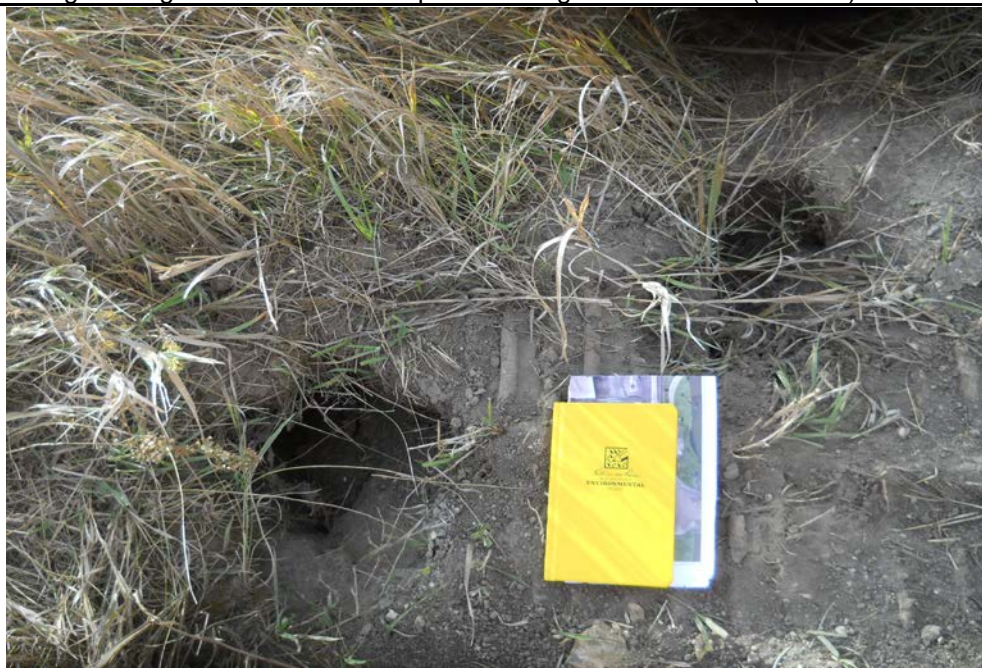
Photograph 20 (North perimeter berm downstream slope) Animal burrows (approximately 6-inch diameter). (9.JPG)
