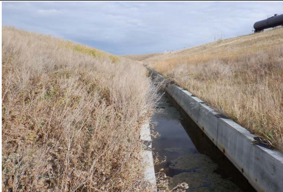
Photograph 17 (Perimeter berm downstream slope and toe) Site surface water drainage ditch and well-vegetated perimeter berm downstream slope. (DSCF1704.JPG)
