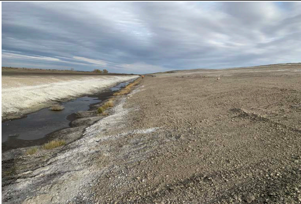
Photograph 15 (North CCR downstream slope) Perimeter contact water control channel. (IMG_4602.JPG)
