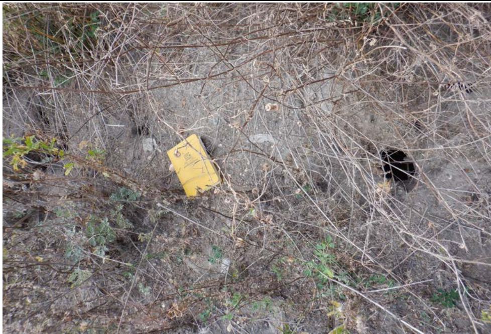
Photograph 3 (South berm downstream slope) Small (~2-inch diameter) animal burrows on downstream slope. (IMG_DSCF1714.JPG)
