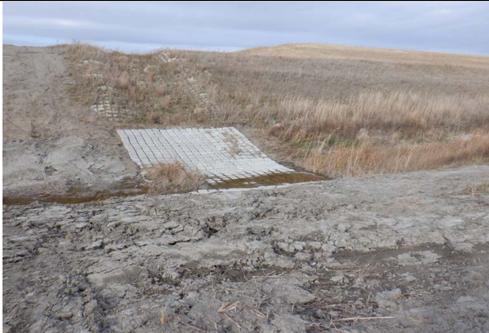
Photograph 4 (South berm downstream slope and site surface water drainage ditch) Downchute channel and recently constructed hydraulic jump basin requiring reseeding. (IMG_DSCF1719.JPG)
