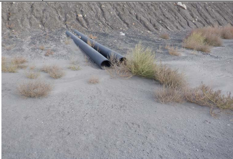
Photograph 18 (Inflow piping) Gravity drain inflow piping from Upstream Raise 92 in good condition. (DSCF1726.JPG)
