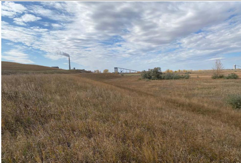
Photograph 22 (North perimeter berm downstream slope) Well-vegetated (grass) perimeter berm downstream slope and toe. (IMG_AD20P.JPG)
