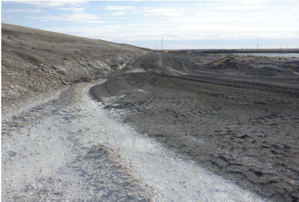
Photograph 3 (West CCR downstream slope (road)) Road between UR91 and UR92. (IMG_DSCF1751.JPG)
