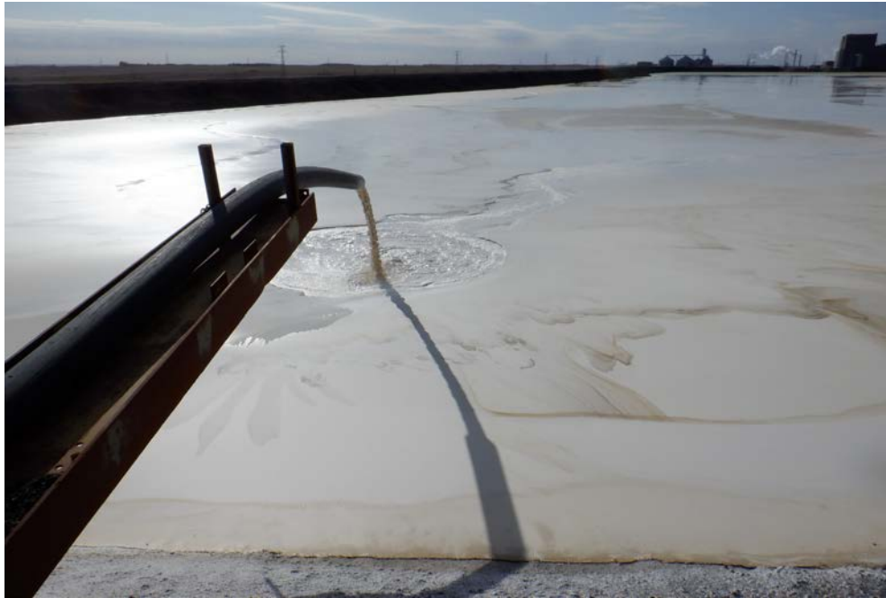
Photograph 19 (East side FGD pool ) Hydraulic deposition of FGD material on east side of Upstream Raise 92. (IMG_DSCF1782.JPG)
