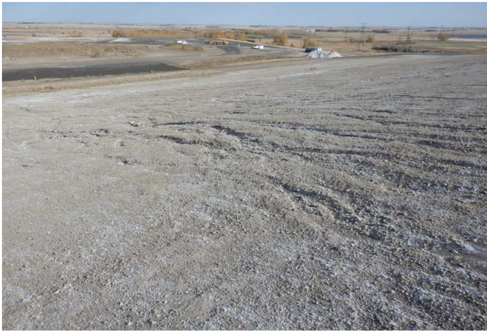
Photograph 12 (East CCR downstream (no cover)) Minor erosion of fly ash. (IMG_DSCF1783.JPG)
