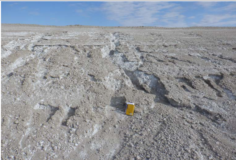
Photograph 4 (West CCR downstream slope (no cover)) Minor fly ash erosion near elevation 1998 feet on west downstream slope. (IMG_DSCF1754.JPG)
