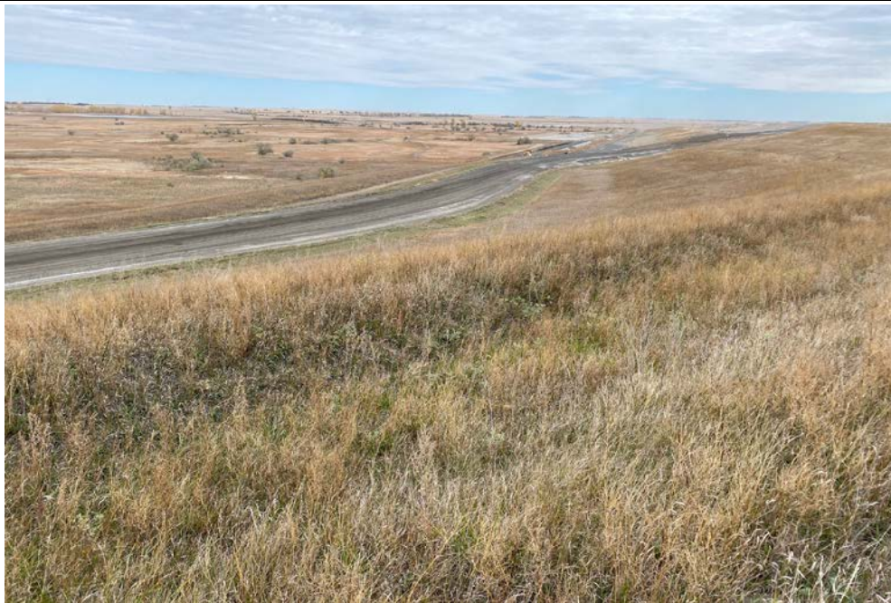
Photograph 16 (North CCR downstream slope (temporary cover)) Temporary vegetative cover on north slope, fair to good grass coverage. (IMG_AD13P.JPG)
