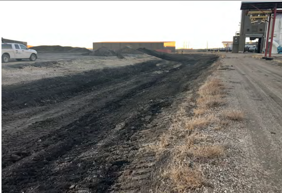
Photograph 2 Cleanout of west ditch grades prior to clay material placement, facing south. (IMG_3060.JPG)
