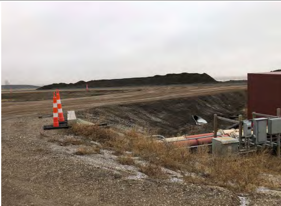
Photograph 10 Post-cleanout and placement of soil at the west ditch and newly installed culvert outlet, facing northeast. (RF-6.JPG)
