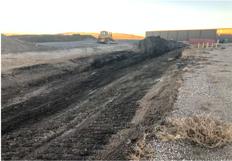
Photograph 3 Cleanout of west ditch grades prior to clay material placement, facing south-southeast. (IMG_3061.JPG)
