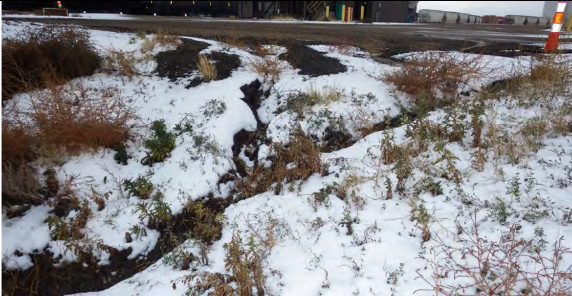
Photograph 4 Downstream slope and stormwater drainage, erosion rills from haul road. (IMGP7367.JPG)
