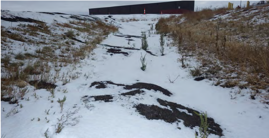
Photograph 3 Downstream slope and stormwater drainage, bottom ash (CCR) accumulated in the drainage ditch. (IMGP7364.JPG)
