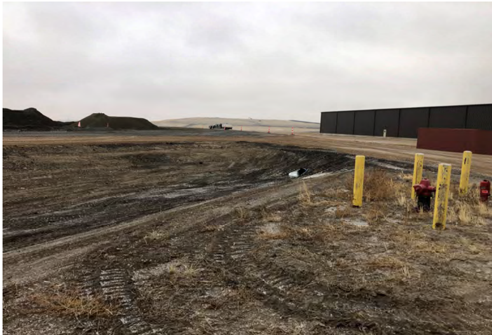
Photograph 8 Post-cleanout and placement of soil at the west ditch and newly installed culvert inlet, facing southeast. (RF-4.JPG)
