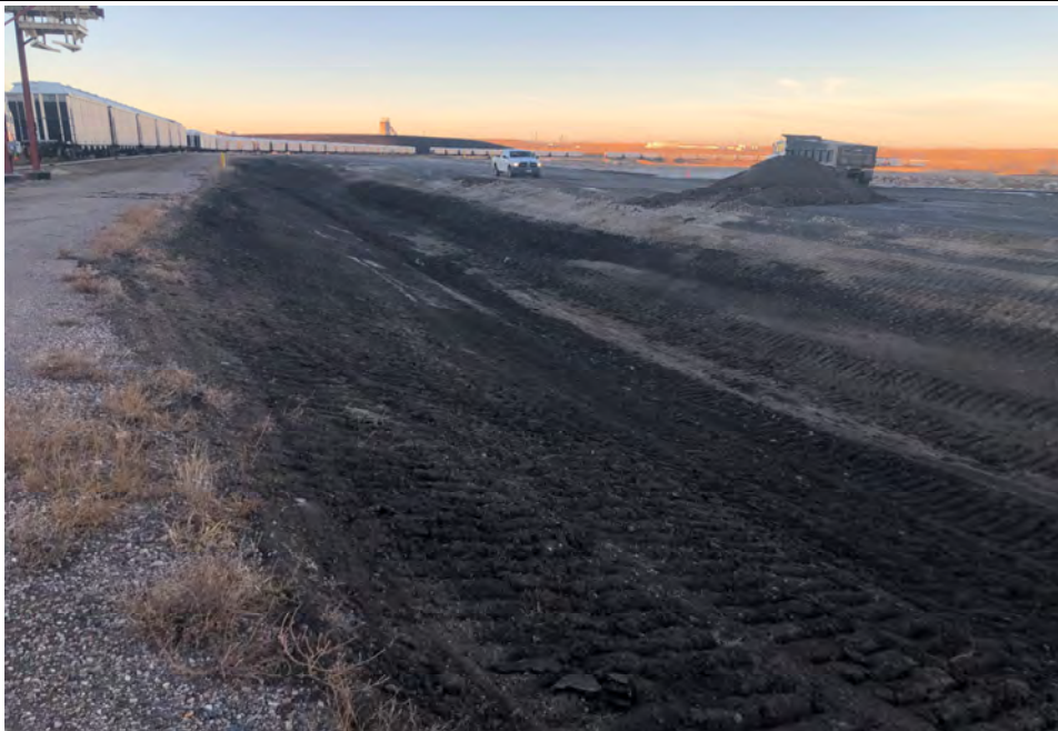
Photograph 4 Cleanout of west ditch grades prior to clay material placement, facing north. (IMG_3062.JPG)
