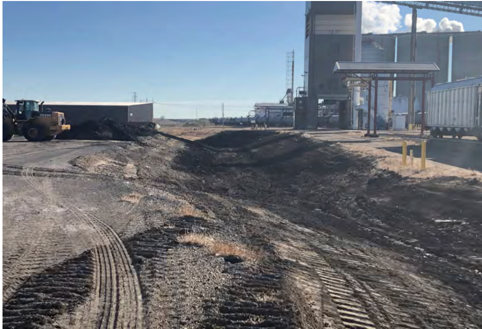
Photograph 1 Cleanout and stockpiling of bottom ash and affected soil, facing south. (IMG_3051.JPG)
