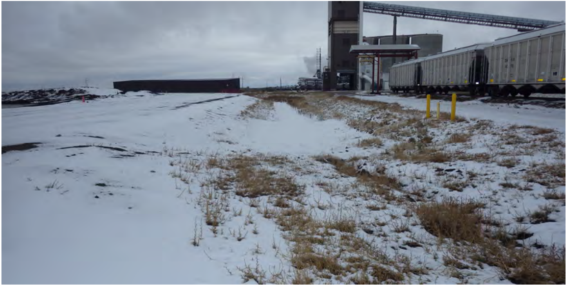
Photograph 1 Downstream slope and stormwater drainage, poor vegetation on slope. (IMGP7360.JPG)
