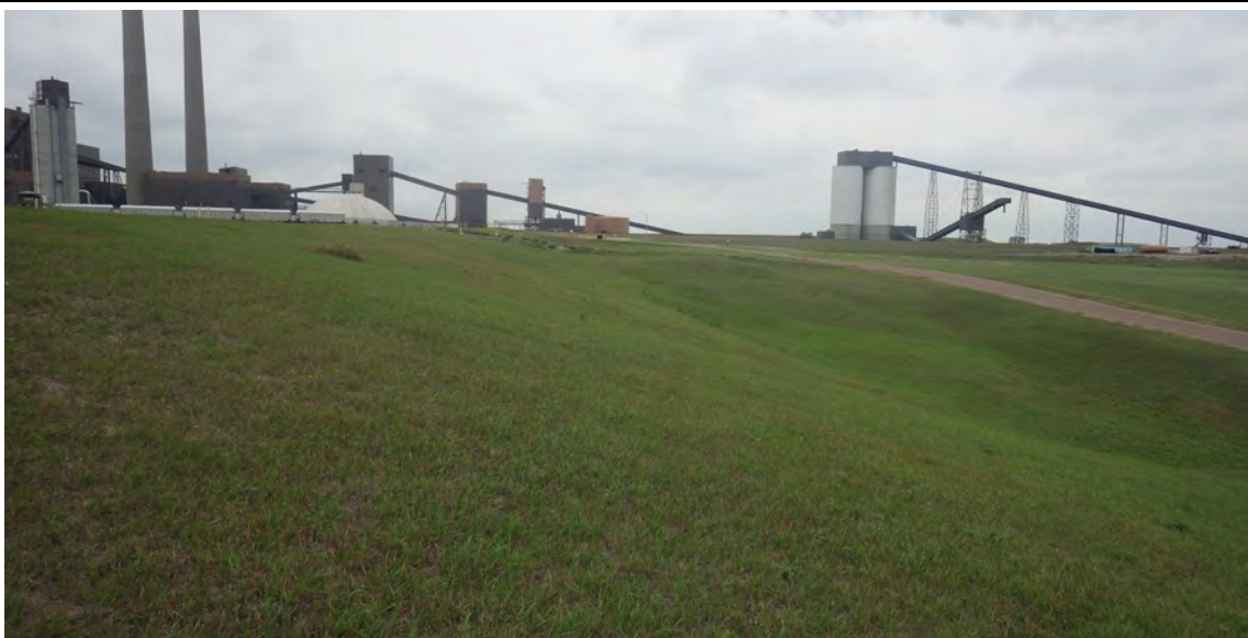
Photograph 2 (West cell, north downstream slope) Well vegetated north downstream slope of west cell, good condition. (IMGP8046.JPG)
