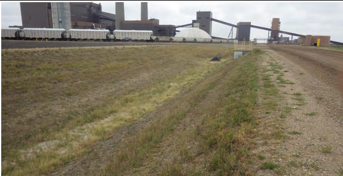
Photograph 3 (West cell, north ditch) Surface water ditch north of the west cell, clear of obstructions. (IMGP8049.JPG)
