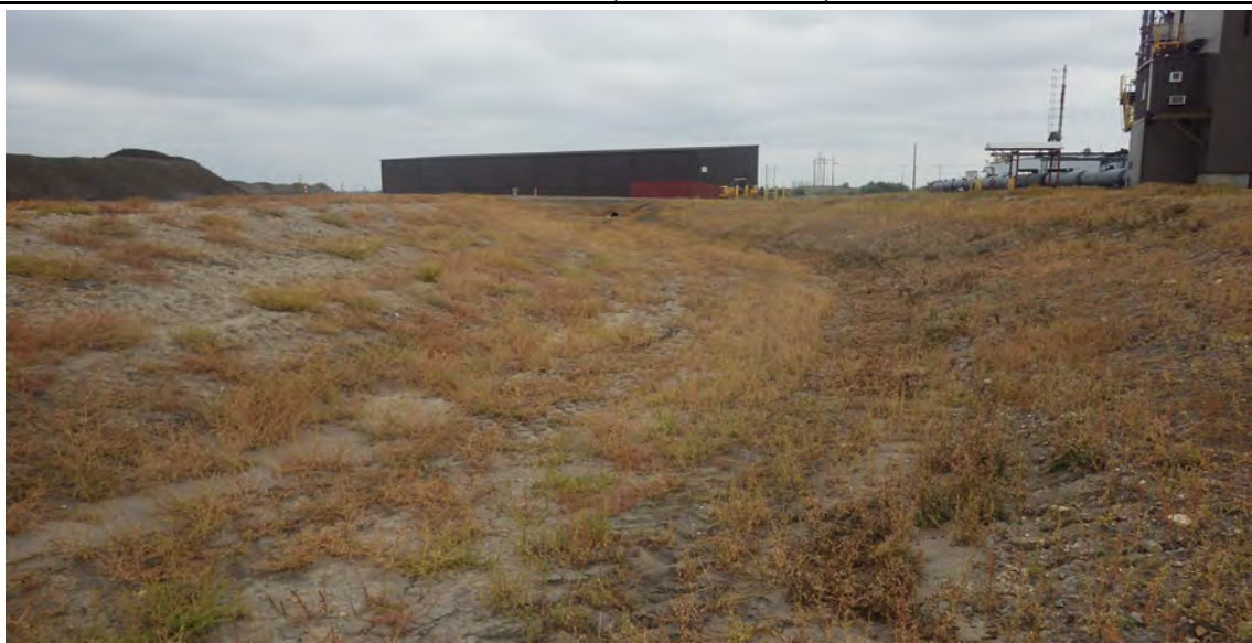
Photograph 6 (West cell, west downstream slope) Downstream slope and stormwater drainage ditch, fair vegetation on slope. (IMGP8054.JPG)
