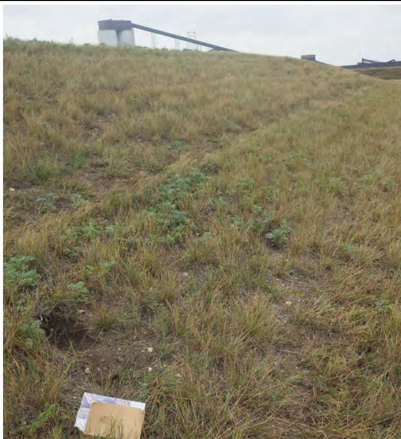
Photograph 17 (West cell, east downstream slope) Grass slope between the center cell and west cell, small animal burrow. (IMG8072.JPG)
