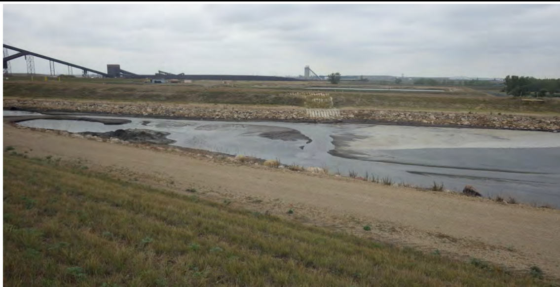
Photograph 18 (Center cell, northwest upstream slope) Stormwater drainage downchute and plant drains inlet to the center cell. (IMG8074.JPG)
