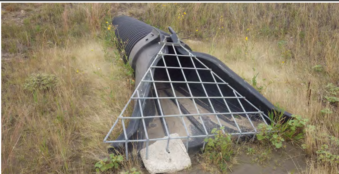
Photograph 4 (West cell, north ditch) Culvert outlet in the northwest corner of west cell, trash rack partly disconnected. (IMGP8050.JPG)
