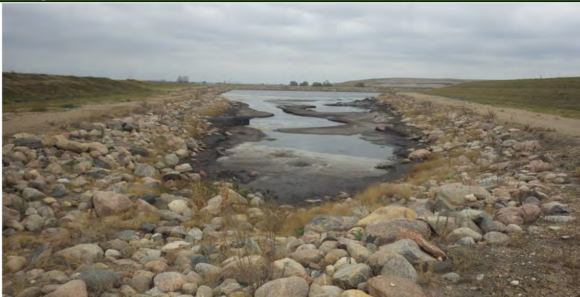
Photograph 19 (Center cell, northwest upstream slope) Center cell upstream slope in good condition, sediment accumulation around plant drains inlet. (IMGP8076.JPG)
