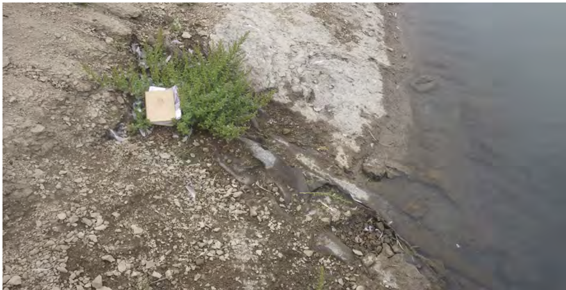
Photograph 21 (East cell, upstream slope) Erosion of fly ash protective cover, minor exposed geotextile. (IMGP8080.JPG)
