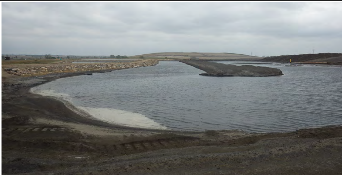
Photograph 5 (West cell) West cell interior, bottom ash sediment control berm. (IMGP8052.JPG)
