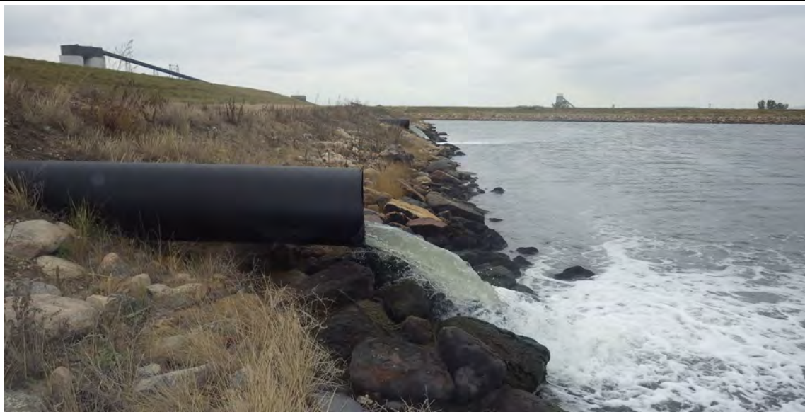
Photograph 15 (Center cell, west upstream slope) Decant outlets to center cell. (IMGP8070.JPG)
