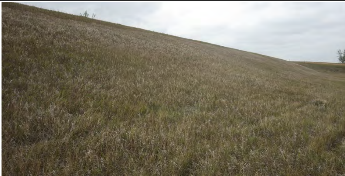
Photograph 22 (East cell, east downstream slope) Well vegetated east cell downstream slope and toe, good condition. (IMGP8083.JPG)
