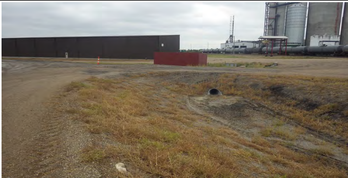
Photograph 7 (West cell, west downstream slope) Culvert inlet from the west stormwater drainage ditch to the ash line ditch, clear of obstructions. (IMGP8055.JPG)
