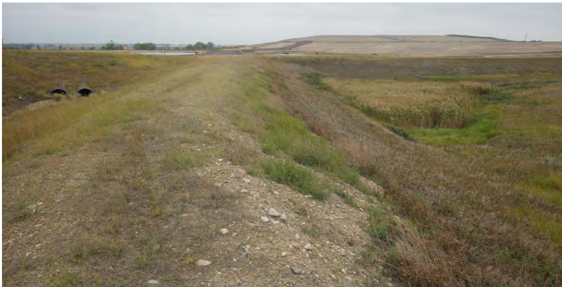
Photograph 13 (West cell, south downstream slope) South side of the west cell downstream slope, fair vegetation. (IMGP8066.JPG)
