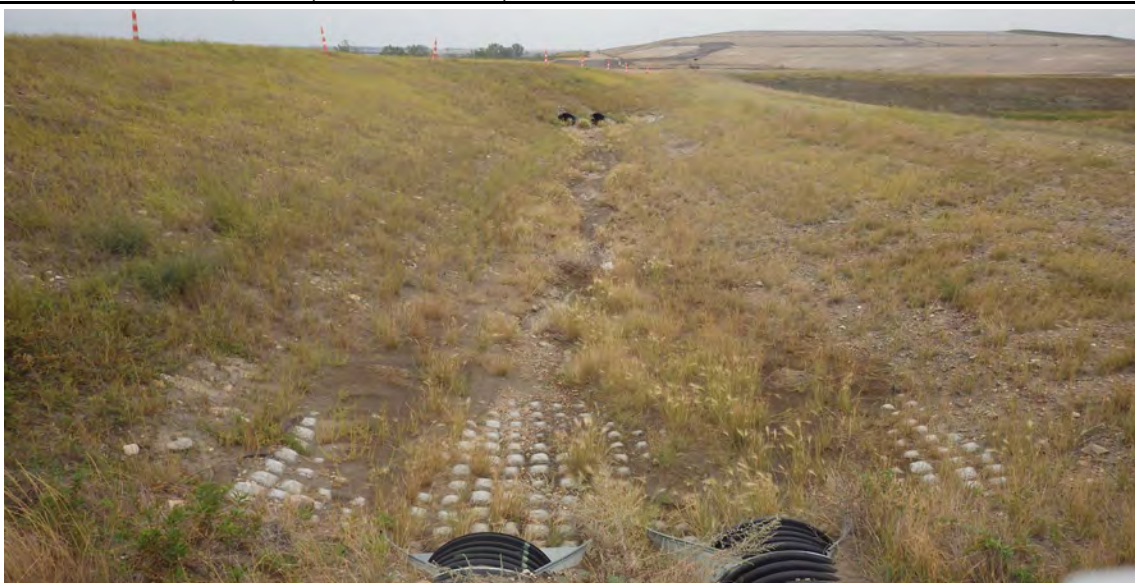
Photograph 12 (West cell, south downstream slope) Culverts and erosion protection south of the west cell, good condition. (IMGP8064.JPG)
