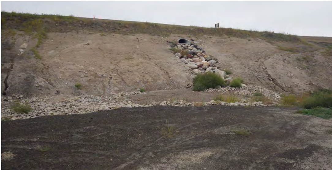
Photograph 12 (North CCR downstream slope) Culvert outlet to contact water collection area, armoring in good condition. (IMGP8021.JPG)
