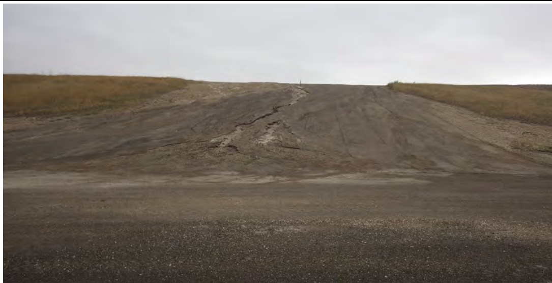
Photograph 13 (North CCR downstream slope) Minor erosion on slope reinforced with fly ash, fair condition. (IMGP8025.JPG)
