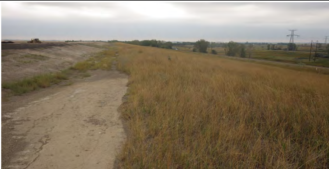
Photograph 17 (South CCR downstream slope and crest) Contact water separation berm and temporary cover in good condition. (IMGP8036.JPG)
