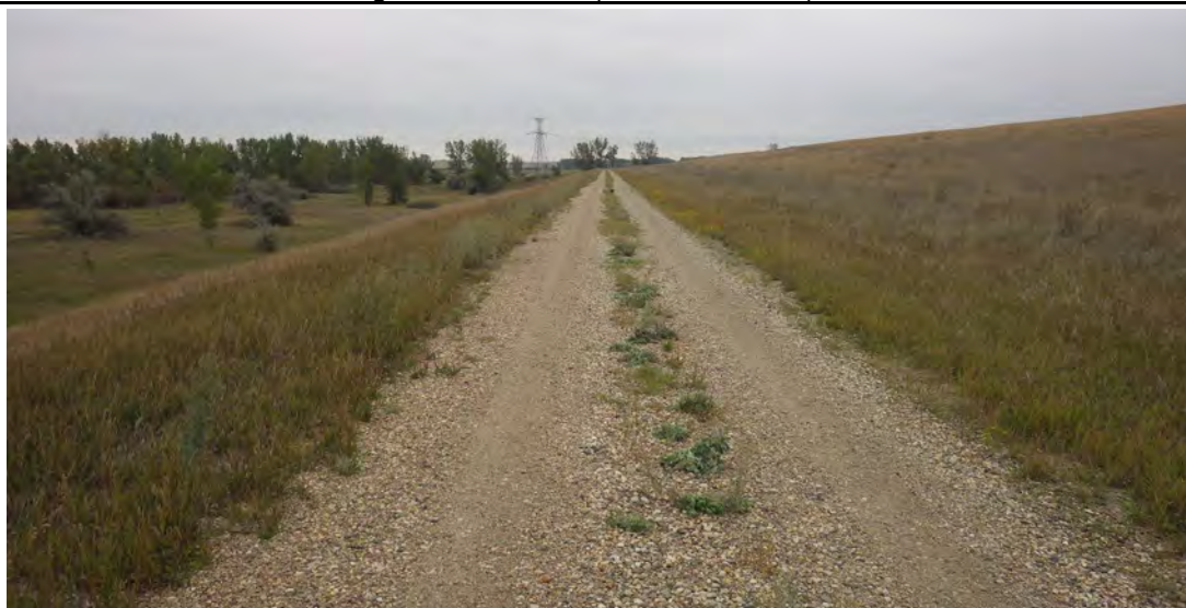
Photograph 6 (East perimeter access road) Perimeter berm gravel road, good condition. (IMG8002.JPG)
