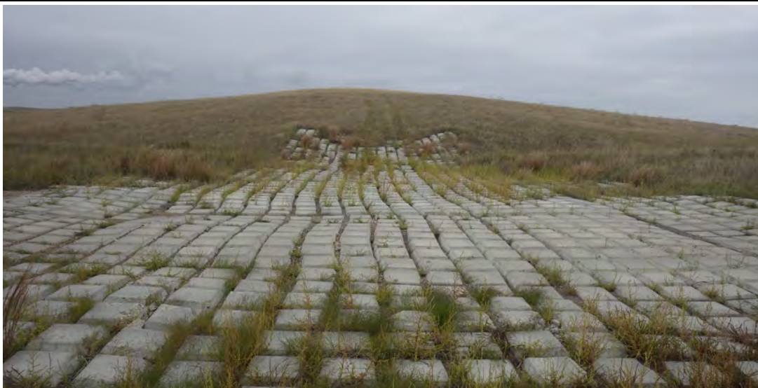
Photograph 1 (Southeast perimeter, downchute) Looking upslope, articulated concrete block in good condition. (IMGP7987.JPG)
