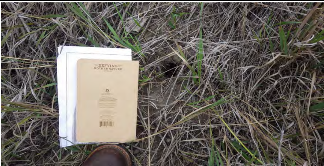
Photograph 2 (Southeast perimeter downstream slope) Small animal burrow. (IMGP7988.JPG)
