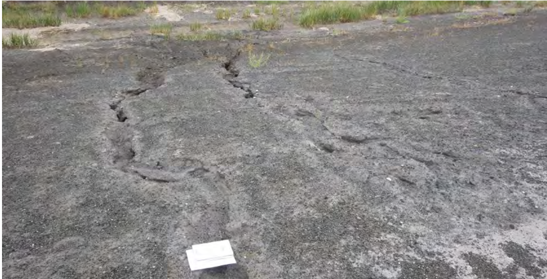
Photograph 11 (North perimeter downstream slope) Minor erosion of the bottom ash upstream slope, no liner visible (typical of approximately 5 locations on north perimeter berm upstream slope). (IMGP8019.JPG)
