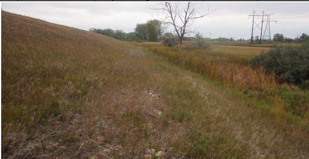
Photograph 18 (South perimeter downstream slope and toe) Well vegetated original toe drain and drainage channel along toe. (IMGP8040.JPG)
