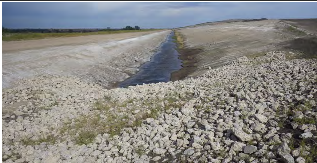
Photograph 4 (North perimeter berm crest, upstream slope, and CCR downstream slope) North perimeter ditch with approximately 6 to 12 inches of standing water and concrete rubble erosion protection near culvert inlets. (IMGP7903.JPG)
