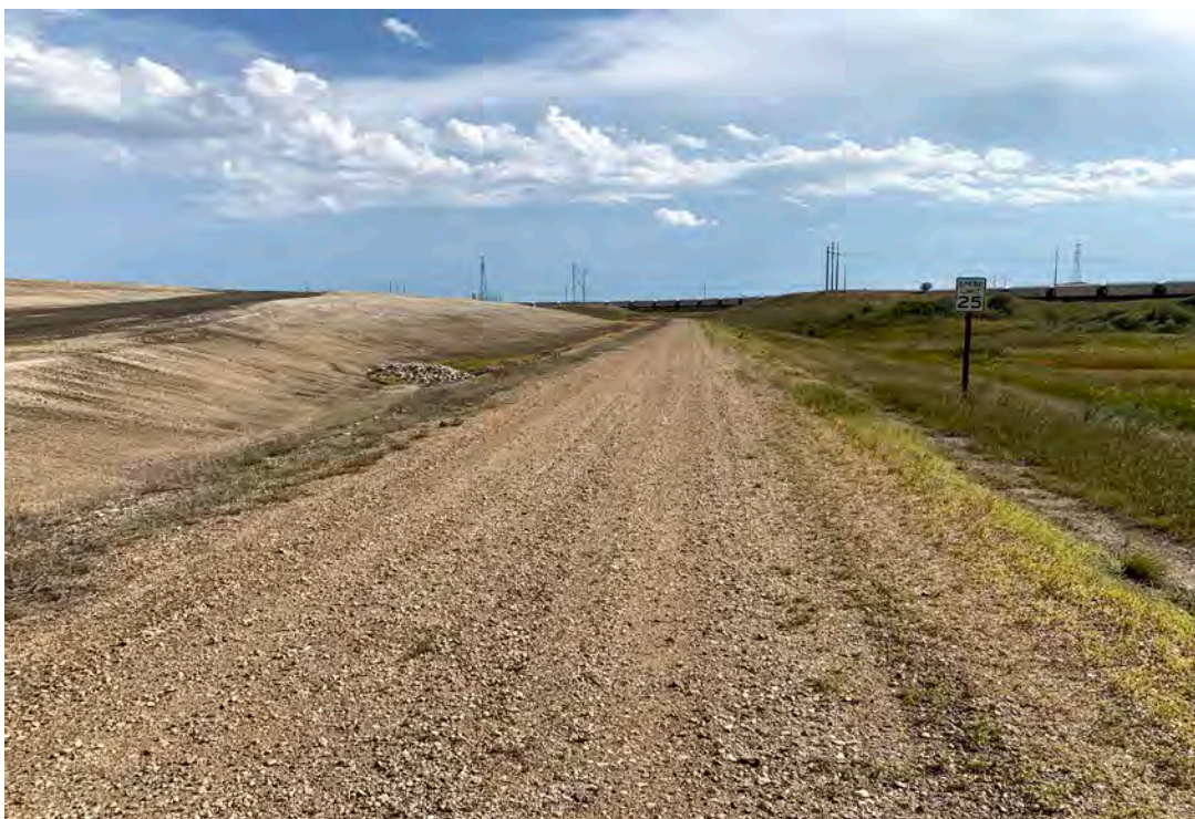
Photograph 16 (West perimeter berm crest) Perimeter berm crest, gravel in good condition. (IMGP2787.JPG)
