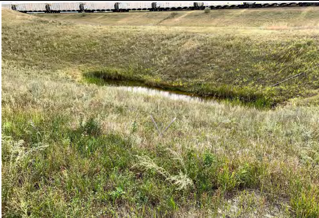
Photograph 22 (Southwest perimeter berm downstream slope) Standing water in perimeter ditch at toe of slope. (IMGP2798.JPG)
