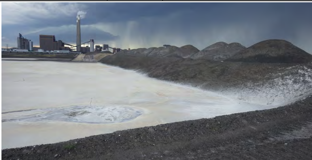
Photograph 12 (North CCR upstream slope) CCR upstream slope and FGD deposition area, good condition. (IMGP7923.JPG)
