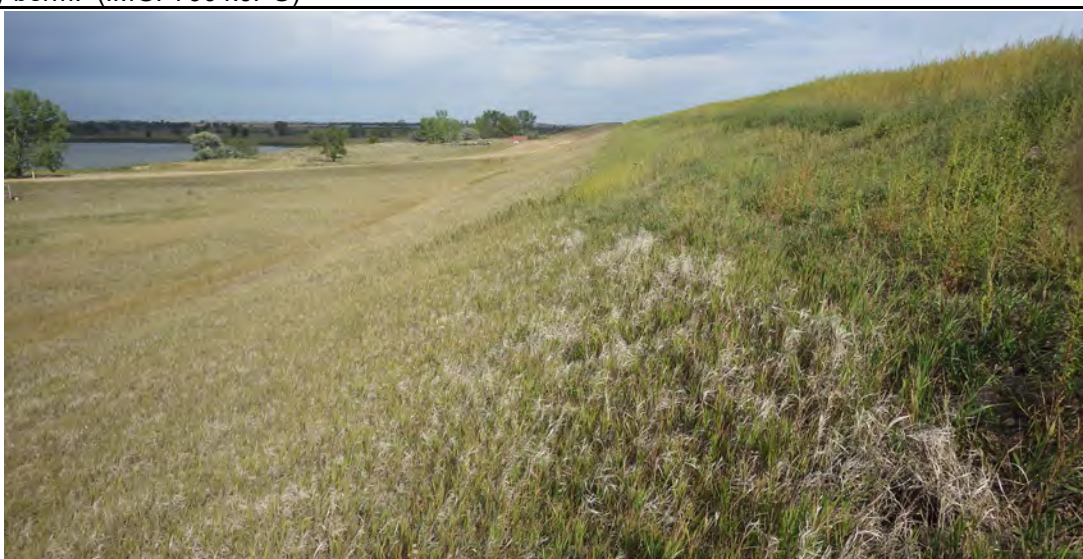
Photograph 6 (North perimeter berm downstream slope) Downstream slope well vegetated with grass, safety berm near crest has mostly weedy vegetation, overall good condition. (IMGP7905.JPG)
