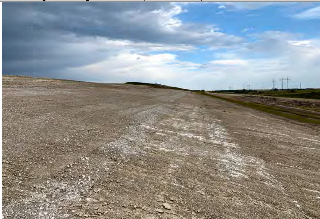
Photograph 26 (South CCR downstream slope) Fly ash slope, good condition. (IMGP2804.JPG)
