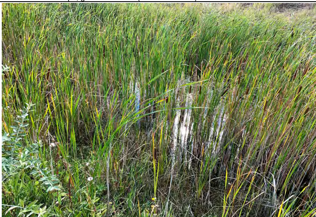
Photograph 18 (West perimeter berm downstream slope and toe) Standing water and cattails at the toe. (IMGP2789.JPG)
