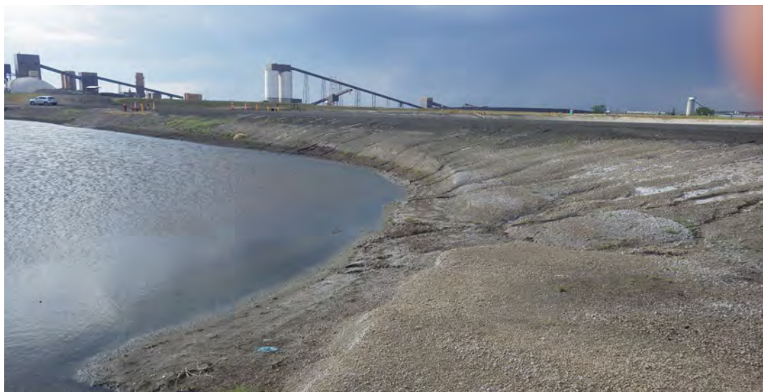
Photograph 3 (North perimeter berm upstream slope) Minor erosion of fly ash protective cover on upstream slope. (IMGP7902.JPG)
