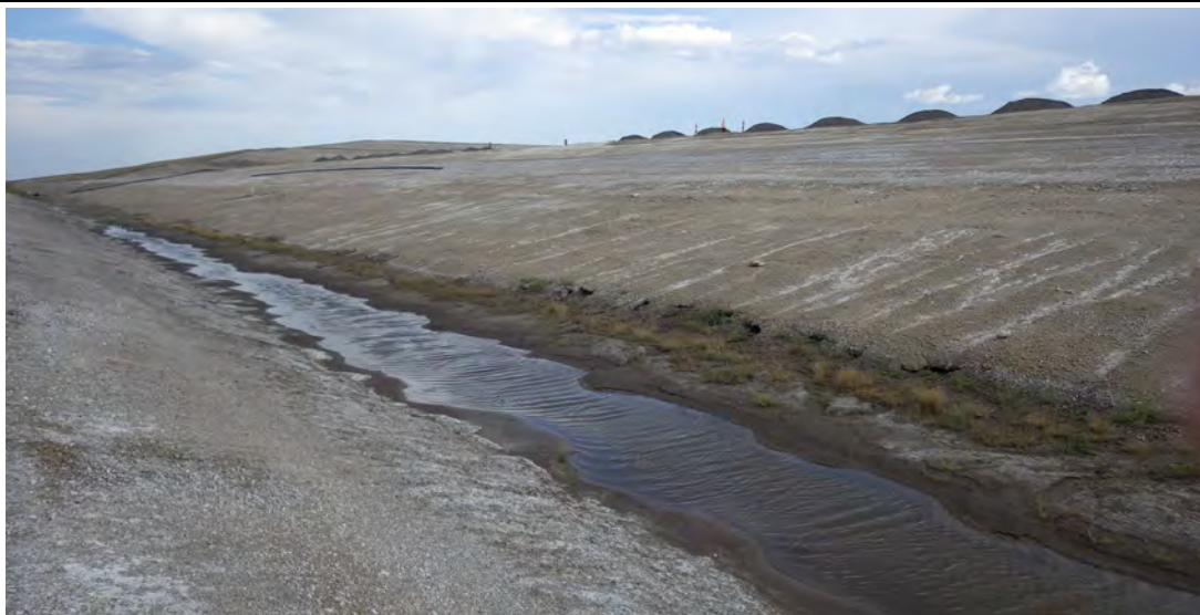
Photograph 7 (North CCR downstream slope) Minor erosion of fly ash CCR downstream slope and 6 to 12 inches of water present in perimeter ditch. (IMGP7910.JPG)
