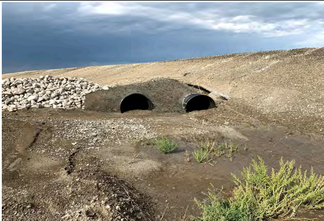
Photograph 19 (West CCR downstream slope) Perimeter channel culverts partially obstructed by erosion of fly ash and bottom ash. (IMGP2790.JPG)
