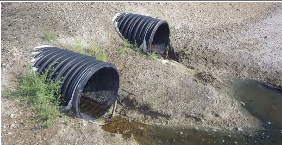
Photograph 2 (North perimeter berm upstream slope) Culvert outlets from north perimeter ditch. (IMGP7901.JPG)
