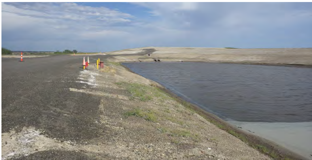
Photograph 1 (North perimeter berm upstream slope and crest) Haul road and fly ash protective cover on upstream perimeter berm slope in good condition. (IMGP7898.JPG)
