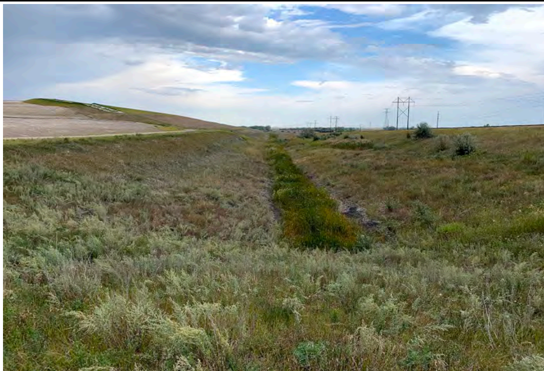
Photograph 28 (Southeast perimeter berm downstream slope and toe) Well-vegetated downstream slope and toe, good condition. (IMG2807.JPG)
