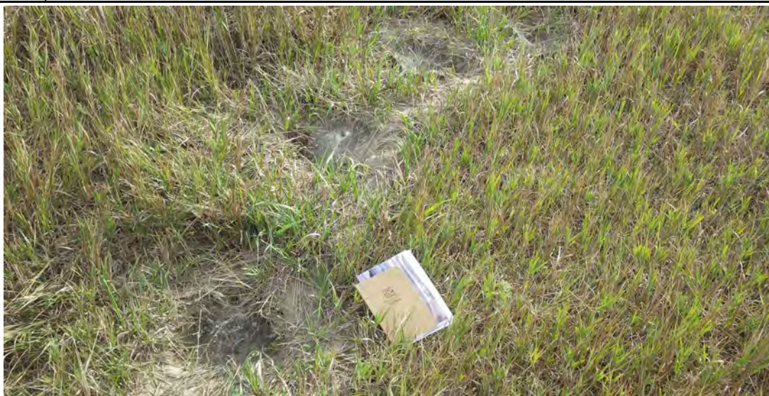
Photograph 8 (North perimeter berm downstream slope) Animal burrows (approximately 6 inches diameter) (IMGP7911.JPG)
