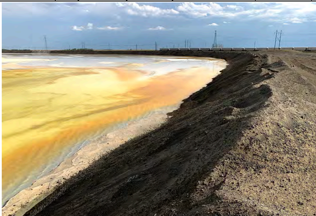
Photograph 20 (West CCR upstream slope) Upstream bottom ash slope and FGD material pool. (IMGP2793.JPG)
