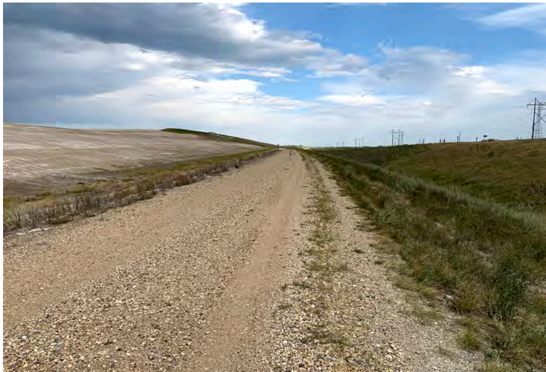
Photograph 25 (South perimeter berm crest) Perimeter berm crest, gravel road, good condition. (IMGP2803.JPG)
