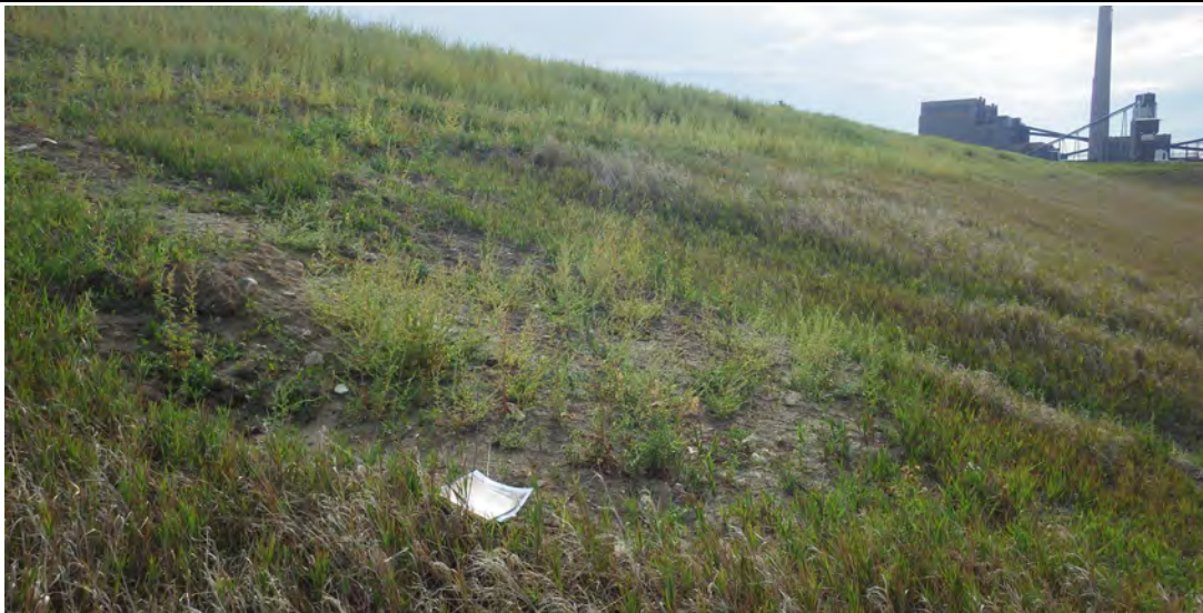
Photograph 9 (North perimeter berm downstream slope) Irregular grades from safety berm construction and weedy vegetation. (IMGP7912.JPG)
