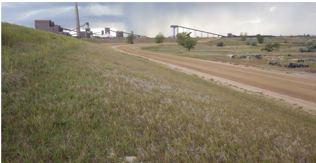
Photograph 15 (North perimeter berm downstream slope) Good vegetation on downstream slope. (IMGP7930.JPG)
