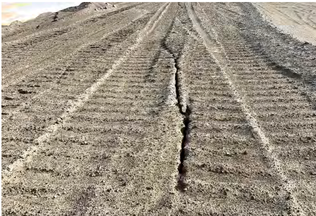
Photograph 21 (West CCR crest) Cracks in bottom ash on crest. (IMGP2795.JPG)
