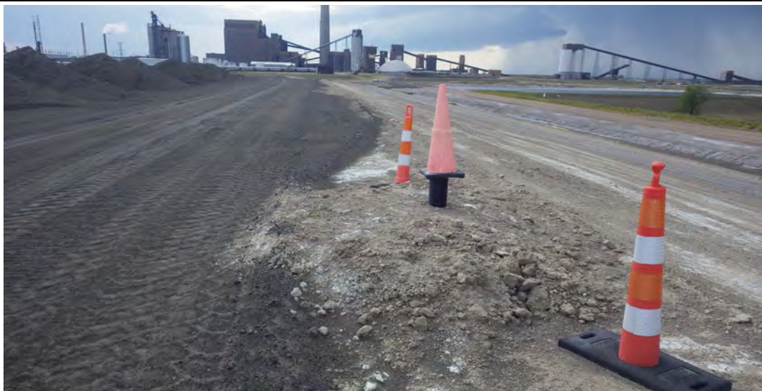
Photograph 11 (North CCR crest) Standpipe piezometer PZ-15, north side. (IMGP7914.JPG)
