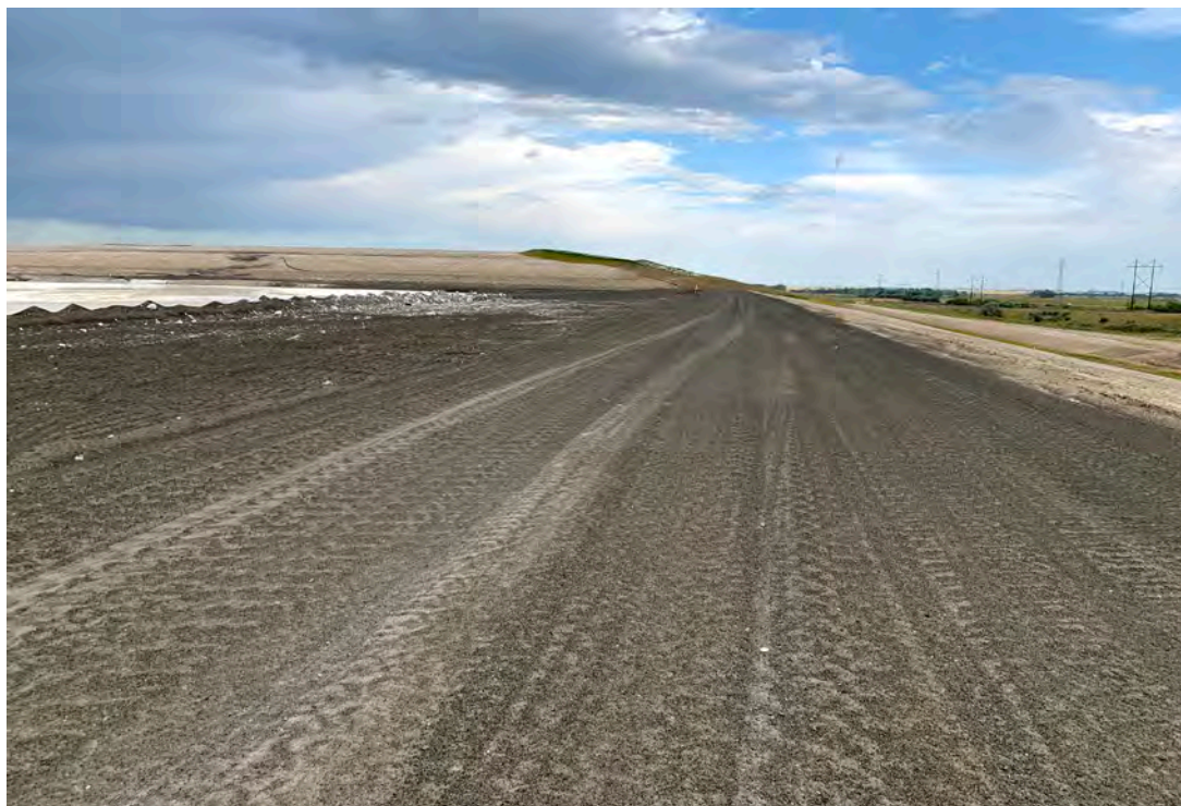
Photograph 27 (South CCR crest) Bottom ash crest, good condition. (IMG2805.JPG)
