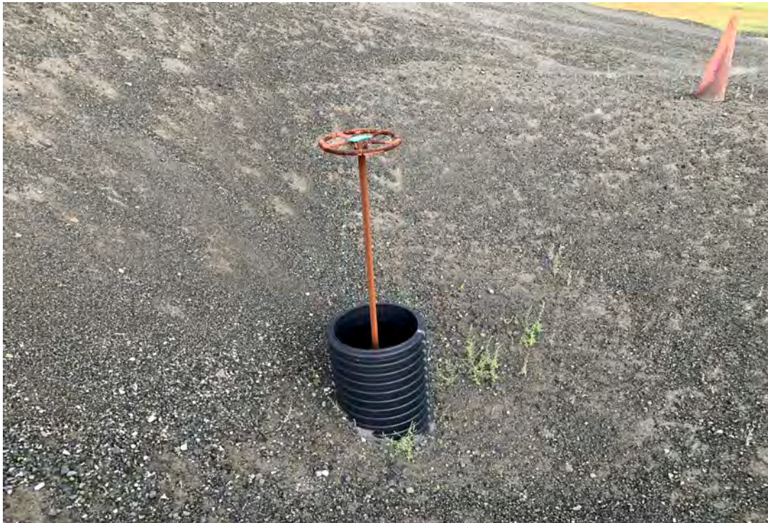
Photograph 29 (East CCR crest) Seepage piping isolation valve connection to Upstream Raise 92, good access via bottom ash placement. (IMGP2811.JPG)
