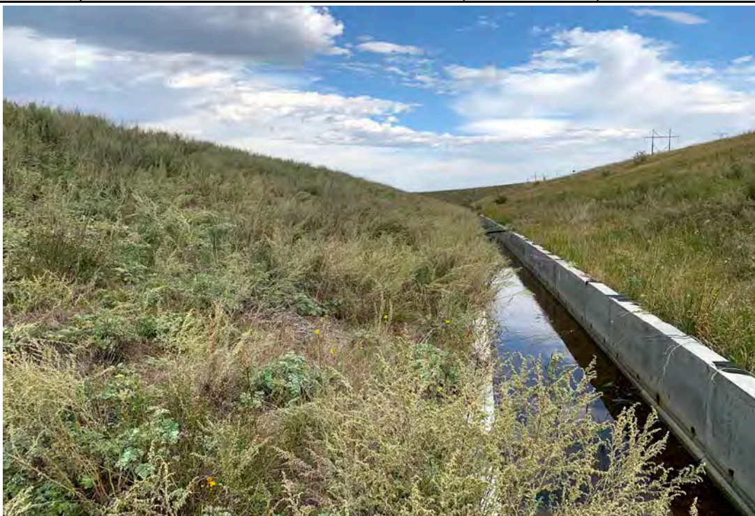
Photograph 24 (Southwest perimeter berm downstream slope and toe) Well-vegetated downstream slope and perimeter ditch concrete channel. (IMGP2802.JPG)
