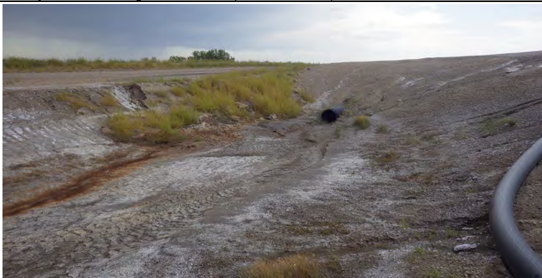
Photograph 14 (North CCR downstream slope) Culvert inlet from Upstream Raise 92 north perimeter ditch, free from obstructions. (IMGP7926.JPG)
