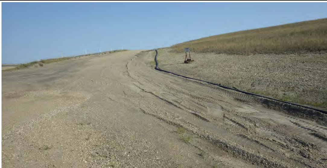
Photograph 11 (North haul ramp) Recent erosion repairs on inside of ramp (fly ash erosion), Upstream Raise 92 signage. (IMGP7960.JPG)
