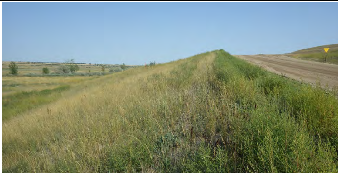
Photograph 10 (North perimeter berm downstream slope) Good grass vegetation on outer berm. (IMGP7957.JPG)
