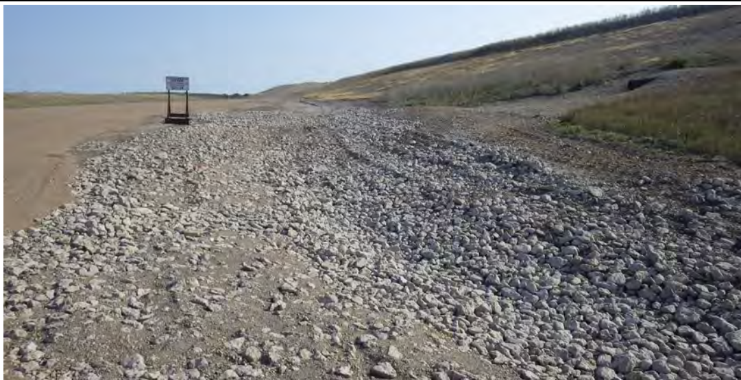
Photograph 19 (East CCR downstream slope) Concrete rubble erosion protection in good condition at bottom of east haul ramp. (IMGP7982.JPG)
