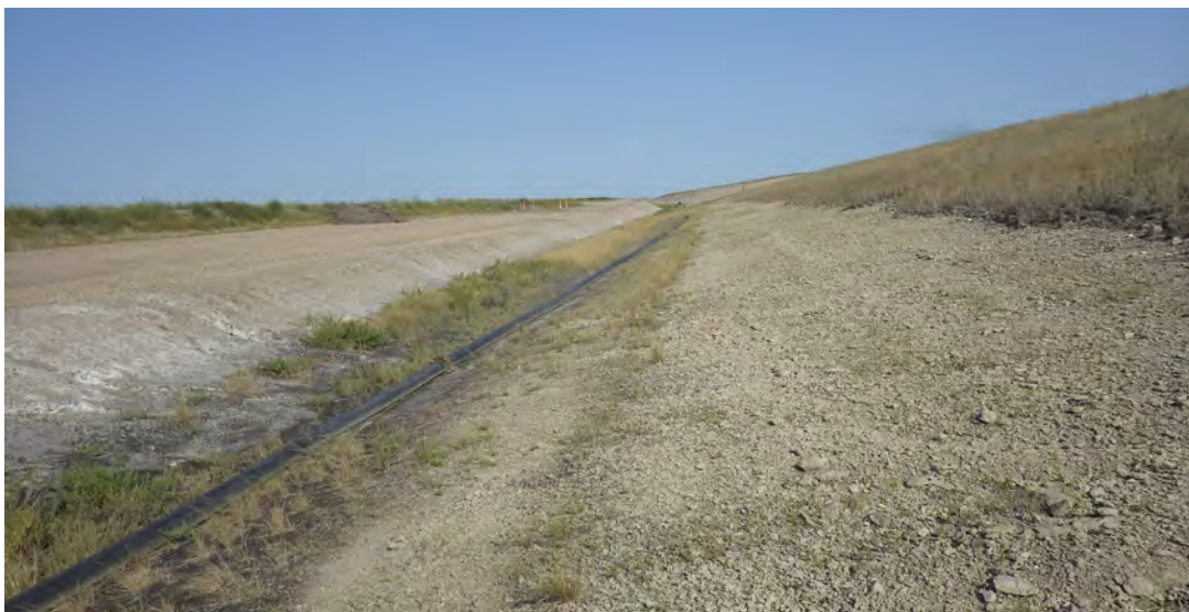
Photograph 7 (North CCR downstream slope (temporary cover) and perimeter berm upstream slope) Perimeter ditch and culvert to UR91, good condition. (IMG7951.JPG)
