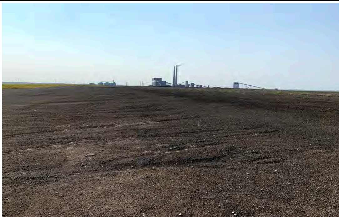
Photograph 28 (South CCR downstream slope) CCR and non-CCR waste placed as part of crown/cap above El. 1,998 ft. (IMGP2836.JPG)
