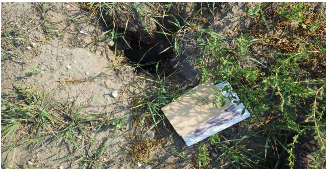
Photograph 14 (North CCR downstream slope (temporary cover)) Erosion of temporary cover, 1-2 feet deep. (IMGP7966.JPG)
