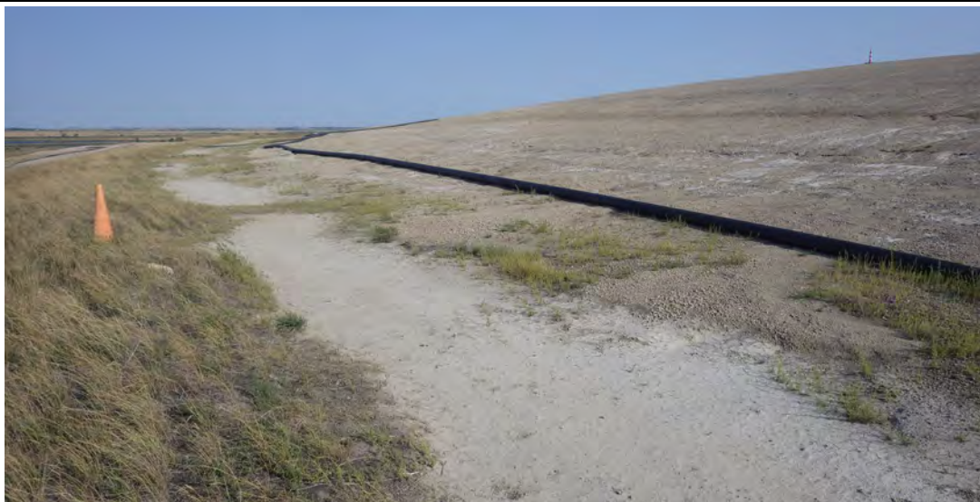
Photograph 17 (North CCR downstream slope) El. 1,974 ft bench and fly ash slopes above, minimal erosion. (IMG7976.JPG)
