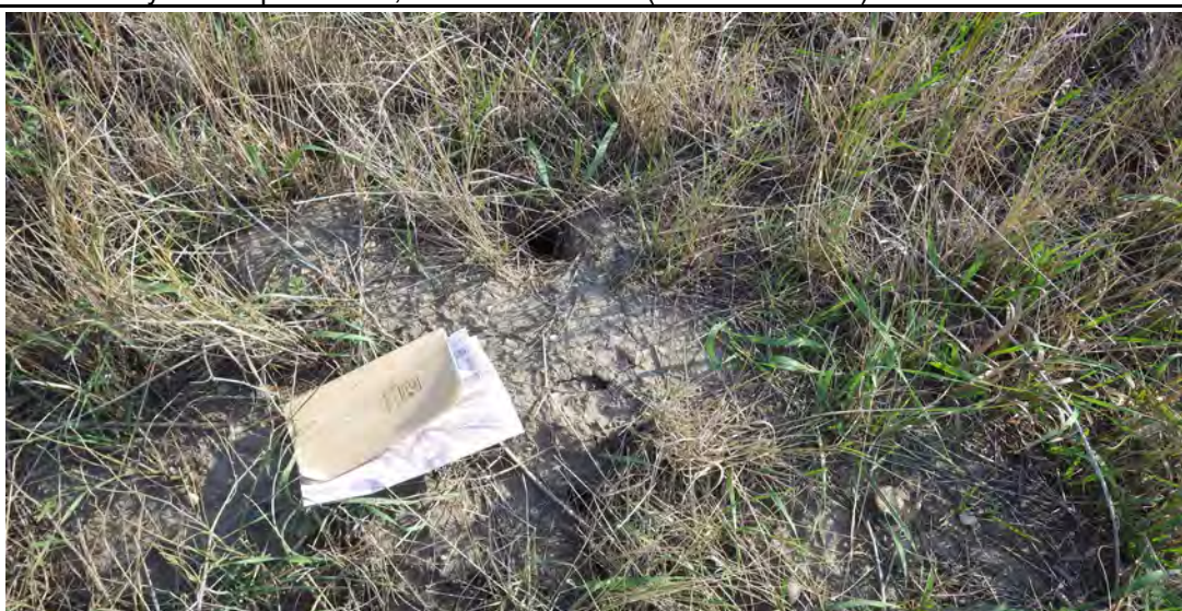
Photograph 18 (North CCR downstream slope (temporary cover)) Small animal burrow in temporary cover. (IMG7978.JPG)
