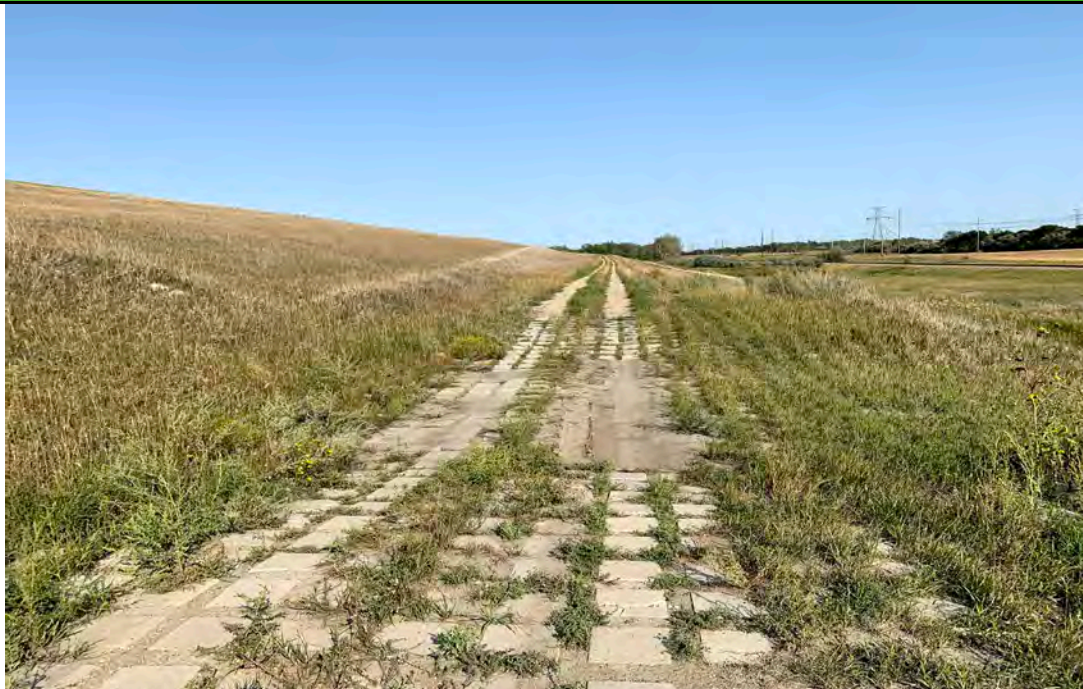
Photograph 31 (South perimeter berm crest) Downchute crossing the perimeter gravel access road. (IMGP2842.JPG)
