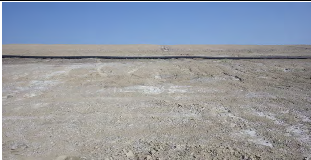
Photograph 4 (West CCR downstream slope) Minor erosion of fly ash slope above El. 1,974 ft bench. (IMGP7945.JPG)
