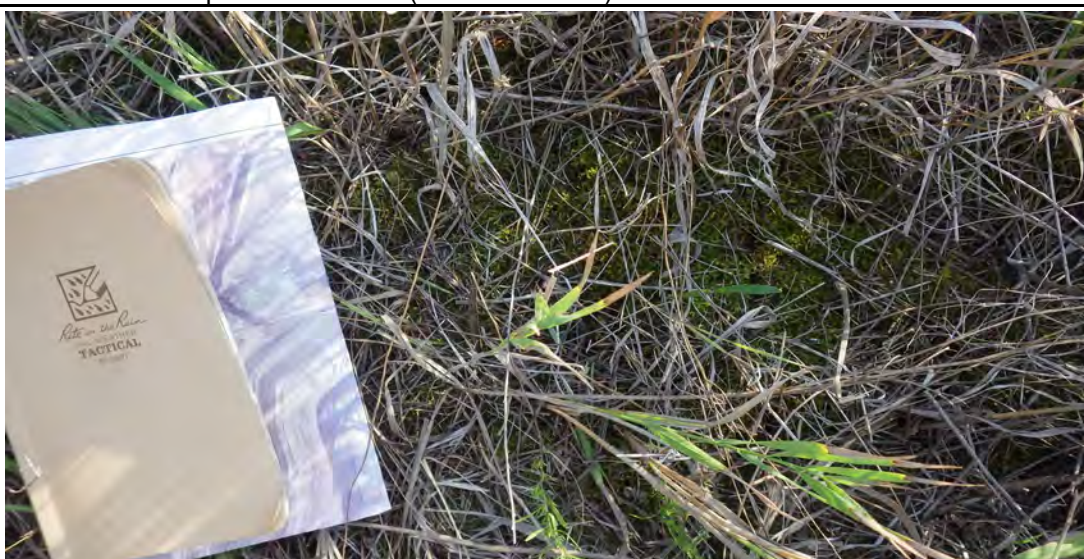
Photograph 16 (North perimeter berm downstream slope) Mossy area on north perimeter berm slope (slope is shaded most of the year) (IMGP7974.JPG)
