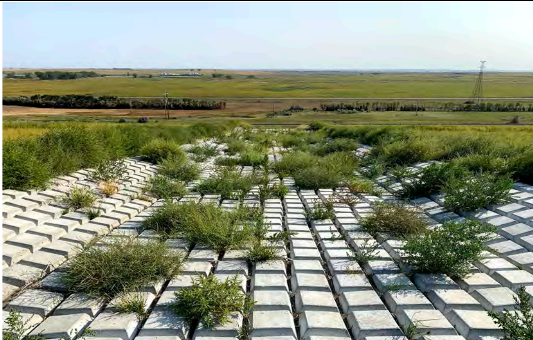
Photograph 29 (South CCR downstream slope (final cover)) Southeast downchute channel, good condition. (IMG2838.JPG)
