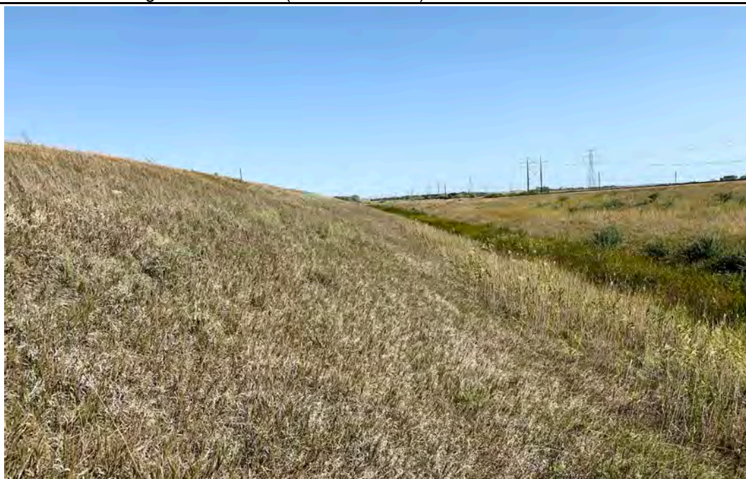
Photograph 22 (South perimeter berm downstream slope) Perimeter berm downstream slope and toe, good condition and well vegetated. (IMG2824.JPG)
