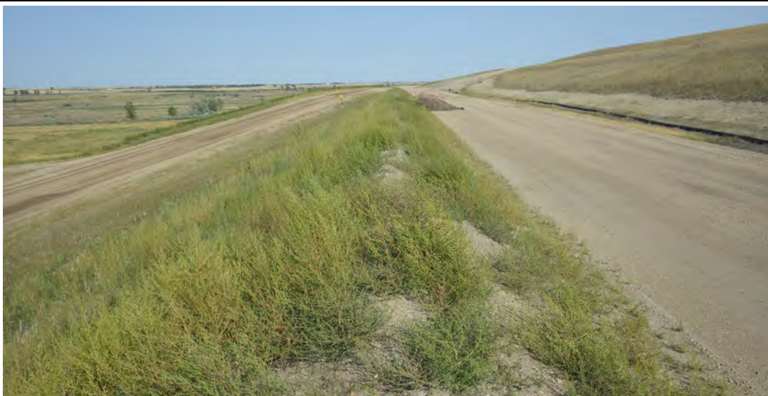
Photograph 8 (North perimeter berm crest and downstream slope) North haul road safety berm, good condition with weedy vegetation. (IMG7953.JPG)
