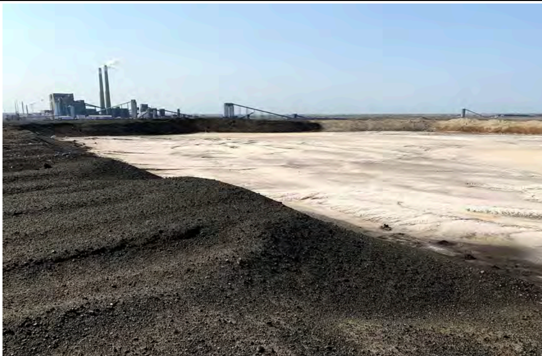
Photograph 25 (CCR upstream slopes) Remaining exposed FGD material and placement of crown CCR material. (IMGP2832.JPG)
