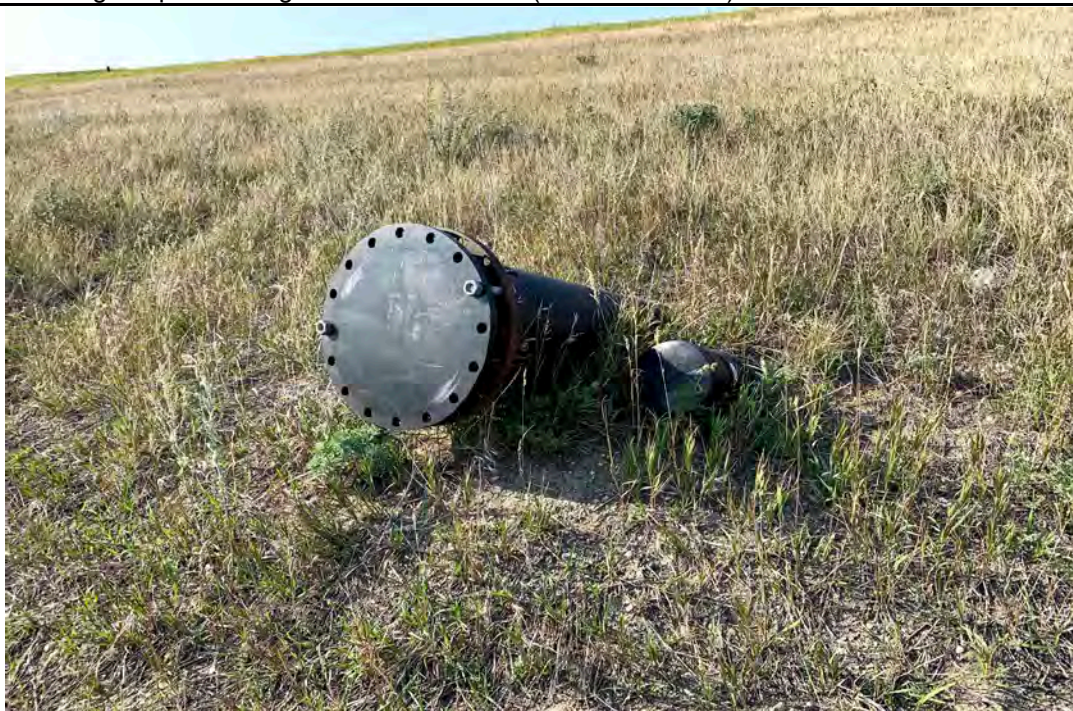
Photograph 32 (South CCR downstream slope (final cover)) Sump riser and cleanout piping. (IMGP2843.JPG)
