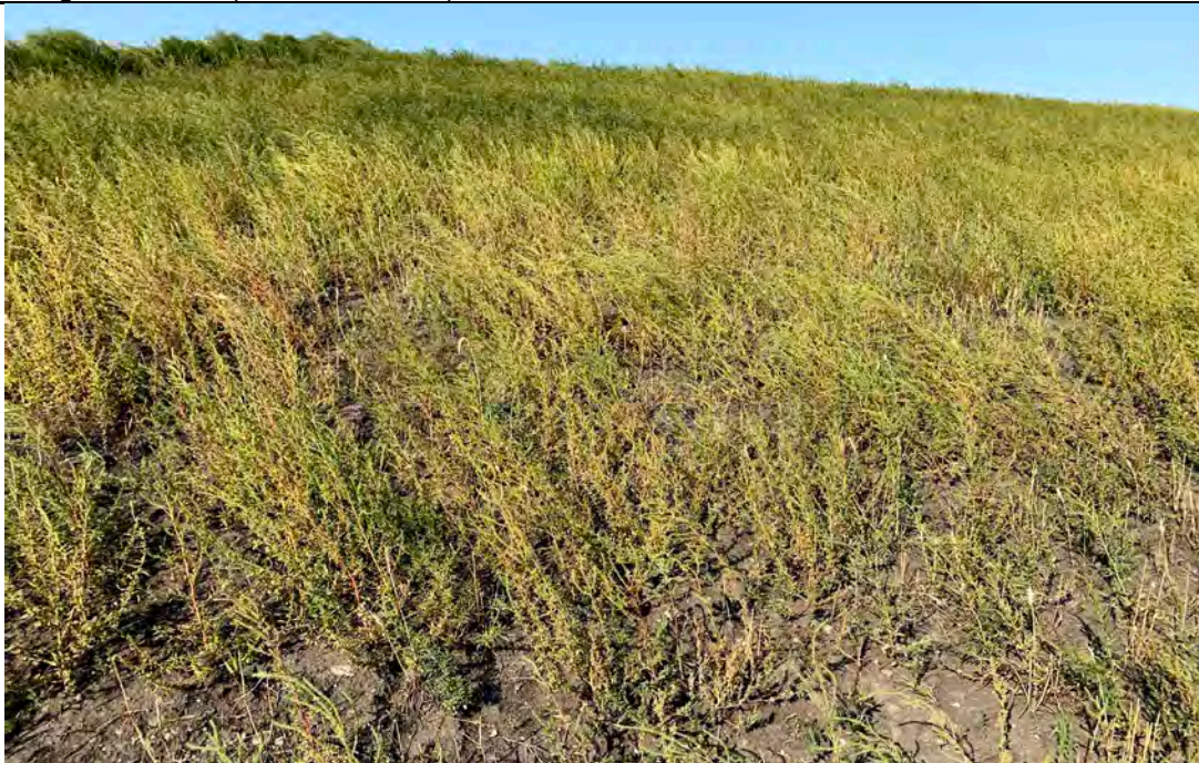
Photograph 24 (South CCR downstream slope (final cover)) Predominately weeds in final cover placed in 2020 (El. 1,974 ft to El. 1,998 ft). (IMGP2827.JPG)
