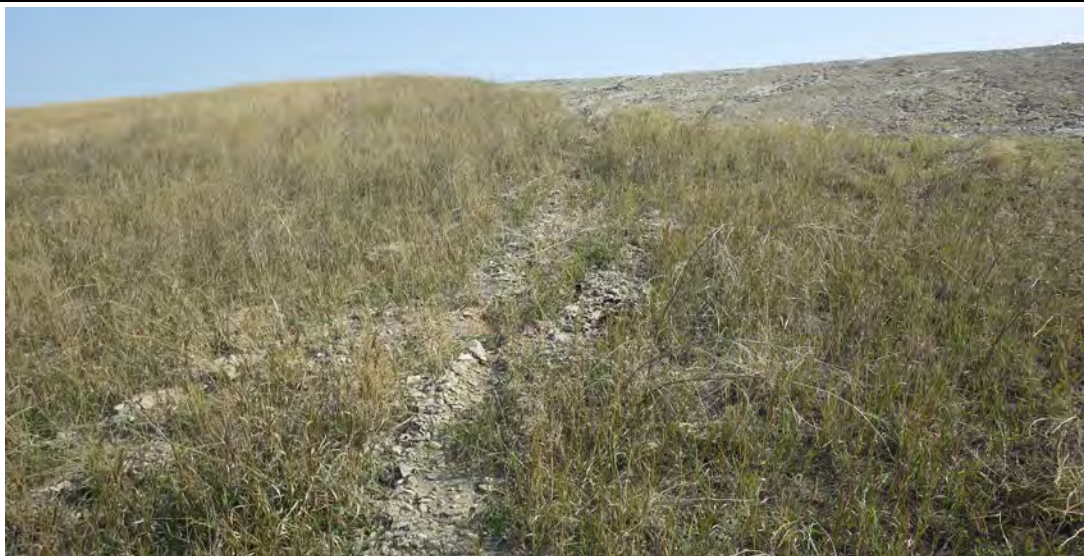
Photograph 5 (North CCR downstream slope (temporary cover)) Minor fly ash erosion onto temporary cover. (IMG7949.JPG)
