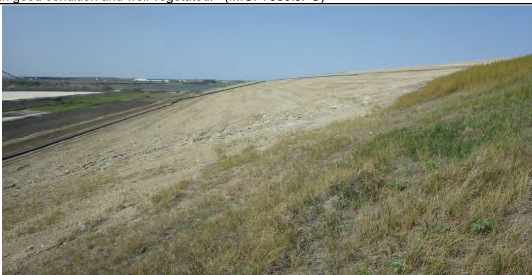
Photograph 2 (West CCR downstream slope) Minor fly ash erosion. (IMGP7940.JPG)
