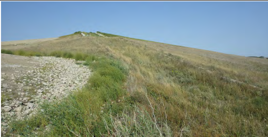
Photograph 1 (Southwest perimeter downchute) Downchute in good condition and well vegetated. (IMGP7939.JPG)
