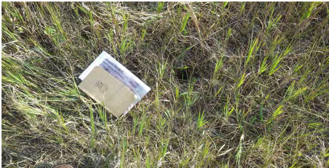
Photograph 9 (North perimeter berm downstream slope) Small animal burrow (typical). (IMGP7954.JPG)
