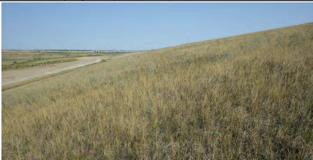
Photograph 6 (North CCR downstream slope (temporary cover)) Temporary cover, well vegetated. (IMG7950.JPG)
