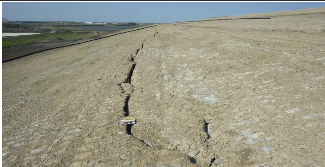
Photograph 3 (West CCR downstream slope) Crack in fly ash CCR downstream slope below El. 1,974 ft bench (4-6 inches wide inside offset a little lower than outside). (IMGP7941.JPG)
