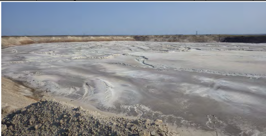
Photograph 20 (CCR upstream slopes) Remaining exposed FGD material and placement of crown CCR material. (IMGP7984.JPG)
