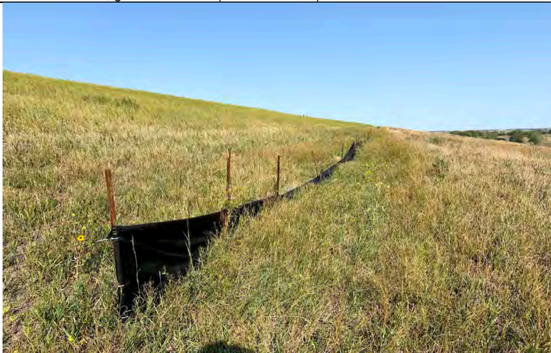
Photograph 30 (South CCR downstream slope) Silt fence downgradient of final cover installed in 2020, fair condition. (IMG2840.JPG)
