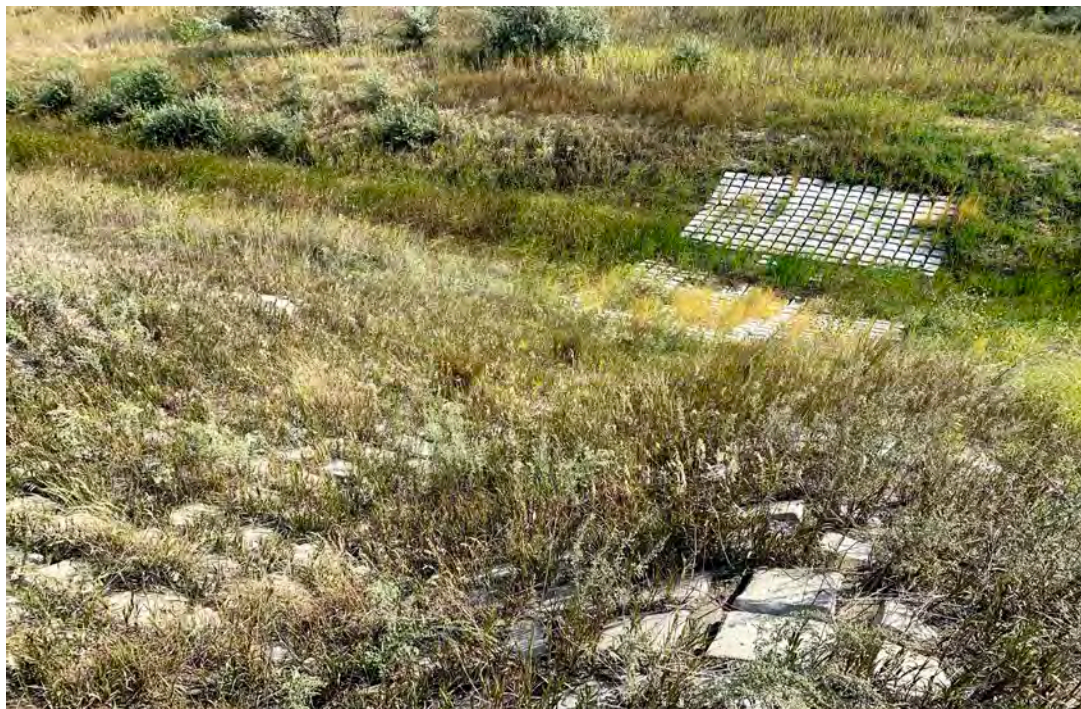
Photograph 21 (Southwest downchute and hydraulic jump basin) Articulated concrete block in good condition. (IMG2823.JPG)
