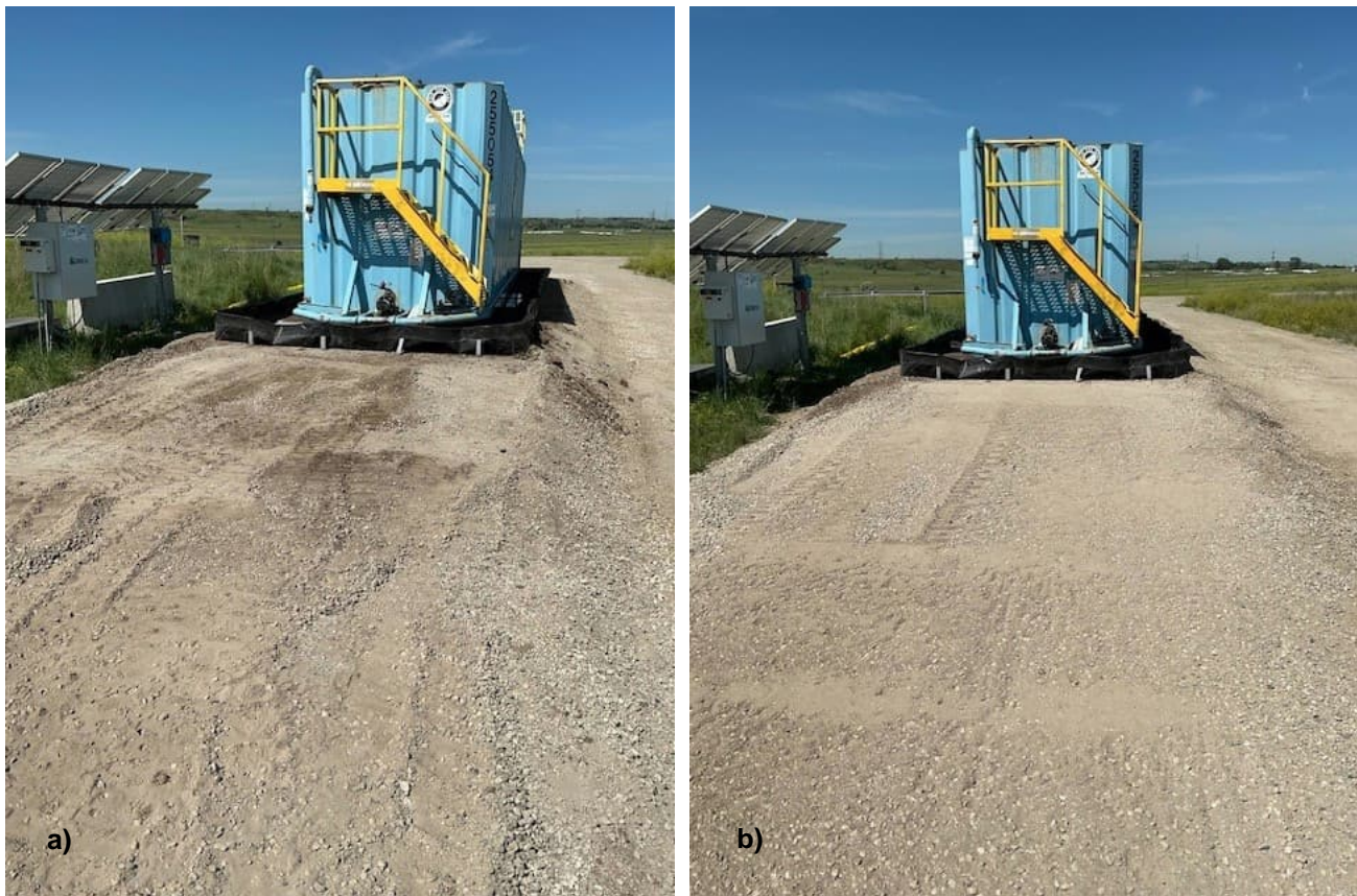
Figure 4: Impacted area east of the Bottom Ash Impoundment tank looking west a) after excavation of impacted tank pad earth materials and b) after backfilling and regrading activities.
