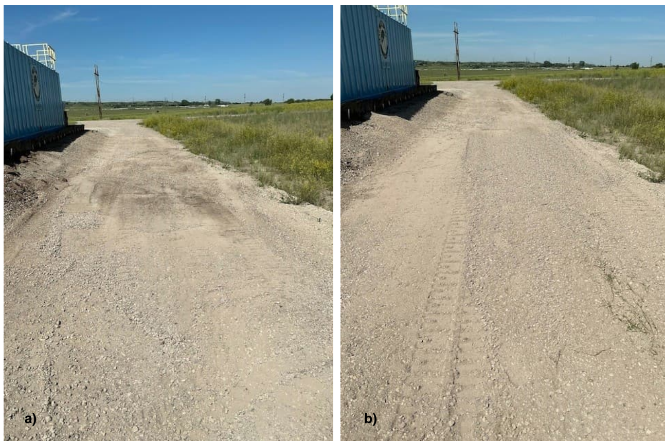
Figure 5: Impacted roadway area north of the Bottom Ash Impoundment tank looking west a) after excavation of impacted roadway earthen materials and b) after backfilling and regrading activities.
