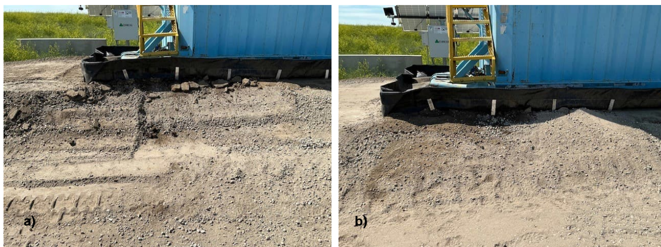
Figure 6: Impacted tank pad earth materials excavated northeast and beneath the tertiary spill containment barrier a) after excavation of earthen materials and b) after backfilling and regrading activities.
